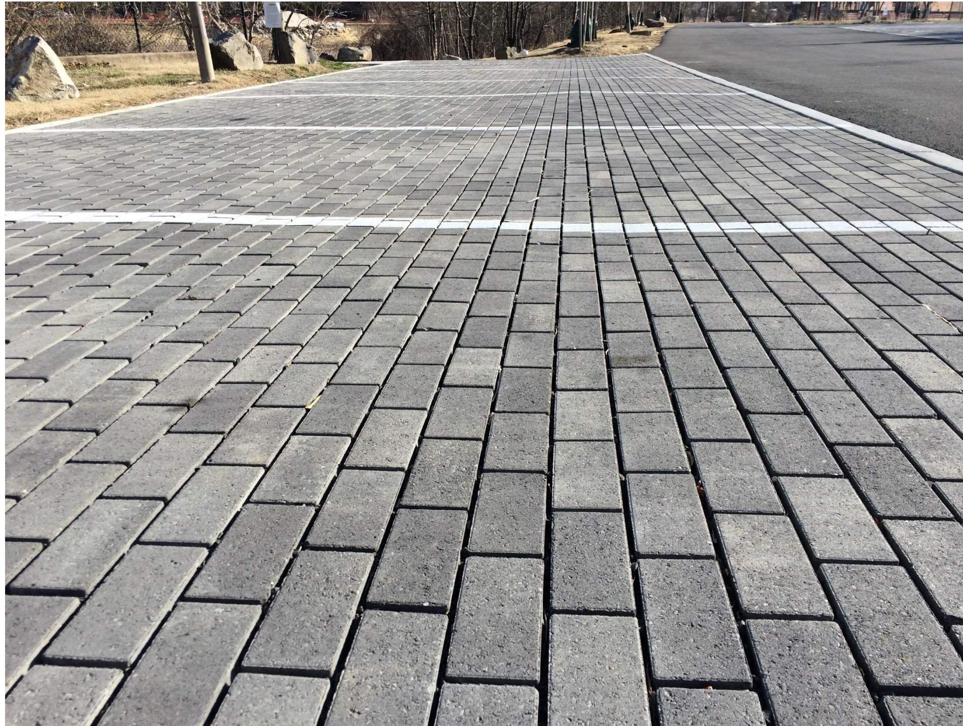
Permeable Pavers, Four Mile Run Park
