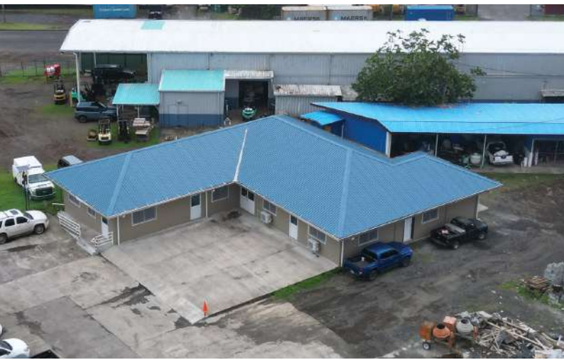
Parks & Recreational Office Renovation- Office Improvements
