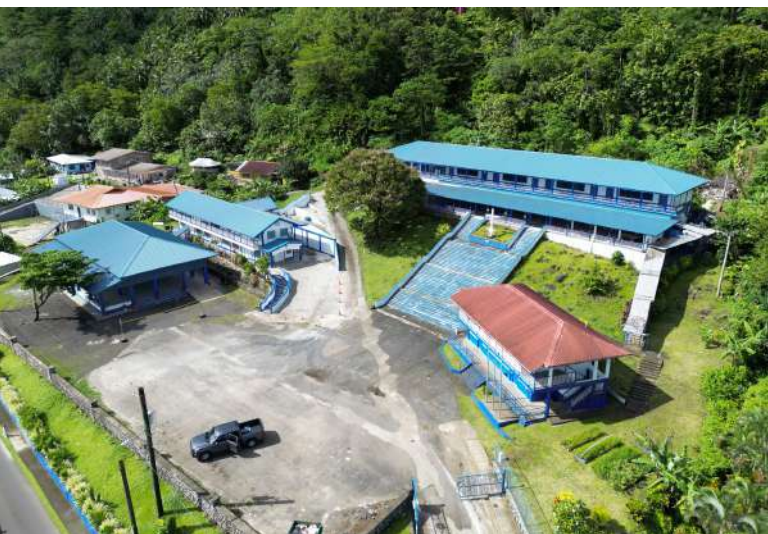
Marist St. Francis ES- Classroom Improvements
