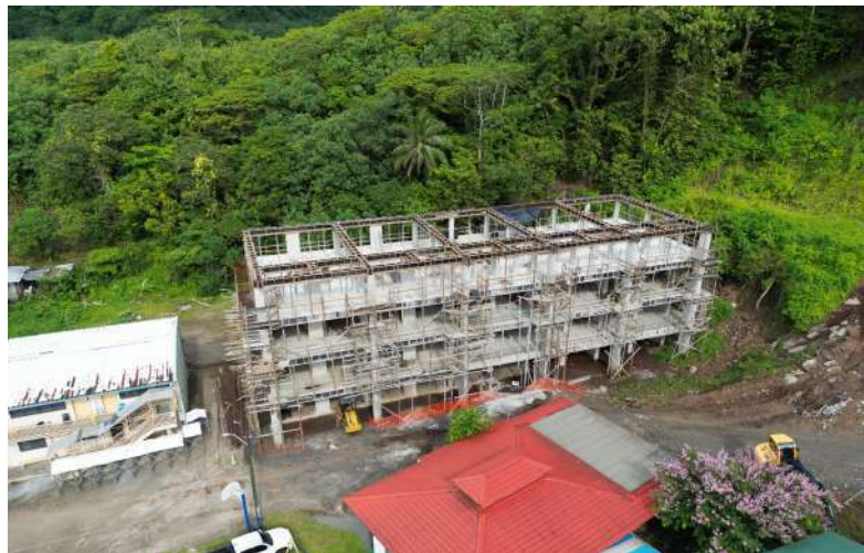
Manumalo Junior & Secondary Academy- 23 Classroom Extension Project
