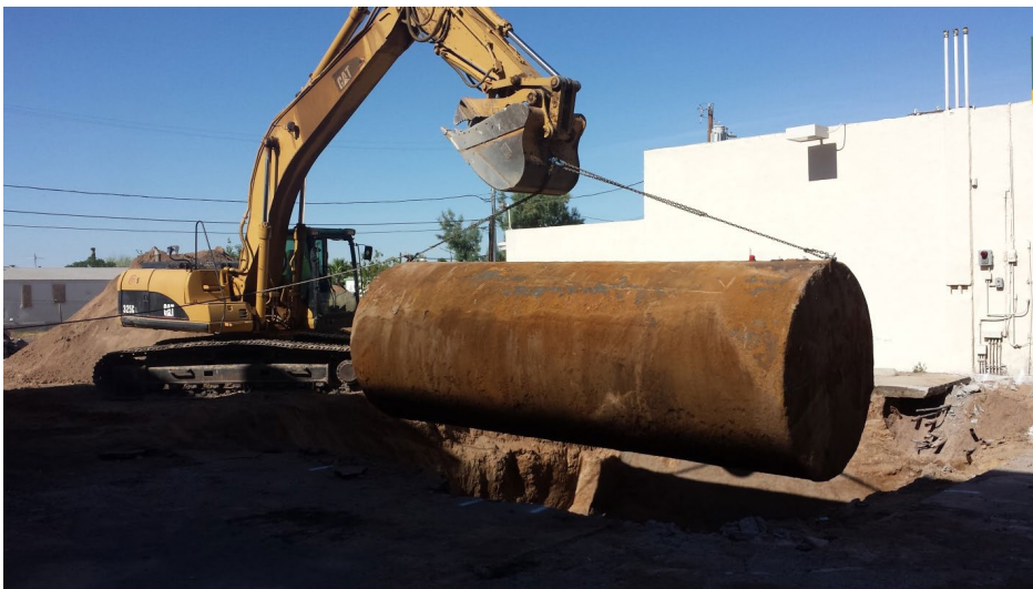
Removal of an underground storage tank
