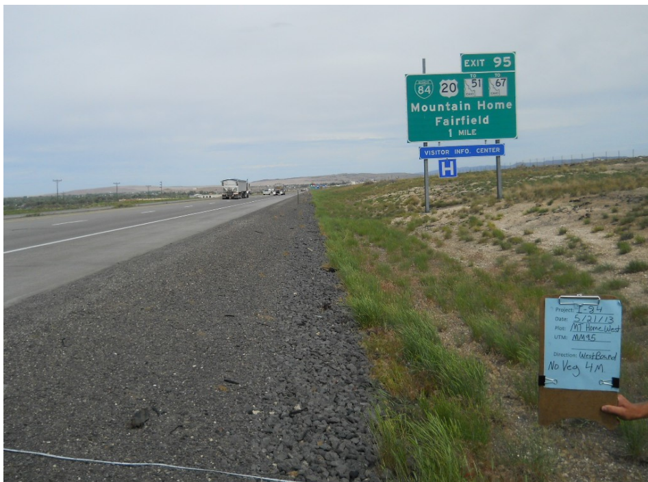
Area along Interstate 84 (MM 95) with enlarged gravel apron to decrease roadside fire potential. Gravel apron improvements have significantly contributed to reducing the number of fire starts.
