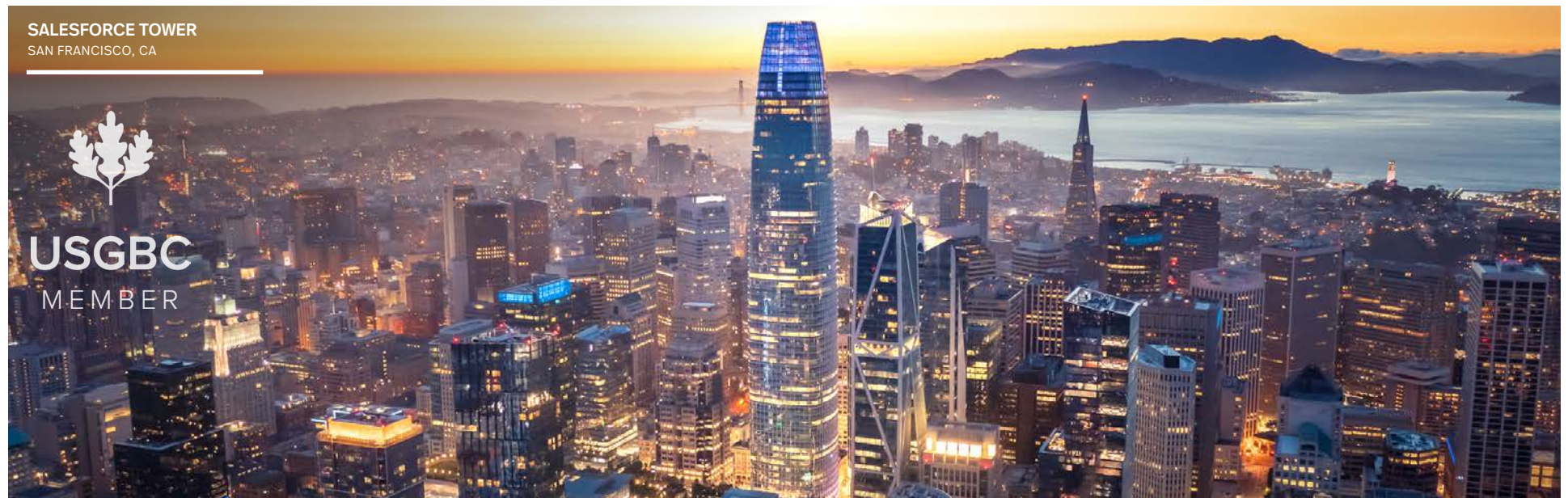
A FORCE TO BE RECKONED WITH | A grand symbol of BXP’s responsible growth and capacity to execute smart, sustainable development. Salesforce Tower is a high performance workspace designed to promote the health and wellbeing of its inhabitants. At 1.4 million square feet, the 61-story tower at the former Transbay Transit Center in the South of Market neighborhood was the first in San Francisco to be pre-certified at the LEED Platinum level.
