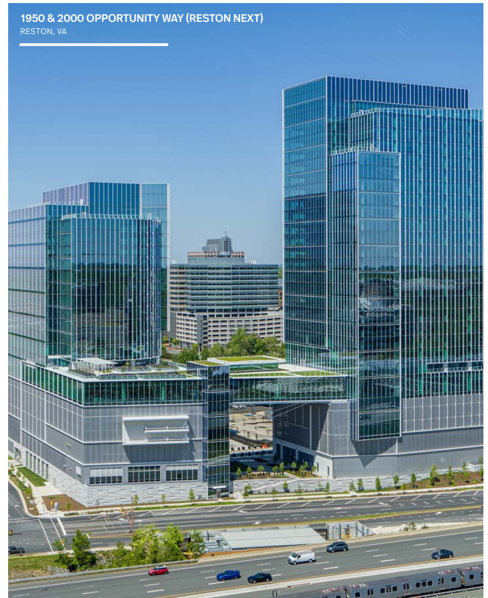
TRANSIT-ORIENTED DEVELOPMENT | Completed in 2022, 1950 & 2000 Opportunity Way (Reston Next) is a grand example of transit-oriented development. The buildings were constructed adjacent to the Reston Town Center Silver Line Metro Station, multiple Reston Town Center bus stops, and are located less than 1/4 mile from the Washington and Old Dominion bicycle trail. The development also includes 200 secure bicycle storage spaces and 125 EV charging stations.
