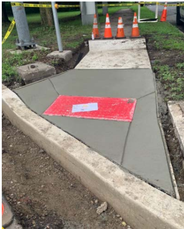
Figure 2: Concrete curb ramp installation
