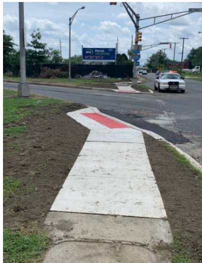
Figure 1: Concrete curb ramp installed
