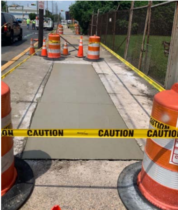
Figure 4: Concrete sidewalk installation
