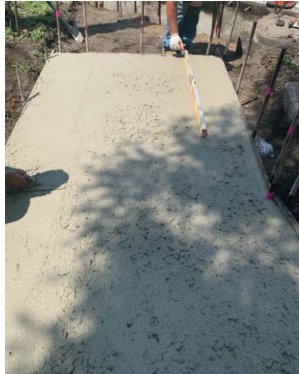
Figure 5: Concrete placement
