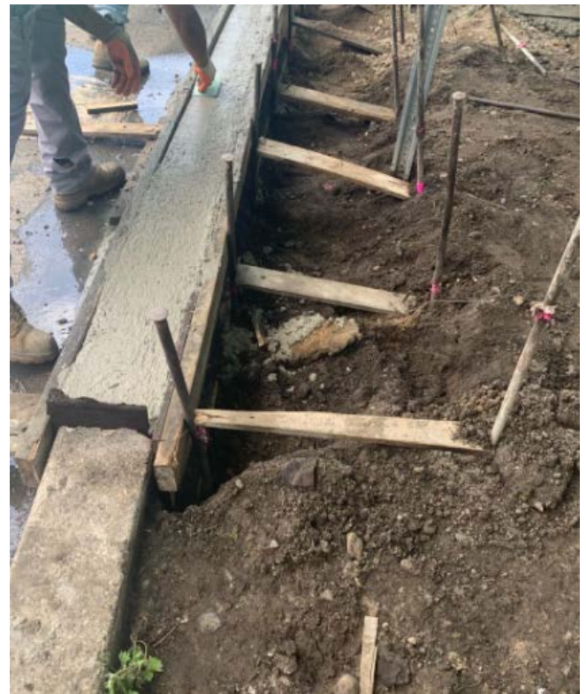
Figure 3: Concrete curb installation
