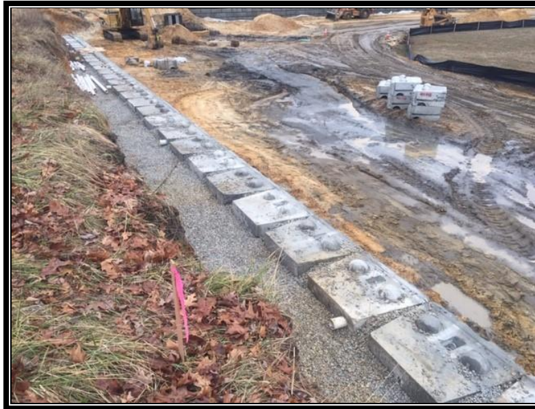
Figure 2: Crew backfilling REDI-ROCK retaining wall block with No.57 stone..
