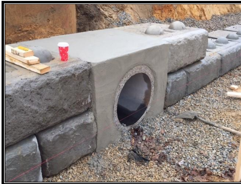
Figure 3: Contractor formed and poured the concrete collar around the existing R.C.P.
