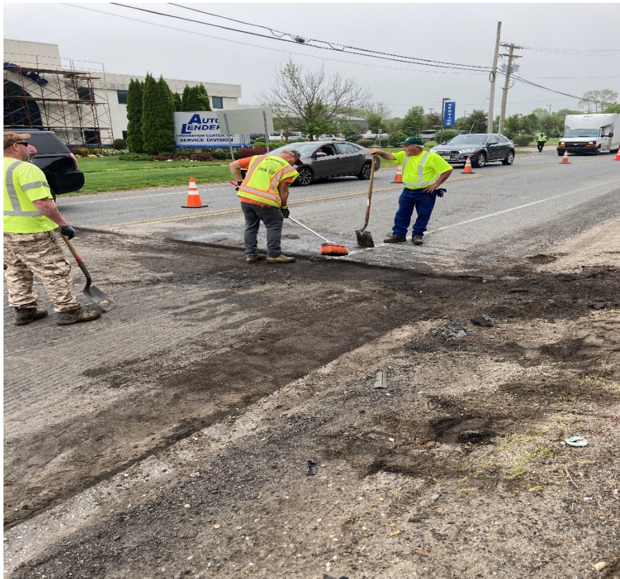
Figure 1: Contractor cut edge prior to 12.5M Hot Mixed Asphalt Top Coat.
