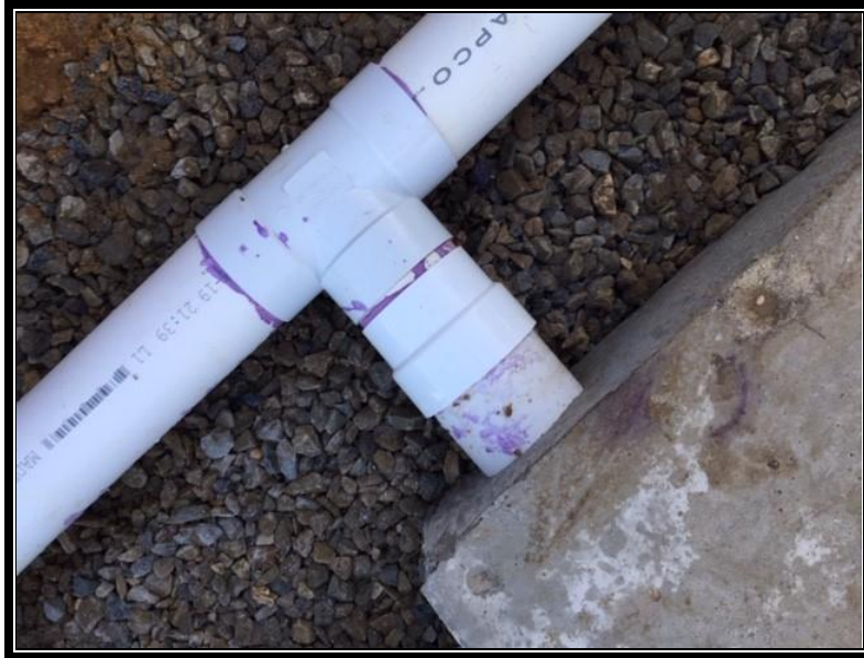
Figure 2: Crew installing PVC under drain pipe behind the wall.
