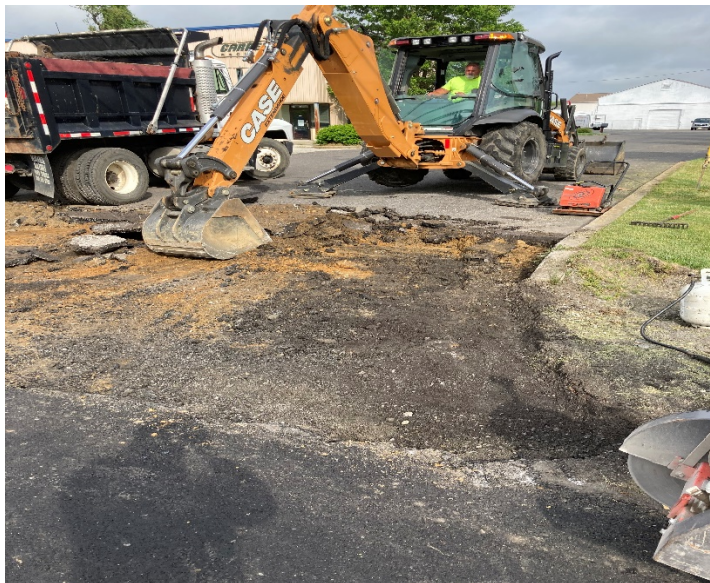
Figure 7: Contractor prepped driveway for Hot Mixed Asphalt.
