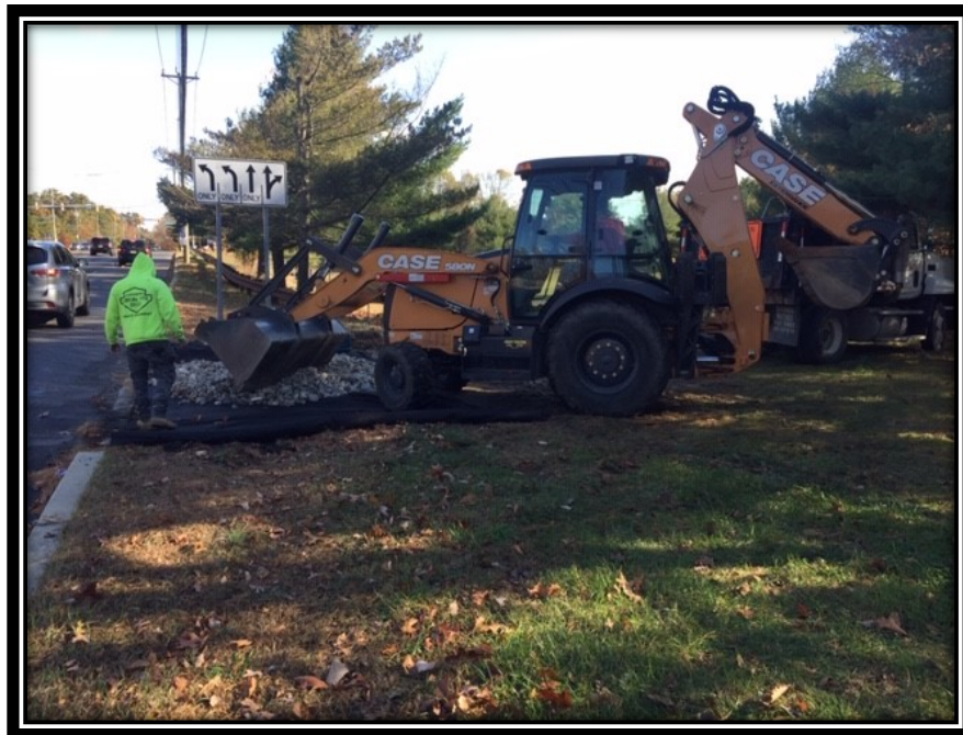
Figure 1: Crew installing stone construction entrance
