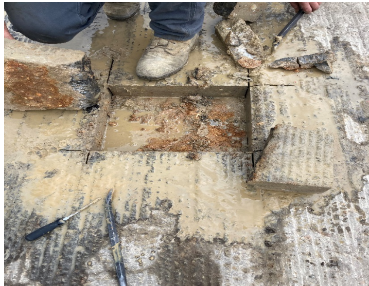
Figure 4&5: A test patch was saw-cut and approximately 4" of cement was revealed.
