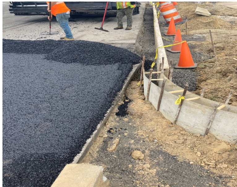
Figure 6: 12.5M HMA intermediate added Northbound sections 155-161.
