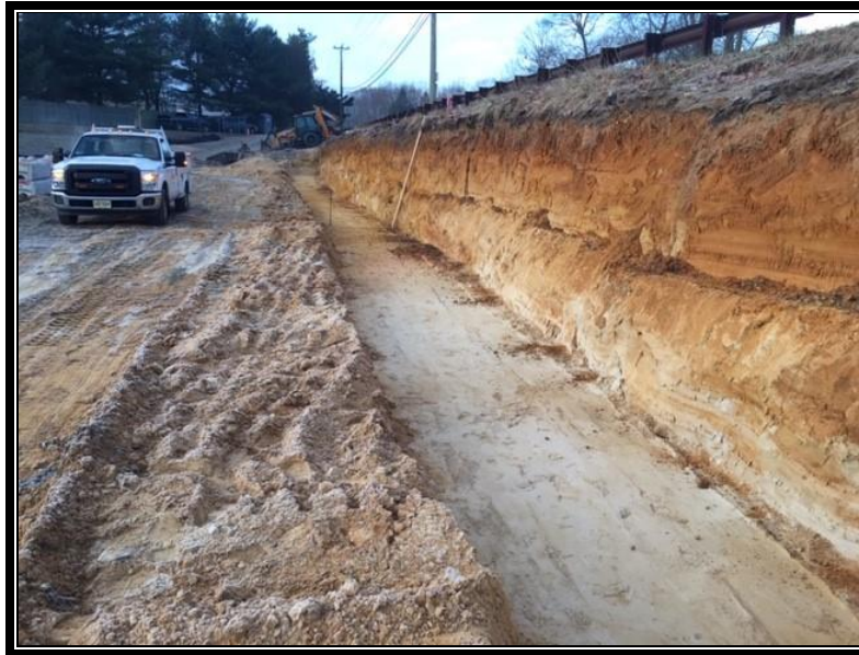
Figure 2: Crew excavating the footing for the west retaining wall..
