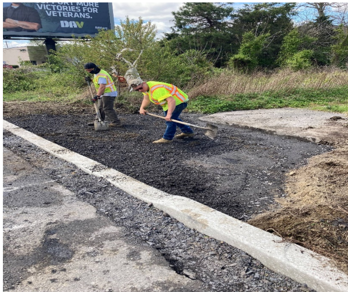
Figure 5&6: Concrete poured and backfilled.
