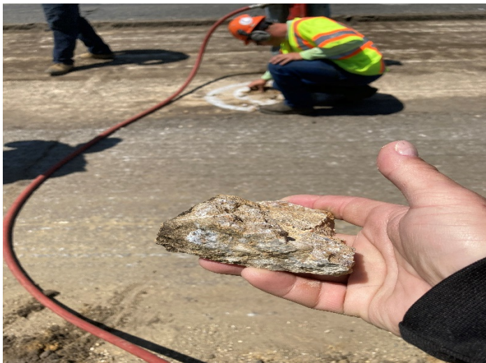
Figure 3: A test patch was removed to identify the material.
