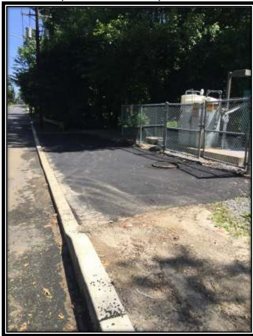
Figure 1 HMA Apron Cherry Hill Township Pump Station
