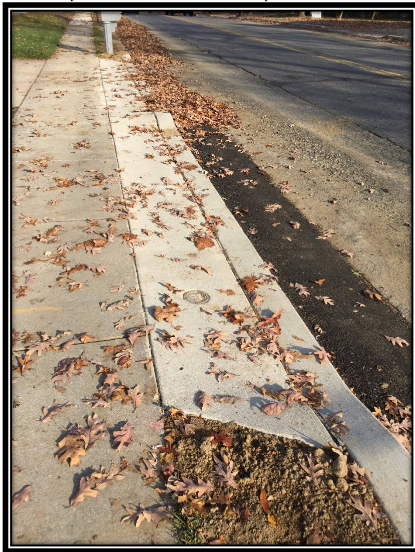
Figure 1 Concrete Aprons STA 120+50 Coles Road (LS)
