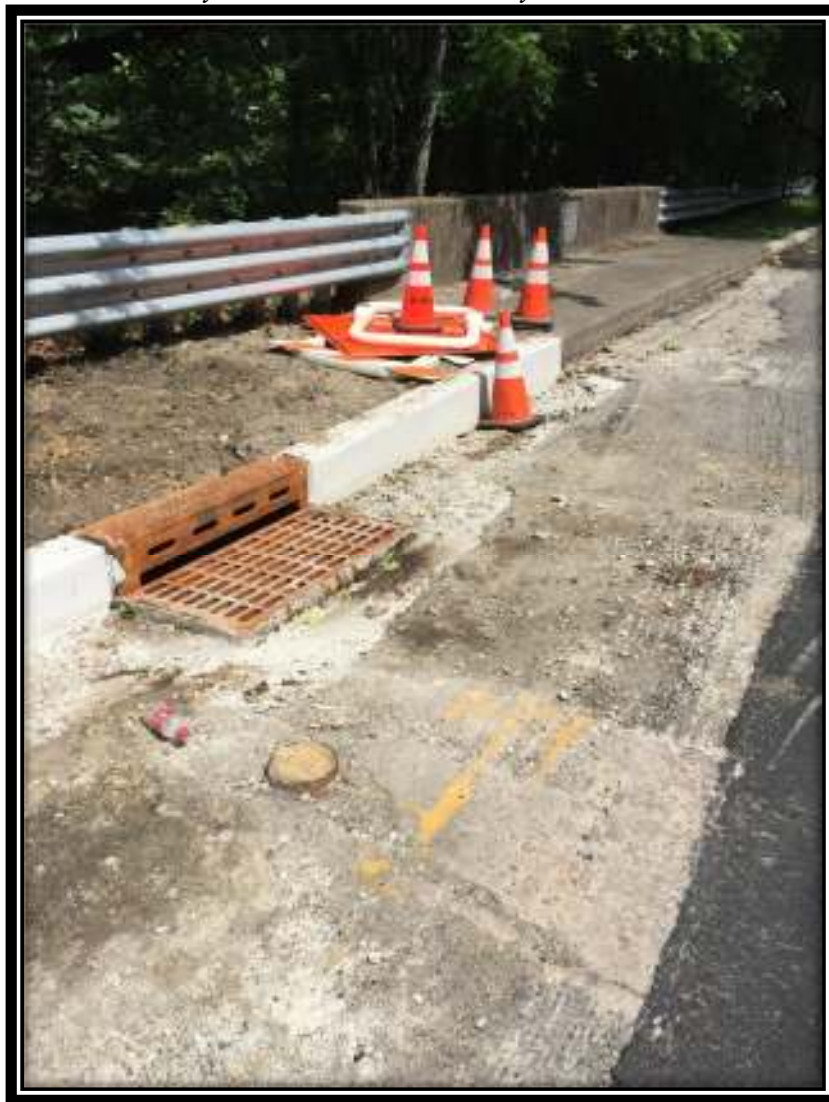
Figure 1 New Curb and ECO Type B Casting
