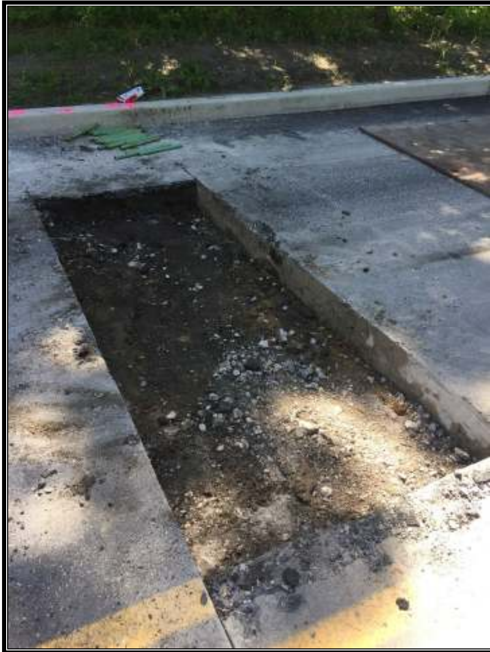
Figure 3 Excavation for Typical Concrete Base Repair
