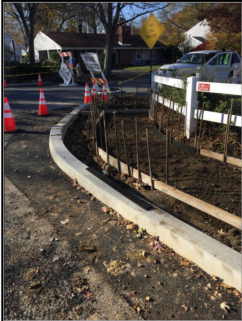
Figure 2 Concrete Curb & Formed Sidewalk & Handicap Ramp at Hassemer Road (LS)
