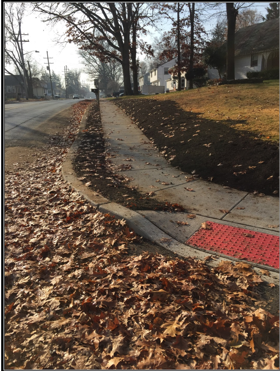
Figure 2 Concrete Sidewalk & Handicap Ramp at Dellwood Road (LS)
