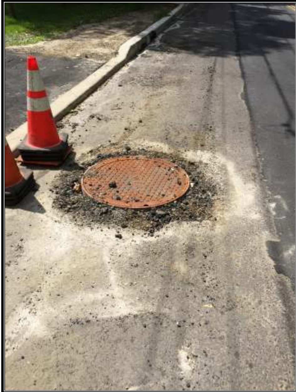
Figure 2 New Reset Manhole Casting
