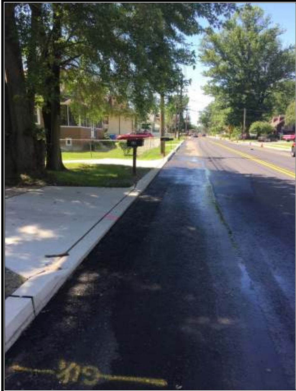
Figure 2 Base Install along Shoulder and Leveling with Temporary Striping
