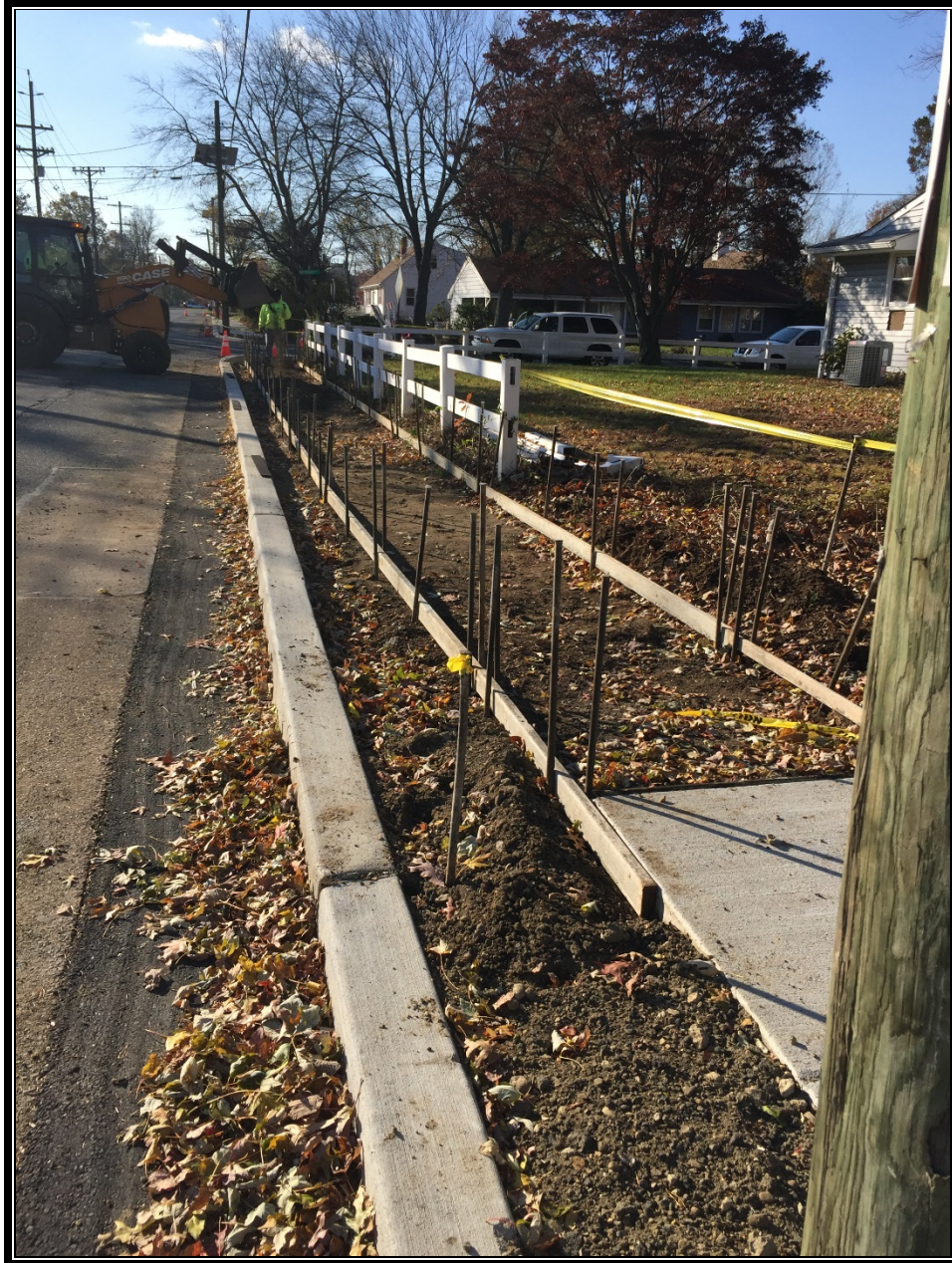
Figure 3 Concrete Curb & Formed Sidewalk Hassemer Road to STA 116+25 (LS)
