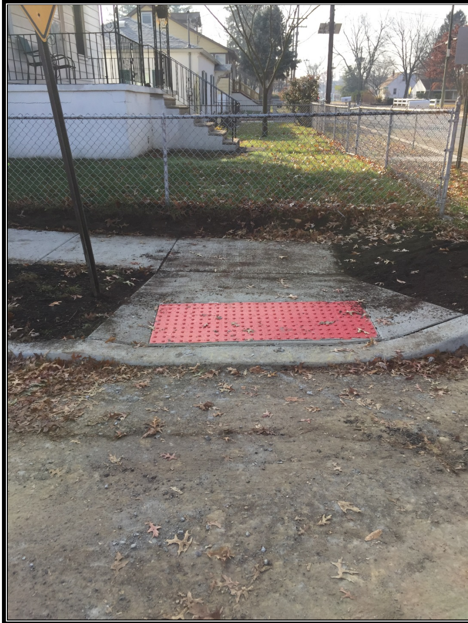
Figure 3 Handicap Ramp at Hassemer (East) STA 117+61 (RS)
