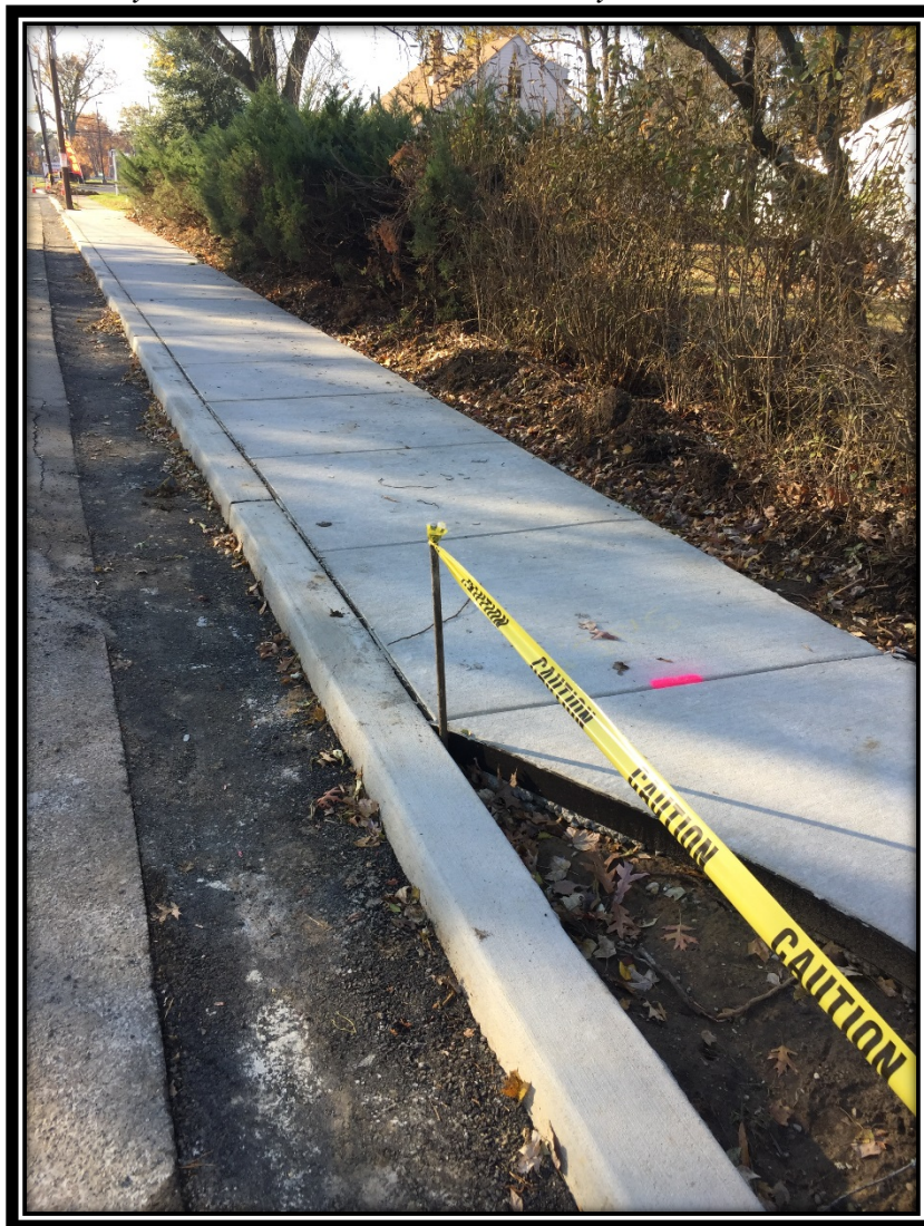
Figure 1 Concrete Curb & Concrete Sidewalk STA 113+25 to Hassemer Road (LS)
