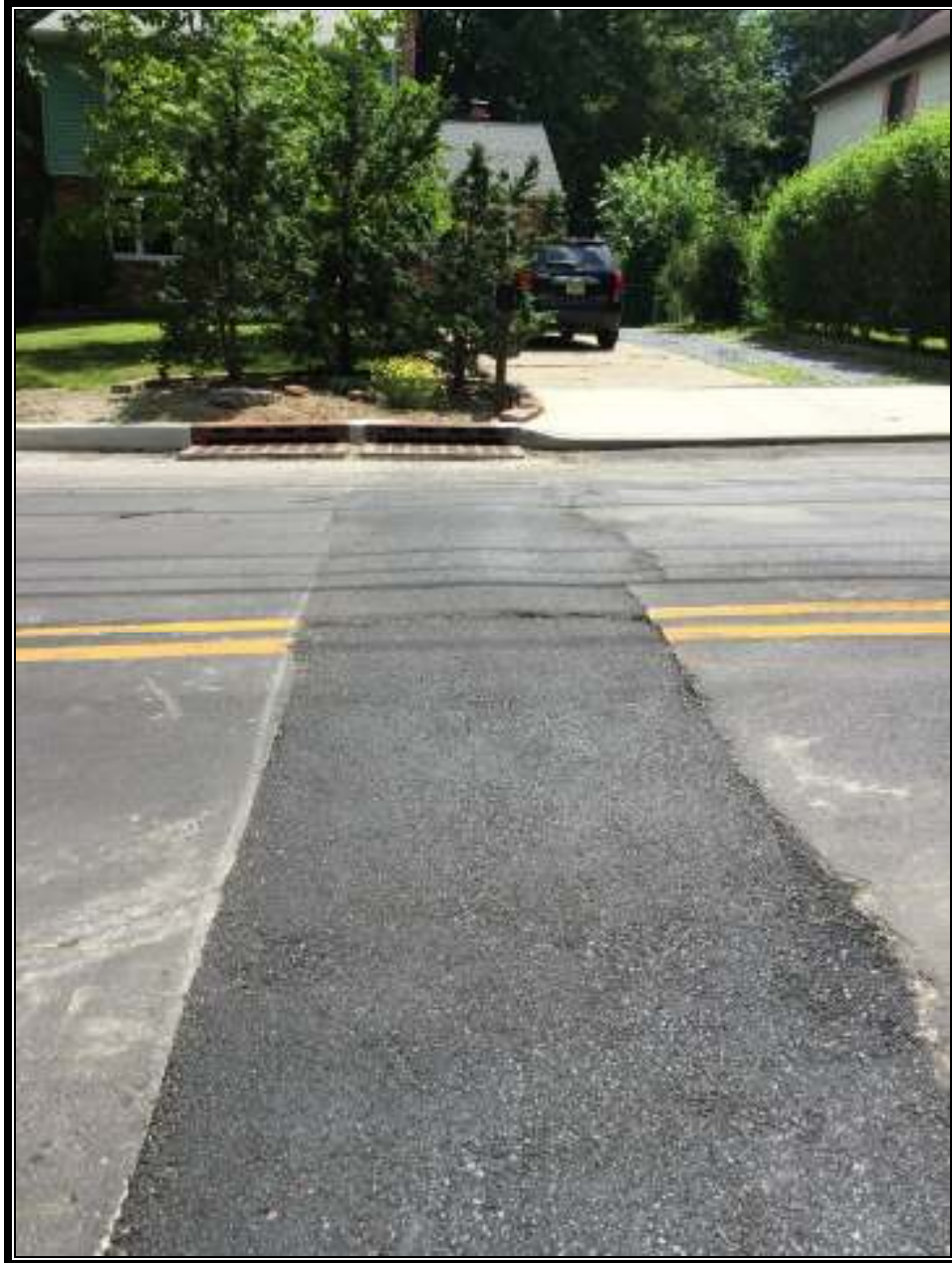
Figure 3 Concrete Joint Repair
