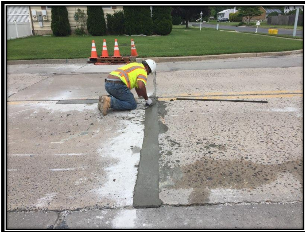
Figure: 1 – Partial depth concrete slab repairs in the northbound lane approaching the intersection with Lee Lane
