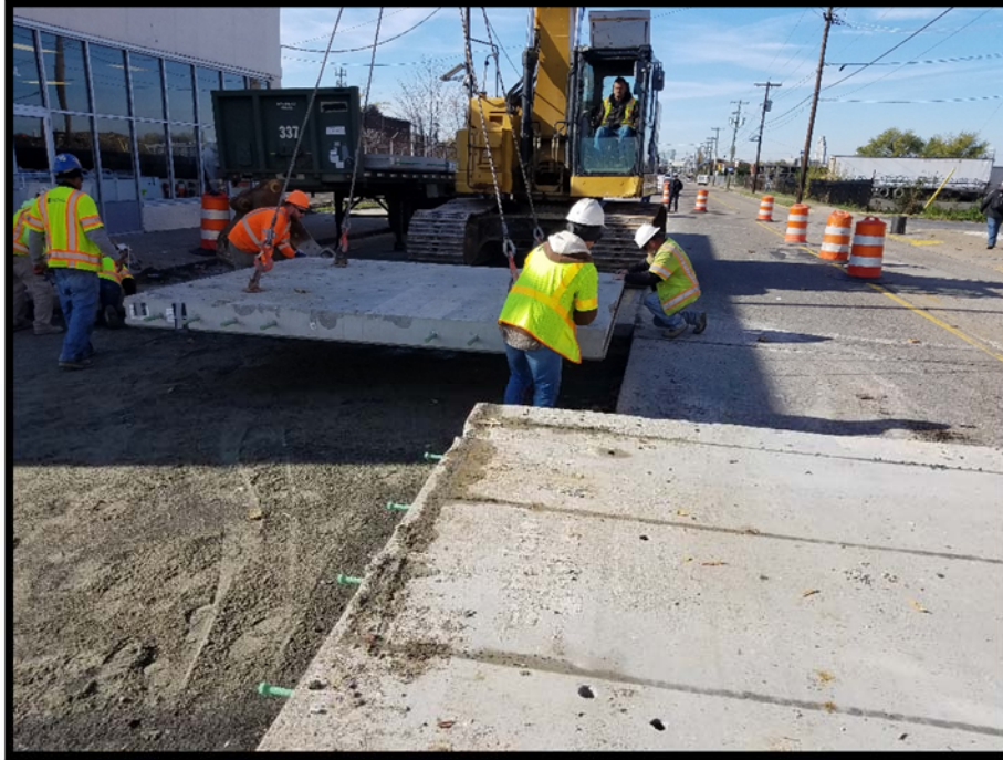
New precast reinforced concrete slab being lowered into place.
