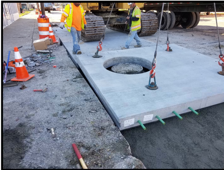
Slab #K38 being lowered into place around reset manhole casting.
