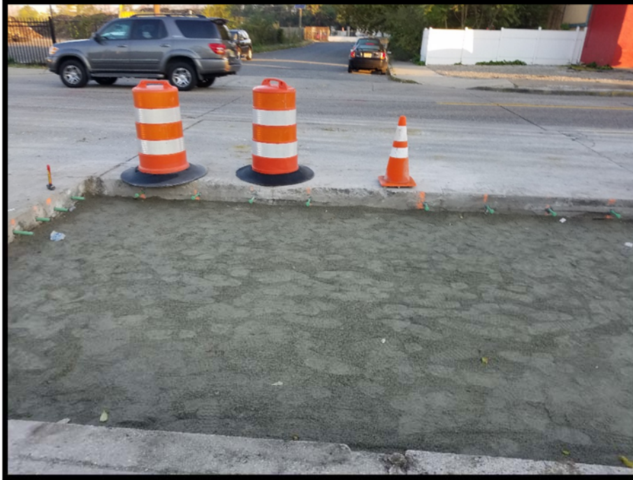
Subbase prepared, dowels installed, ready for precast slab to be installed.
