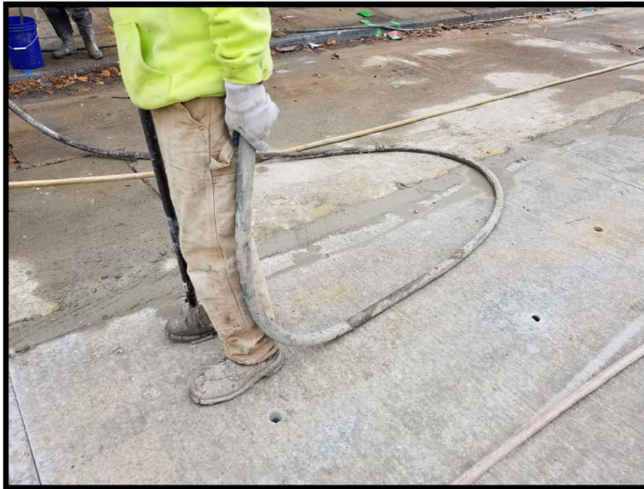
Pressure grouting of Phase 2 slabs.
