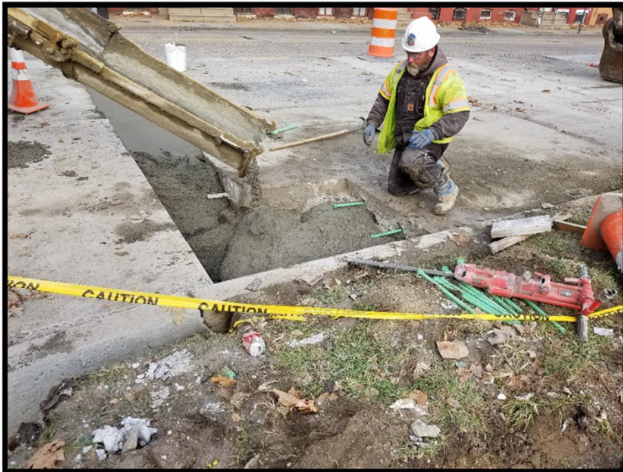
Infilling of slab gaps and repair areas with 4,000 psi concrete.
