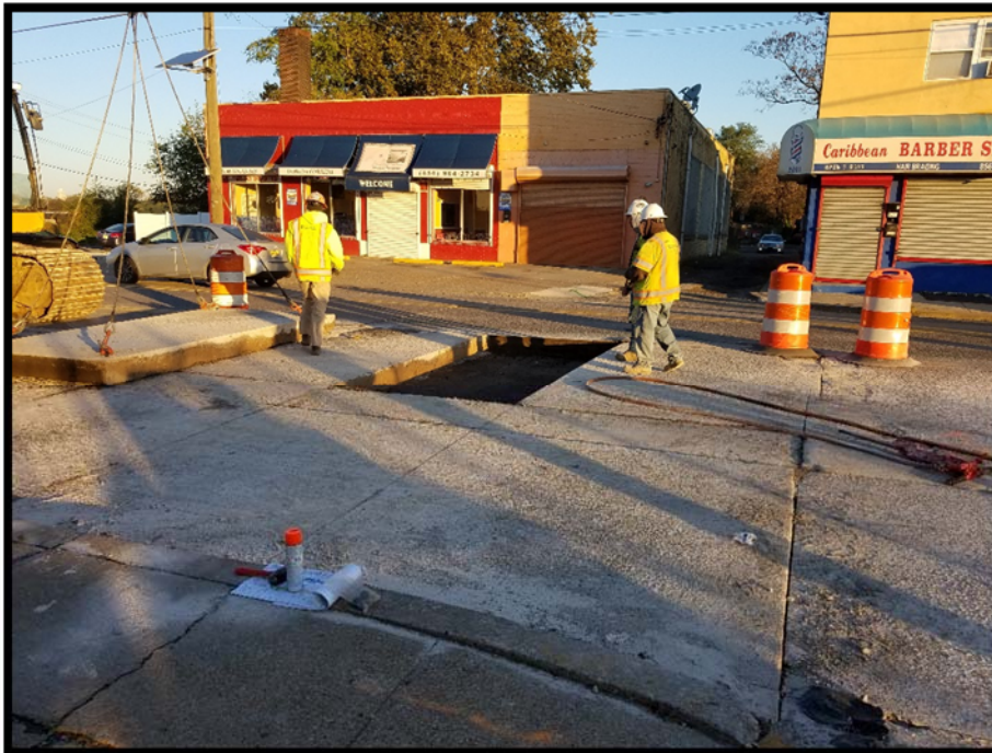
Existing slab removed.
