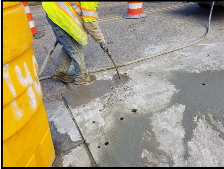
Pressure grouting of underslab in progress.
