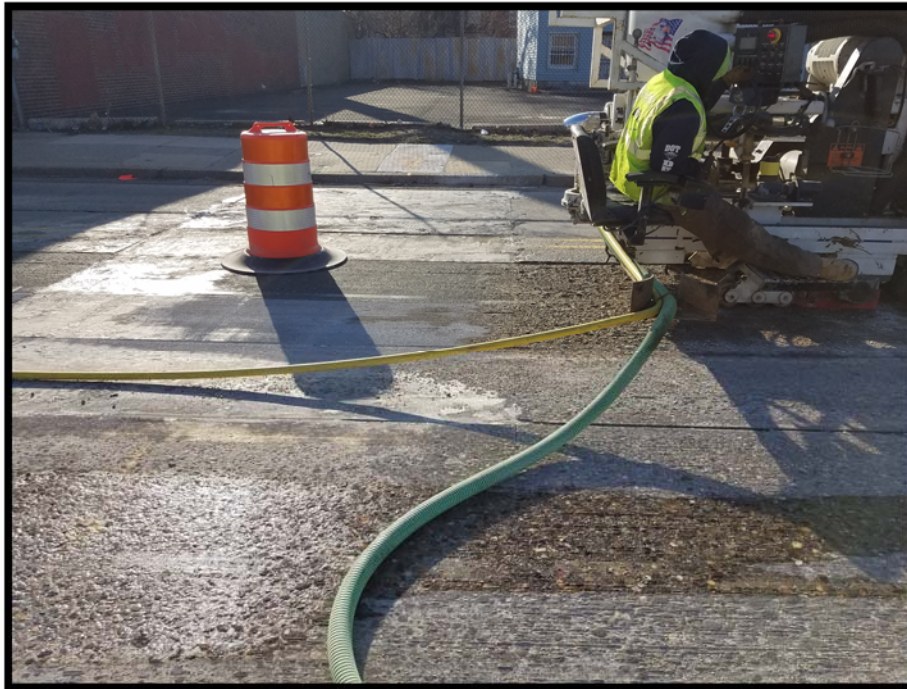
Diamond Grinder after making pass at uneven slab location.
