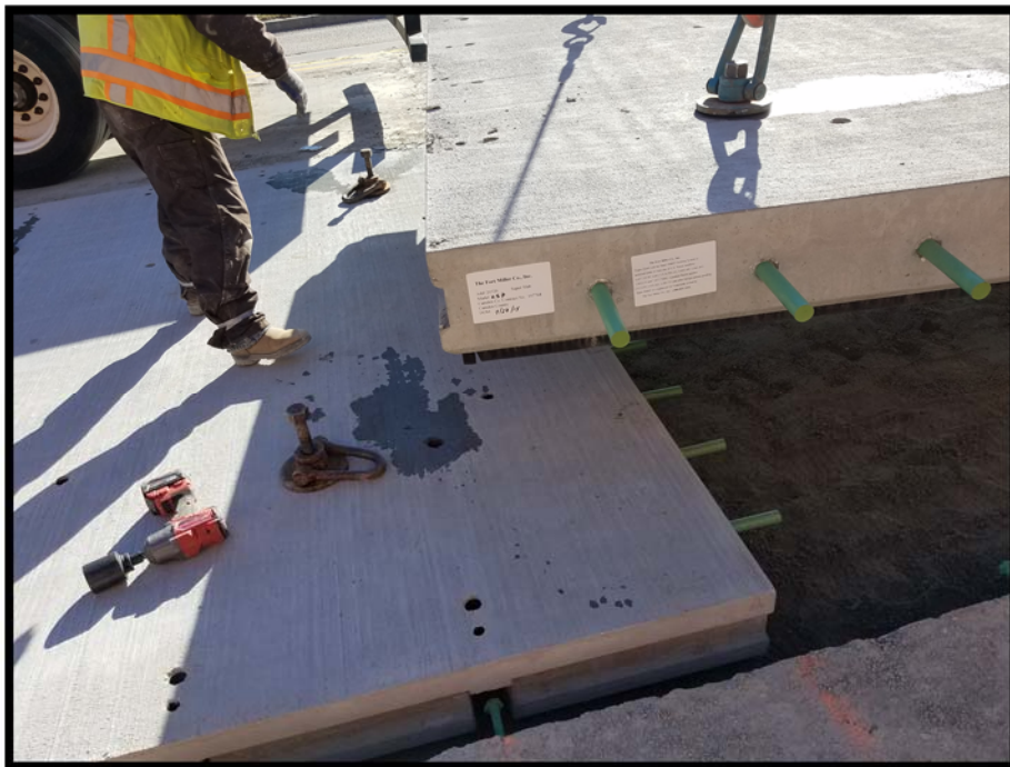
Phase 2 prefabricated slab being lowered into place.
