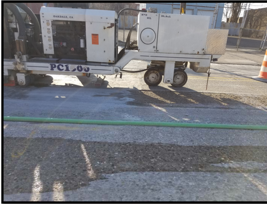
Diamond Grinder approaching uneven slab location.
