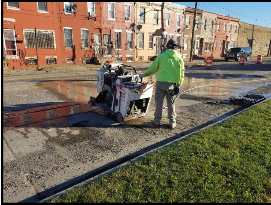
Sawcutting existing slabs prior to removal.
