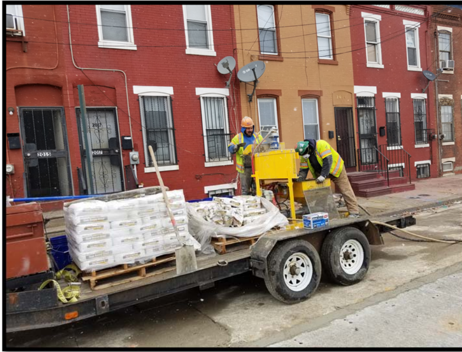
Contractor getting ready to pressure grout Phase 2 slabs.
