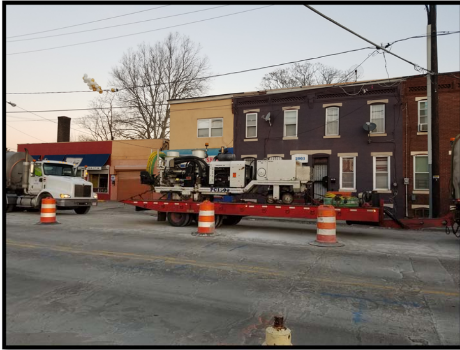
Diamond Grinder arriving on site.
