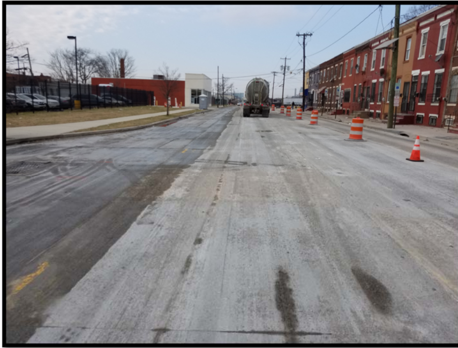
Roadway after completion of Diamond Grinding.
