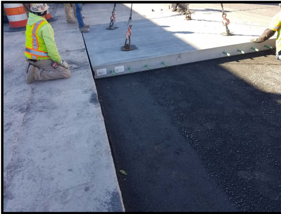
New precast reinforced concrete slab being lowered into place.
