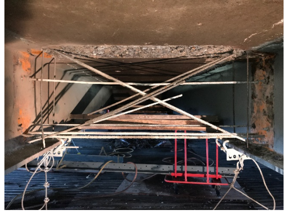
Figure 3: Cuthbert Blvd. Bridge – Diaphragm Reconstruction
