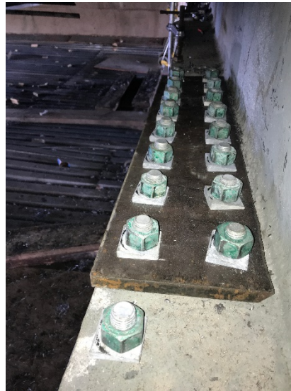
Figure 1: Cuthbert Blvd. Bridge – Steel Installation
