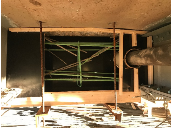
Figure 2: Cuthbert Blvd. Bridge – Rebar and Forms set for Diaphragms
