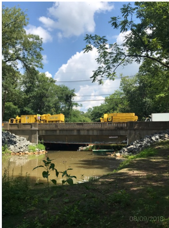
Figure 1: Grove St. Bridge Near-White Blast & Paint
