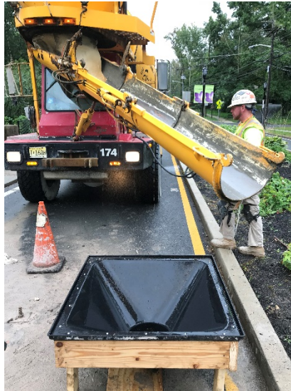
Figure 1: Grove St. Bridge – Concrete Placement
