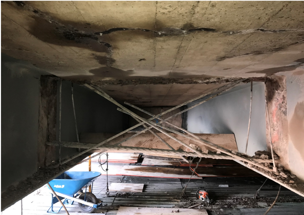
Figure 1: Grove St. Bridge Demolition of Concrete Diaphragms Beam G-9 – G-8
