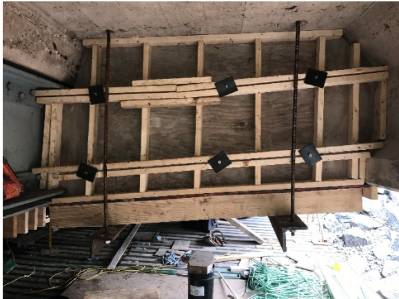
Figure 2: Grove St. Bridge Formwork between G8 and G9
