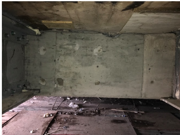
Figure 2: Grove St. Bridge Concrete Diaphragm
