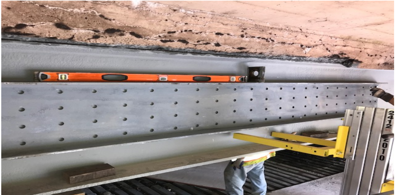
Figure 1: Grove St. Bridge Installation of Structural Steel Channel Beam G-9
