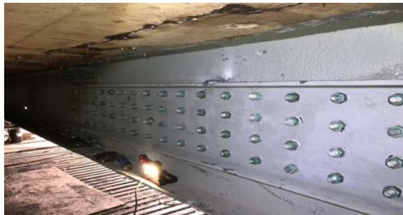
Figure 2: Grove St. Bridge Installation of Structural Steel Channel Beam G-8
