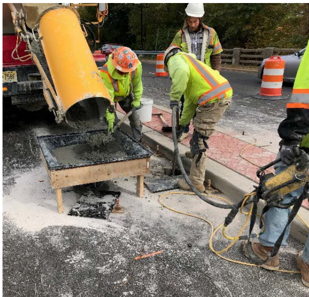
Figure 1: Cuthbert Blvd. Bridge – Concrete Pour
