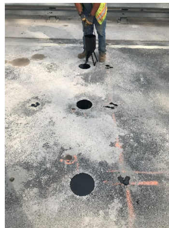
Figure 3: Grove St. Bridge Roadway Restoration
