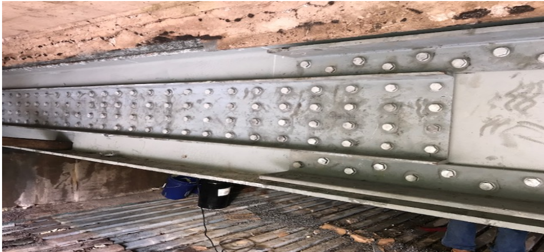
Figure 1: Grove St. Bridge Structural Steel Channel Beam Bolted G-9
