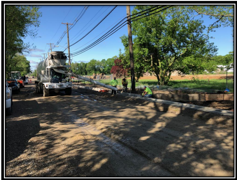
Figure: 3 – Installation of concrete curb and gutter along the westbound lane
