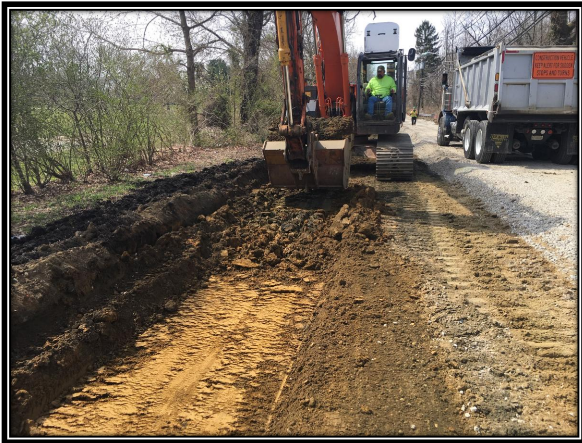
Figure: 1 – Roadway excavation along the northbound lane
