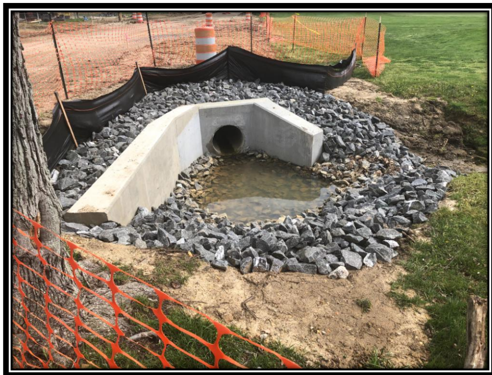
Figure: 3 – Scour hole protection at 24” concrete headwall along the northbound lane
