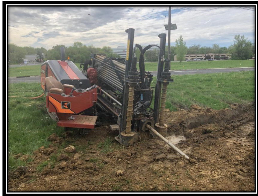
Figure: 2 – Directional drilling of 4” SDR 11 HDPE sanitary sewer force main
