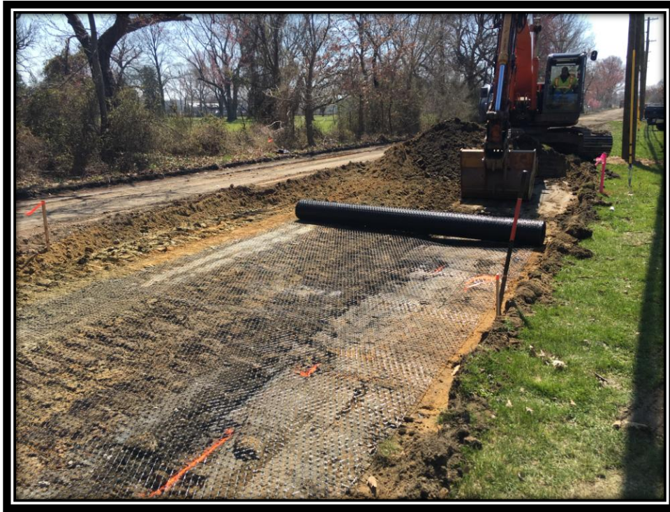
Figure: 2 – Installation of pavement reinforcing geogrid along the southbound lane
