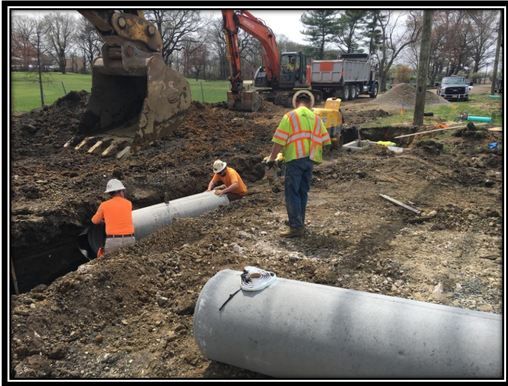
Figure: 2 – Installation of 18” reinforced concrete pipe along the southbound lane
