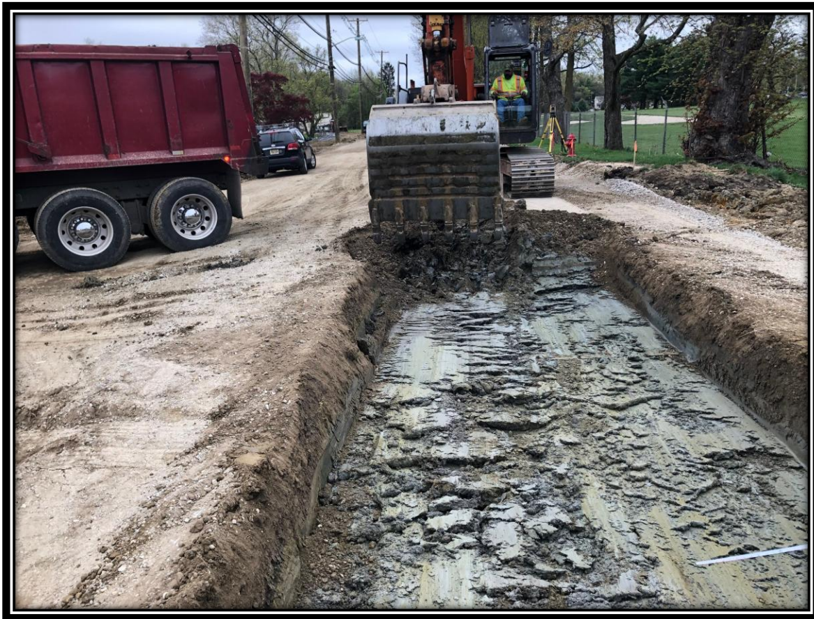
Figure: 1 – Roadway excavation of unsuitable material in the northbound lane
