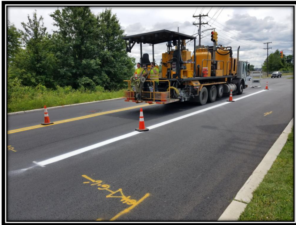
Figure: 3 – Installation of long life epoxy traffic striping
