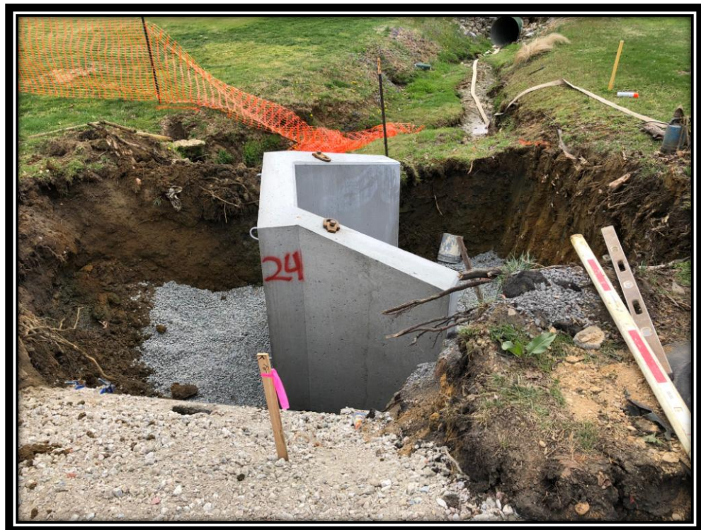
Figure: 3 – Installation of 24” concrete headwall along the northbound lane
