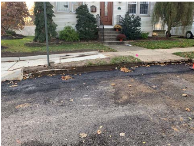
Figure 4: Hopkins Ave shoulder reconstruction
