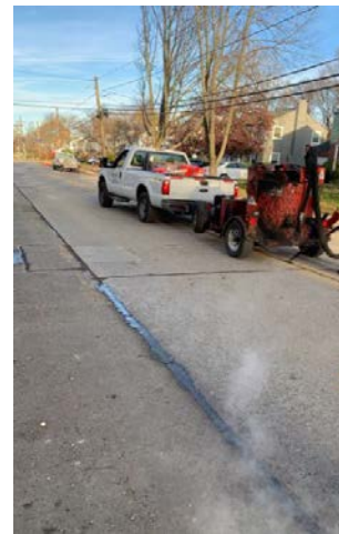
Figure 5: Cleaning and sealing joints
