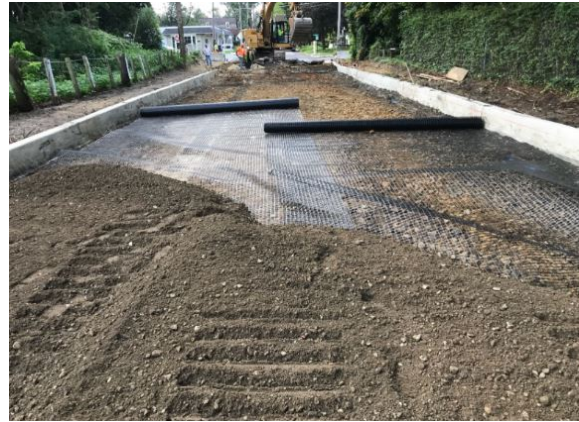
Figure 3: DGA and geogrid placement
