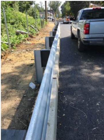
Figure 4: Guide rail installation
