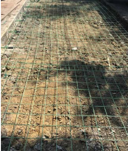
Figure 2: Concrete roadway subbase repairs
