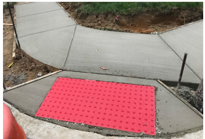
Figure 5: Concrete curb ramp placed
