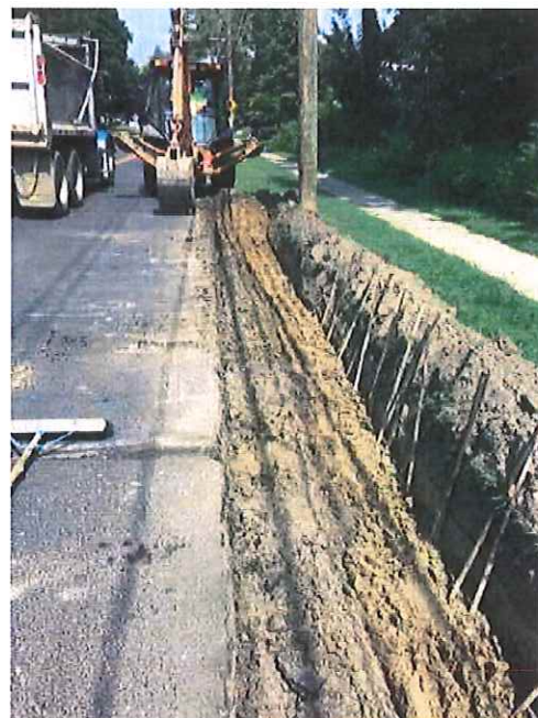
Figure 3: Concrete vertical curb demolition
