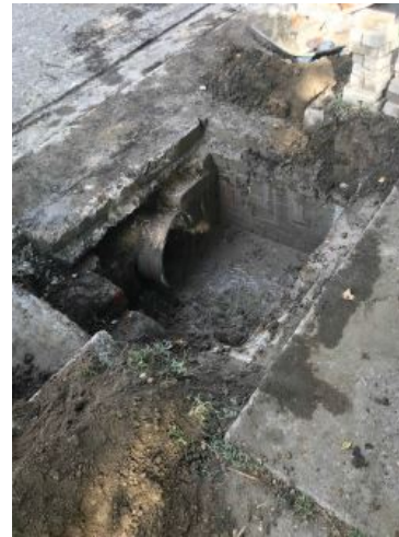
Figure 3: Storm sewer inlet reconstruction
