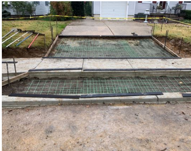
Figure 2: Reinforcement for concrete driveway
