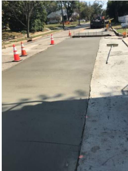
Figure 1: Concrete roadway repair
