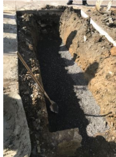
Figure 5: Trench for storm pipe installation
