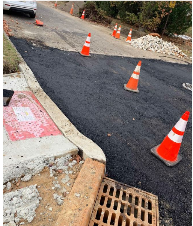
Figure 5: Reconstructed roadway section
