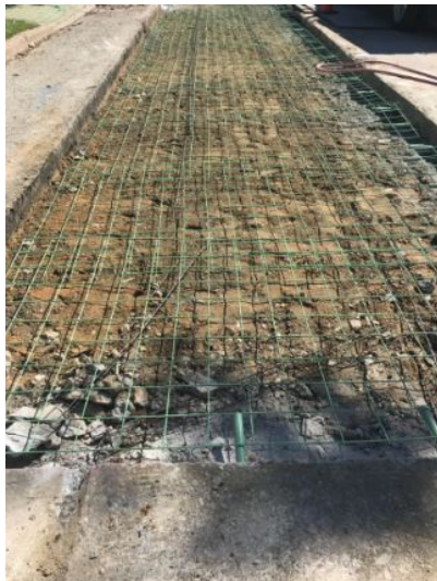
Figure 4: Reinforcement for concrete roadway repairs
