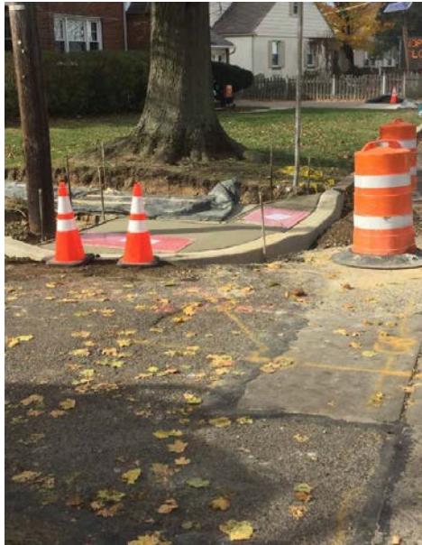
Figure 1: Concrete curb ramps
