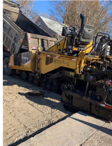
Figure 3: Intersection paving
