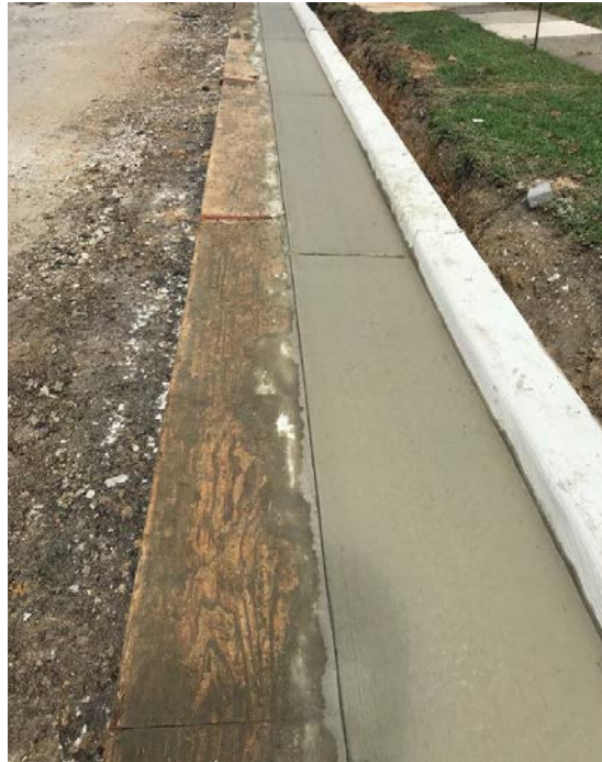
Figure 1: Concrete curb and gutter
