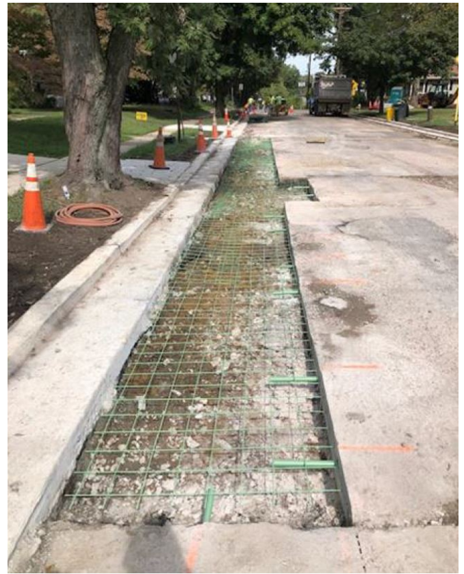
Figure 5: Concrete roadway repairs
