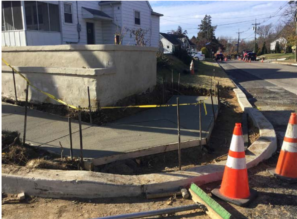
Figure 1: Concrete curb ramp
