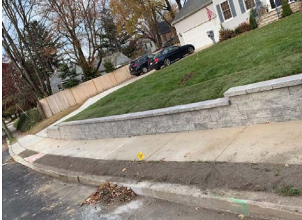
Figure 2: Concrete block wall
