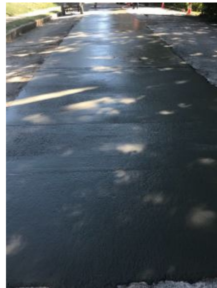
Figure 5: Concrete placed for roadway repairs
