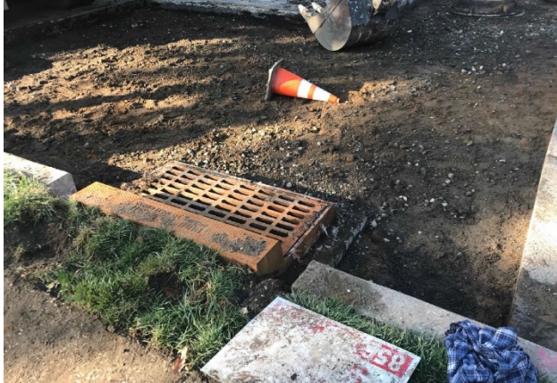
Figure 2: Excavation for concrete road repair
