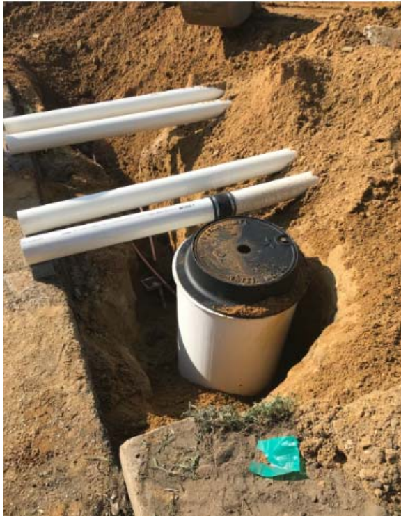
Figure 4: Water valve fixed and relocated
