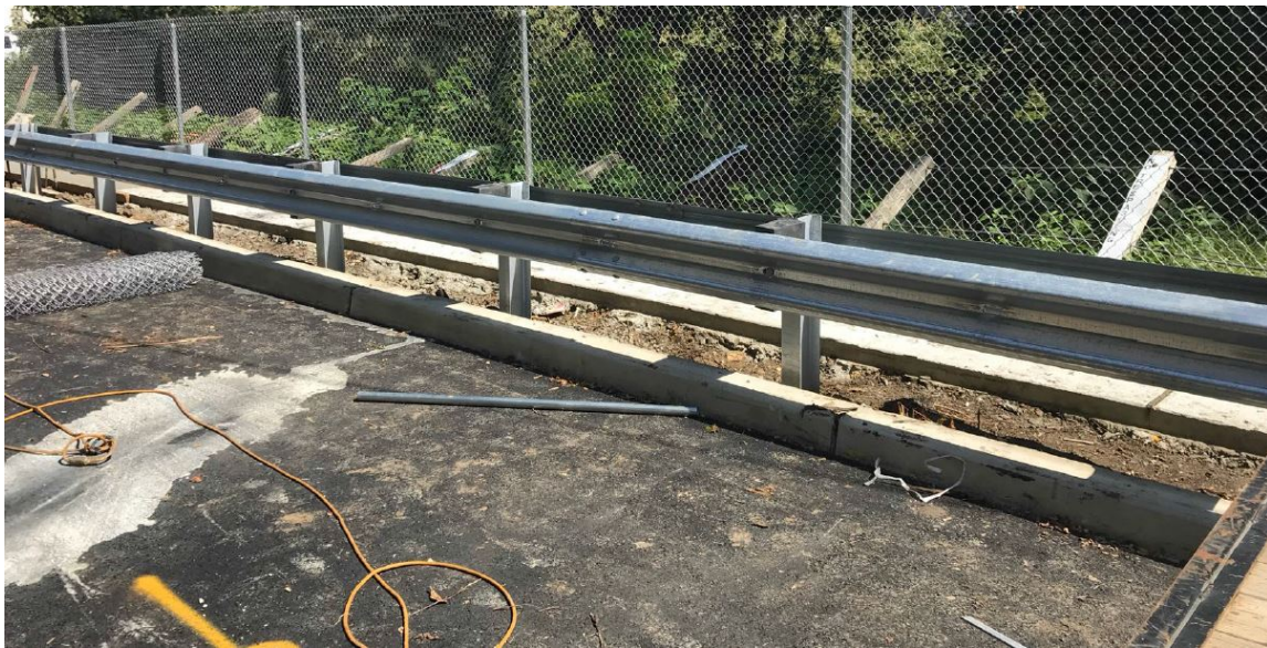
Figure 1: Concrete sidewalk, curb, guide rail and chain link fence by culvert
