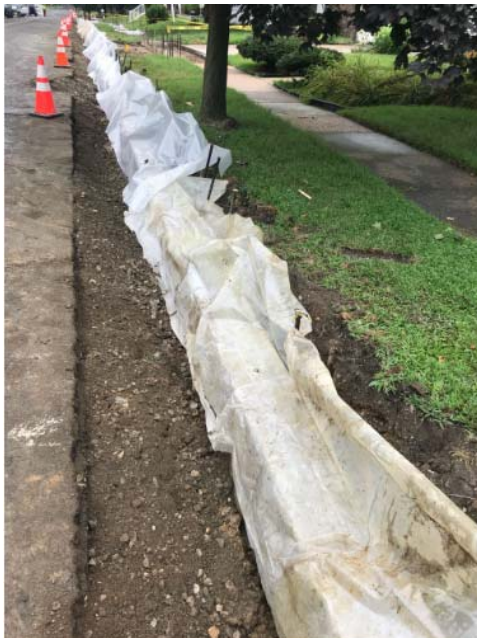
Figure 2: Temporary plastic covering over curb due to rain throughout the day
