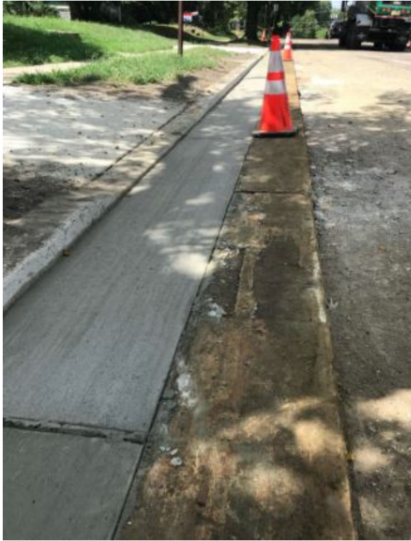
Figure 4: Concrete gutter work
