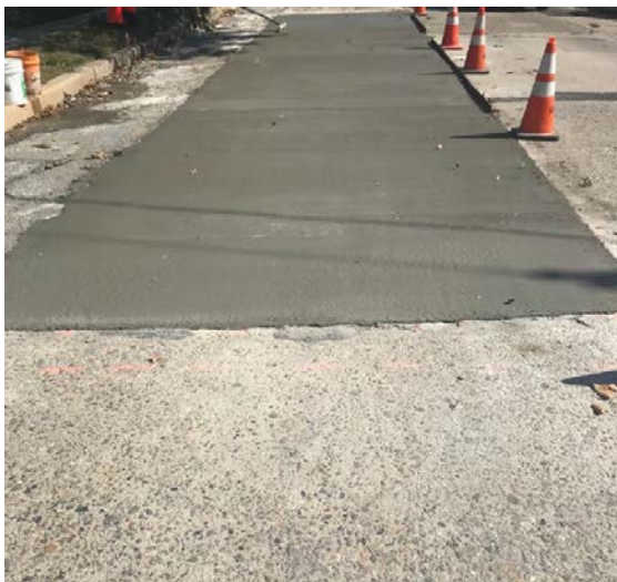
Figure 4: Concrete roadway repairs
