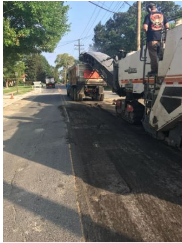
Figure 5: Milling operations along Hopkins Ave
