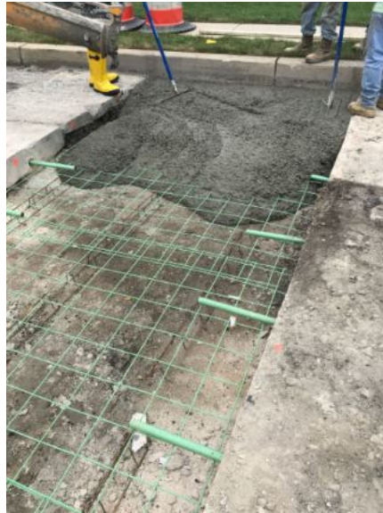
Figure 1: Concrete roadway repairs
