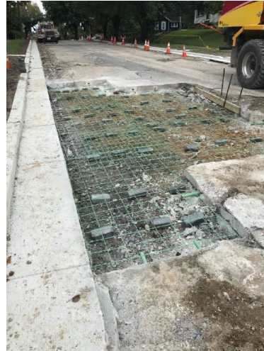
Figure 3: Concrete roadway subbase repair
