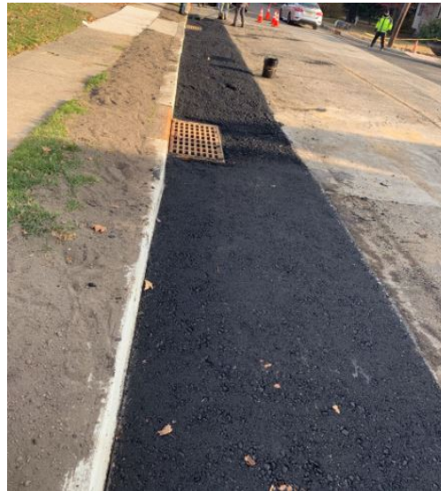
Figure 3: Hopkins Ave shoulder reconstruction
