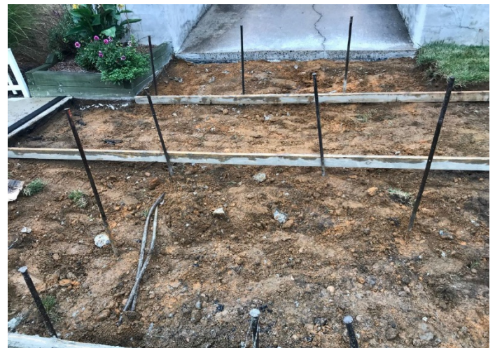
Figure 3: Concrete sidewalk and driveway apron formed
