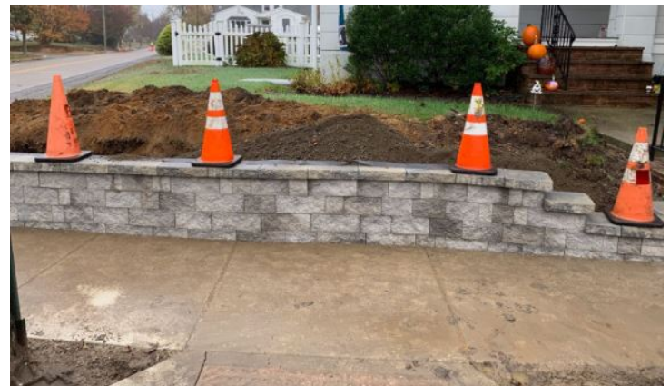
Figure 3: EP Henry wall constructed
