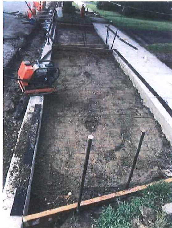
Figure 5: Reinforcement installed for concrete driveway
