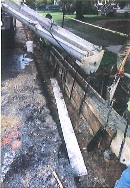
Figure 4: Concrete vertical curb installation
