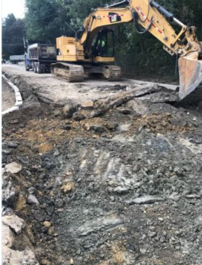
Figure 2: Culvert excavation
