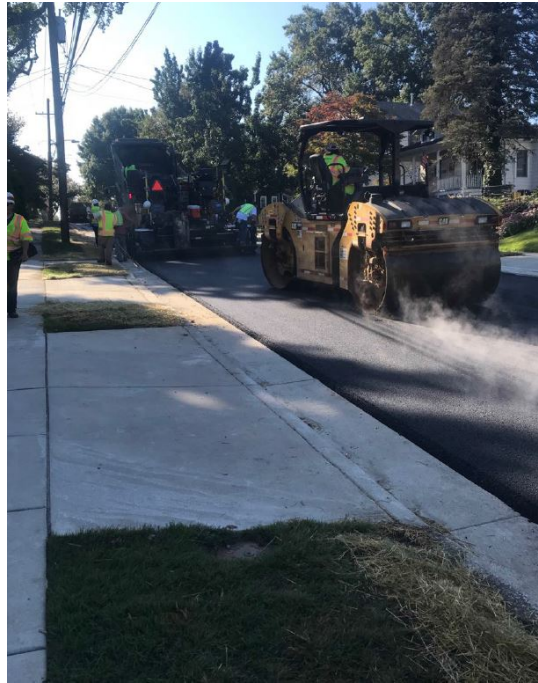
Figure 1: Paving operations by Paul VI
