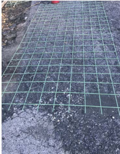
Figure 1: Wire reinforcement used for commercial parking lot
