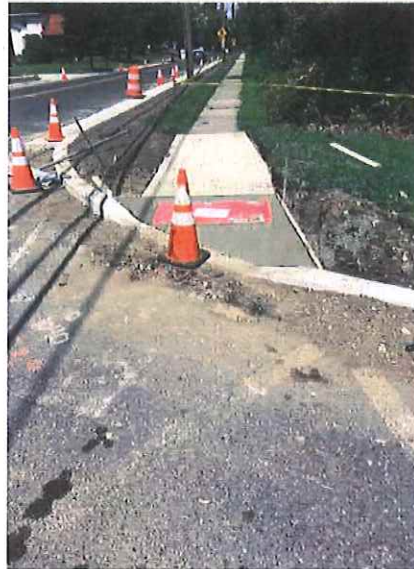
Figure 1: Concrete curb ramp installation
