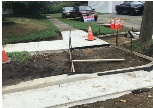
Figure 1: Concrete curb ramp reconstruction
