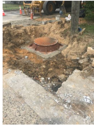
Figure 3: Inlet converted to a manhole
