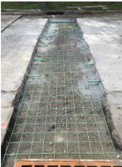
Figure 4: Concrete roadway repairs
