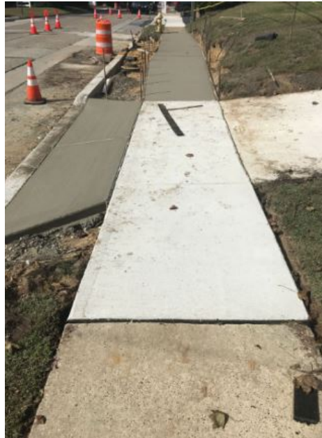
Figure 1: Concrete sidewalk and driveway
