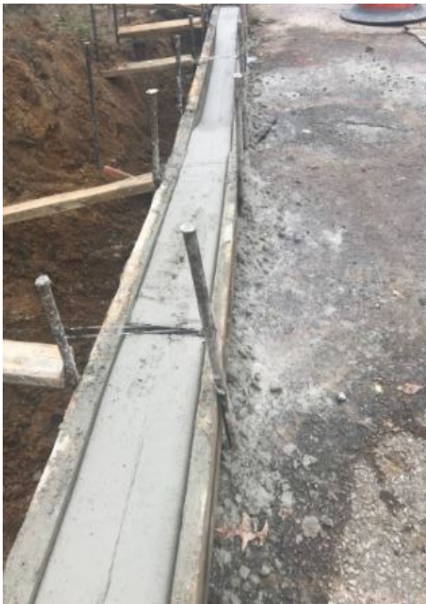
Figure 2: Concrete vertical curb placed
