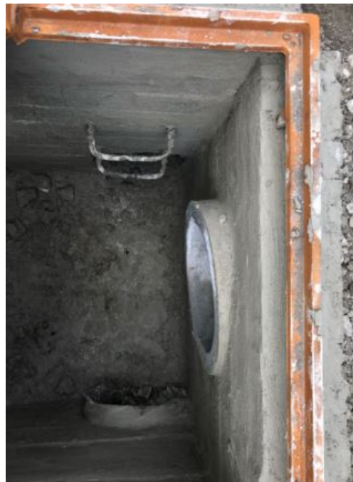
Figure 3: Inlet reconstructed
