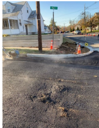
Figure 5: Reconstructed roadway section
