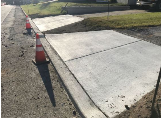
Figure 4: Concrete reinforced driveways
