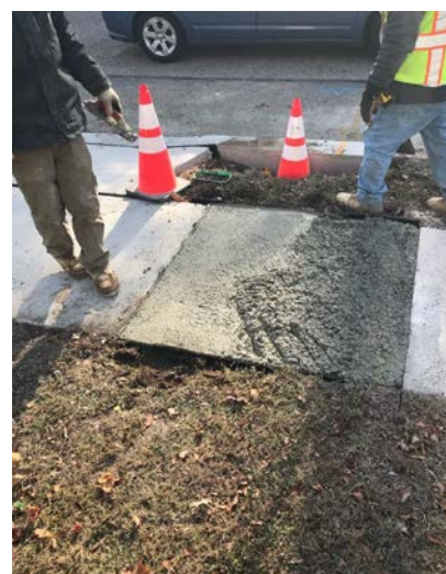
Figure 3: Concrete sidewalk placement
