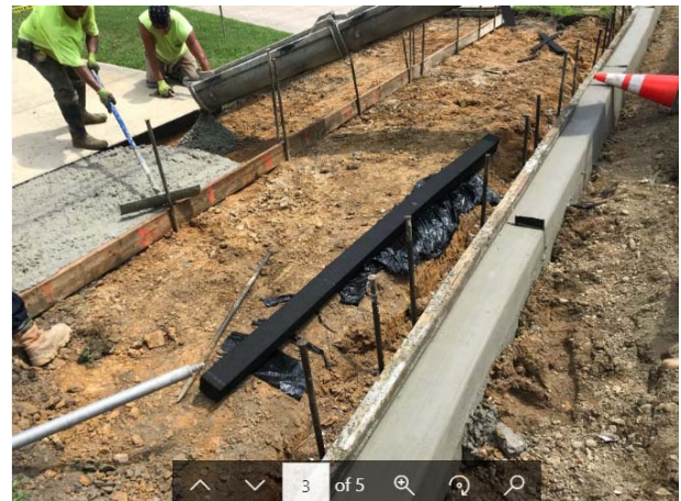
Figure 3: Concrete for 6” driveway being placed
