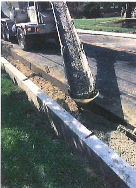
Figure 2: Concrete curb & gutter installation
