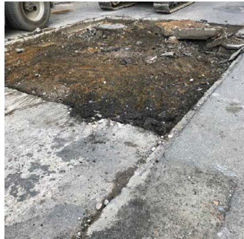
Figure 5: Excavation for concrete roadway repairs
