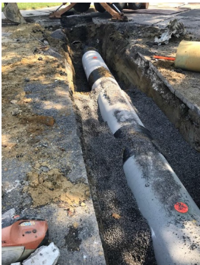
Figure 4: Installation of storm sewer system
