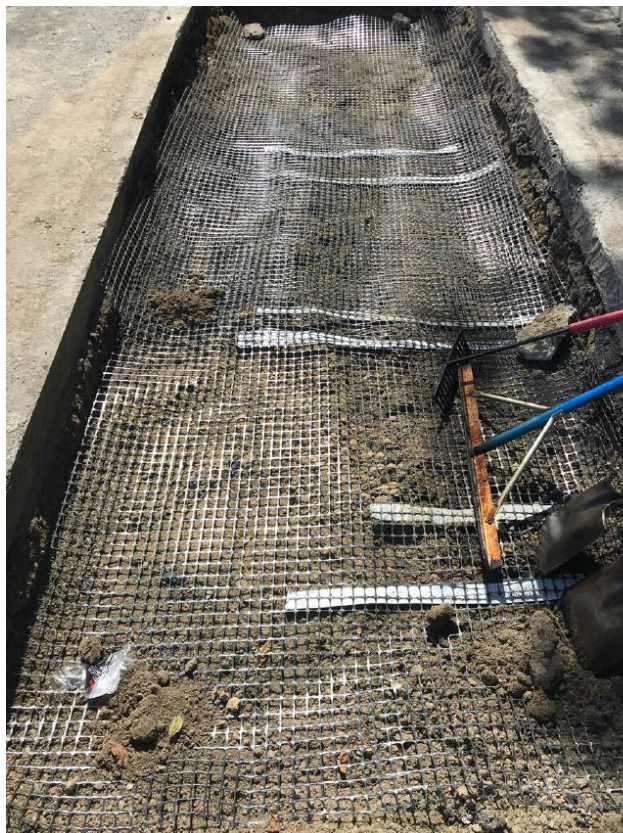
Figure 2: Roadway base repair
