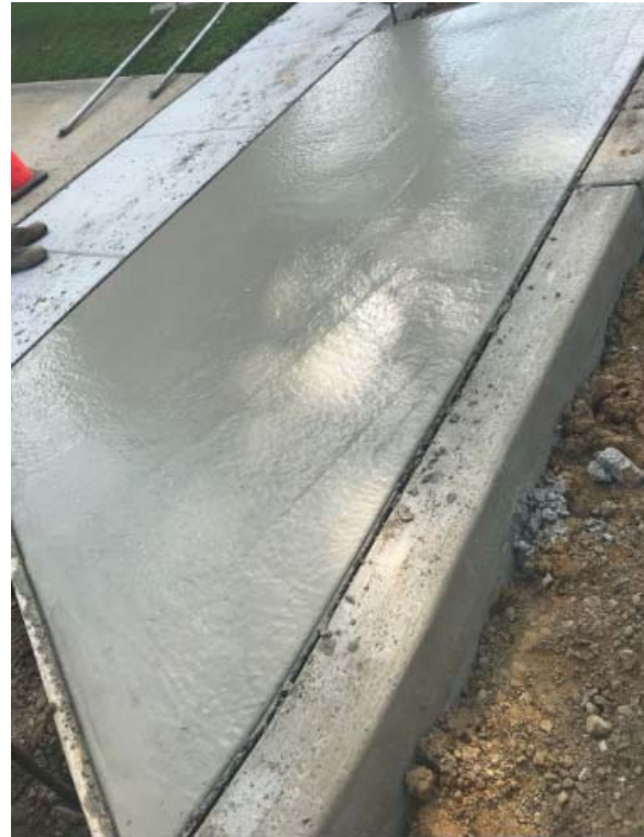
Figure 5: Concrete for 6" driveway being placed
