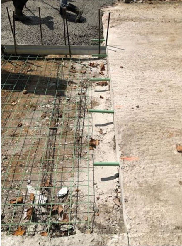
Figure 4: Concrete roadway repairs
