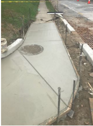
Figure 2: Concrete sidewalk placed
