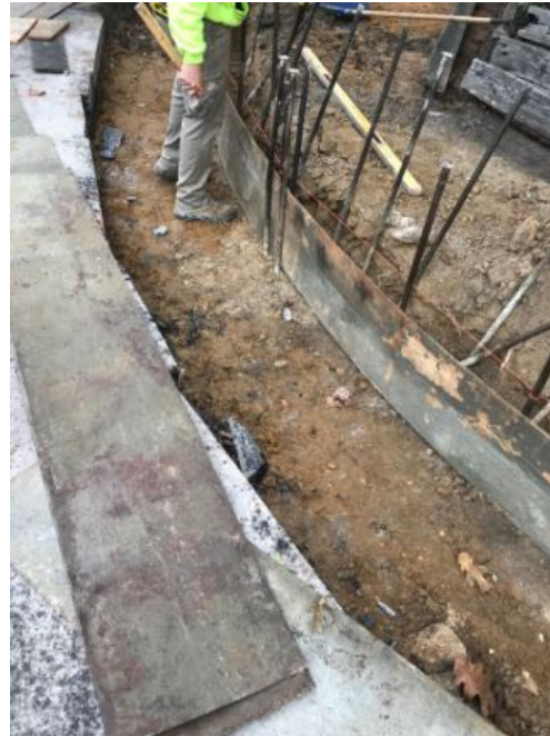
Figure 5: Forms set for concrete vertical curb
