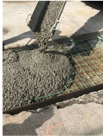
Figure 3: Concrete placement for road repair
