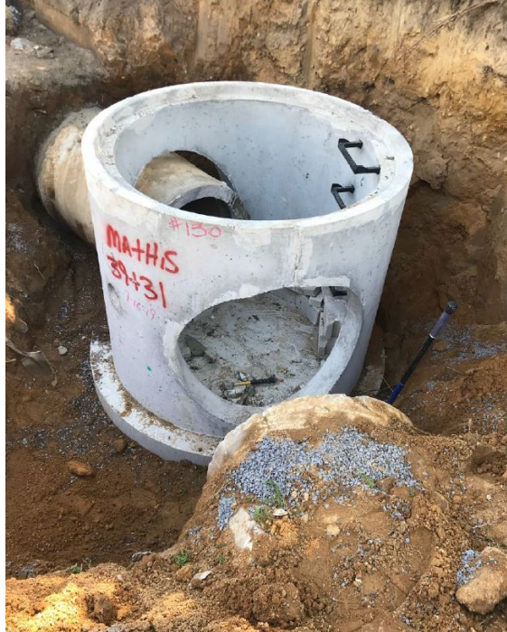
Figure 1: Storm sewer installation
