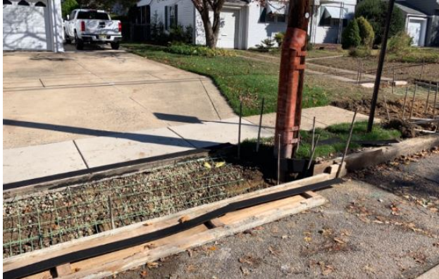
Figure 4: Concrete driveway replacement
