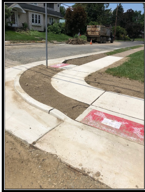
Figure 2: New concrete sidewalk and handicap ramps at Avondale & Foreman Avenues.
