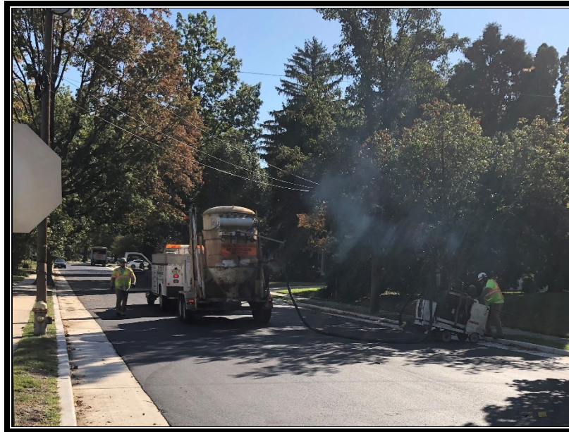
Figure 2: Joints along Avondale Avenue saw cut in bituminous surface course.
