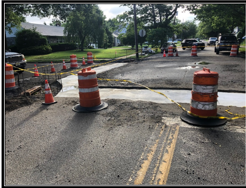
Figure 2: Concrete roadway replaced above pipe on Avondale and Austermuhl Avenues.
