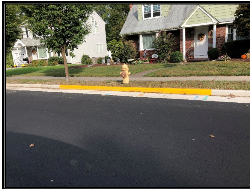
Figure 3: Yellow curb marking fire hydrants along Avondale Avenue.
