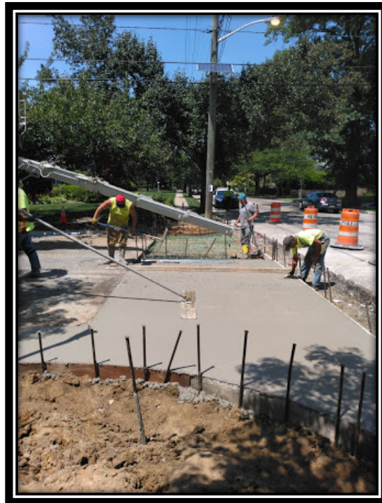
Figure 1: New concrete roadway on Avondale Avenue at Crystal Lake.
