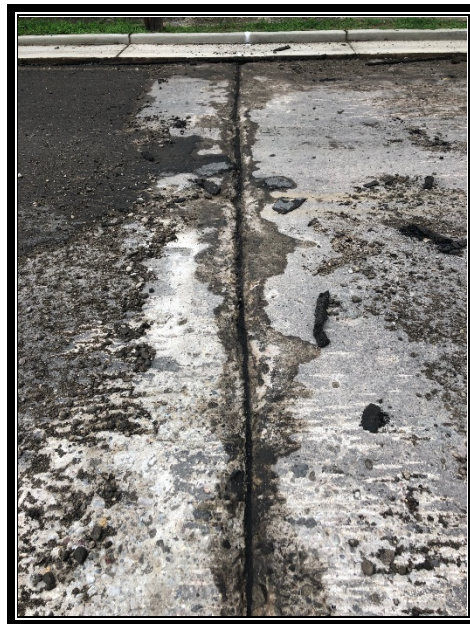
Figure 3: Joints in concrete base cleaned out and ready to be sealed.
