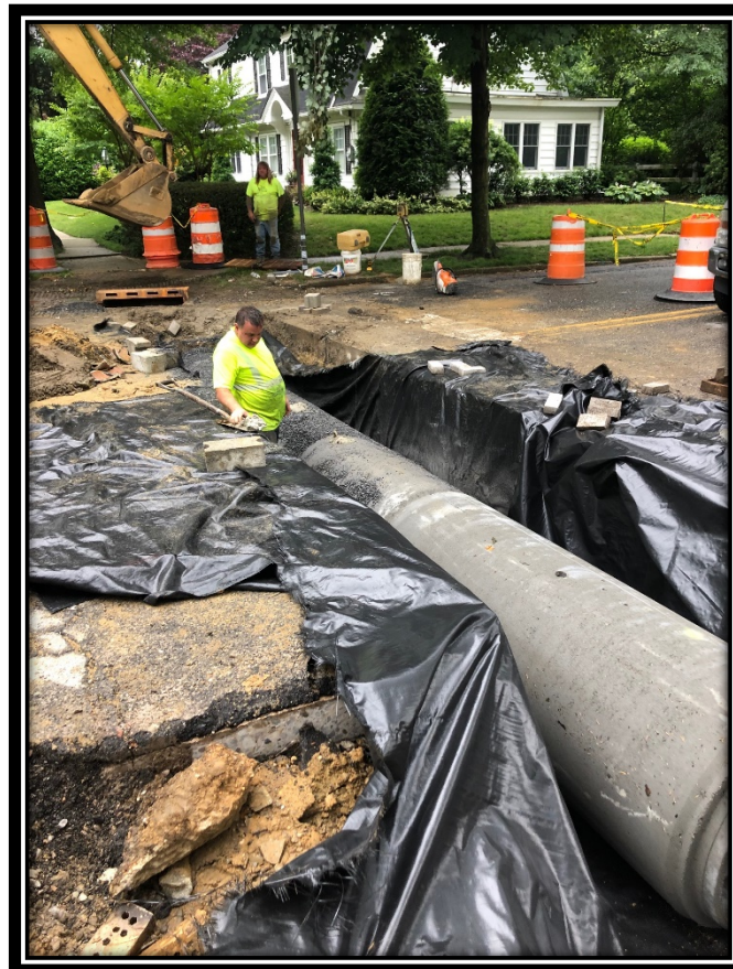
Figure 1: New drainage pipe at the intersection of Avondale & Austrermuhl Avenues.
