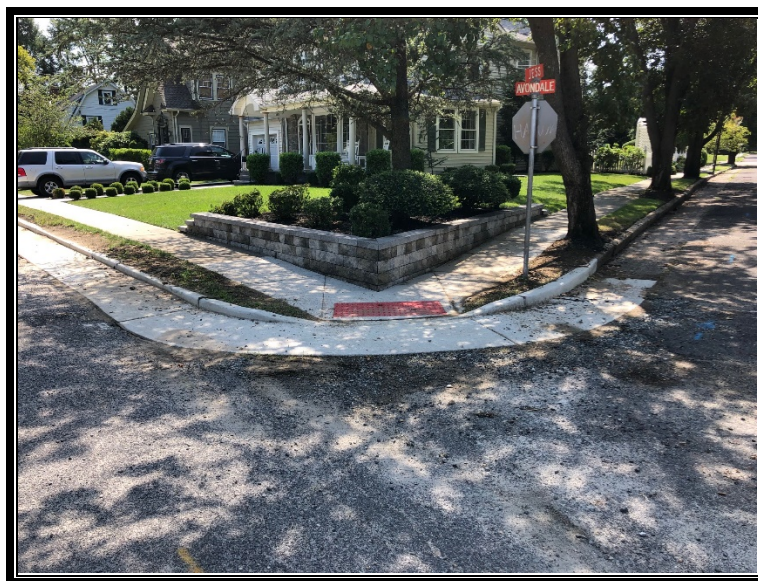
Figure 3: New interlocking retaining wall at Avondale and Jess Avenues.
