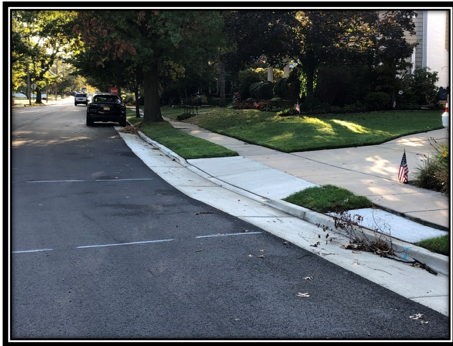
Figure 1: Transverse joints in concrete base laid-out on surface course.
