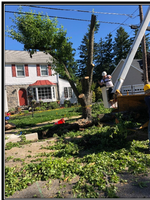
Figure 3: Removing selected trees within the project limits.
