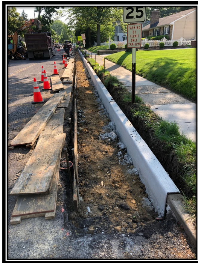
Figure 1: New curb on Avondale Avenue near Hopkins Road.
