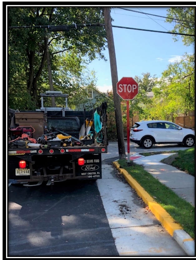
Figure 1: Contractor on-site installing new signs on Avandale Avenue.
