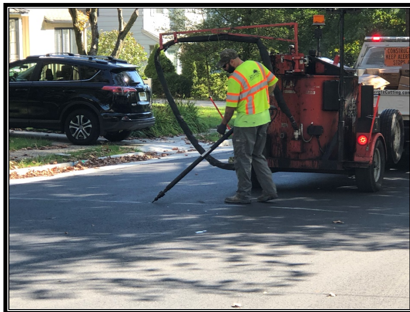
Figure 3: After saw cutting, joints are sealed with bituminous joint sealer.
