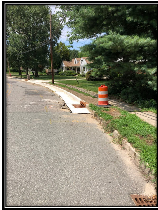
Figure 1: Completed curb, gutter and new inlets on Avondale Avenue.
