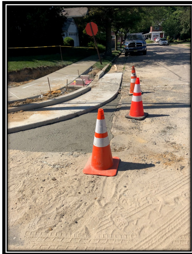
Figure 1: Replacement of concrete base course at each corner.
