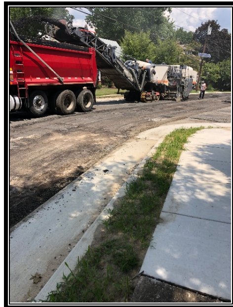
Figure 3: Milling existing asphalt from concrete base course.
