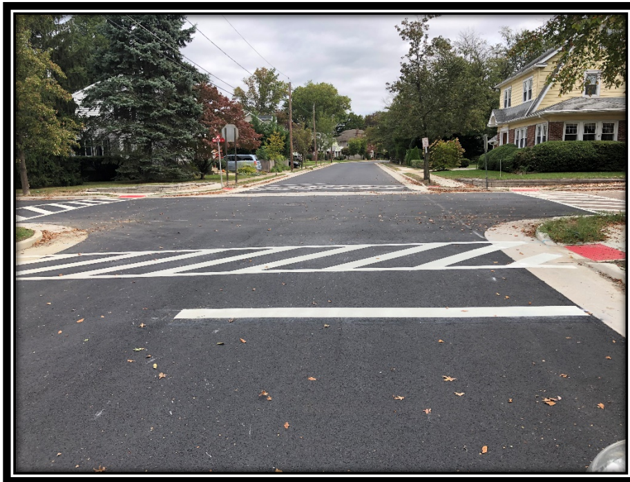
Figure 1: Contractor installed crosswalks and stop bars on Avondale & Breslin Avenues.
