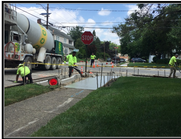
Figure 3: New sidewalk at Avondale & Foreman Avenues.
