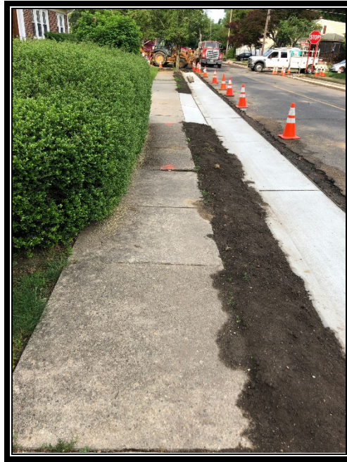
Figure 2: New concrete curb, gutter and driveway with topsoil restoration.
