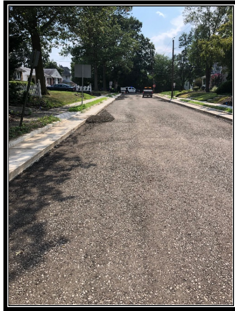
Figure 2: DGA installed and fine-graded, ready for base paving.
