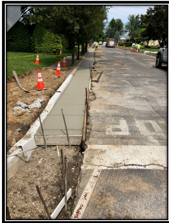
Figure 1: New curb and gutter on Breslin Avenue.
