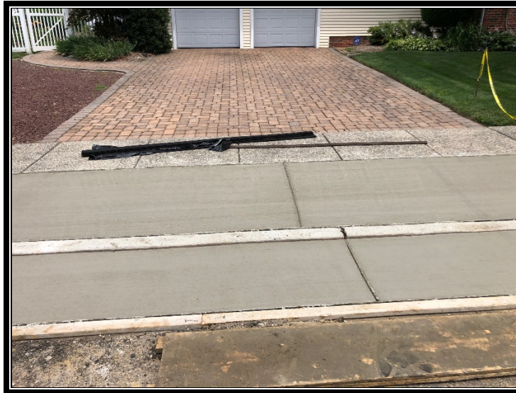
Figure 2: New concrete driveway apron and gutter.
