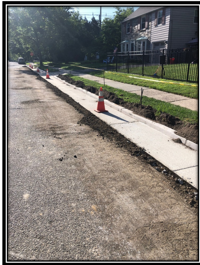
Figure 1: Completed curb and gutter on Avondale Avenue.
