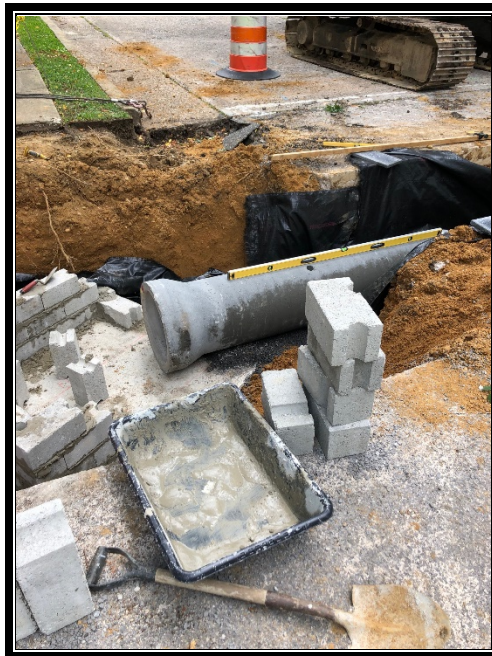
Figure 3: Concrete pipe and new inlets at Avondale & Austermuhl.
