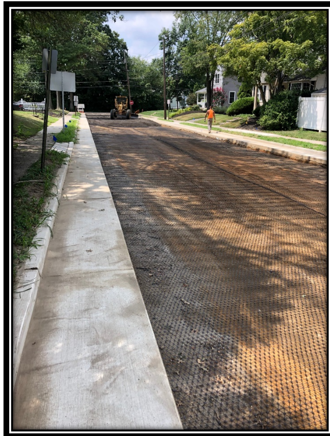
Figure 1: Full-depth reconstruction of Avondale from Hopkins to Breslin.
