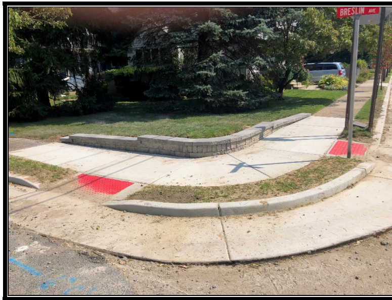
Figure 2: New interlocking retaining wall at Avondale and Breslin Avenues.
