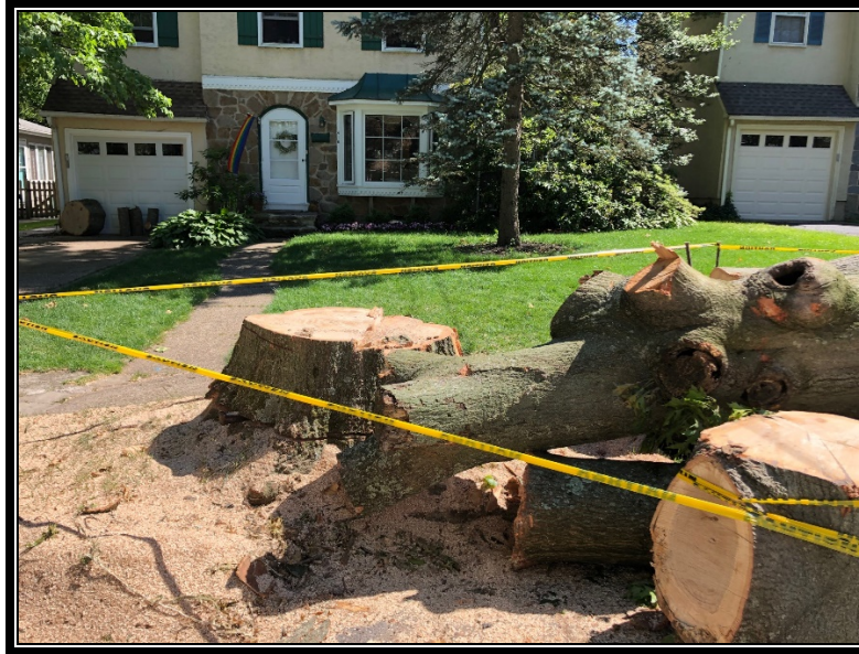
Figure 2: Selected tree removal along Avondale Avenue.
