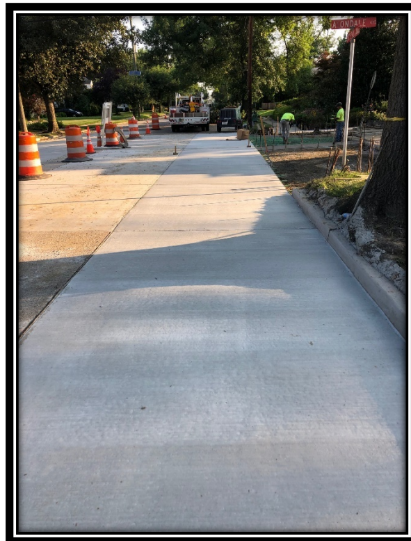
Figure 1: New concrete roadway on the east side of Crystal Lake Avenue.
