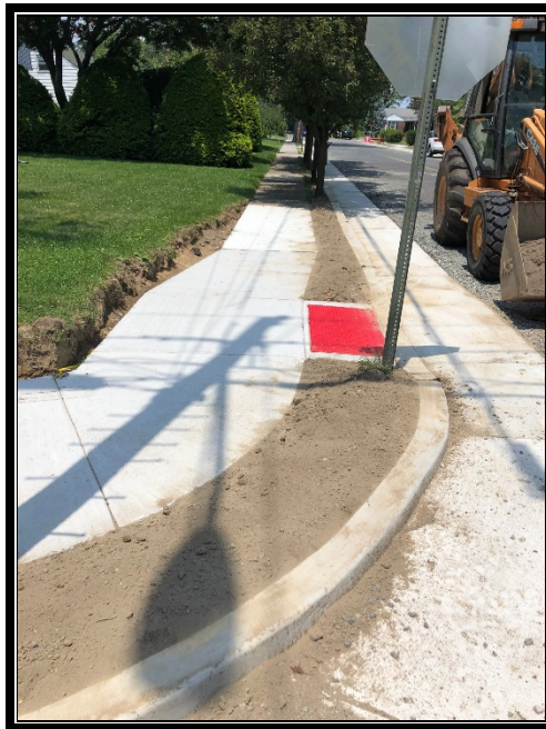
Figure 3: New sidewalk and handicap ramp at Avondale & Tomlinson Avenues.
