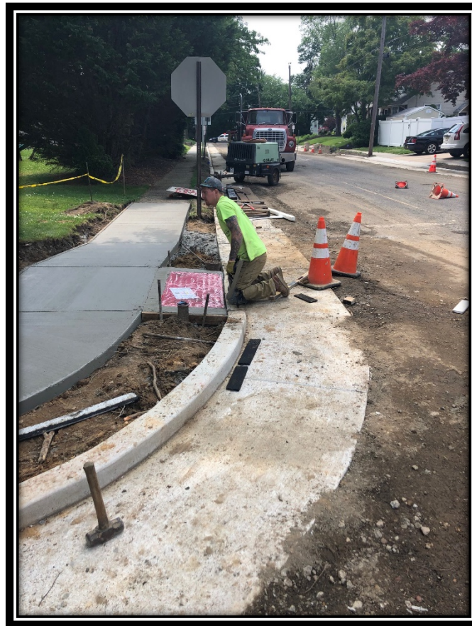
Figure 1: New sidewalk and handicap ramp on Avondale Avenue.
