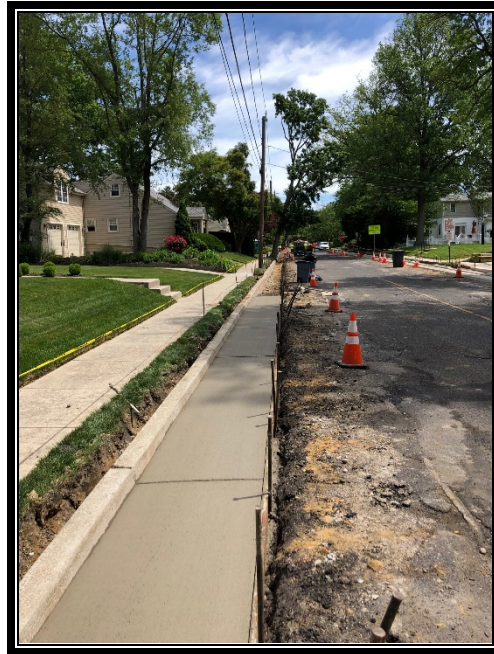
Figure 2: New concrete curb and gutter on Avondale Avenue.
