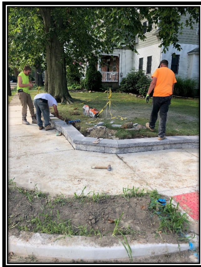
Figure 1: Contractor installing new interlocking retaining walls.
