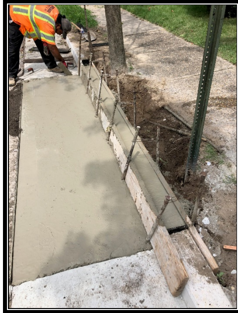
Figure 2: All damaged gutter replaced by contractor.
