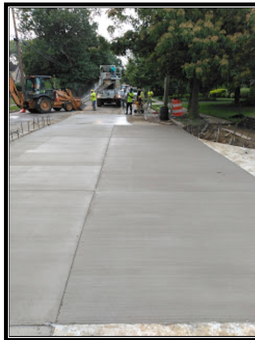
Figure 3: New SB roadway on Crystal Lake Avenue at Avondale.
