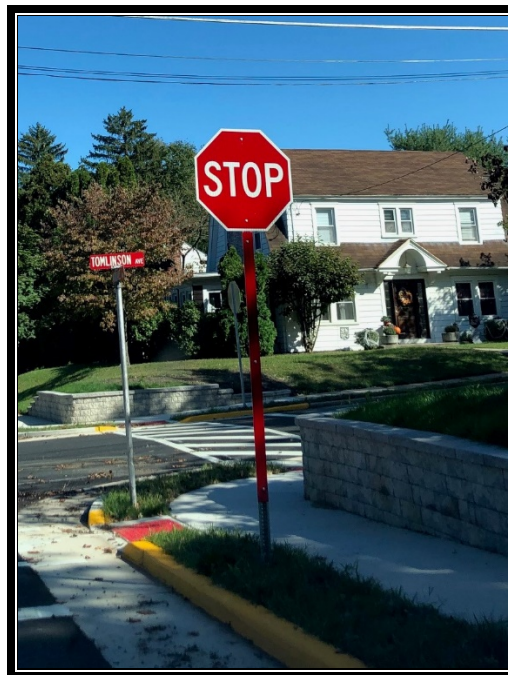
Figure 3: Contractor installed new stop signs with reflective posts on project.
