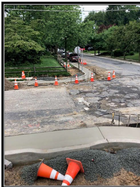
Figure 3: New curb and gutter at Avondale & Tomlinson Avenues.
