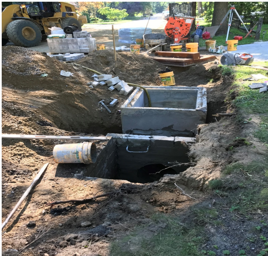
Figure: 1 – Reconstruct Inlet near Manor Landing on lake Blvd (Looking East side).
