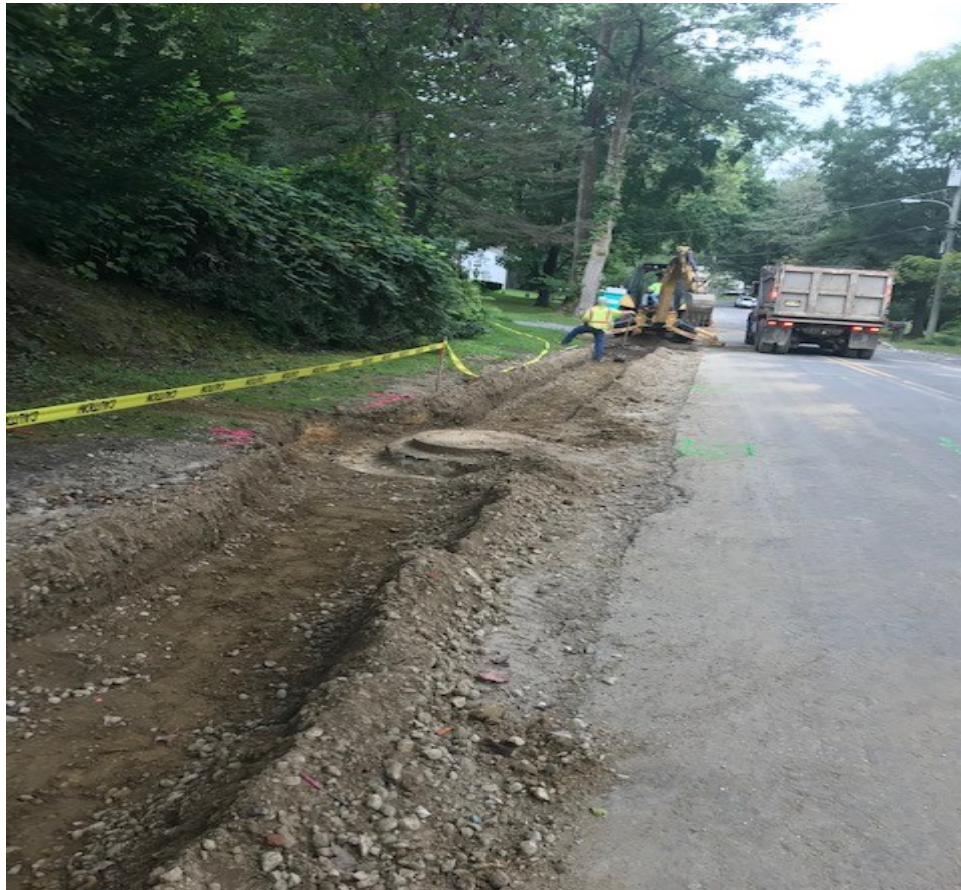
Figure: 1 – Curb Reconstruction Near Manor Landing Road (Looking East side).
