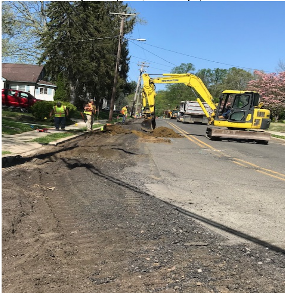
Figure: 1 – Utility pipe replacement near W.park Ave on lake Blvd.
