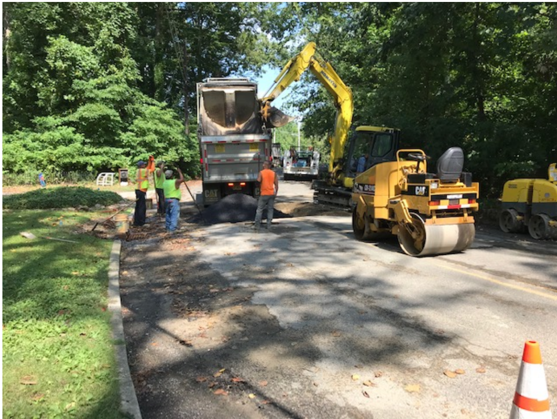
Figure: 1 – Trench compaction where Pipe reconstruction done (Looking East side).
