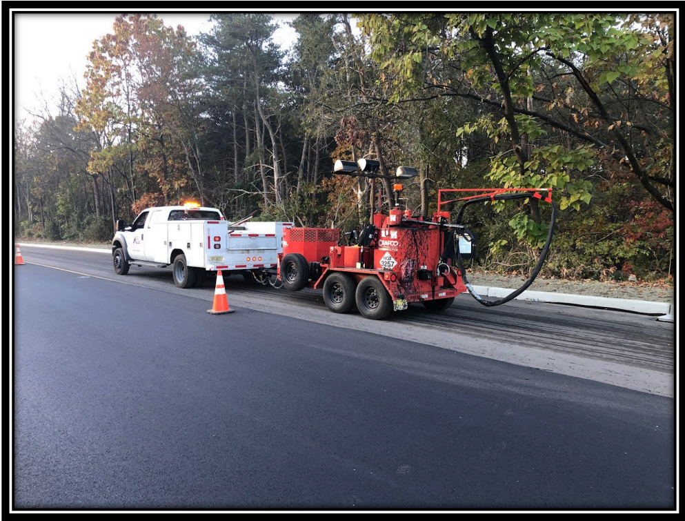
Figure: 2 –APS applying joint adhesive along Lower Landing/Good Intent Road (CR 681).
