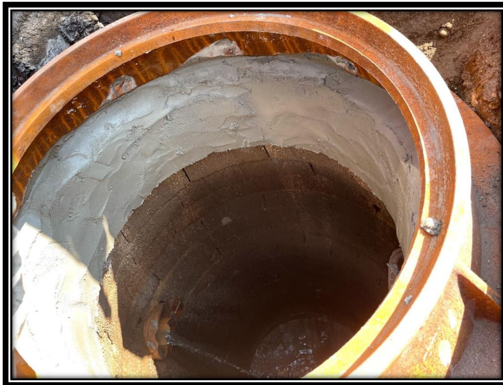
Figure: 3 – Clean Earth Matters reconstructed manholes along Lower Landing/Good Intent Road.
