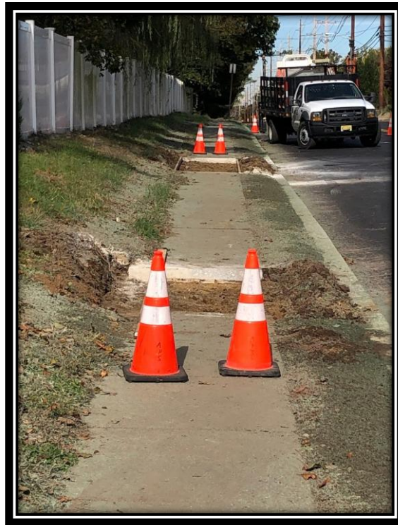
Figure: 2 –APS replacing necessary sidewalk along Lower Landing/Good Intent Road (CR 681).
