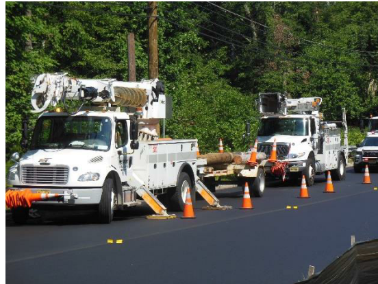
Figure 6 Verizon made it in to perform the pole transfer
