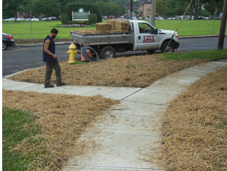
Figure 4 Straw mulch completed after seed was placed
