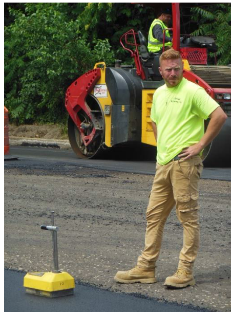
Figure 5 Contractor had service checking density as they paved
