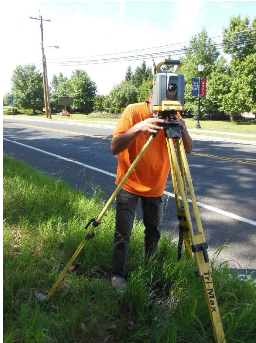
Surveyor establishing control points for layout of the project
