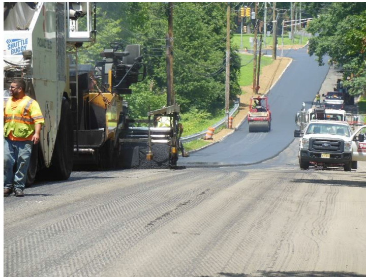
Figure 3 Paving train with roller in the background
