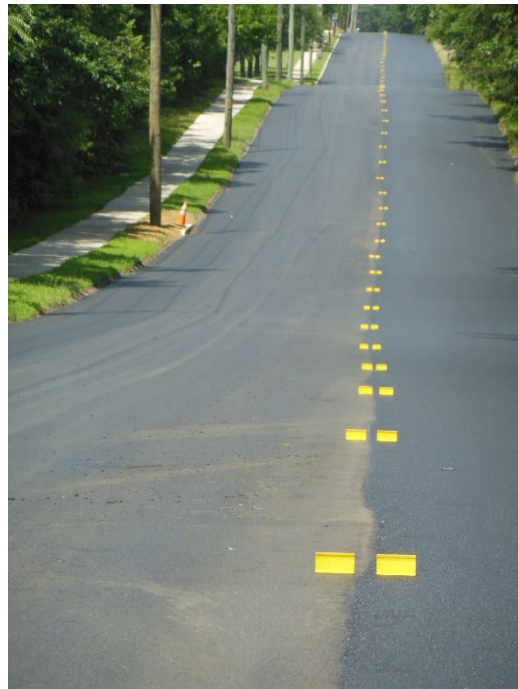
Figure 5 Paved roadway with temporary marked in center
