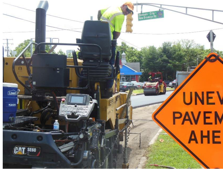
Figure 4 Bituminous paving started with leveling and intermediate course
