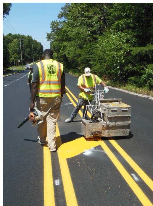
Figure 5 Installing the yellow gorge 24" lines
