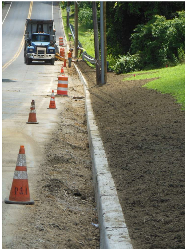
Figure 1 Topsoil was installed throughout the project
