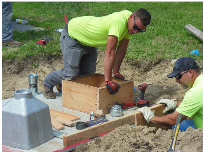
Figure 3 Electrical Sub was in installing the Pedestrian Push button Foundations
