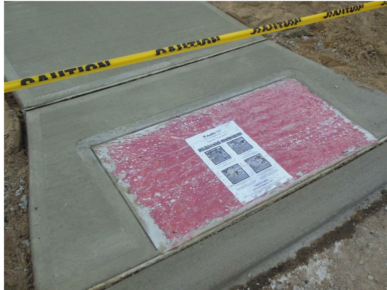
Figure 2 Detectable warning Surface installed at all required locations
