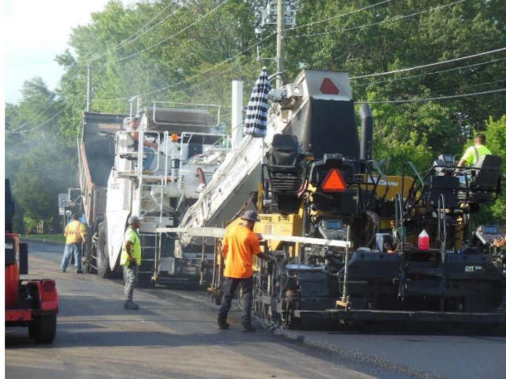
Figure 2 Paver being loaded by the MTV
