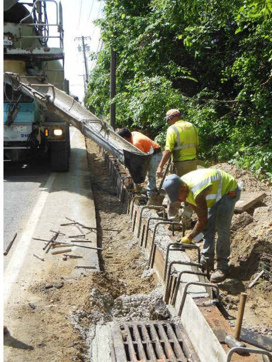
Figure 4 Pouring curb in forms set the grade and offset
