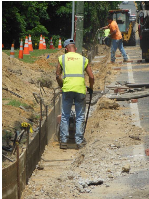
Figure 3 Compaction of material under the curb to be poured
