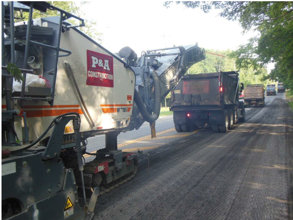
Figure 1 Milling operations were completed this week
