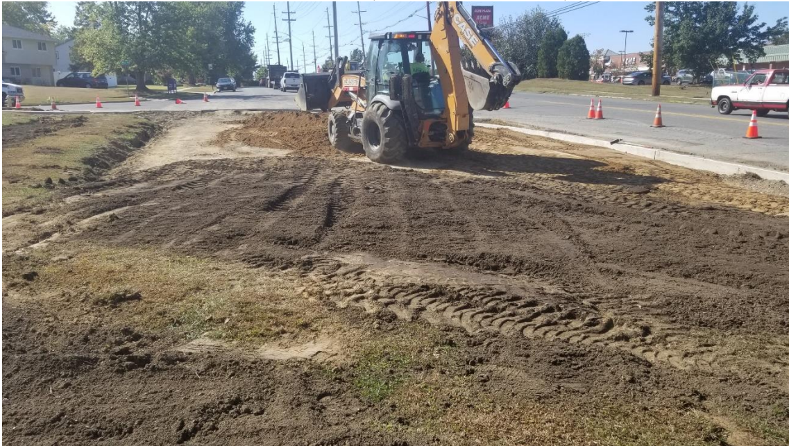
Figure 1. Lexa placed fill and topsoil behind curb at Location #1 eastbound.
