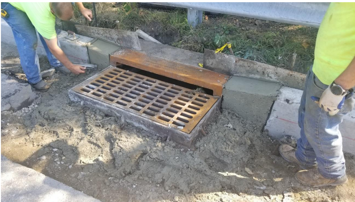
Figure 2. New curb sections and bicycle safe grates placed at Location 1 and 2.
