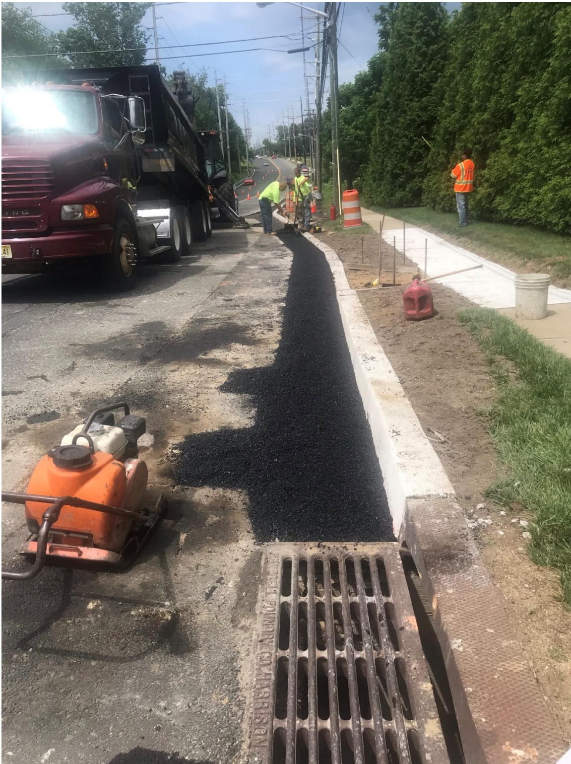
Figure 3. HMA placement along newly installed curb..
