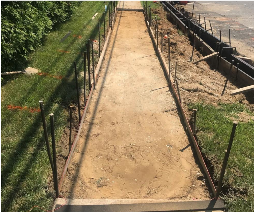
Figure 1. Lexa preparing to place concrete sidewalk and curb.
