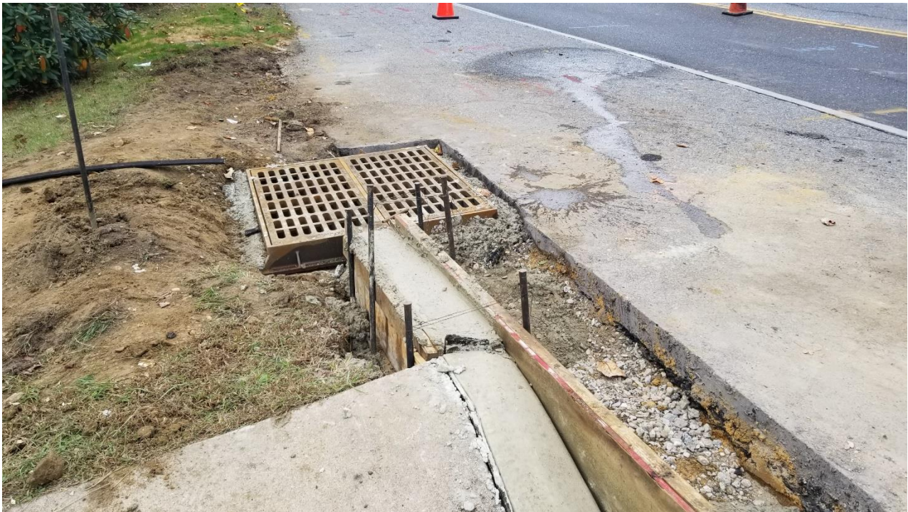
Figure 4. Lexa placed new inlet with bicycle safe grates at Location #4 eastbound.
