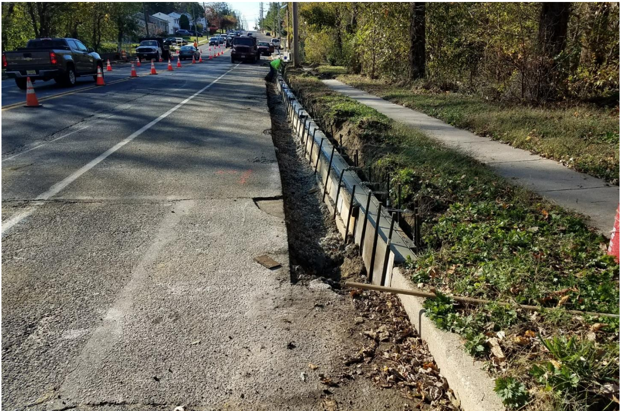
Figure 4. Lexa placing curb at Location #5 westbound.
