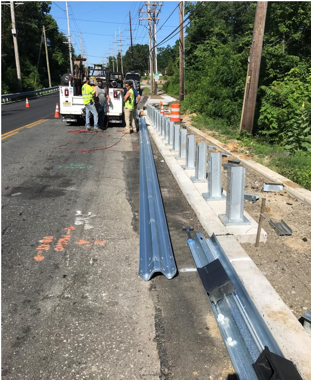
Figure 1. The guiderail subcontractor preparing to install Guiderail at Location #2.
