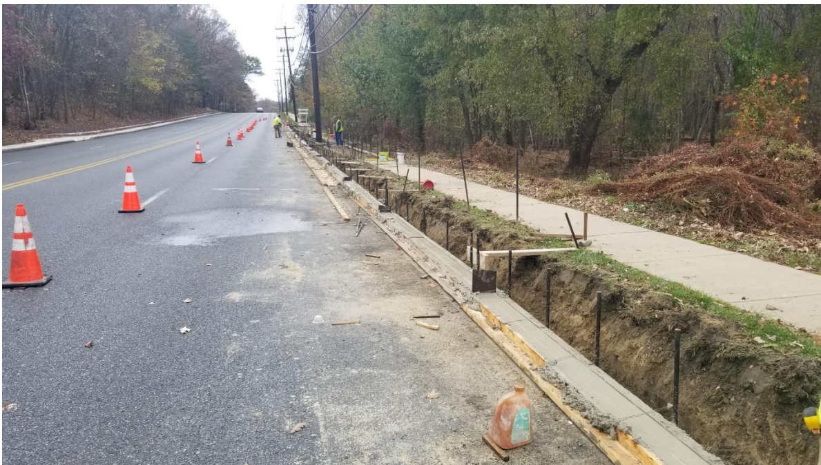
Figure 2. New curb placed at Location 6 westbound.
