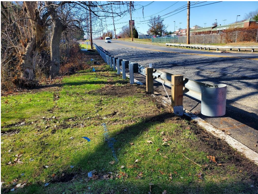
Figure 2. Guide rail placed along curb at Location 1 eastbound.
