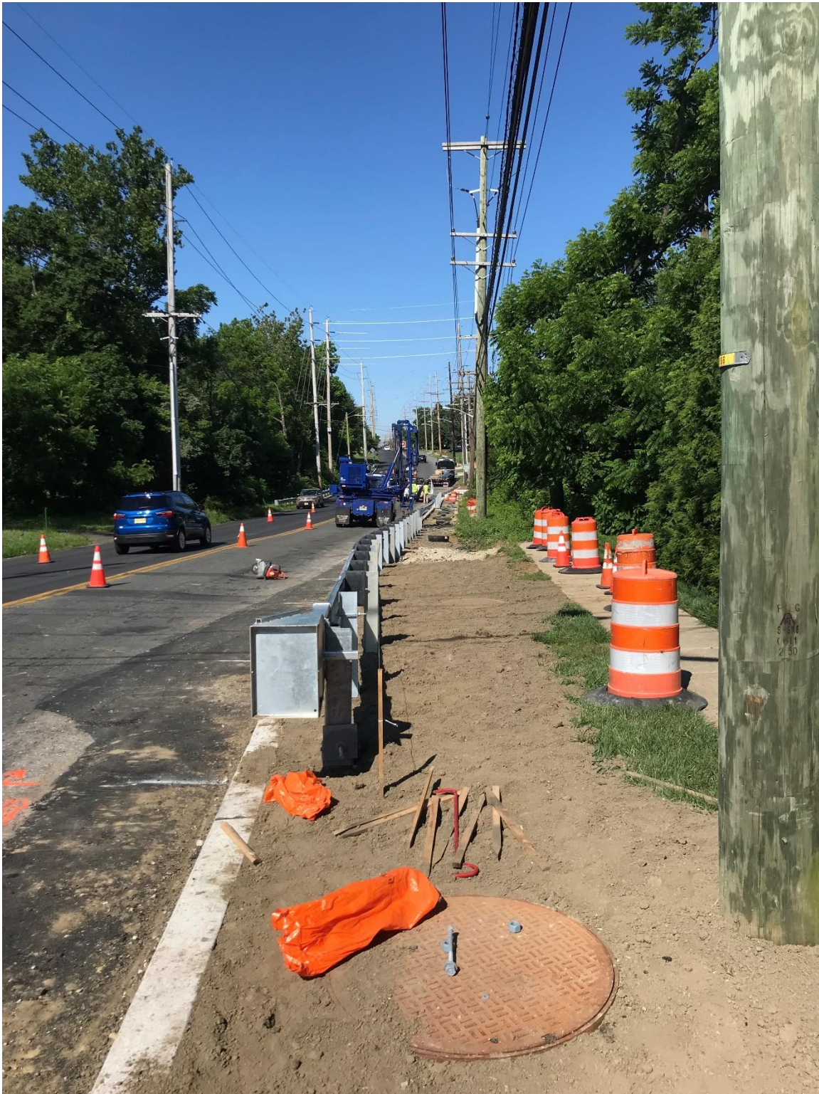
Figure 2. Installation of guiderail at Location #2.
