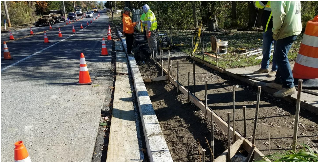
Figure 2. Lexa framing sidewalk subsequent to new curb installation at Location #5 eastbound.
