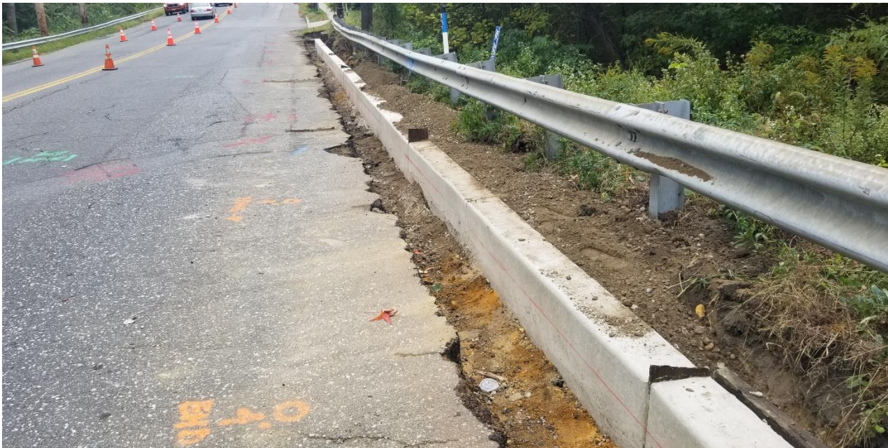
Figure 2. The finished curb following formwork removal.
