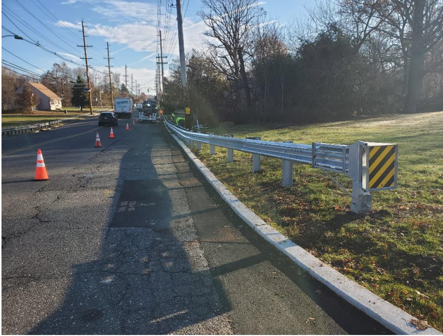
Figure 1. Guide rail placed along curb at Location 1 eastbound.
