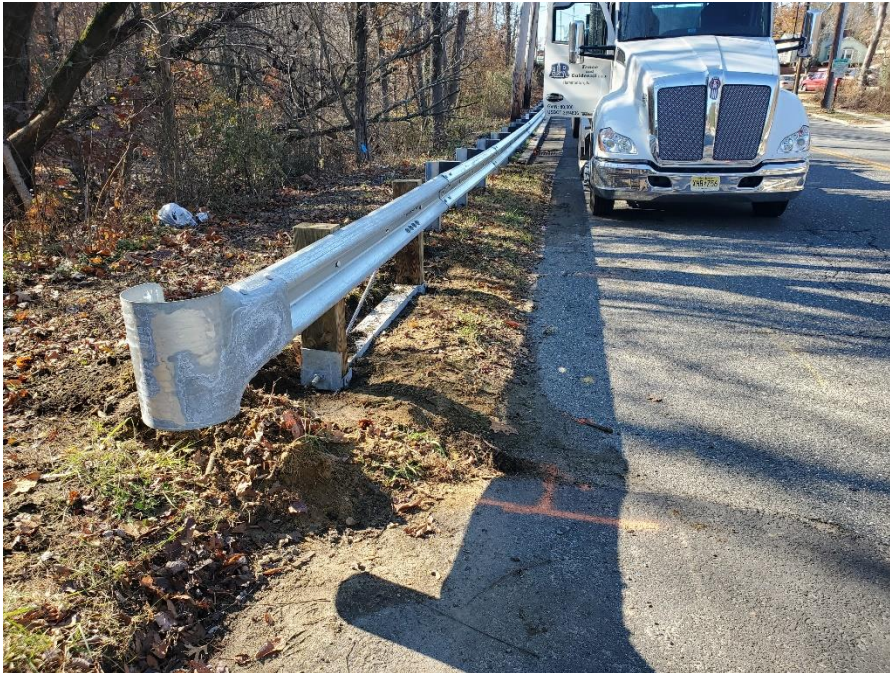
Figure 4. Guide rail placed along curb at Location 2 eastbound.
