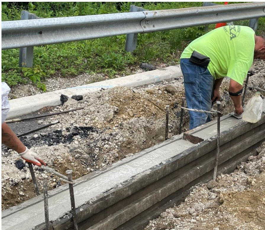
Figure 2. Concrete curb placed along Location #2 westbound.
