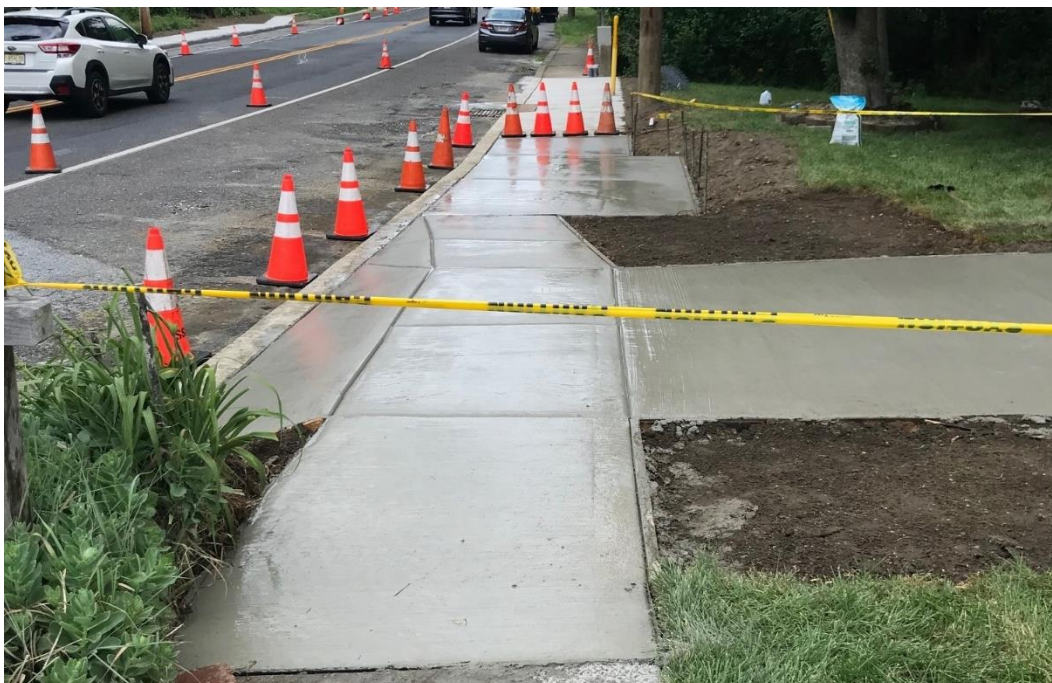
Figure 2. Installation of concrete for sidewalk and driveway apron #5.
