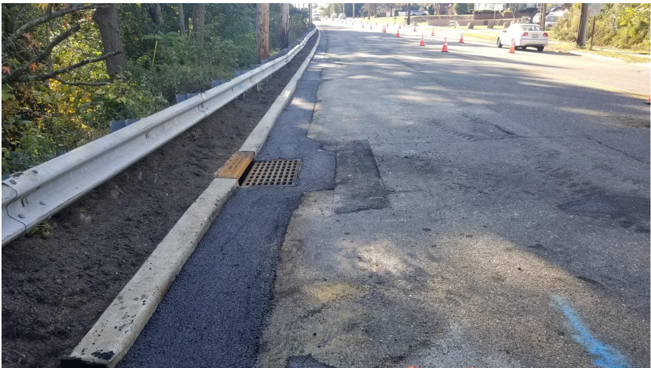
Figure 4. Lexa placed concrete curb at Location #2 eastbound.
