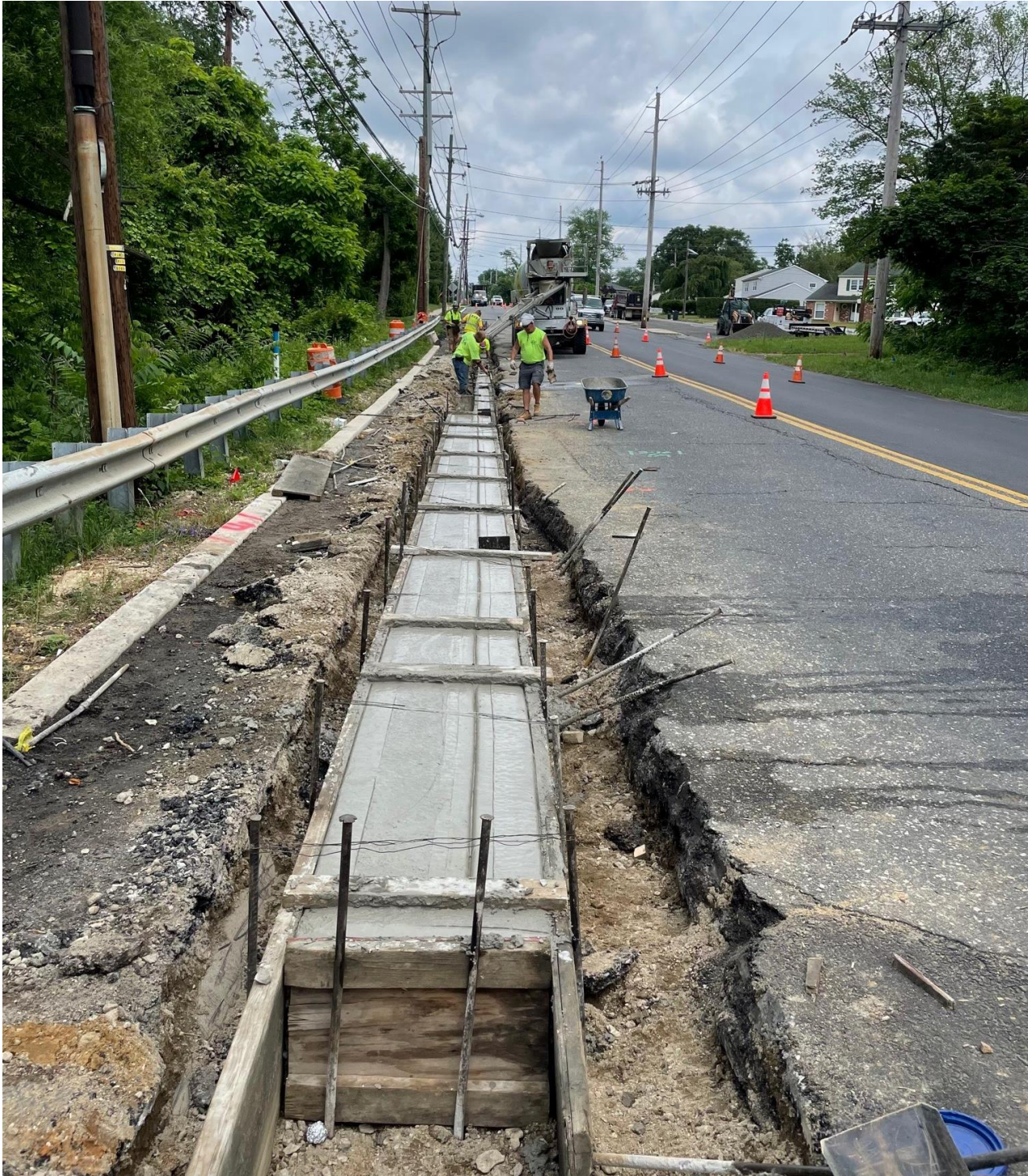
Figure 3. Concrete curb placed along Location #2 westbound.
