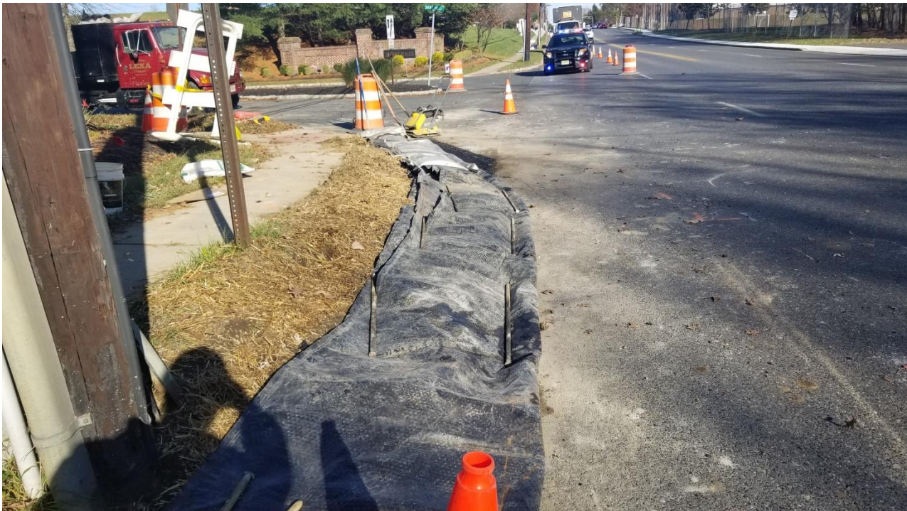
Figure 4. Cold-weather measures used at Location 6 to protect concrete from freezing temperatures.
