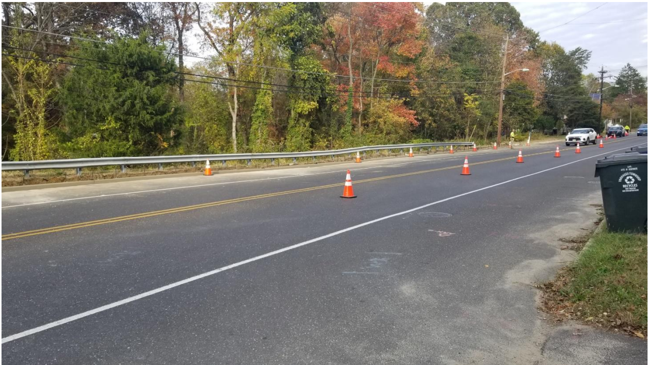
Figure 3. New curb along Location #3 westbound. Sidewalk to be restored.
