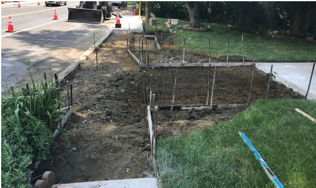
Figure 1. The sidewalk and driveway apron being prepared at Location #5.
