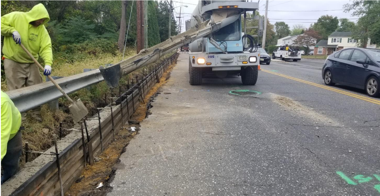
Figure 1. Lexa placed concrete curb at Location #1.
