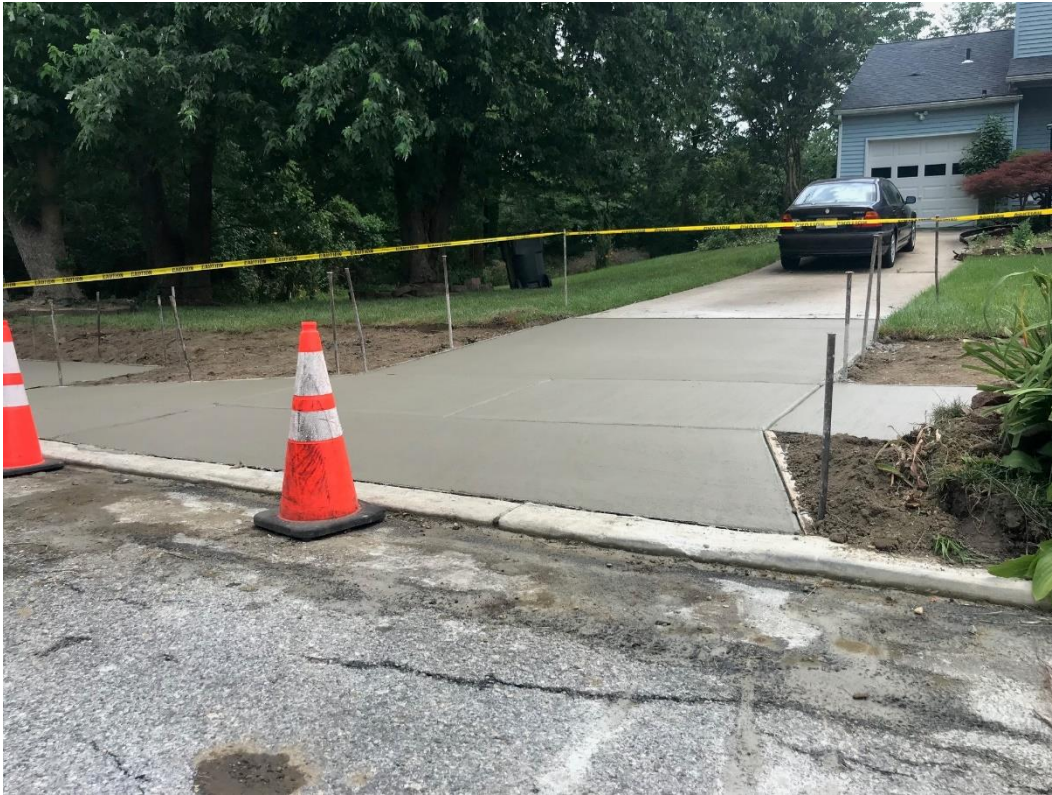
Figure 3. Installation of concrete for sidewalk and driveway apron #5
