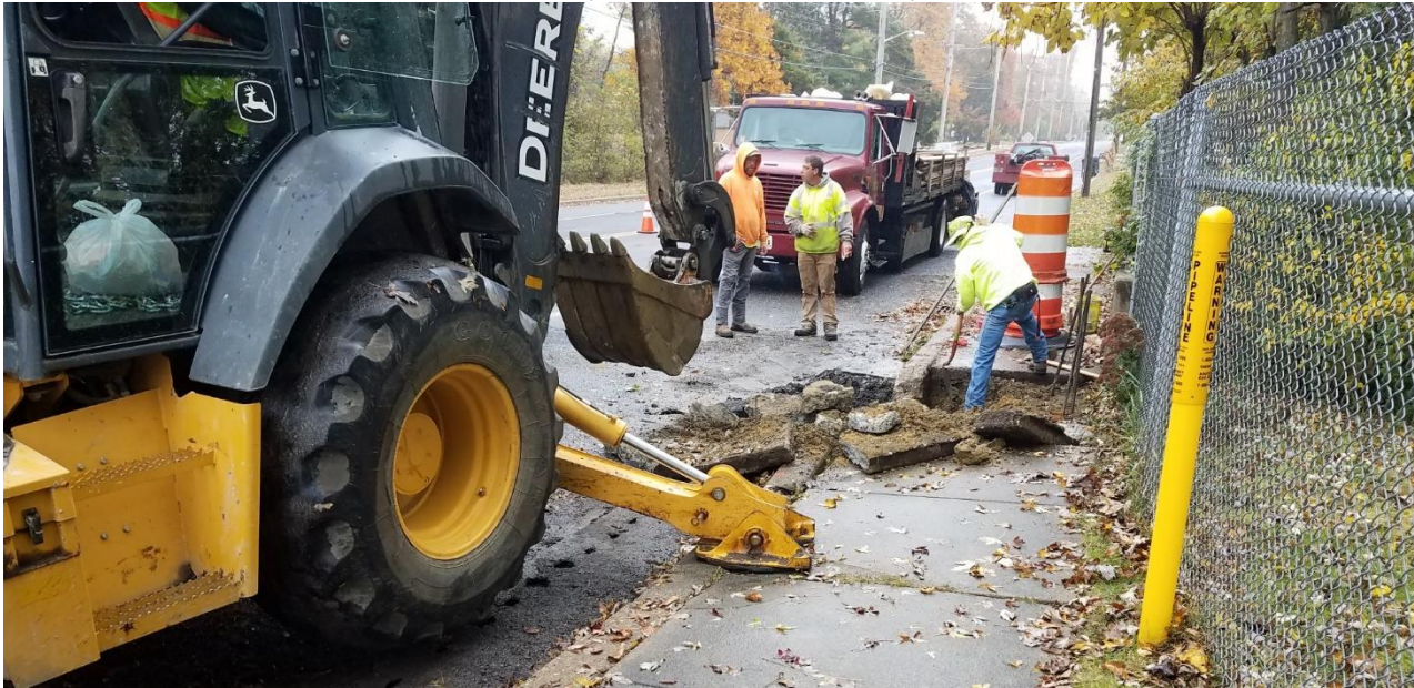
Figure 1. Lexa removing sidewalk at Location #5 eastbound.
