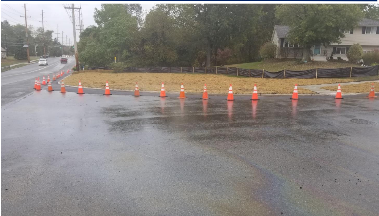
Figure 3. Location #1 eastbound finished.
