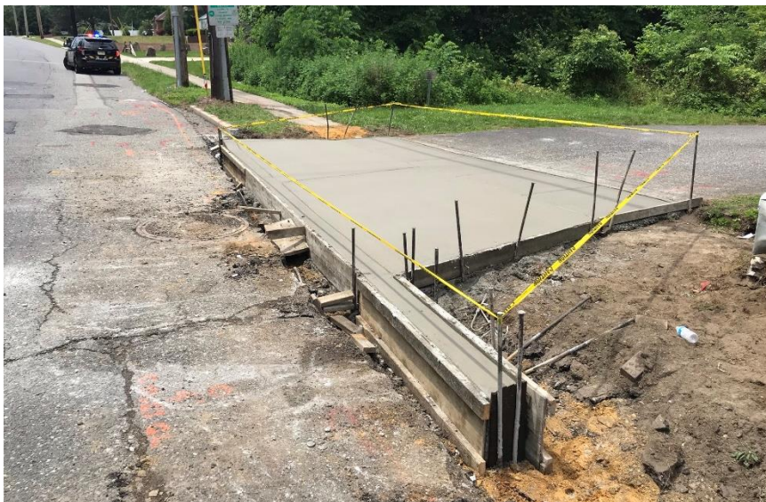
Figure 2. Lexa installed a reinforced concrete driveway apron and curb.
