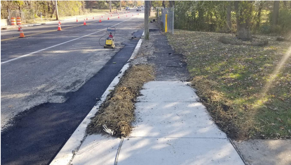
Figure 1. Location 5 eastbound after backfill and asphalt repair..
