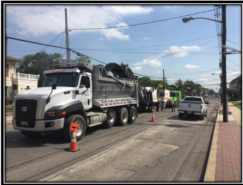
Figure: 1 – HMA milling of the eastbound lane between 42 nd Street and Browning Road
