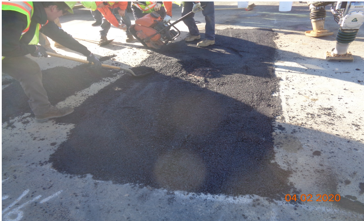
Figure 12: Gas leak was fixed along Sherman Avenue.
