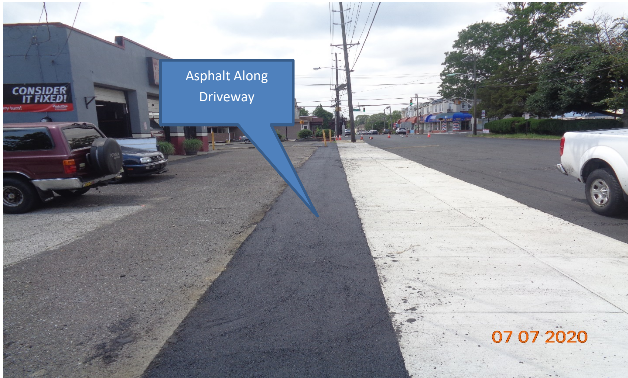
Figure 5: Concrete driveway along Westfield Avenue, RT – Asphalt Along Driveway
