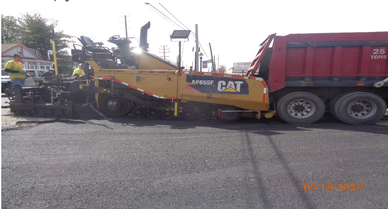
Figure 1: Full depth side street Asphalt Roadway construction along Scovel Avenue LT – Compaction of Subbase course is under progress.
