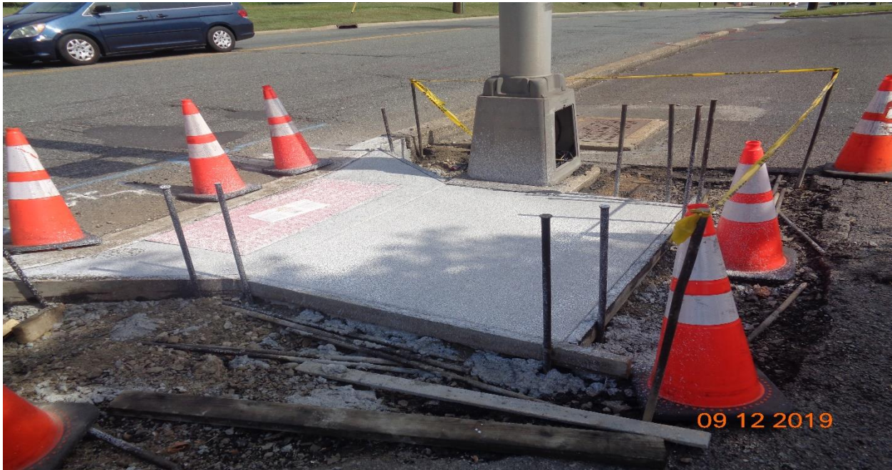
Figure 12: Concrete Curb and Sidewalk along Westfield Ave, STA 124+60 Right
