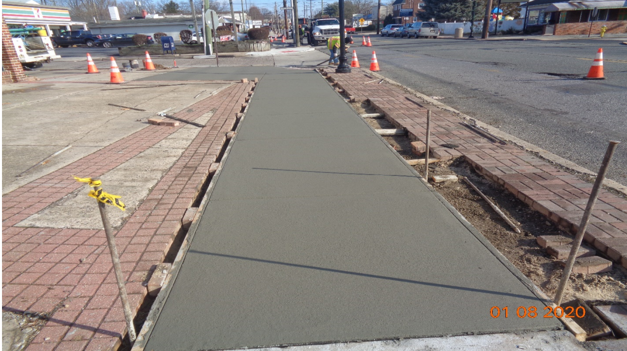
Figure 5: Sidewalk reconstructed over 16" DIP Trench between Hillcrest Avenue and Hollinshead Avenue.
