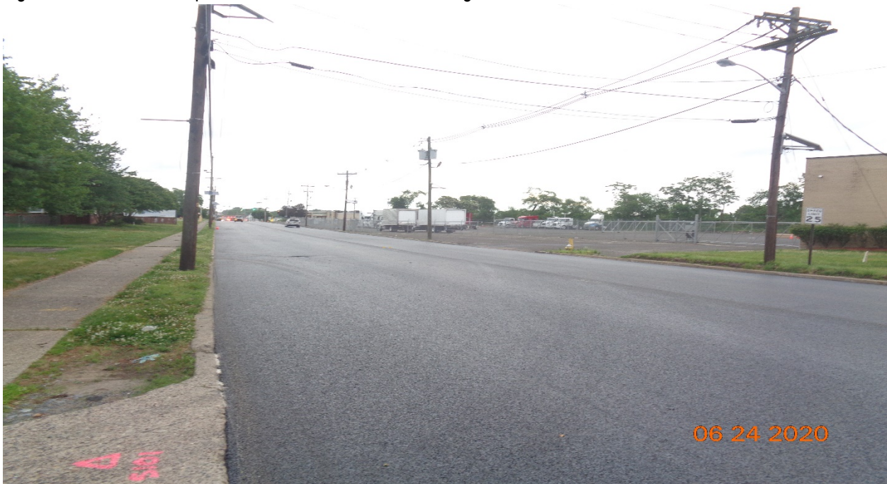
Figure 8: Stone Matrix Asphalt 12.5 MM Surface Course along Westfield Avenue between STA 133+64 – 109+50.
