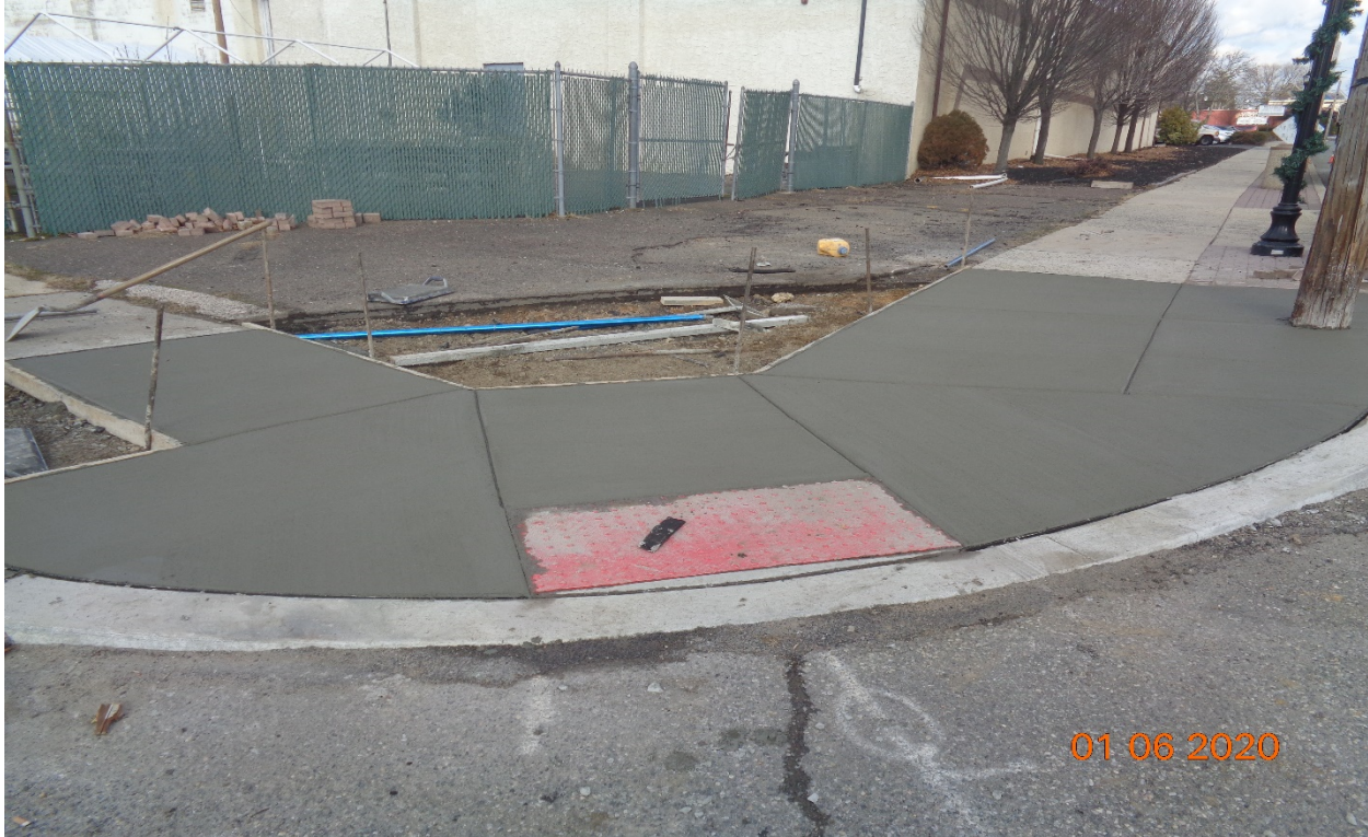
Figure 1: Horner Avenue – East Handicap Ramp was reconstructed.
