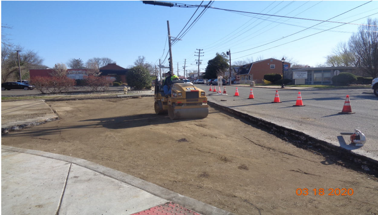
Figure 1: Full depth side street Asphalt Roadway construction along Scovel Avenue LT – Compaction of Subbase course is under progress.
