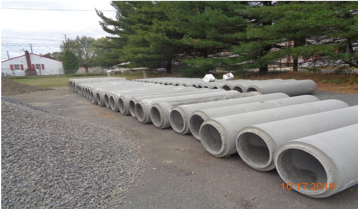
Figure 11: Reinforced Concrete Pipes were delivered at Site.
