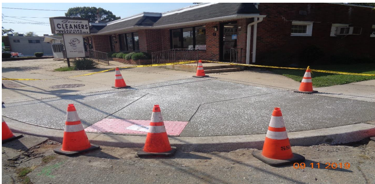
Figure 10: Concrete Curb and Sidewalk along Horner Ave, West
