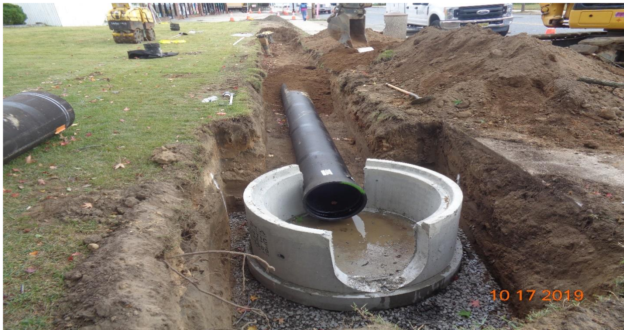
Figure 6: Installation of 16" DIP to Proposed Manhole at Holinshed Avenue
