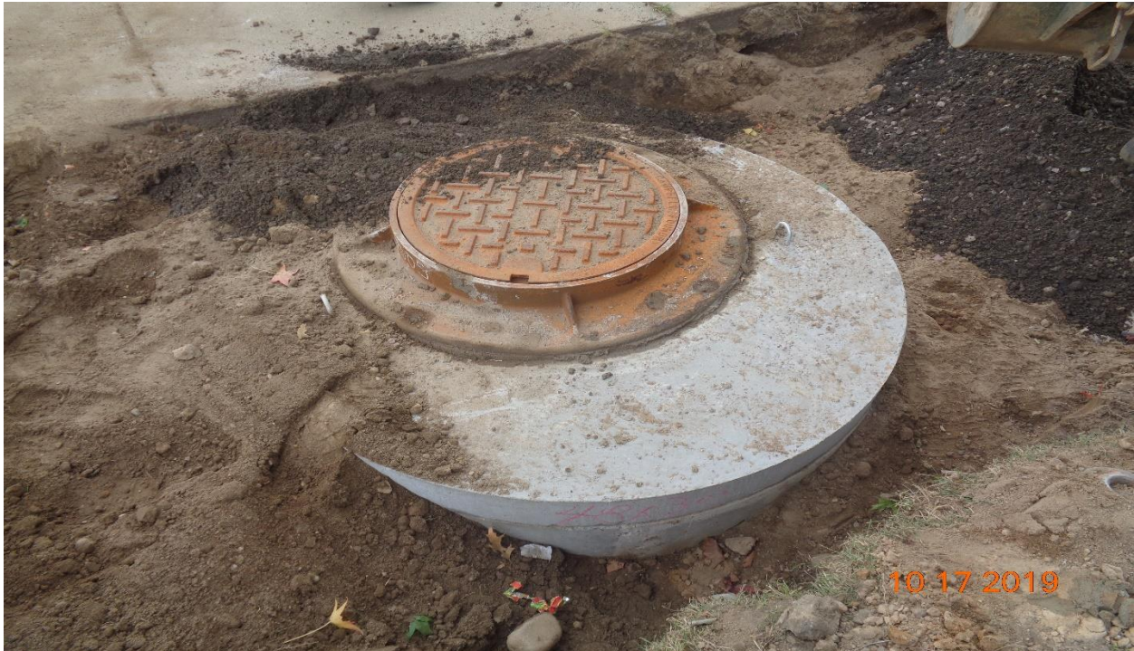
Figure 8: Manhole Cover frame was installed with Manhole Cover
