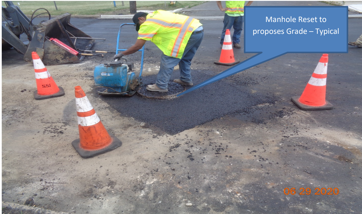
Figure 5: Resting Manhole to proposed grade – Typical
