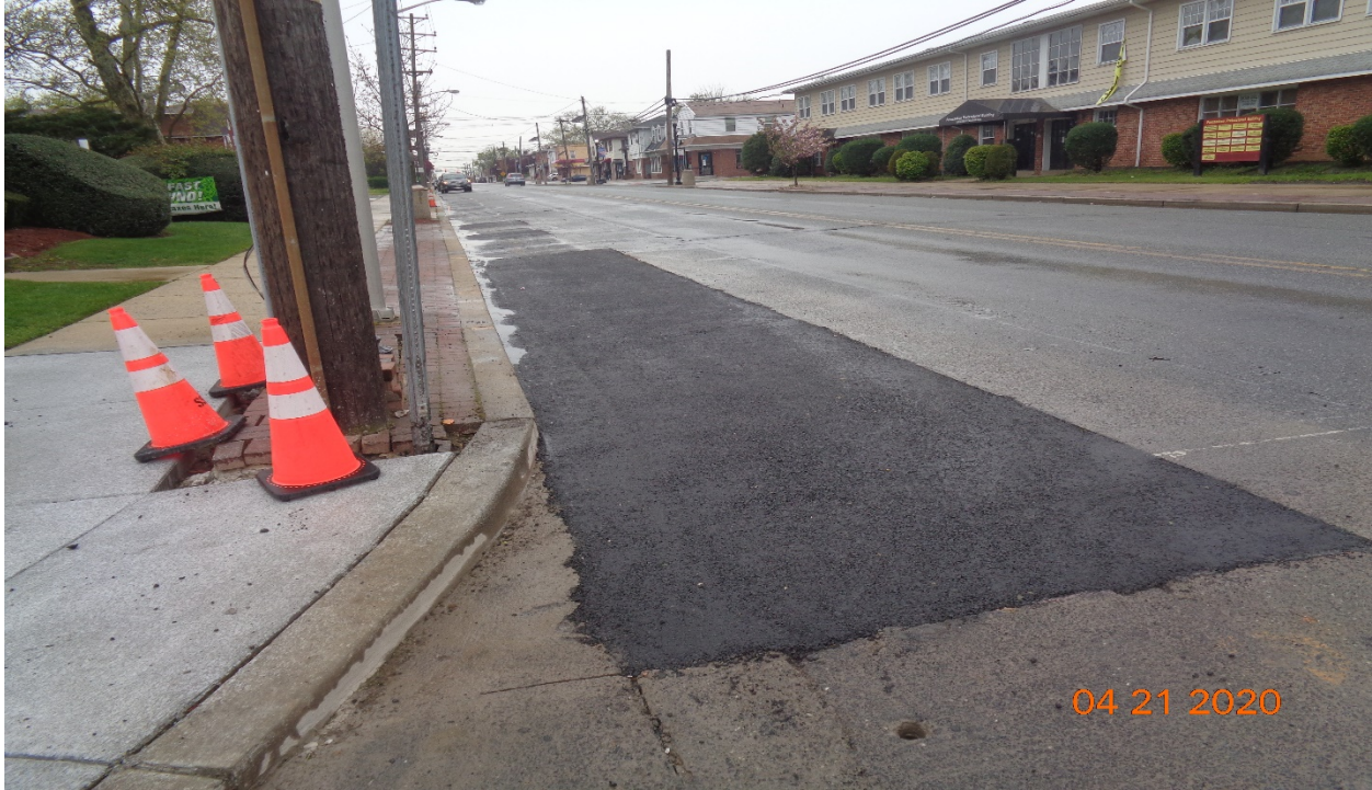
Figure 17: PSE&G Gas – Asphalt was placed for all permanent patch locations.
