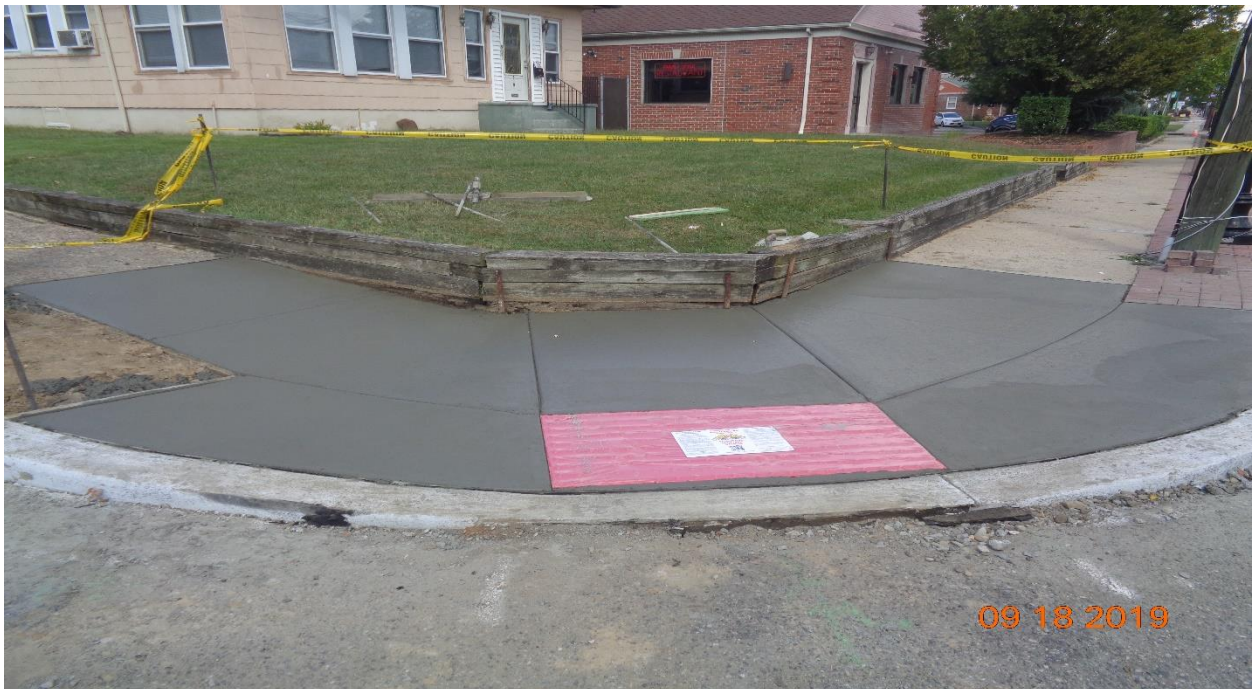
Figure 3: Concrete Curb and Sidewalk along Gross Avenue, East
