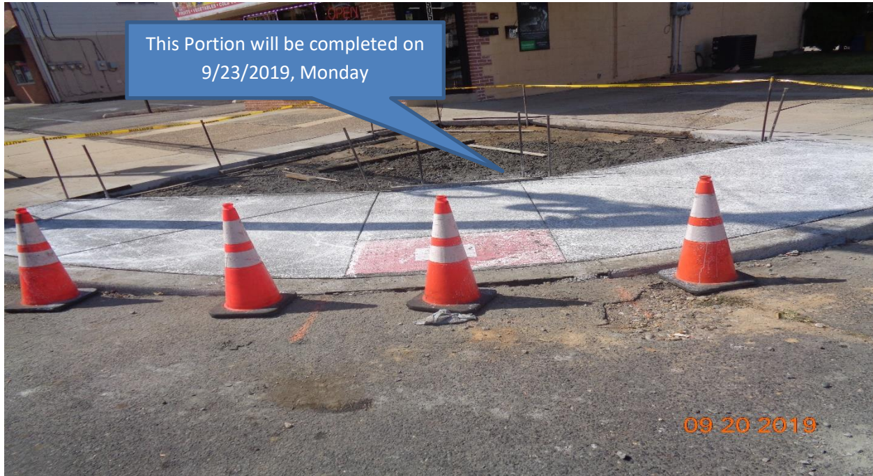
Figure 10: Concrete Curb and Sidewalk along Lexington Avenue, West
