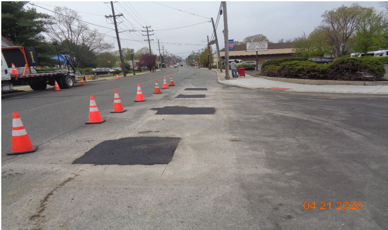
Figure 18: PSE&G Gas – Asphalt was placed for all permanent patch locations.
