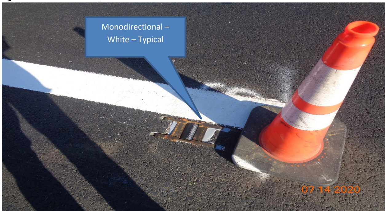
Figure 6: RPM – Monodirectional, White Lens.
