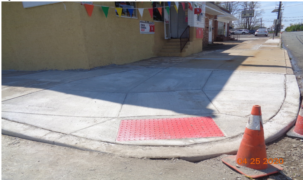
Figure 4: West concrete curb, sidewalk and handicap ramp at Sherman Avenue, RT
