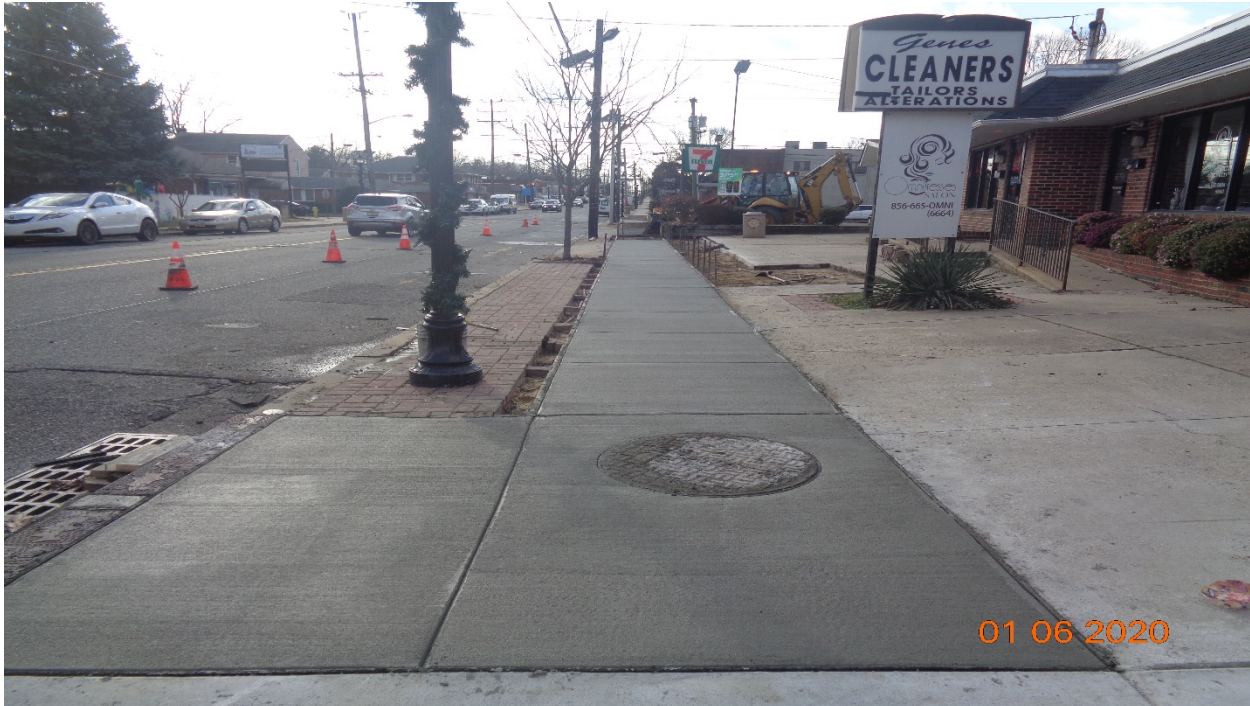
Figure 2: Sidewalk reconstructed over 18" RCP Trench between Horner Avenue and Hillcrest Avenue
