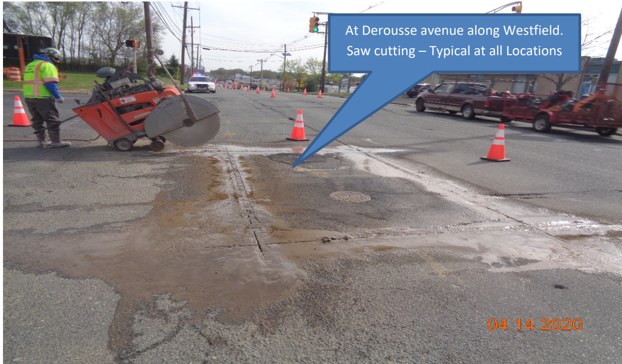
Figure 5: PSE&G Gas – Saw cutting existing concrete pavement for permanent concrete patching.
