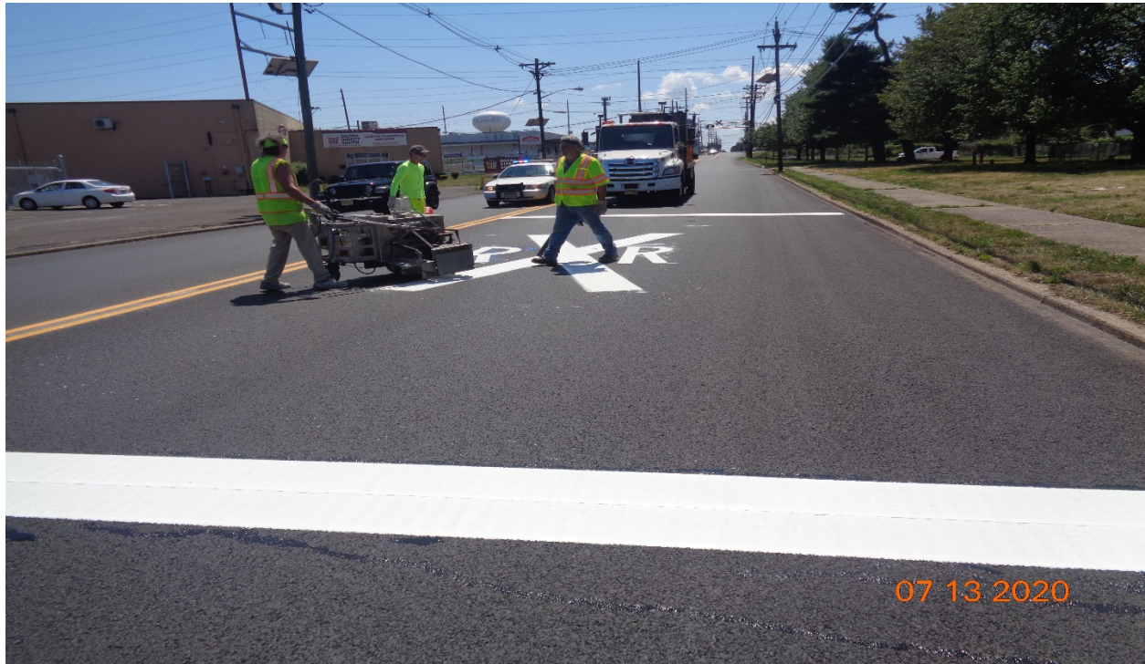
Figure 3: Traffic Markings – RR Crossing
