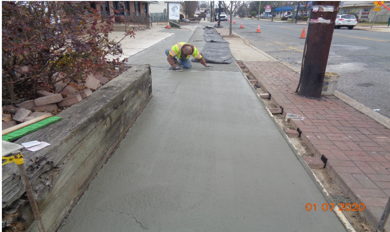
Figure 3: Sidewalk reconstructed over 18" RCP Trench between Horner Avenue and Hillcrest Avenue
