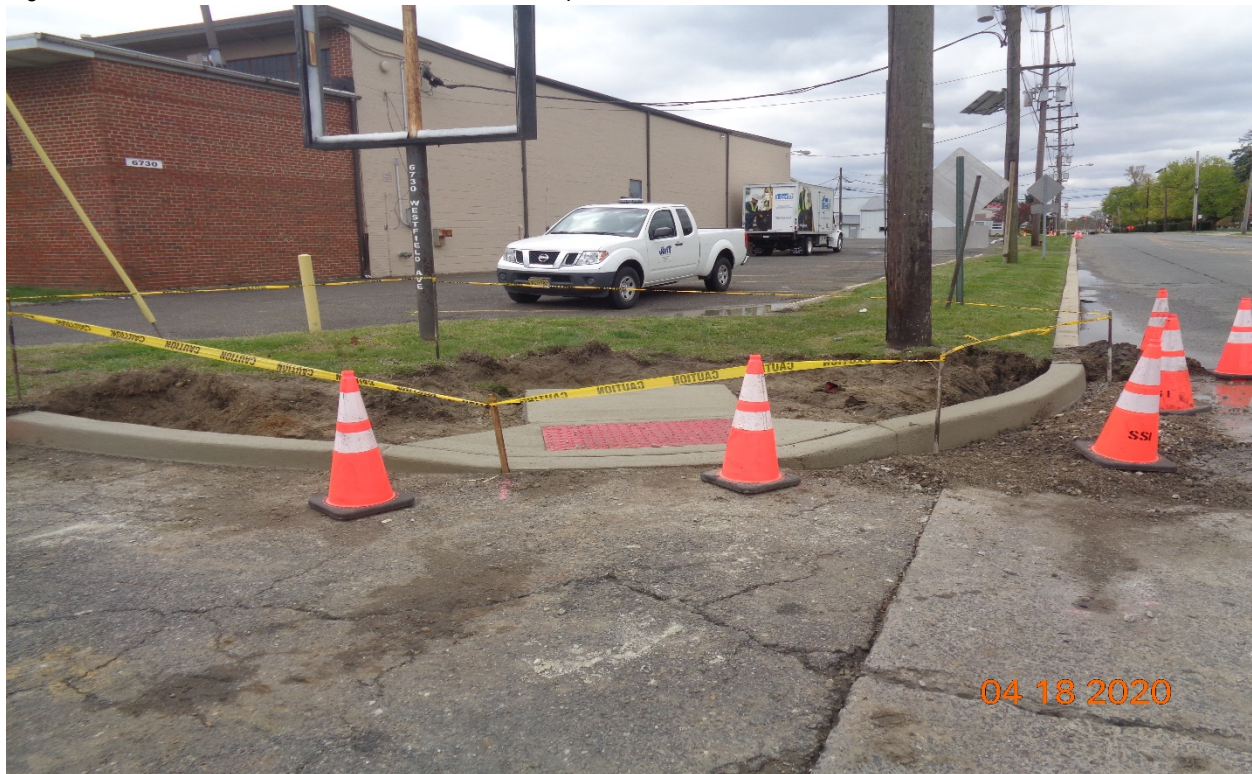
Figure 4: East concrete curb, sidewalk and HC Ramp at Clements Avenue, RT
