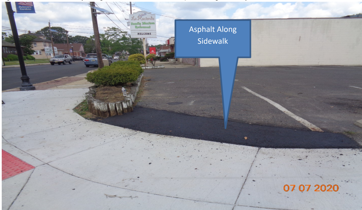
Figure 6: East Concrete sidewalk along Merchantville Avenue, RT – Asphalt Along Sidewalk
