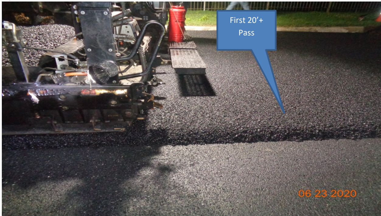
Figure 4: Stone Matrix Asphalt 12.5 MM Surface Course along Westfield Avenue between STA 133+64 – 109+50.
