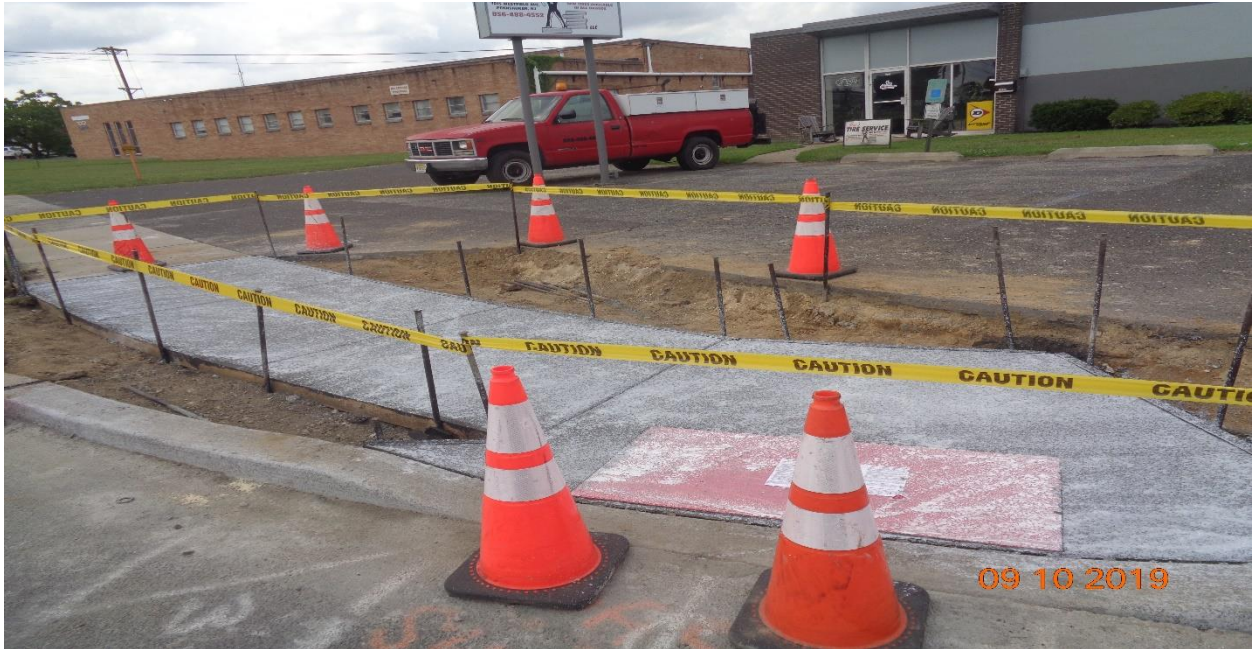
Figure 7: Concrete Curb and Sidewalk along Sherman Ave, West side
