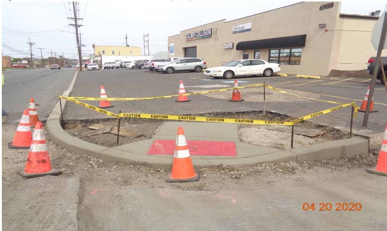
Figure 2: East concrete curb, sidewalk and handicap ramp at Bethel Avenue, RT
