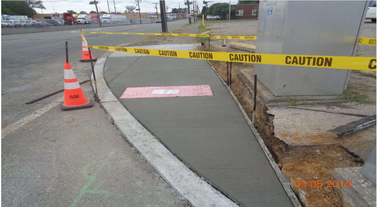
Figure 1: Concrete Curb and Sidewalk Along Derosse Avenue, West
