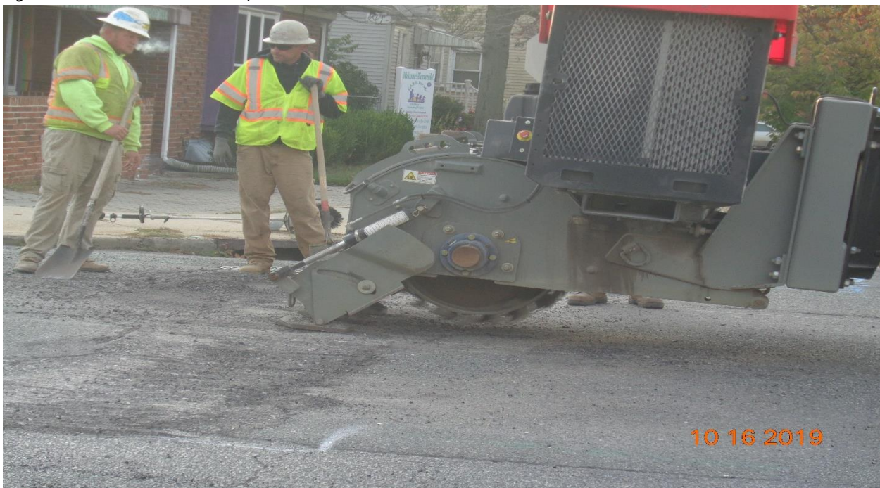
Figure 12: Grinding Humps along Westfield Avenue
