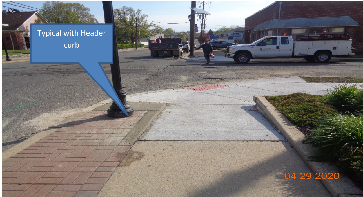
Figure 11: Resetting existing brick pavers along proposed sidewalk and existing brick pavers
