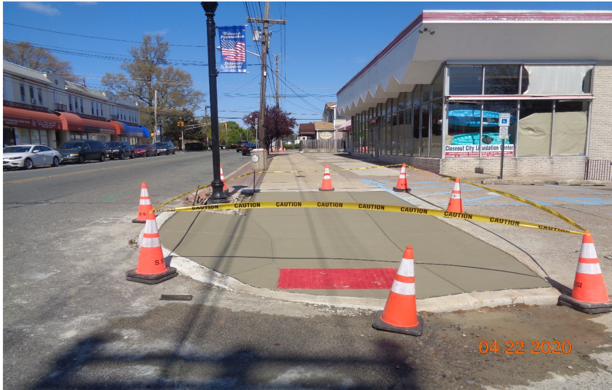
Figure 7: East concrete curb, sidewalk and handicap ramp at Penn Street, RT
