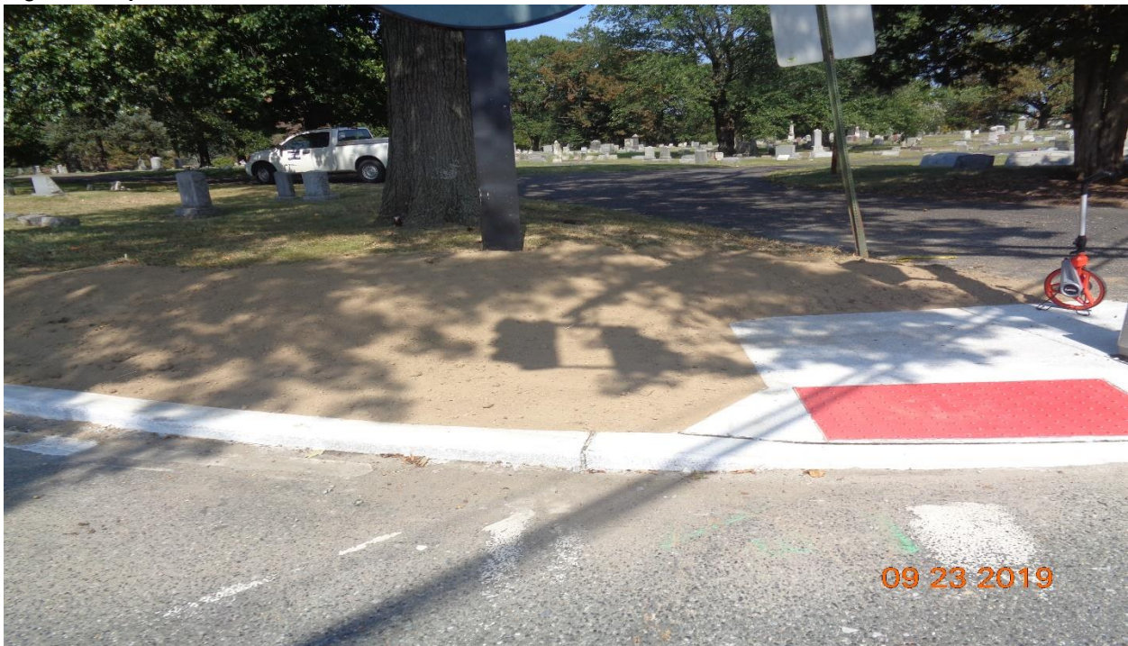
Figure 7: Topsoil around Curb and Sidewalk along Cove Road, East
