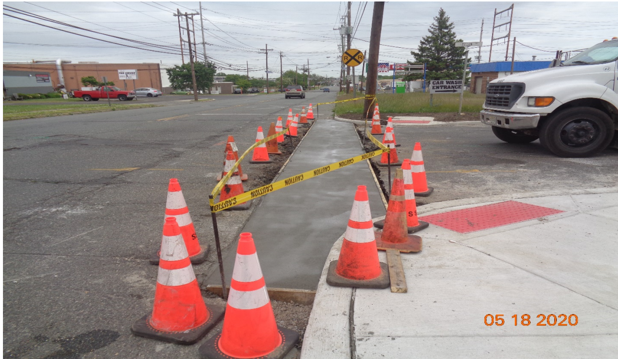
Figure 1: Concrete gutter along Westfield Avenue, RT at Sherman Avenue
