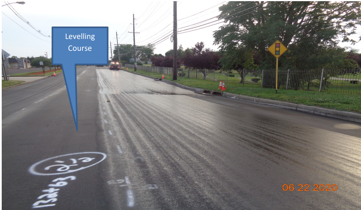
Figure1: Stone Matrix Asphalt 12.5 MM Surface Course along Westfield Avenue between STA 133+64 – 109+50.
