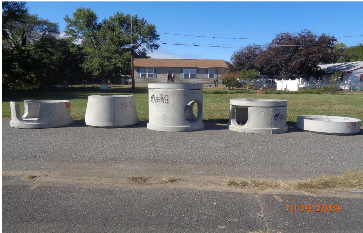
Figure 1: Drainage structures were delivered at site on 10/10/2019.
