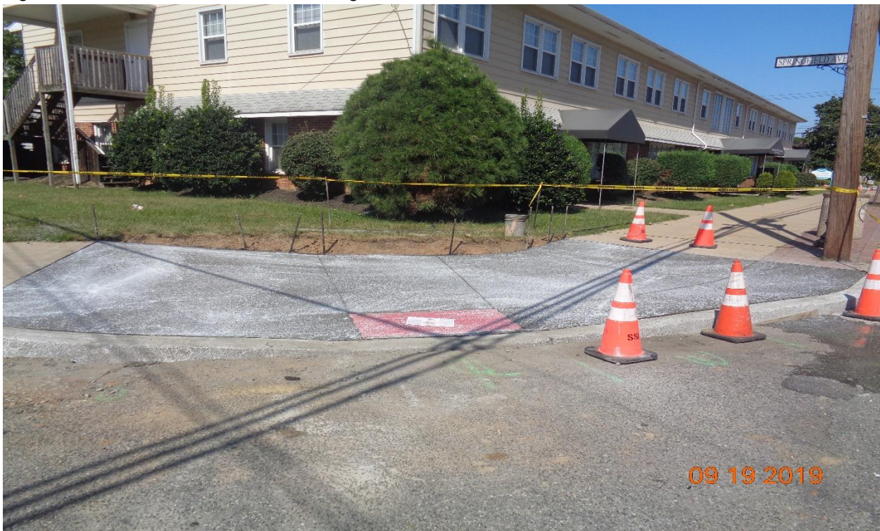
Figure 7: Concrete Curb and Sidewalk along Springfield Avenue, West
