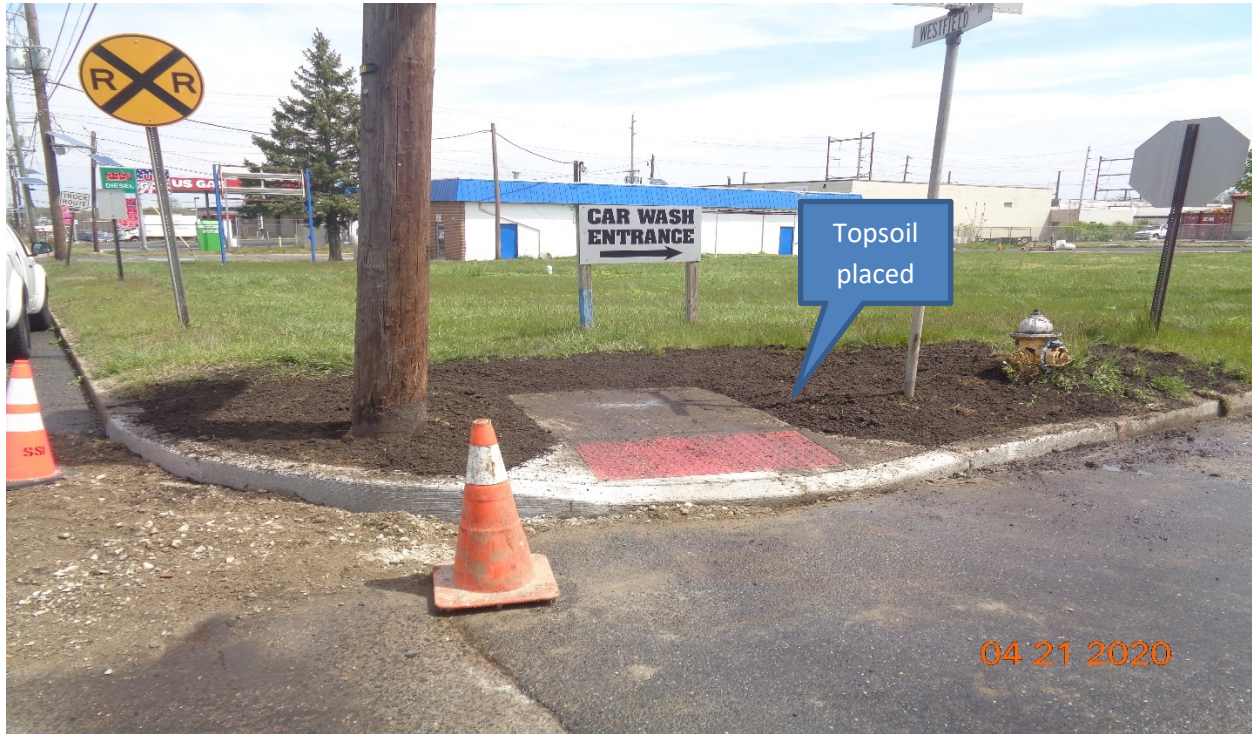
Figure 3: East concrete curb, sidewalk and handicap ramp at Sherman Avenue, RT
