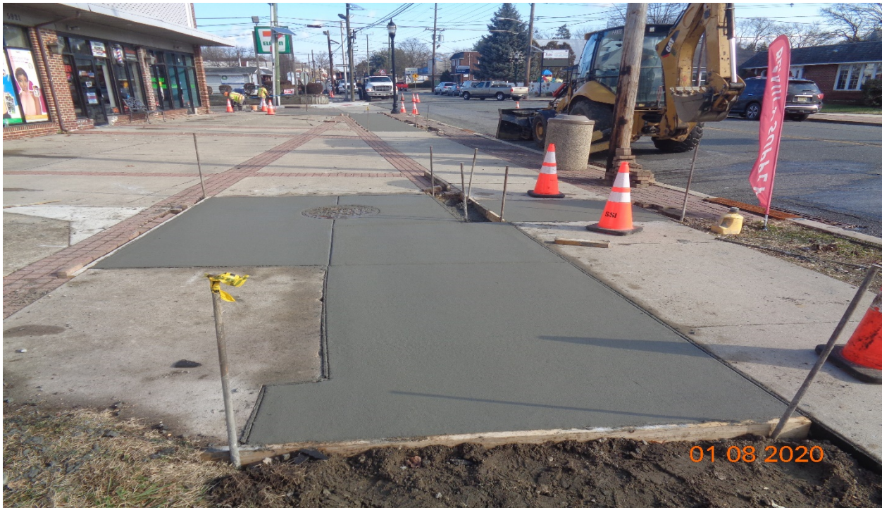
Figure 6: Sidewalk reconstructed over 16" DIP Trench between Hillcrest Avenue and Hollinshead Avenue.
