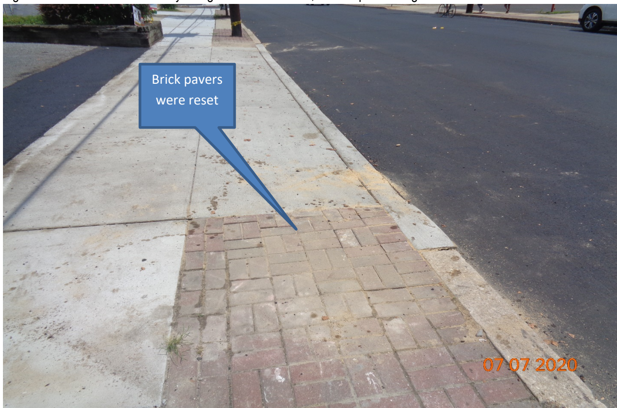
Figure 8: Concrete driveway at Seven Eleven, LT - Brick pavers were reset at both side of driveway.
