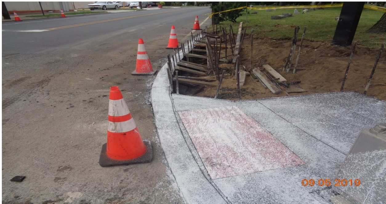
Figure 4: Concrete Curb and Sidewalk along Cove Road, East
