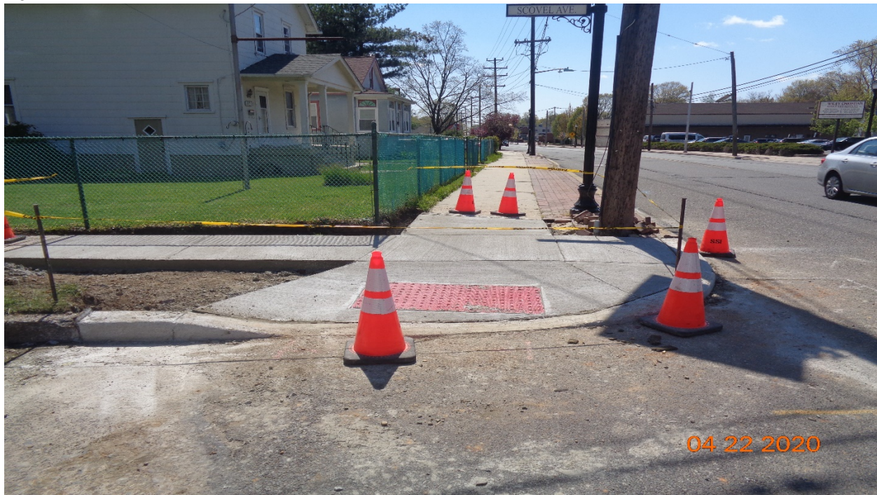
Figure 6: West concrete curb, sidewalk and handicap ramp at Scovel Avenue, RT
