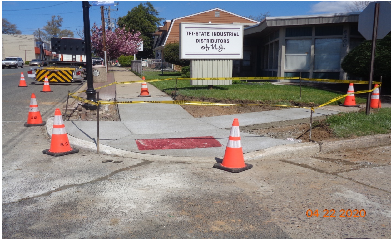
Figure 5: East concrete curb, sidewalk and handicap ramp at Scovel Avenue, RT
