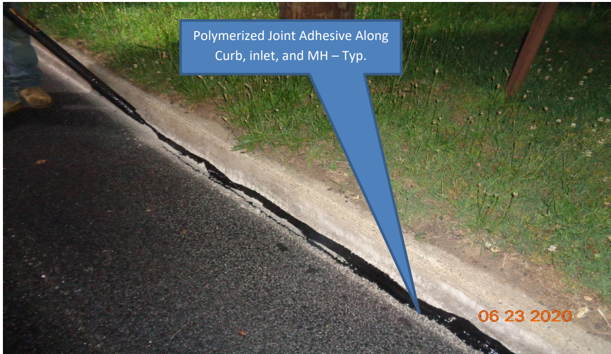
Figure 3: Stone Matrix Asphalt 12.5 MM Surface Course along Westfield Avenue between STA 133+64 – 109+50.
