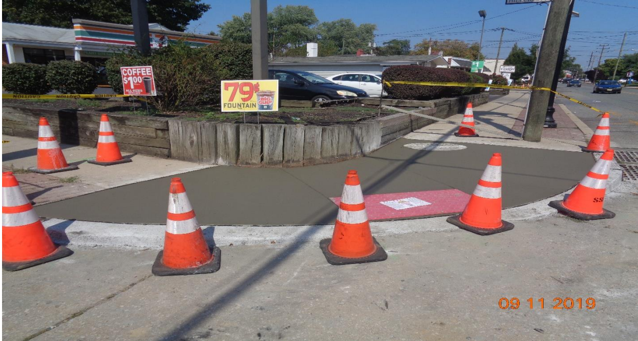
Figure 11: Concrete Curb and Sidewalk Along Hollinshead Ave, East
