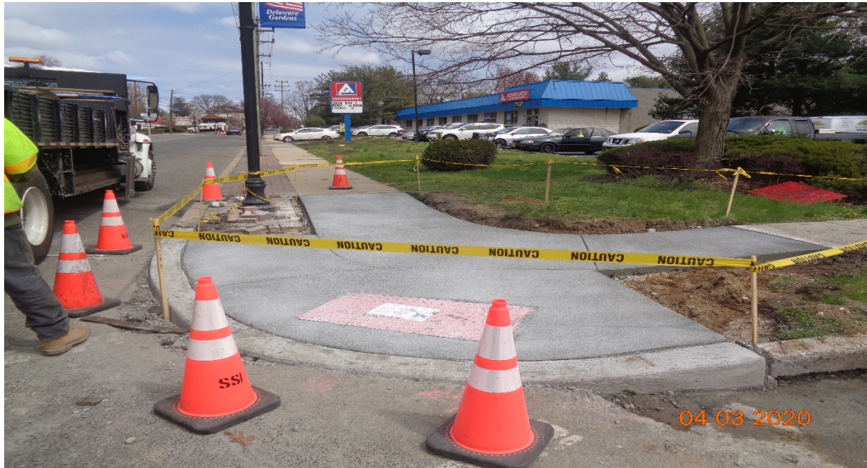
Figure 9: West Concrete curb, sidewalk and HC Ramp at Horner Avenue along Westfield Avenue, RT.
