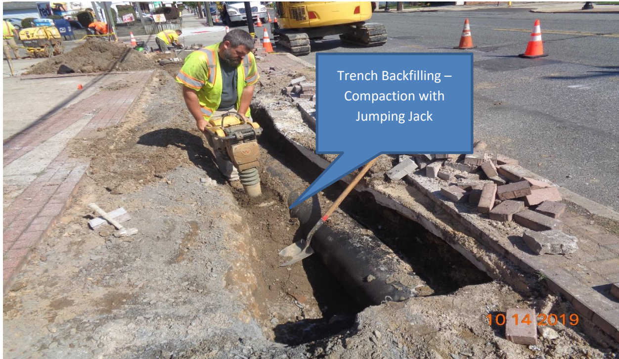
Figure 3: Installation of 16" Ductile Iron Pipe from Inlet on Hillcrest Avenue to Inlet along Westfield Avenue, LT
