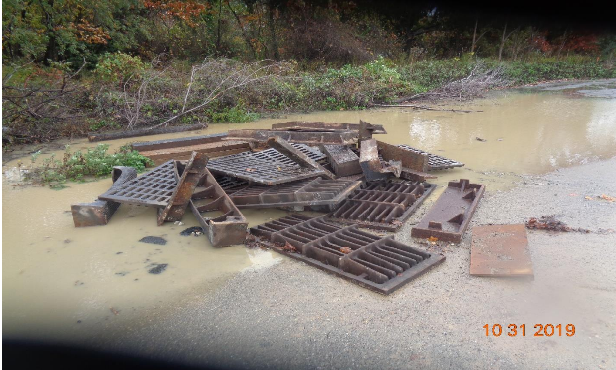
Figure 9: Existing castings and curb pieces were stockpiled at laydown yard.
