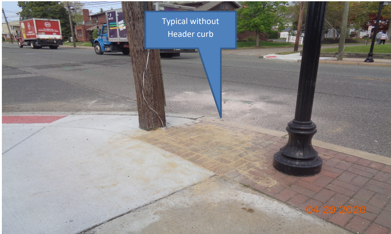
Figure 12: Resetting existing brick pavers along proposed sidewalk and existing brick pavers
