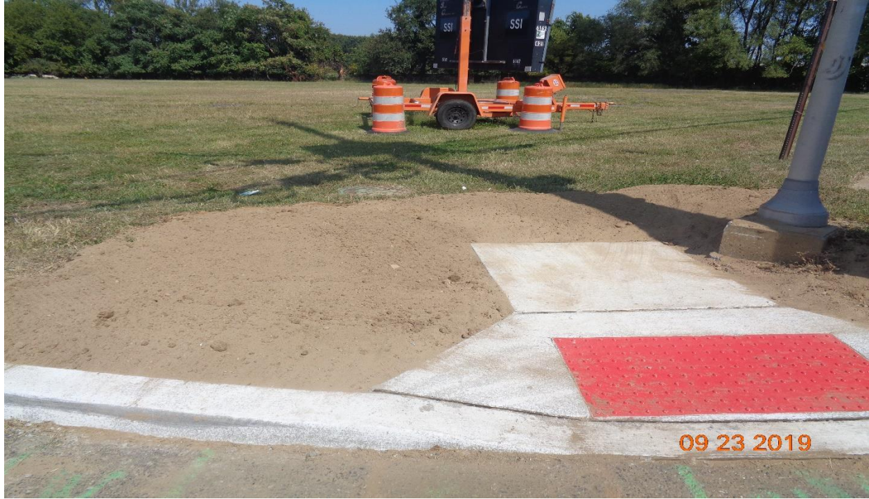
Figure 2: Topsoil placement around Curb and Sidewalk at Derosse Avenue, East
