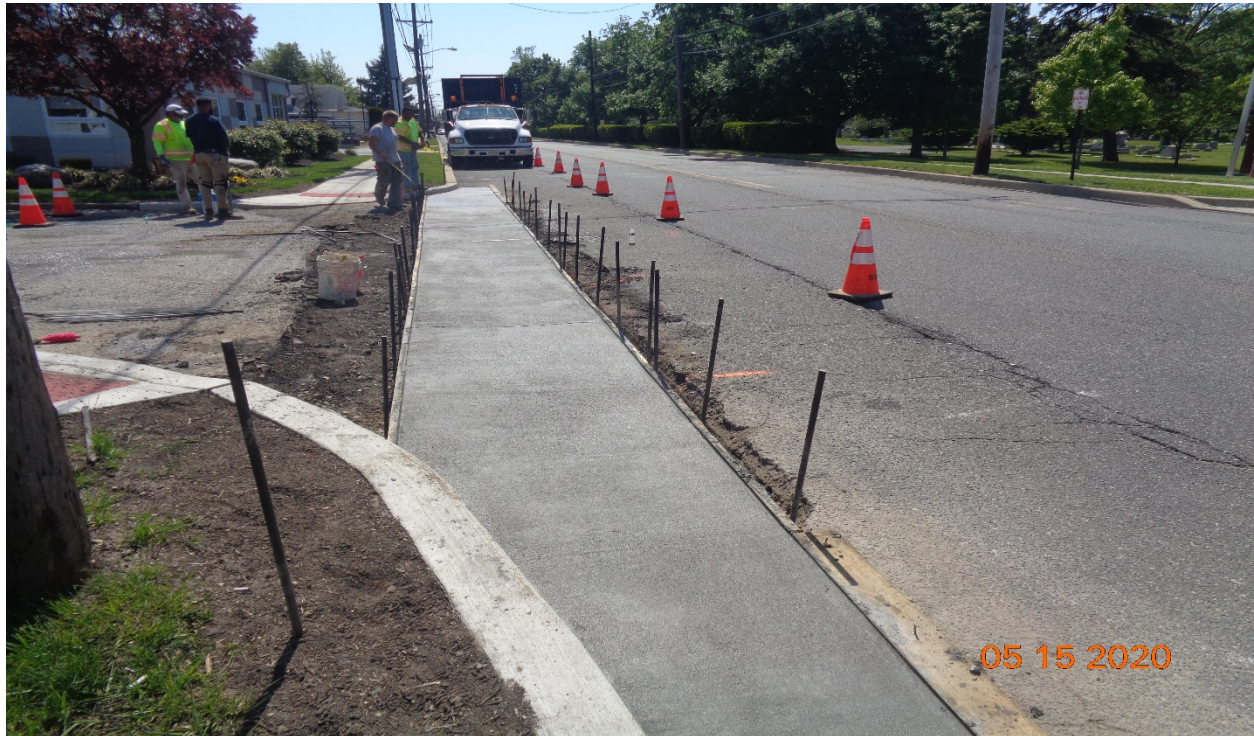
Figure 1: Concrete gutter along Westfield Avenue, RT at Norwood Avenue.
