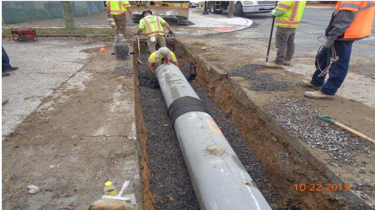
Figure 3: 15" Reinforced Concrete Pipe, Class IV was installed across Horner Avenue, LT.
