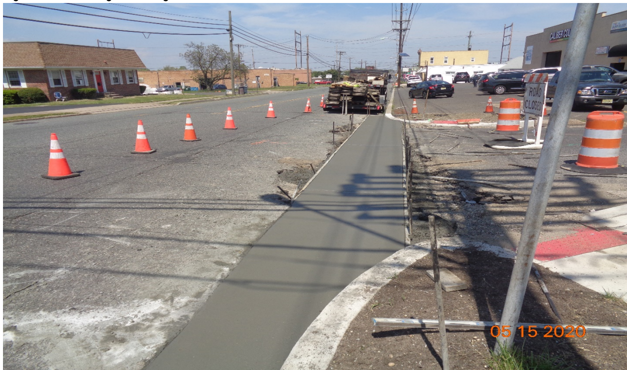
Figure 2: Concrete gutter along Westfield Avenue, RT at Bethel Avenue.
