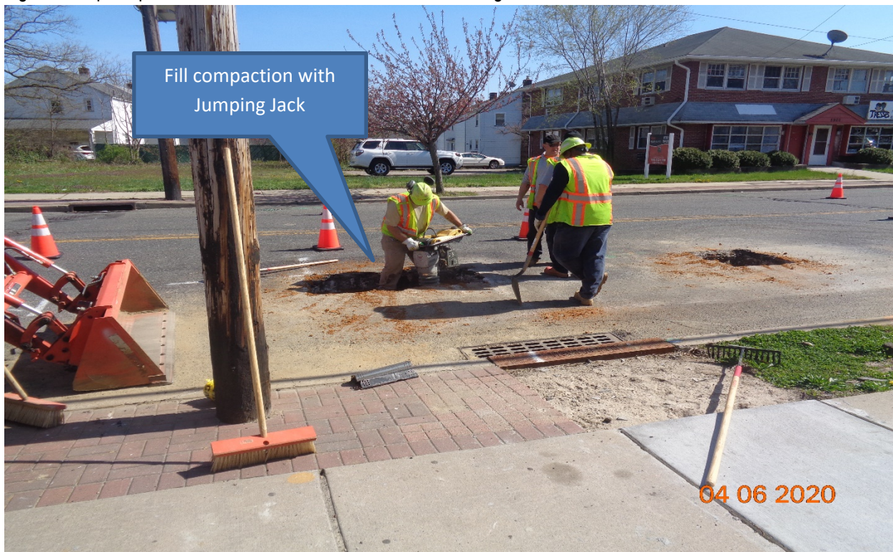
Figure 2: PSE&G Gas – leak fixed along Westfield Avenue at Hillcrest Avenue.
