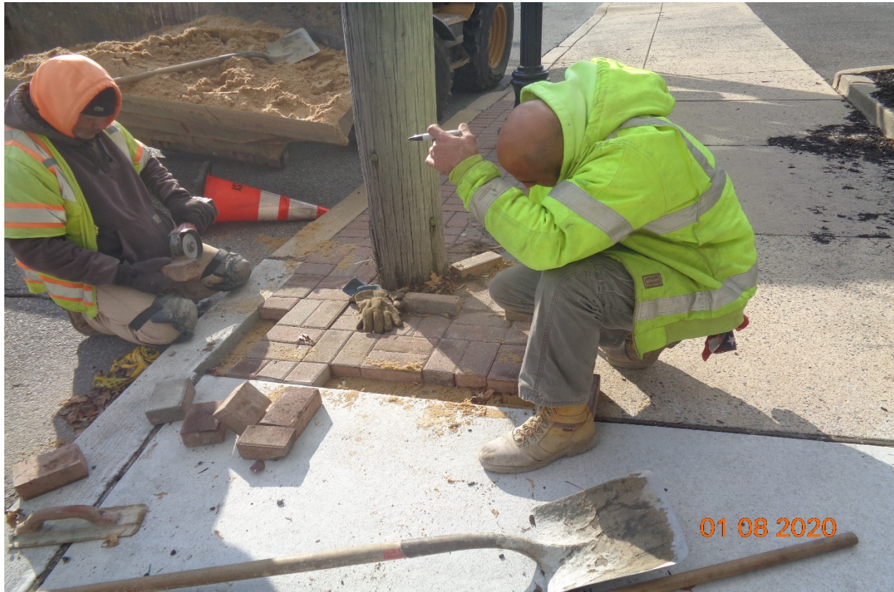
Figure 7: Scovel Avenue West – Resetting existing brick pavers.
