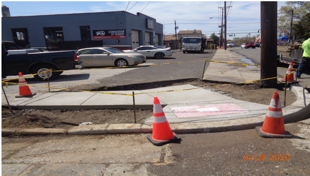
Figure 10: West concrete curb, sidewalk and handicap ramp at Marlon Avenue, RT
