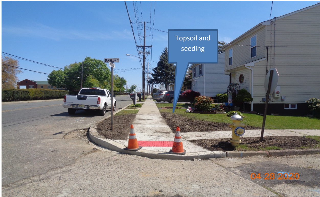
Figure 8: Topsoil and seeding along East sidewalk at Marlon Avenue, RT
