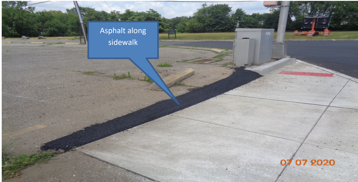
Figure 7: West Concrete driveway along Derousse Avenue, LT – Asphalt Along sidewalk
