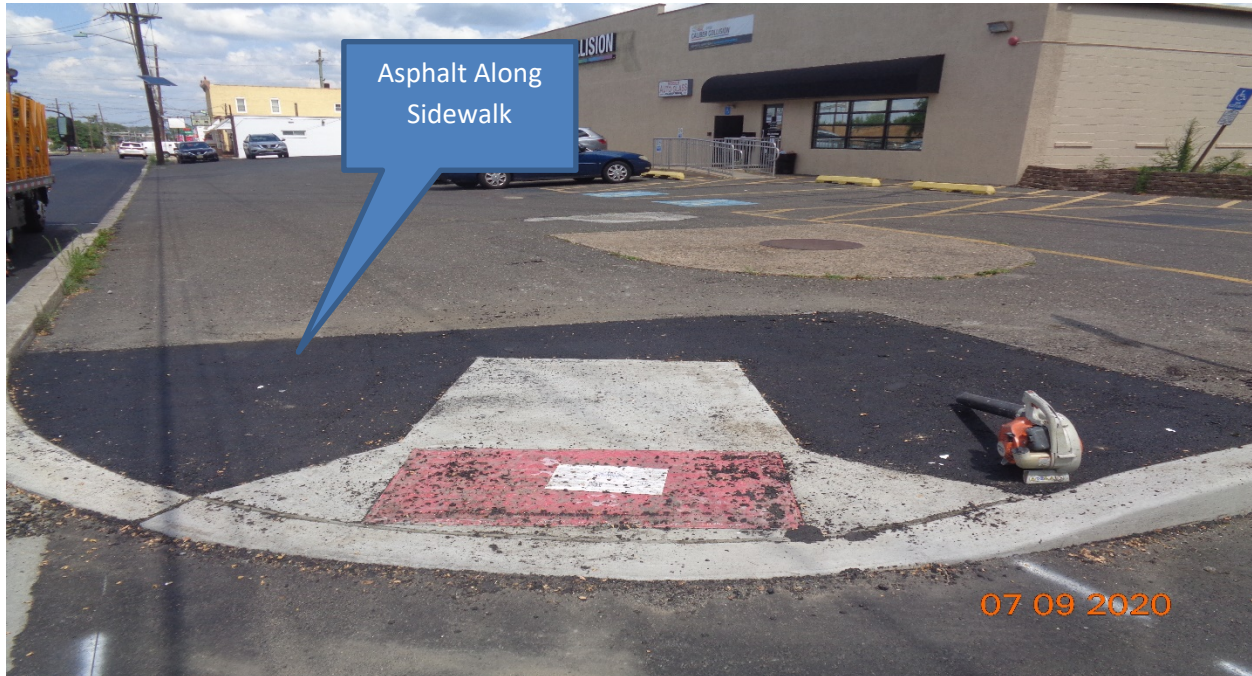
Figure 9: East Concrete sidewalk along Bethel Avenue, RT – Asphalt along sidewalk
