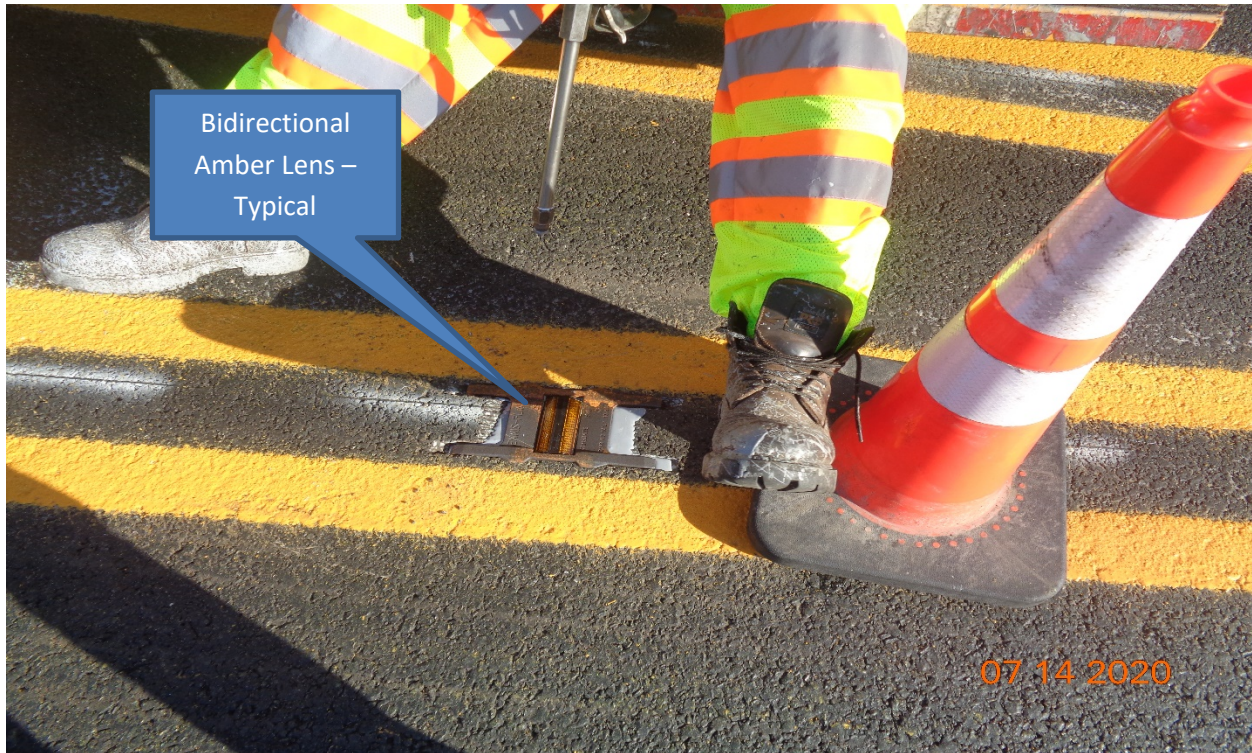
Figure 5: RPM – Bidirectional, Amber lens.
