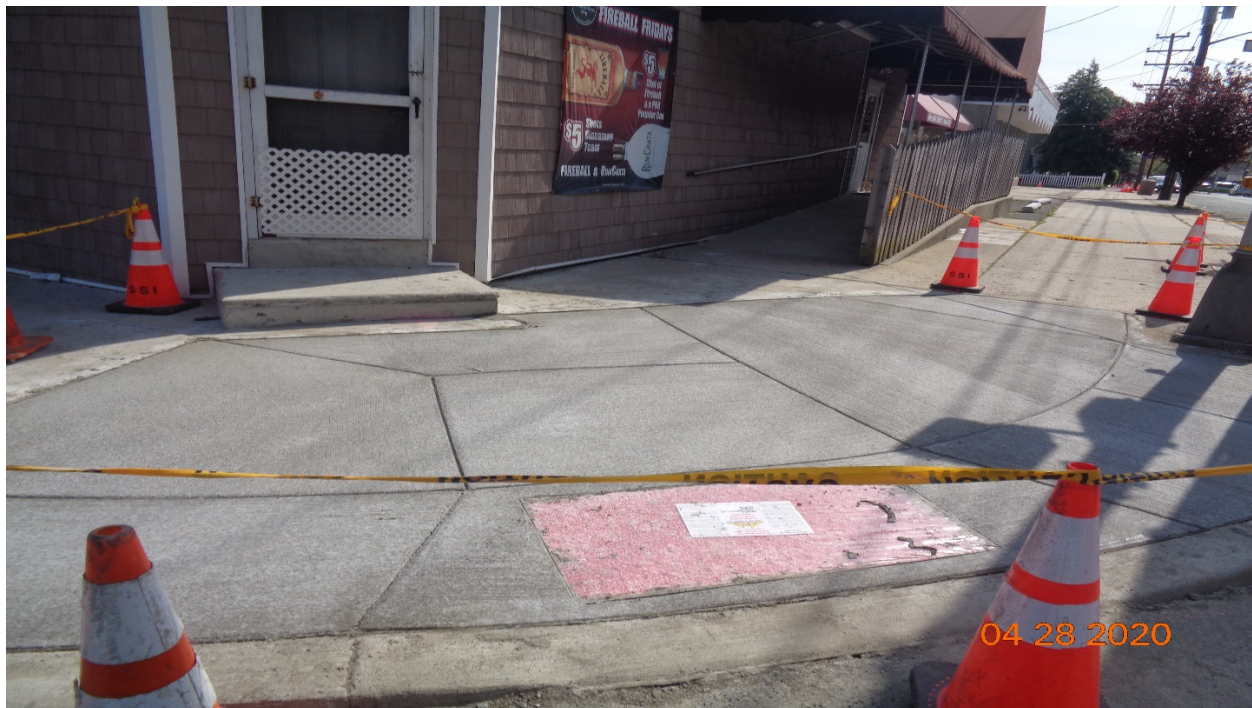
Figure 2: West concrete curb, sidewalk and HC Ramp at Cove Road, RT
