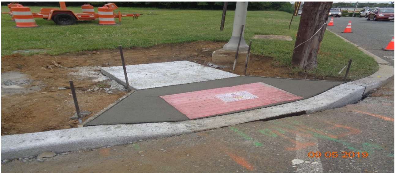
Figure 2: Concrete Curb and Sidewalk Along Derosse Avenue, East
