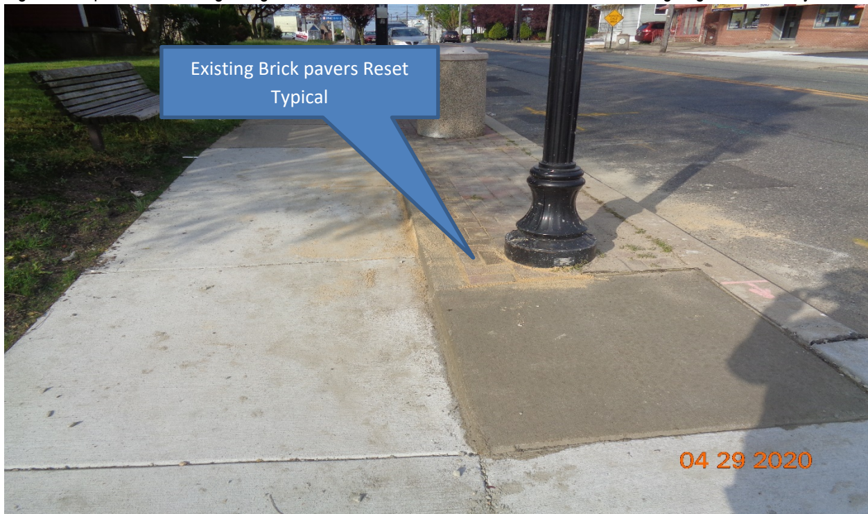
Figure 10: Resetting existing brick pavers along proposed sidewalk and existing brick pavers
