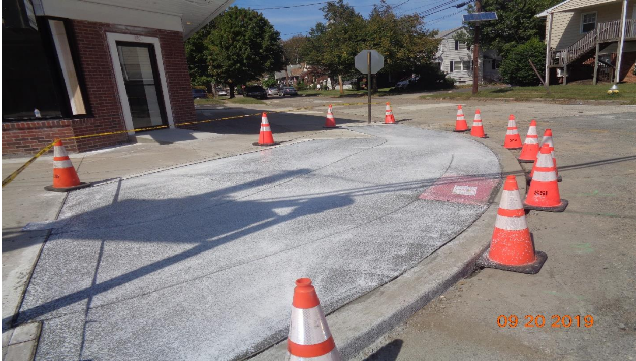
Figure 8: Concrete Curb and Sidewalk along Springfield Avenue, West
