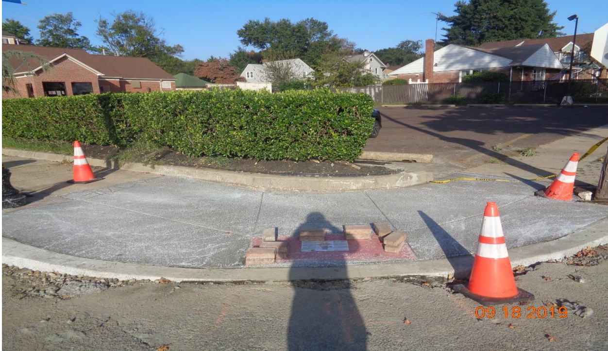
Figure 2: Concrete Curb and Sidewalk along Hollinshead Avenue, West
