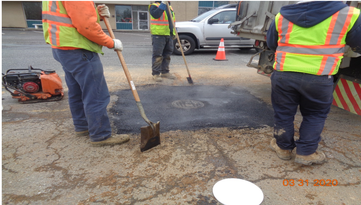
Figure 11: Gas leak fix was completed along Westfield Avenue at Derausse Avenue
