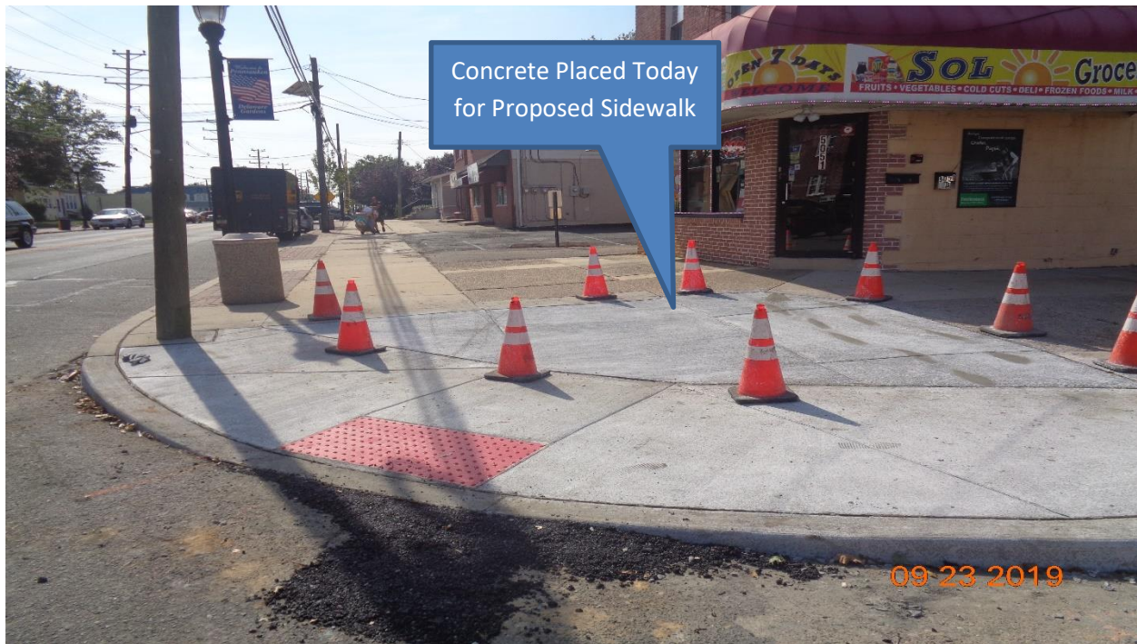
Figure 1: Sidewalk completed along Lexington Avenue West
