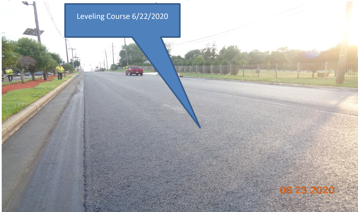
Figure1: Stone Matrix Asphalt 12.5 MM Surface Course along Westfield Avenue between STA 133+64 – 109+50.
