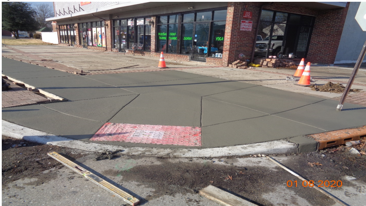
Figure 4: Hillcrest Avenue Construction of west handicap ramp.
