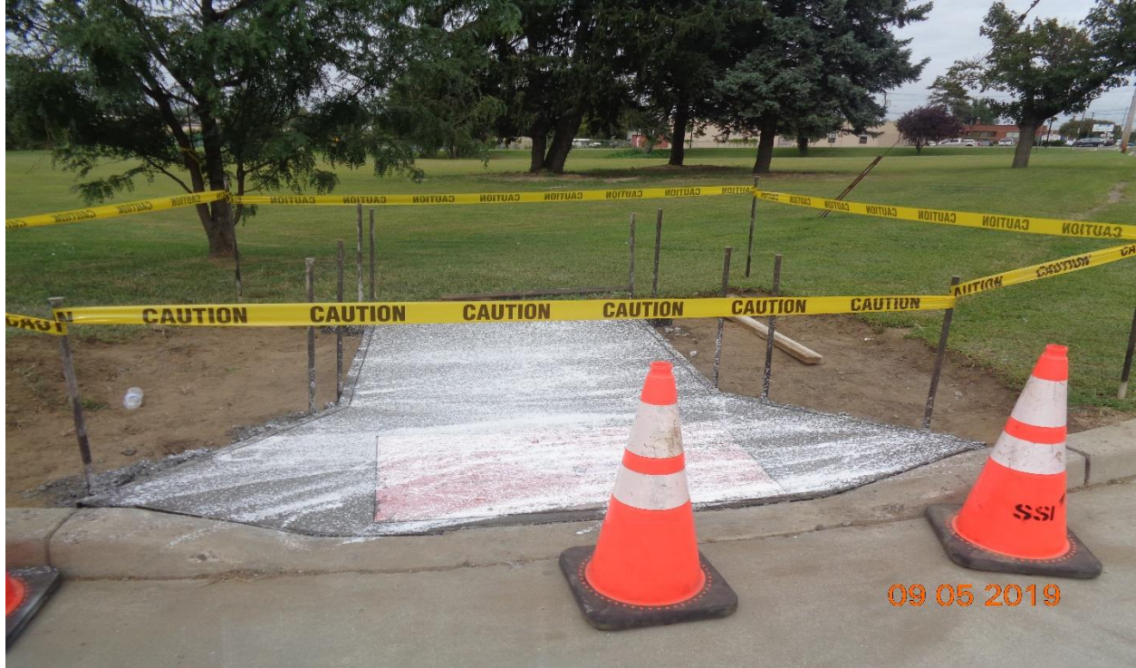
Figure 3: Concrete Sidewalk along Entrance of MPW, East
