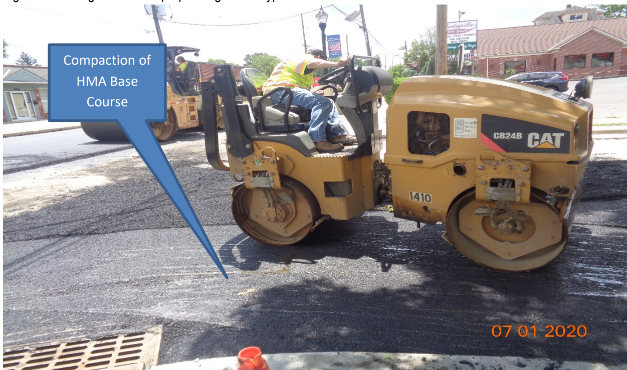
Figure 6: Full depth Asphalt Paving along Hollinshead Avenue, LT
