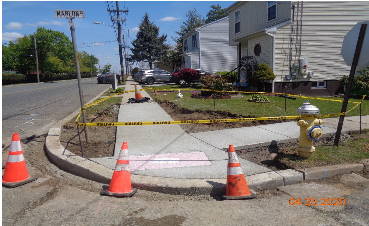
Figure 9: East concrete curb, sidewalk and handicap ramp at Marlon Avenue, RT
