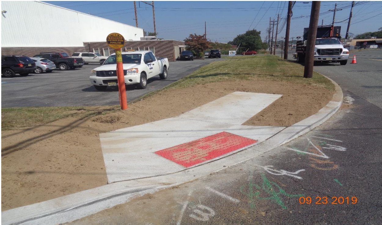
Figure 4: Topsoil placement along Sidewalk and Curb at Sherman Avenue, East
