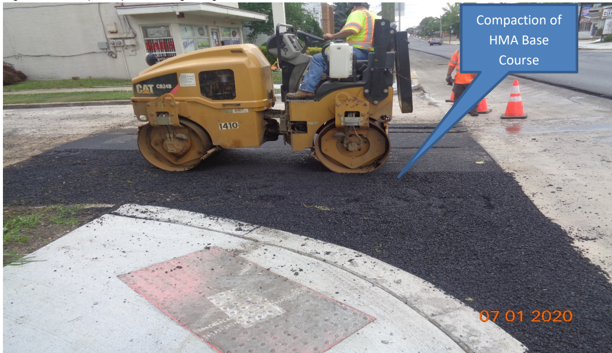
Figure 8: Full depth Asphalt Paving along Horner Avenue, RT
