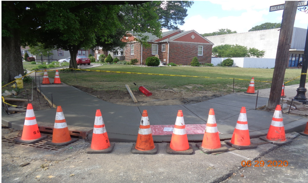
Figure 1: Concrete Curb, Sidewalk and HC Ramp at Hollinshead Avenue, LT
