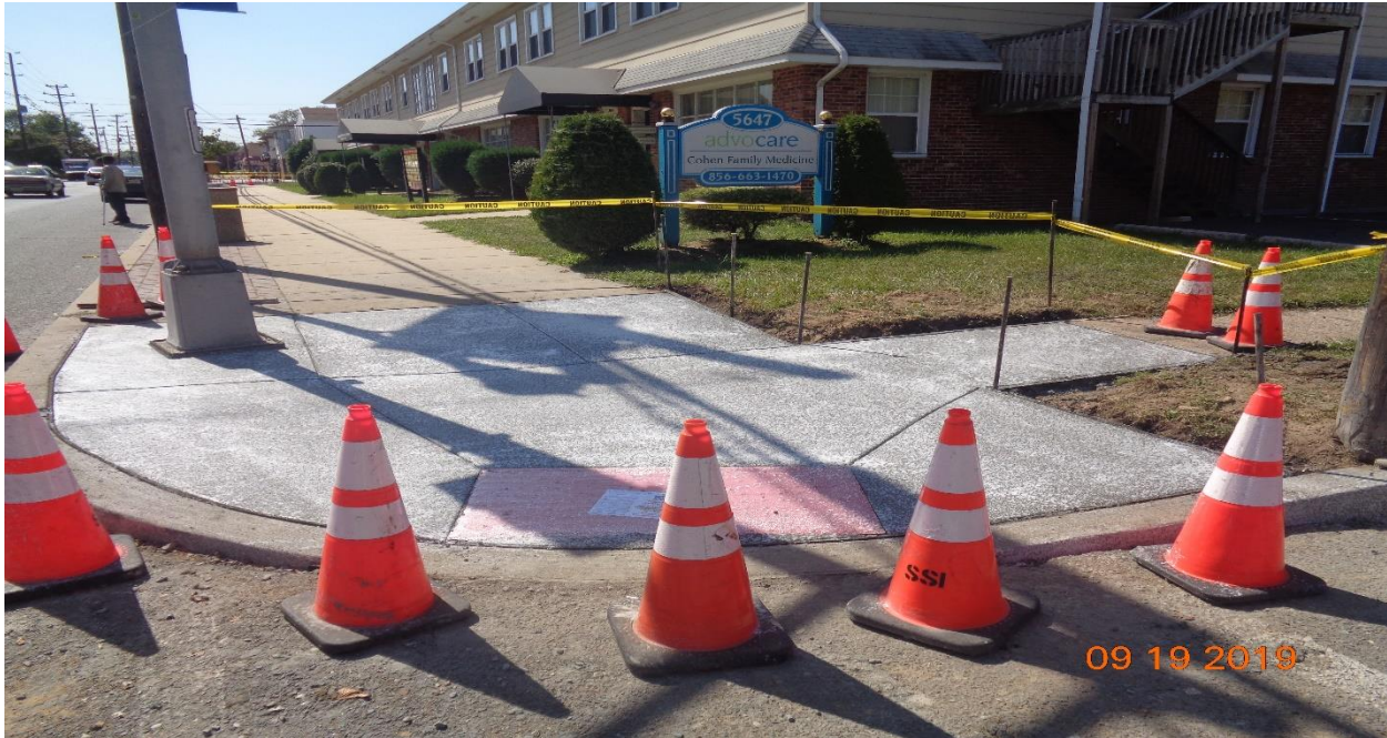
Figure 6: Concrete Curb and Sidewalk along Merchantville Avenue, West
