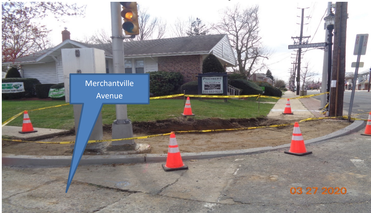
Figure 2: West concrete curb at Merchantville Avenue along Westfield Avenue, RT
