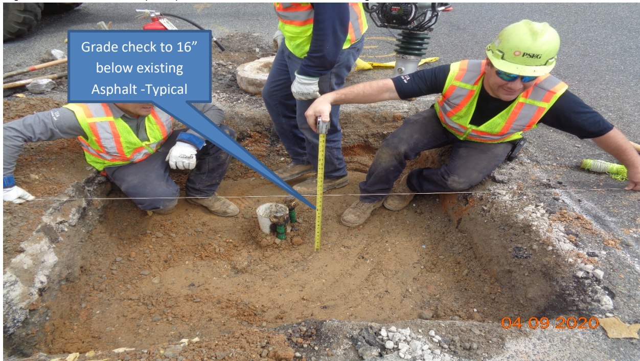
Figure 4: PSE&G Gas – Along Westfield Avenue at Derausse Avenue – Garde Check.
