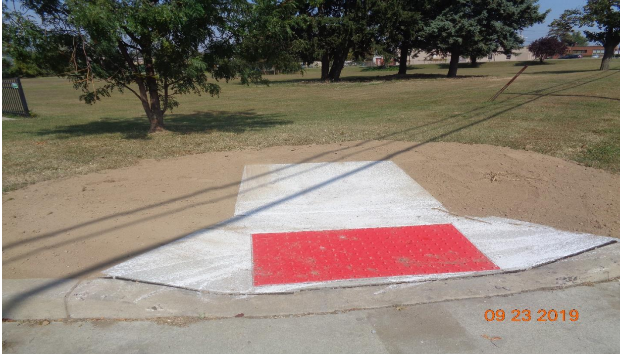
Figure 6: Topsoil around sidewalk at Entrance of MWPC, East
