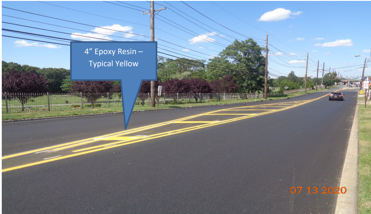
Figure 1: Traffic stripes, Long Life Epoxy Resin, 4" Wide along Westfield Avenue.
