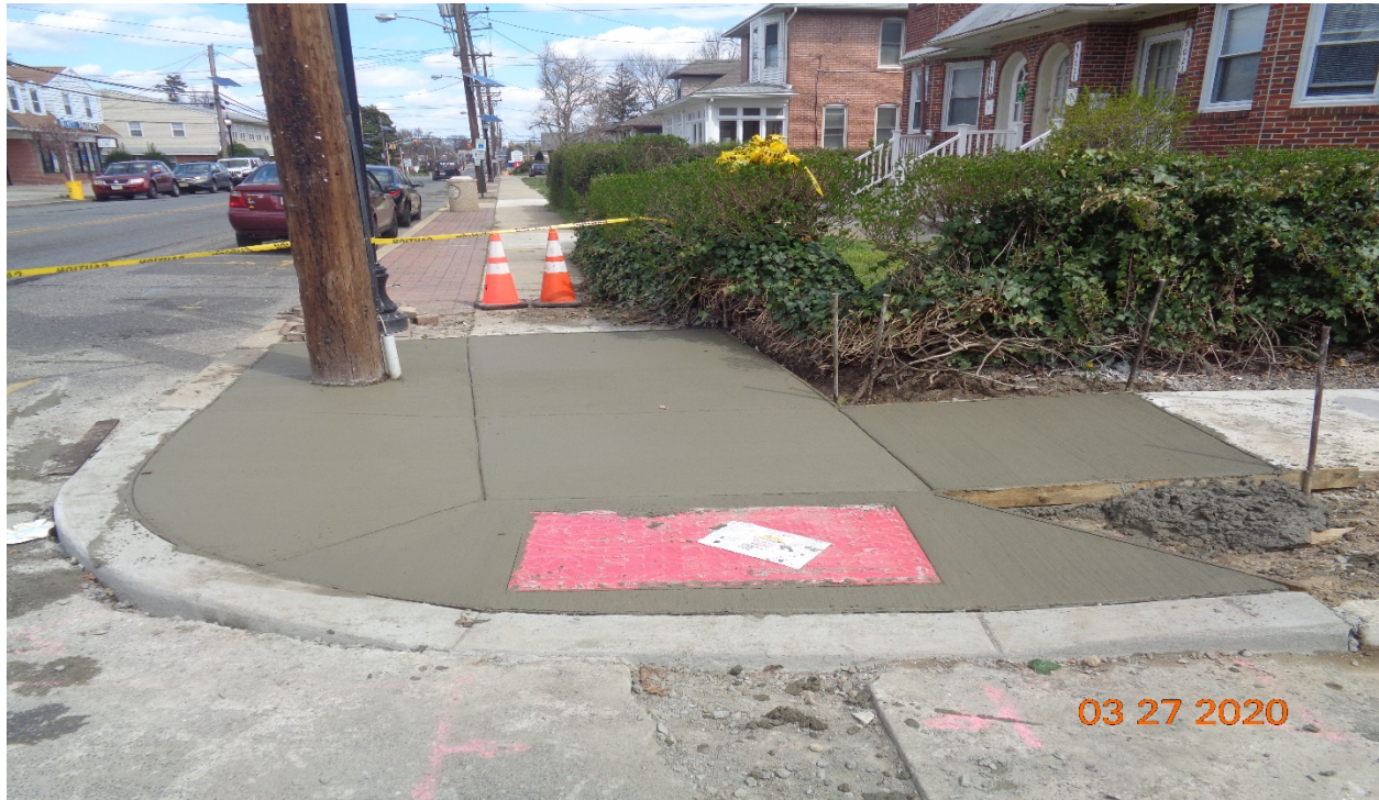
Figure 3: East concrete curb and sidewalk at Lexington Avenue along Westfield Avenue, RT
