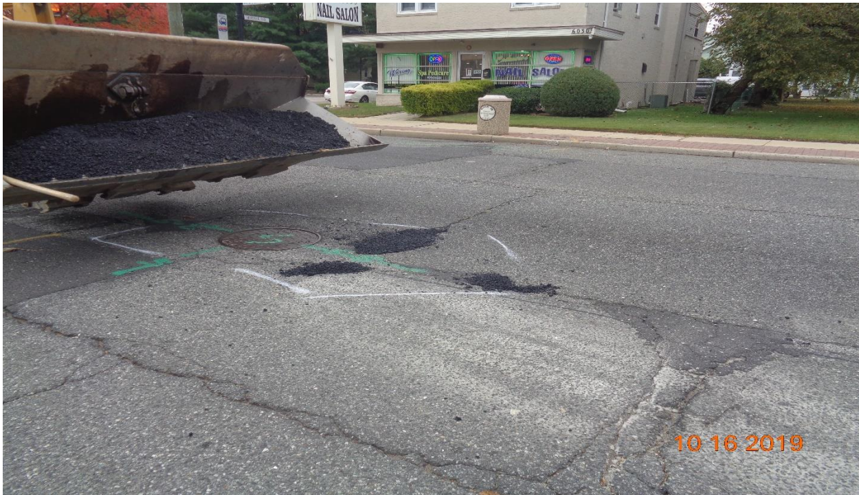
Figure 14: Repairing Potholes along Westfield Avenue
