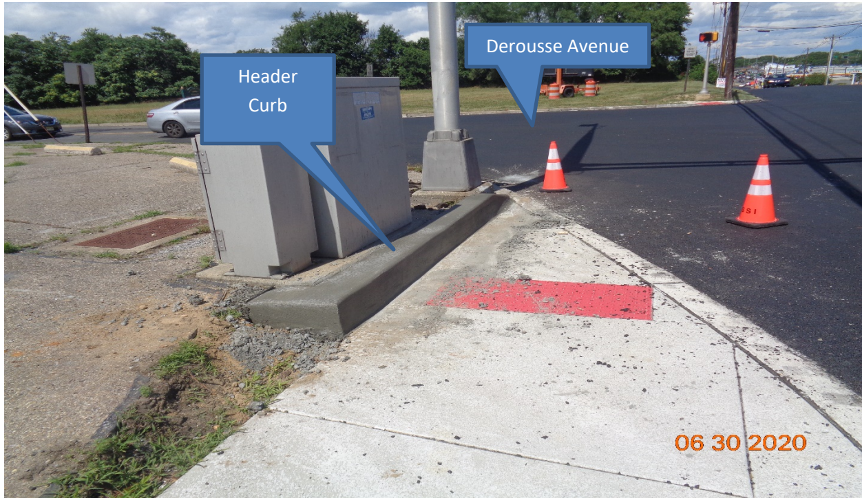
Figure 3: Header curb Along West sidewalk at Derosse Avenue, LT
