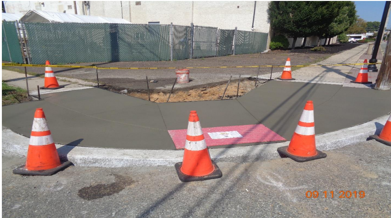
Figure 9: Concrete Curb and Sidewalk along Horner Ave, East
