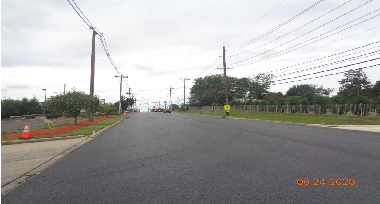
Figure 6: Stone Matrix Asphalt 12.5 MM Surface Course along Westfield Avenue between STA 133+64 – 109+50.
