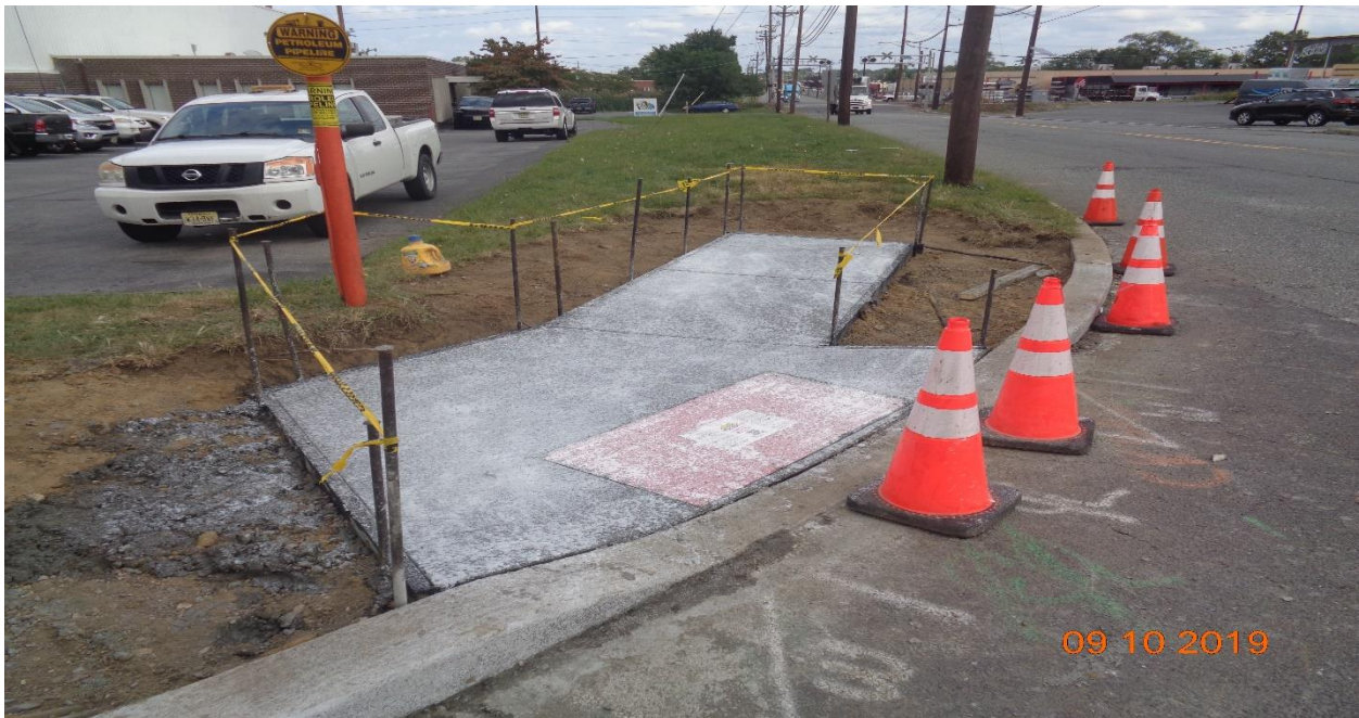
Figure 8: Concrete Curb and Sidewalk along Sherman Ave, East
