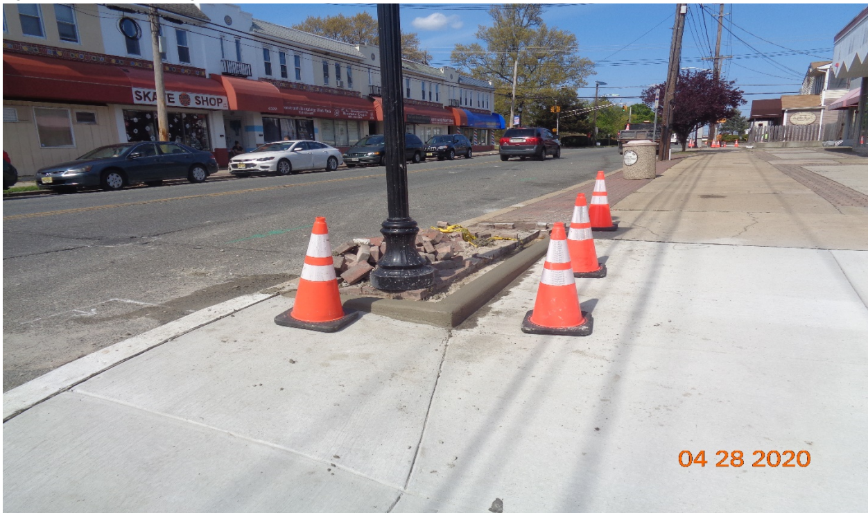
Figure 6: Hader Curb along Penn Street, East, RT
