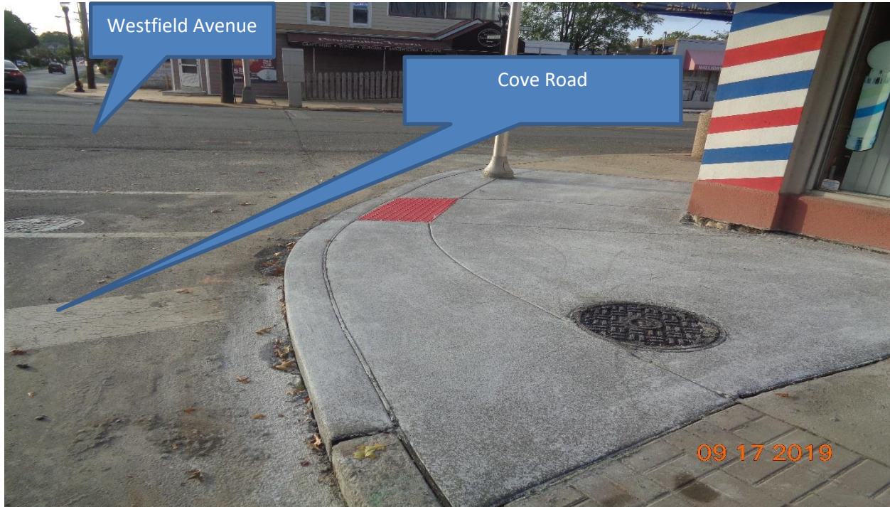
Figure 1: Concrete Curb and Sidewalk along Cove Road, West
