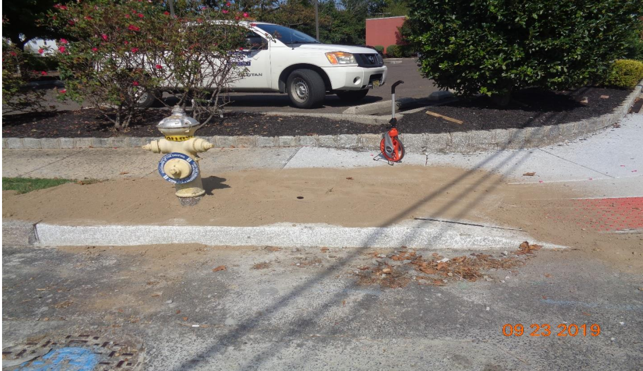
Figure 8: Topsoil around Curb and Sidewalk along Scovel Ave, West
