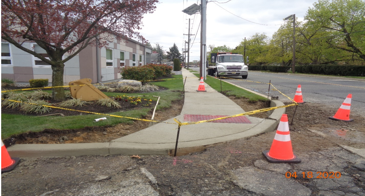
Figure 1: West concrete curb, sidewalk and HC Ramp at Norwood Avenue, RT
