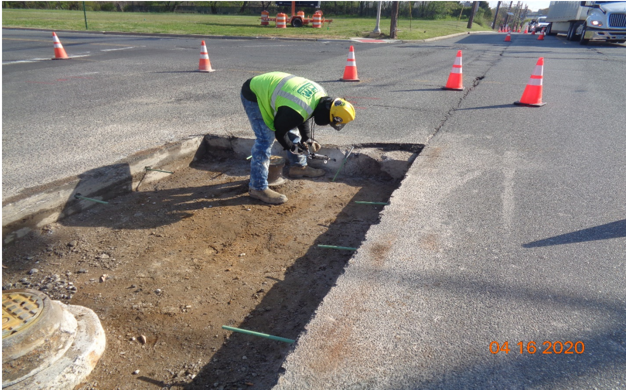
Figure: 7 - PSE&G Gas – 5/8" diameter dowels epoxy grouted – Typical at each location.
