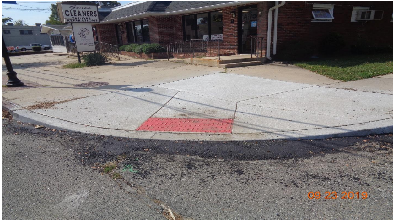
Figure 10: Asphalt around Curb Sidewalk along Horner Avenue, West
