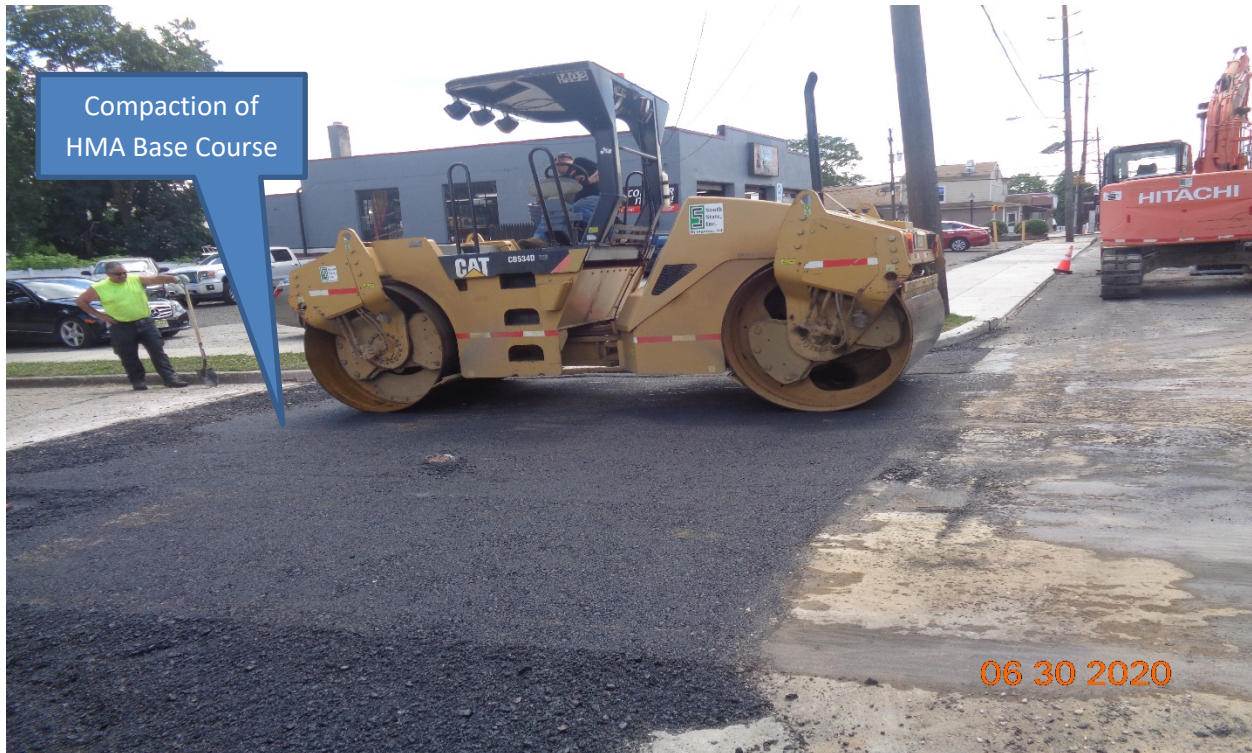
Figure 7: Full depth Asphalt Paving along Marlon Avenue, RT
