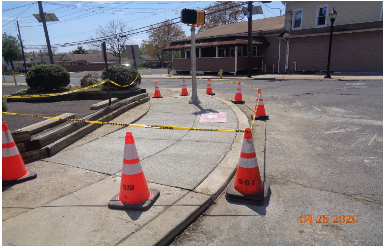
Figure 11: East concrete curb, sidewalk and handicap ramp at Cove Road, RT
