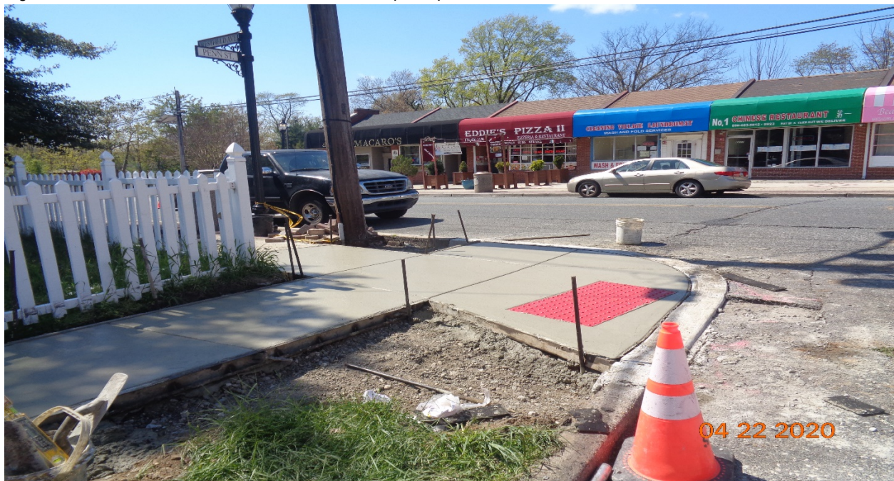
Figure 8: West concrete curb, sidewalk and handicap ramp at Penn Street, RT
