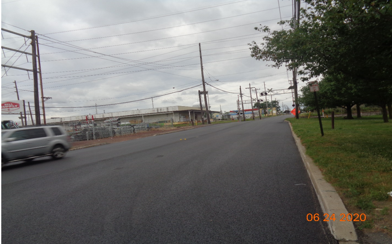
Figure 7: Stone Matrix Asphalt 12.5 MM Surface Course along Westfield Avenue between STA 133+64 – 109+50.
