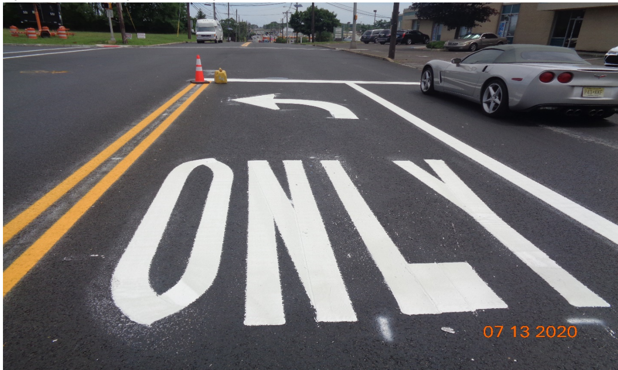
Figure 4: Traffic Marking – ONLY and Arrow – Typical
