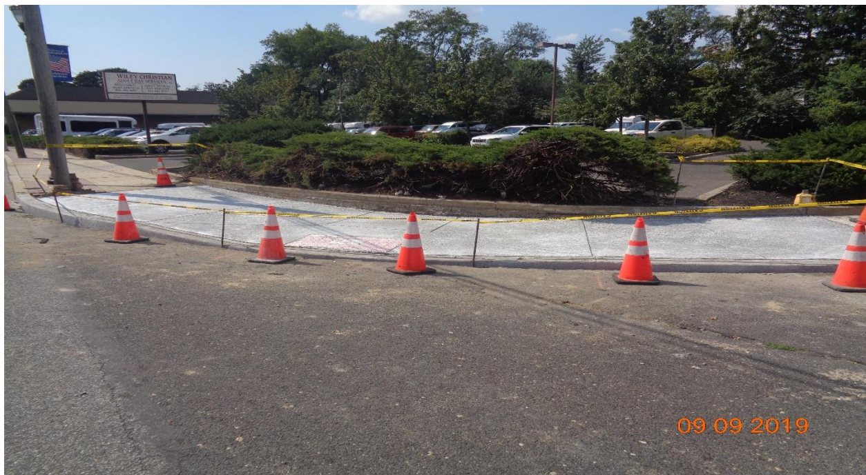
Figure 6: Concrete Curb and Sidewalk along Scovel Avenue, West
