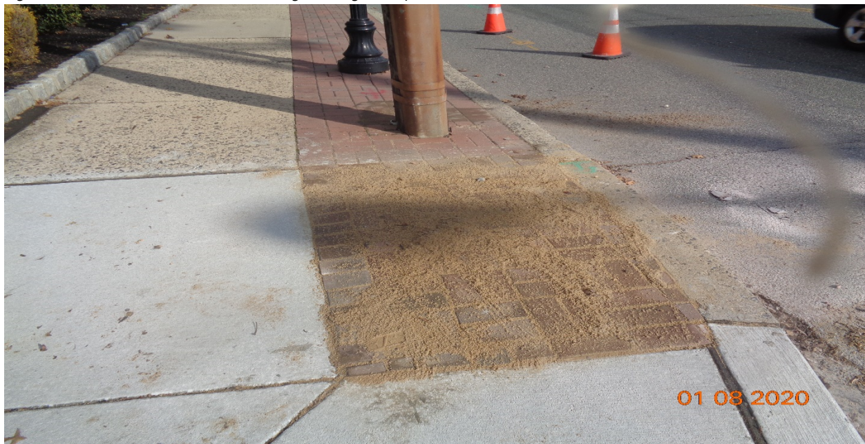
Figure 8: Scovel Avenue East – Resetting existing brick pavers.
