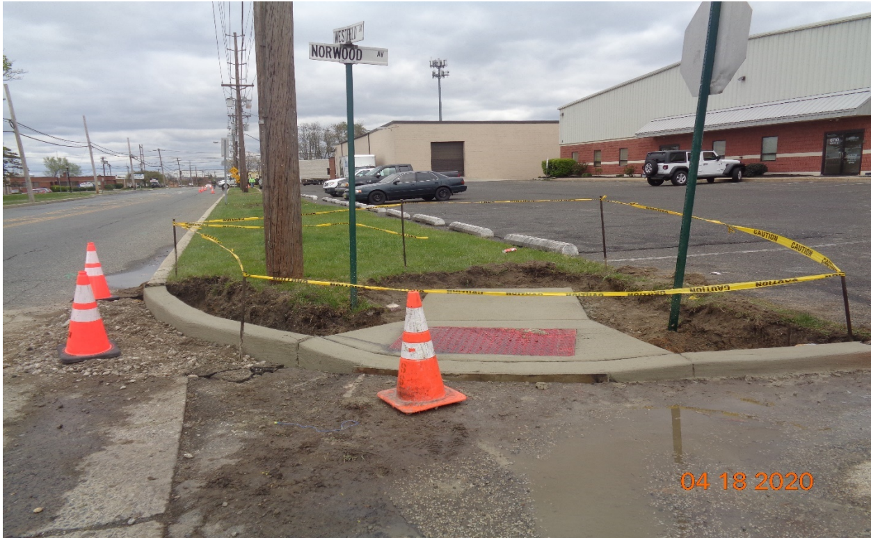
Figure 2: East concrete curb, sidewalk and HC Ramp at Norwood Avenue, RT
