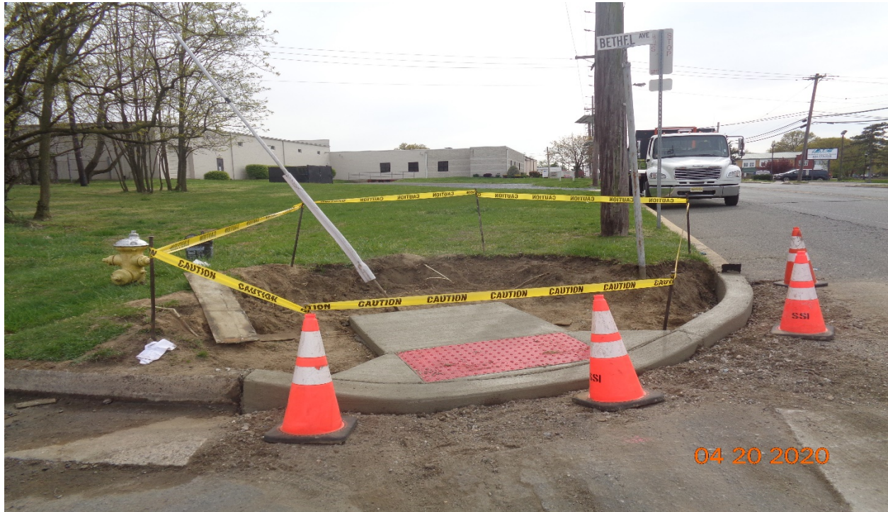
Figure 1: West concrete curb, sidewalk and handicap ramp at Bethel Avenue, RT
