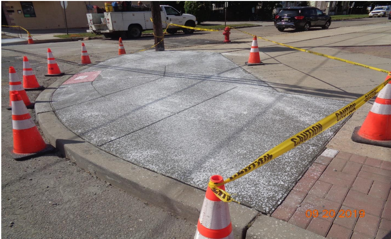
Figure 9: Concrete Curb and Sidewalk along Lexington Avenue, East
