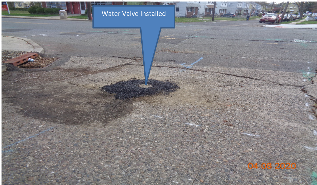
Figure8: MPWC – Water valve installed along Hollinshead Avenue, LT
