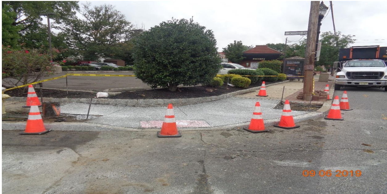
Figure 5: Concrete Curb and Sidewalk along Scovel Avenue, East
