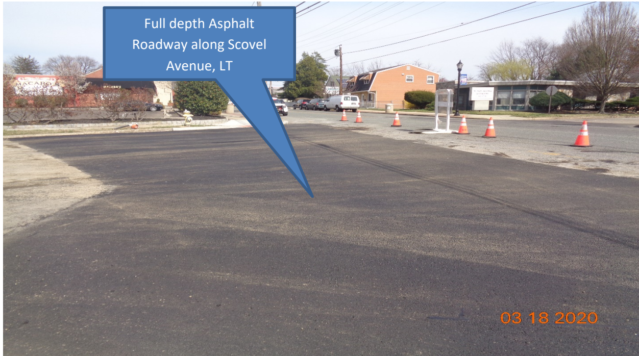
Figure 3: Full depth side street Asphalt Roadway construction along Scovel Avenue LT
