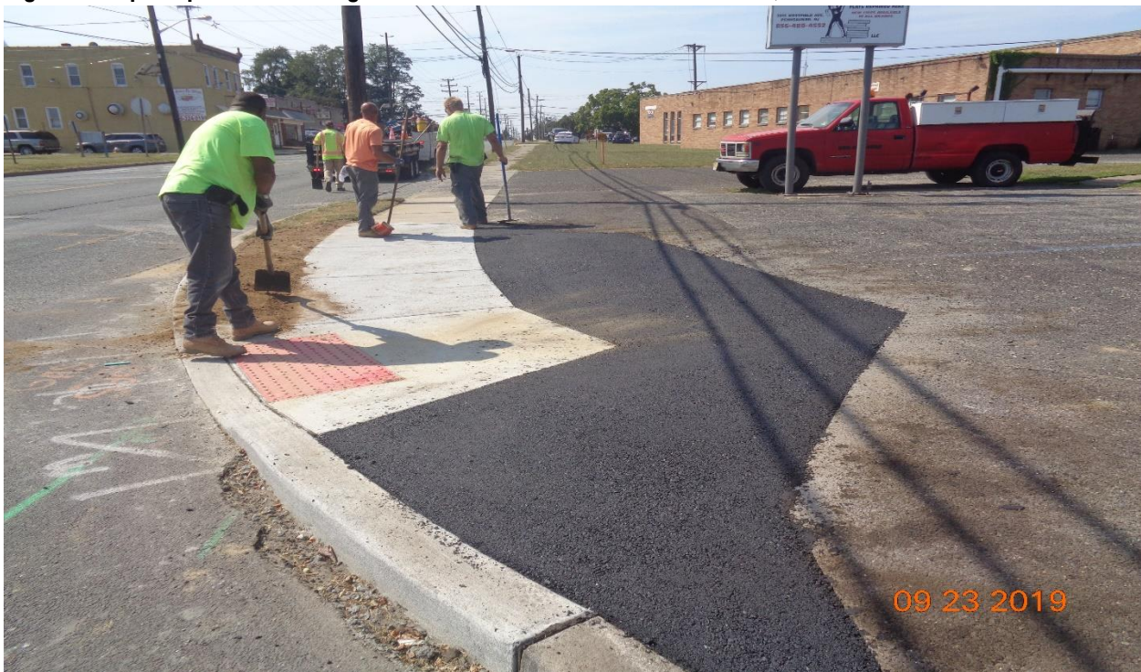
Figure 5: Topsoil and Asphalt along sidewalk and Curb at Sherman Avenue, West
