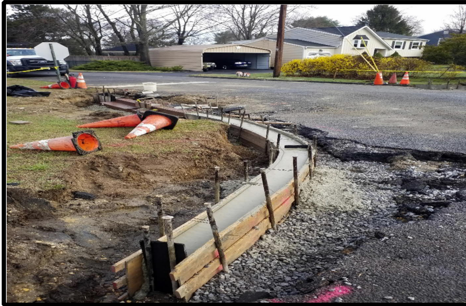
Photograph 6 – Progressing with Vertical Curb.
