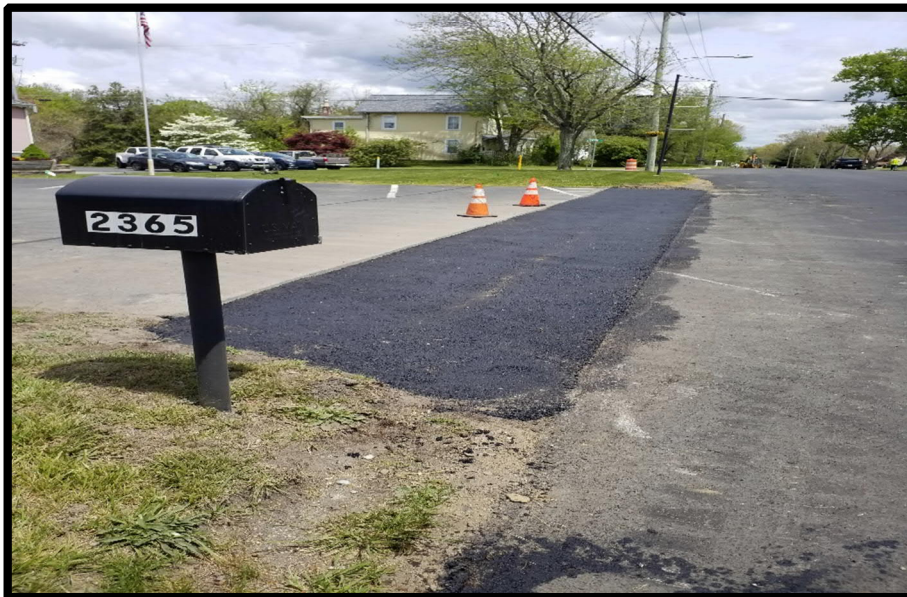
Photograph 4 – Driveway crew installing asphalt aprons – Yes you can drive on this once cooled.
