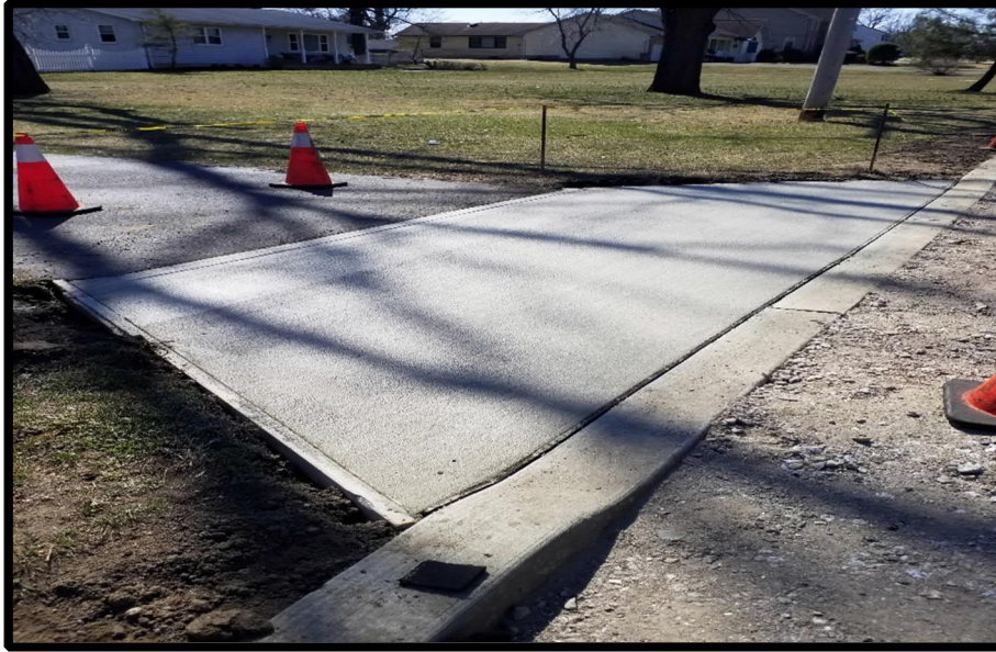
Photograph 4 – New Driveway apron behind depressed curb.
