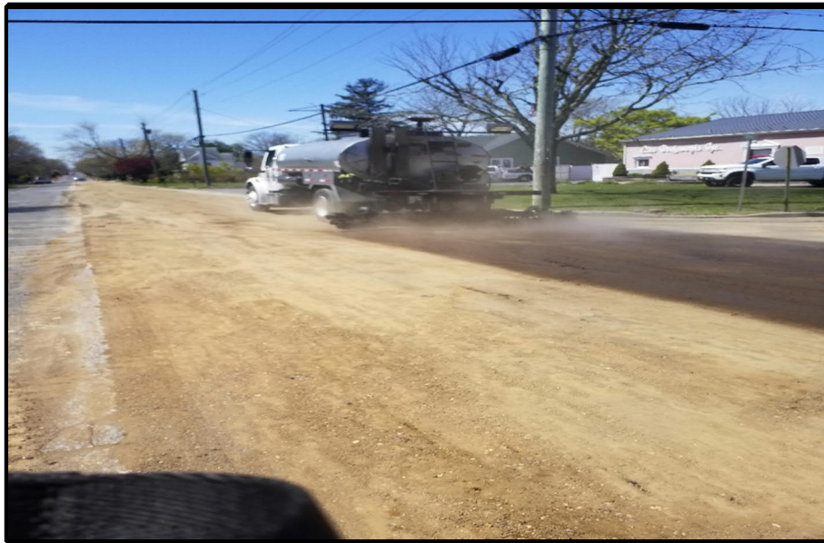
Photograph 7 – Material compacted, Graded and tack applied to help with dust.
