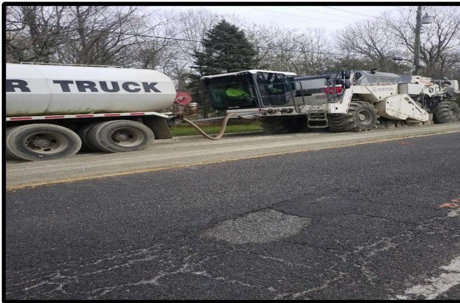
Photograph 4 – Cement is added to the FDR material.
