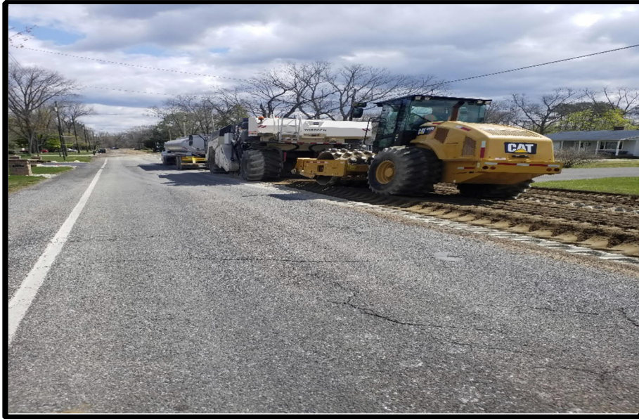
Photograph 6 – Same area compacted .
