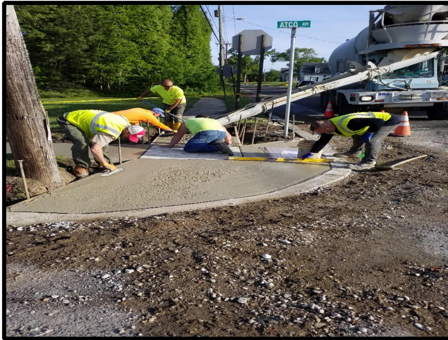
Photograph 2 – Curb Crew pouring sidewalk and handicap ramps at Third.
