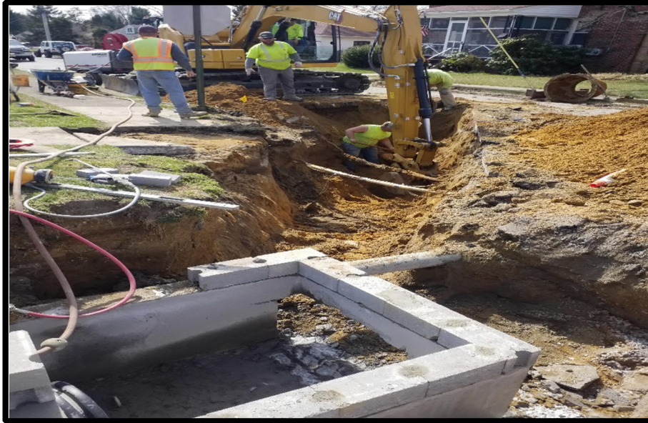
Photograph 4 – Installing New “B” Inlet and Drainage pipe under existing utilities.
