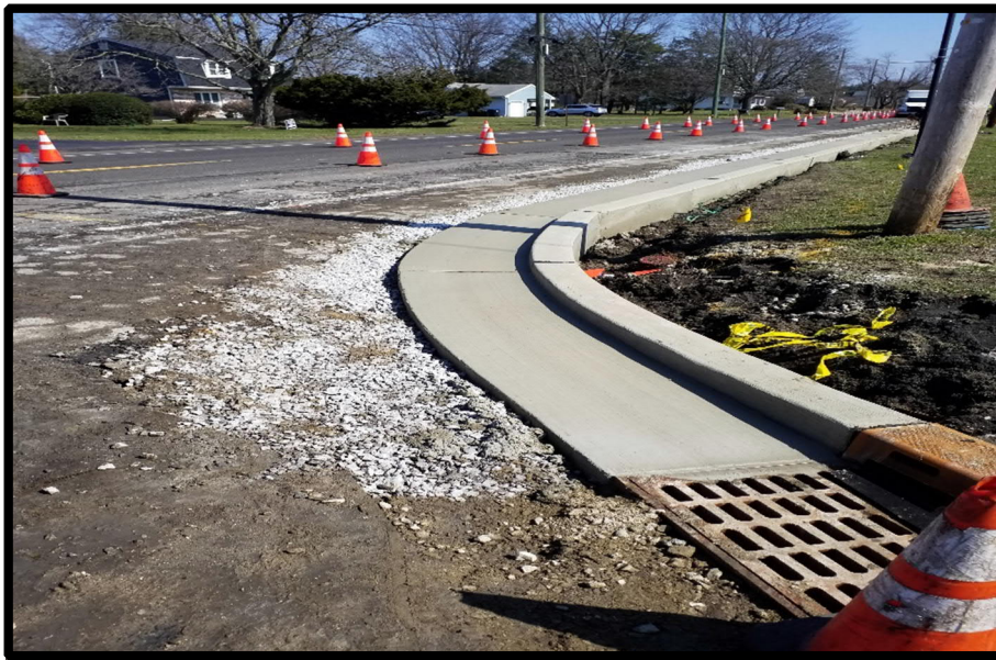
Photograph 4 – New Driveway apron behind depressed curb.
