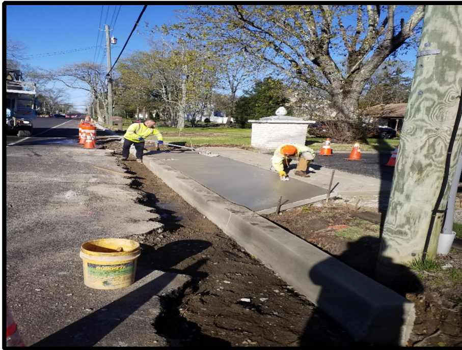
Photograph 2 – Curb Crew finishing driveway apron.
