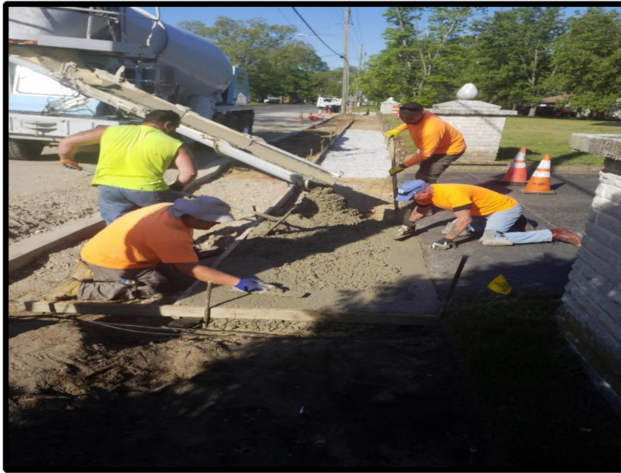
Photograph 2 – Curb Crew pouring sidewalk.
