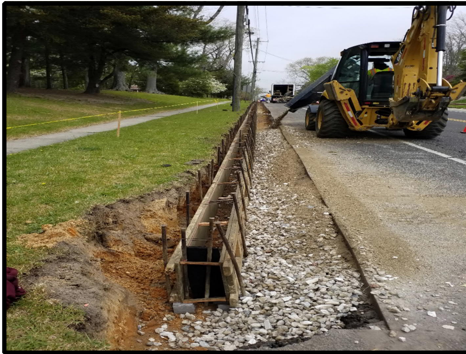
Photograph 1 – Curb Crew Forming for vertical curb near Second.
