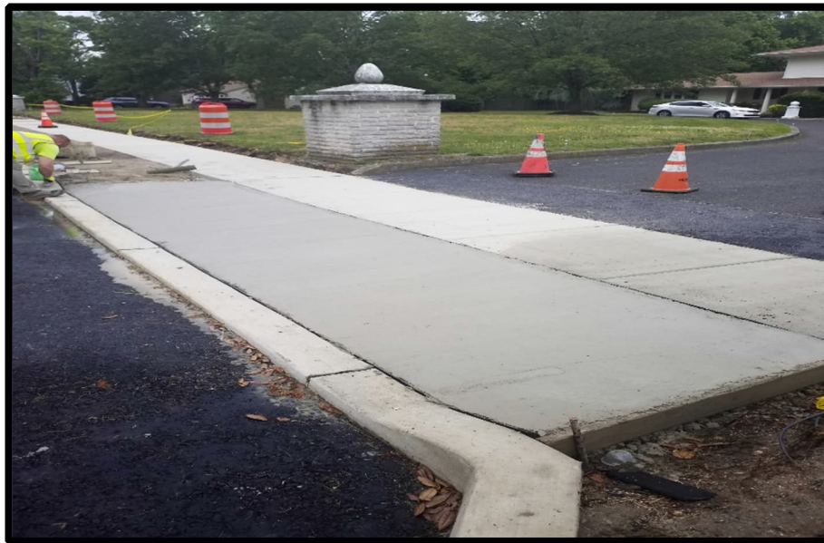
Photograph 4 – Forming for a concrete driveway apron near Church Street.
