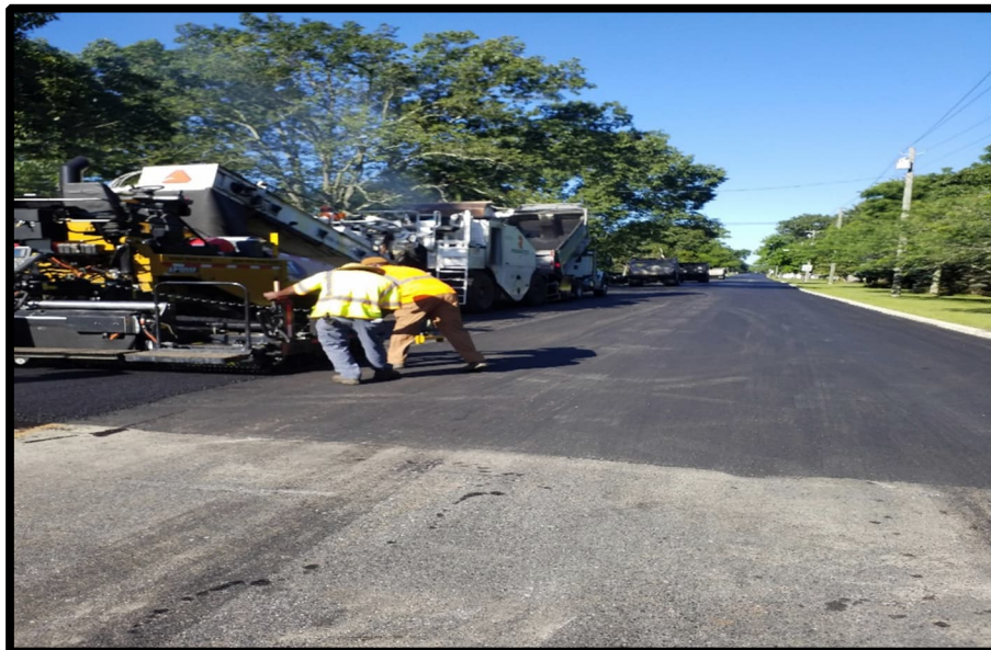
Photograph 3 – Surface Course Paving.
