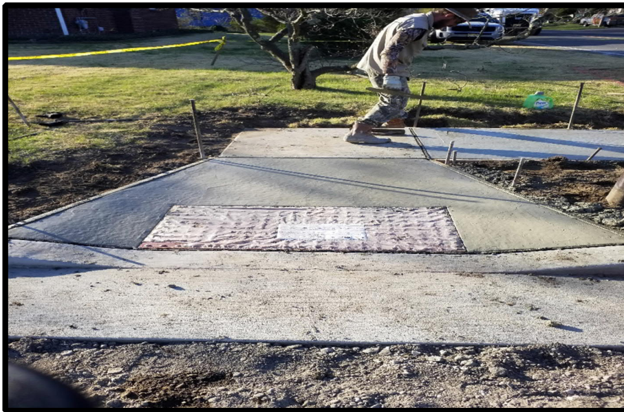
Photograph 4 – New Monolithic curb and handicap ramp installed at Atco & Third.
