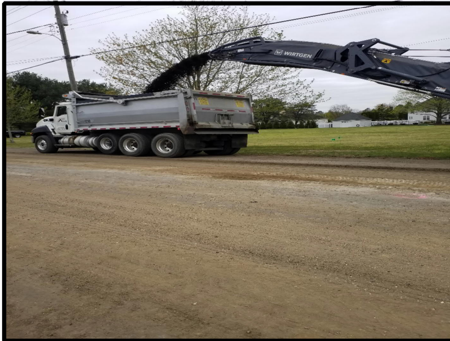
Photograph 1 – Road Crew milling “Full Depth Reclamation” to sub-base grade
