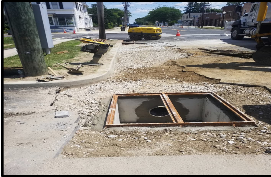
Photograph 4 – New inlet installed and connected .
