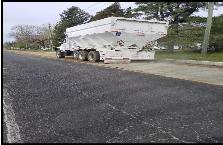
Photograph 4 – Cement is added to the FDR material.
