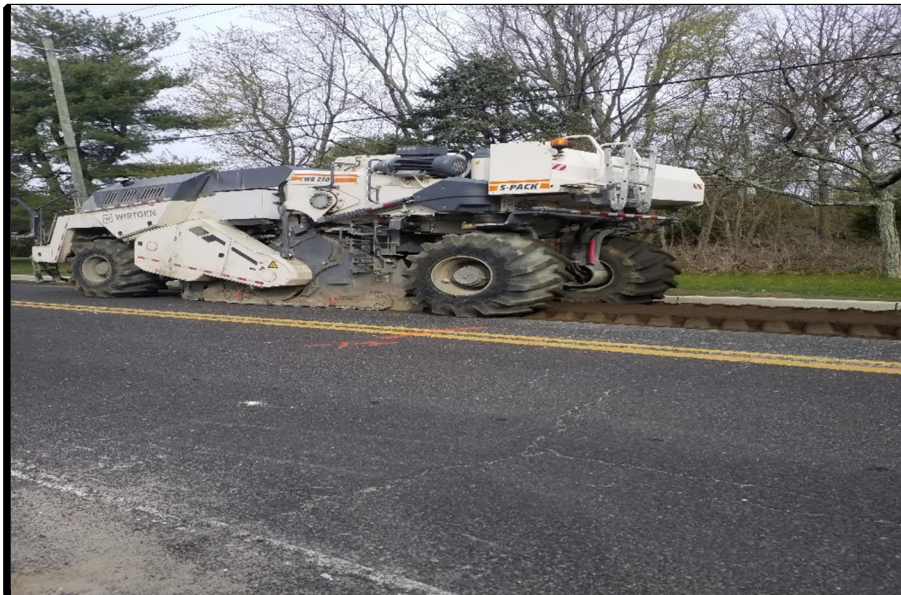
Photograph 3 – Full Depth Reclamation (FDR) started Monday.
