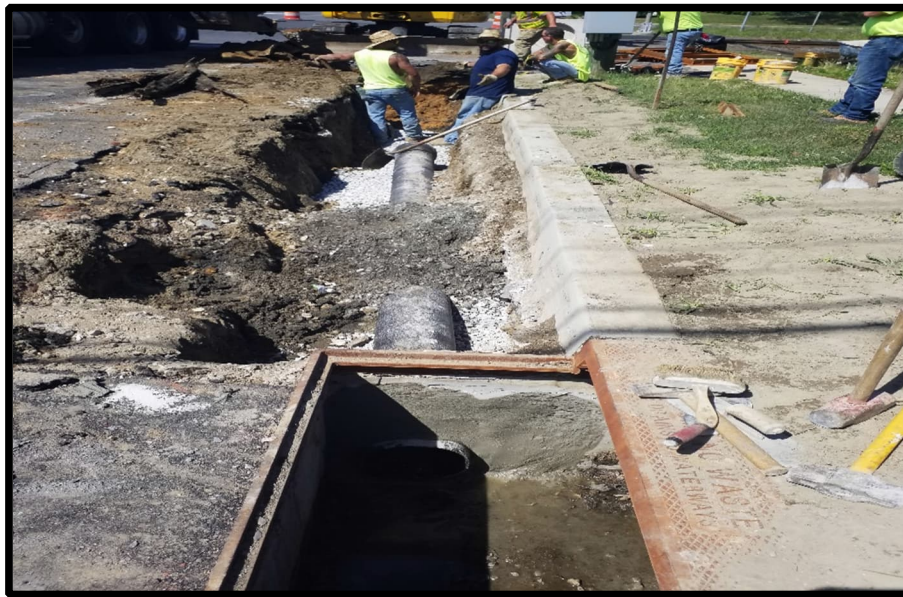
Photograph 3 – Another picture of the inlet / drainage construction.
