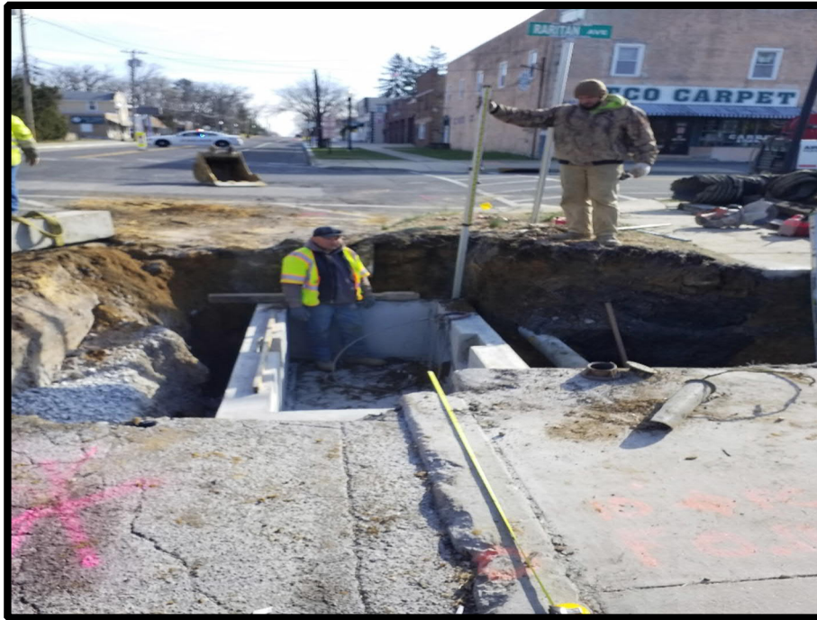
Photograph 2 – Pipe Crew installing double “B” inlet at Raritan ave.
