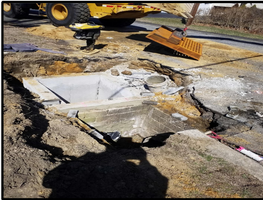
Photograph 1 – Contractor installed New “B” inlet and connected to existing inlet.
