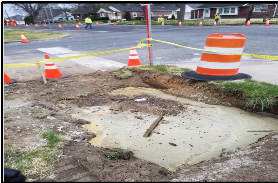
Photograph 3 – Flowable fill installed in sewer structure.
