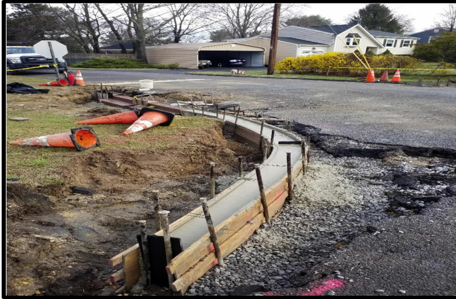
Photograph 6 – Progressing with Vertical Curb.
