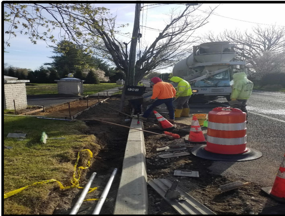
Photograph 1 – Curb crew pouring vertical curb.
