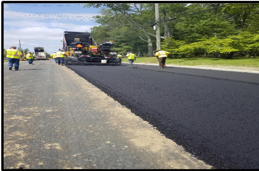
Photograph 6 – Paving base after milling to grade.
