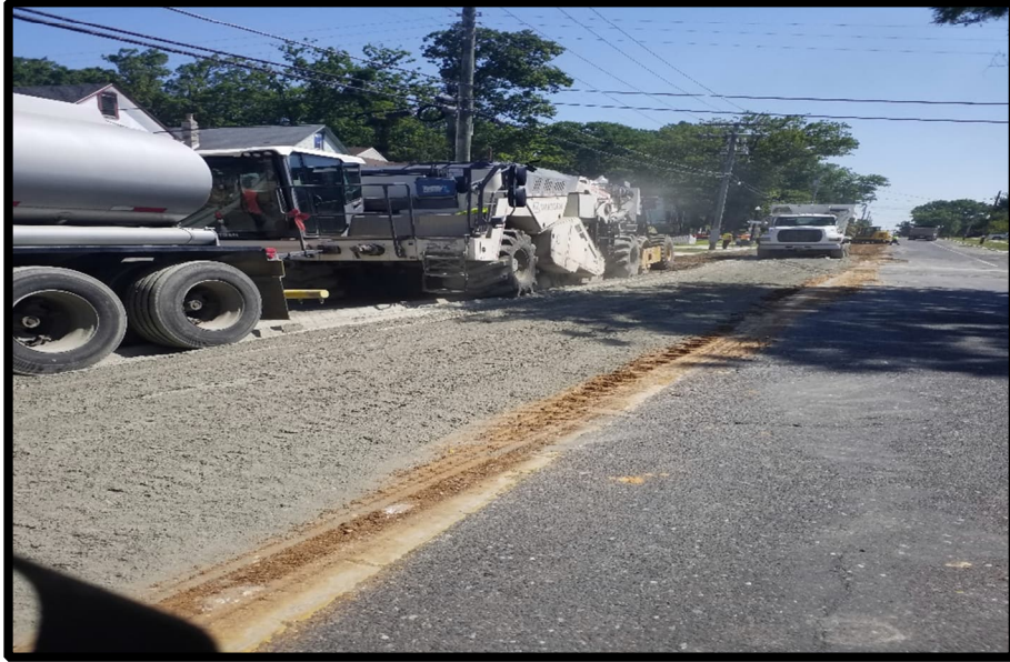
Photograph 6 – Full Depth Reclamation process.
