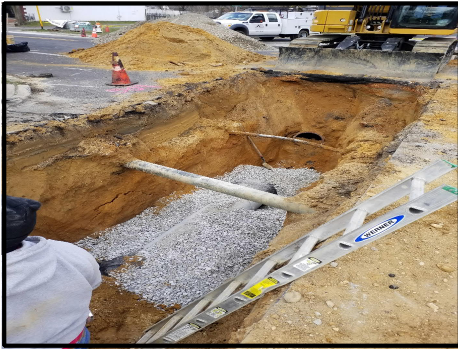
Photograph 1 – Pipe crew installing drainage pipe at Atco & Raritan aves.
