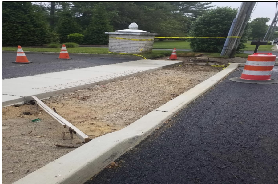
Photograph 3 – Forming for concrete driveway apron.
