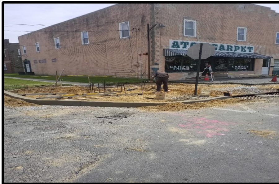
Photograph 3 – Handicap Ramp/Sidewalk Construction.
