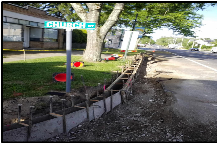
Photograph 3 – Forming for vertical curb at Church Street.
