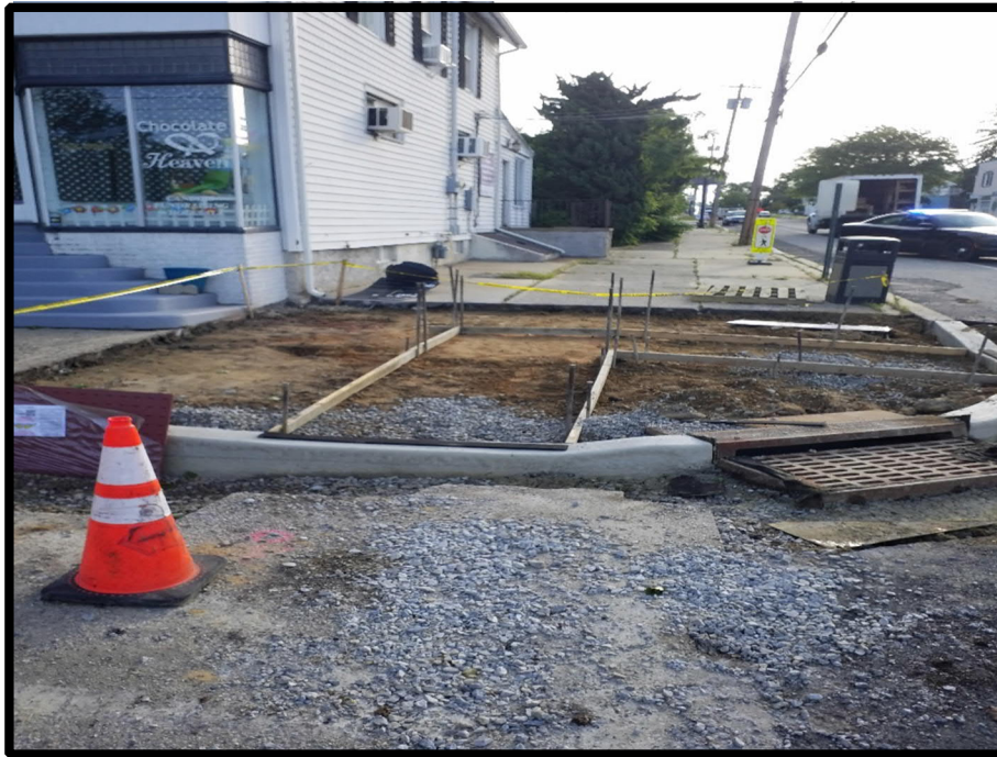
Photograph 1 – Curb Crew forming for sidewalk and handicap ramps at Raritan Avenue.
