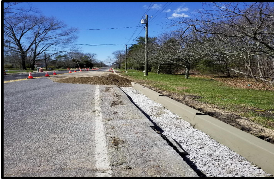
Photograph 4 – New Vertical curb installed.
