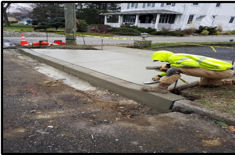
Photograph 4 – Getting ready to pour a new driveway apron.
