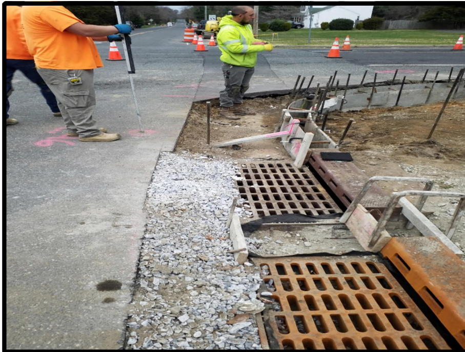
Photograph 1 – Curb crew installing forms for vertical curb.
