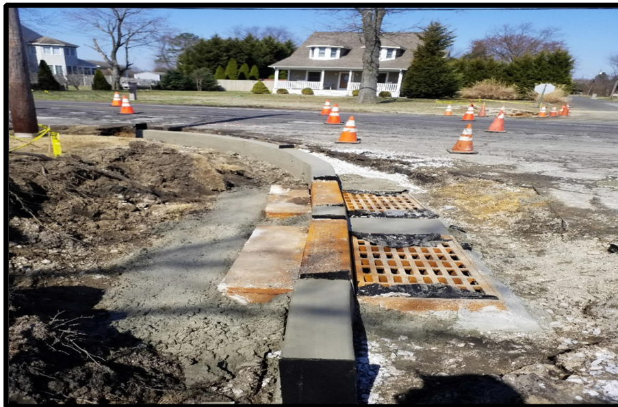
Photograph 3 – Vertical Curb poured and Inlets set to new grade.
