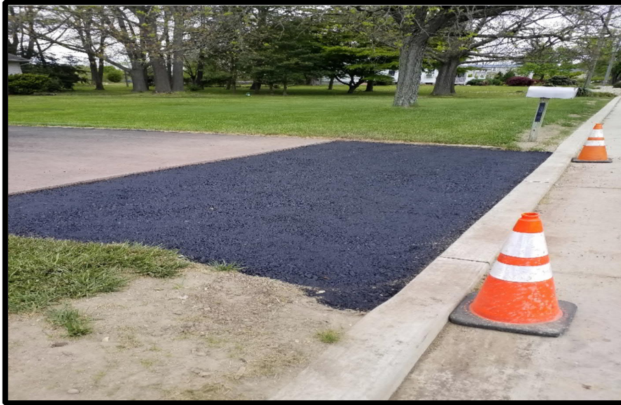
Photograph 4 – Driveway crew installing asphalt aprons – Yes you can drive on this once cooled.
