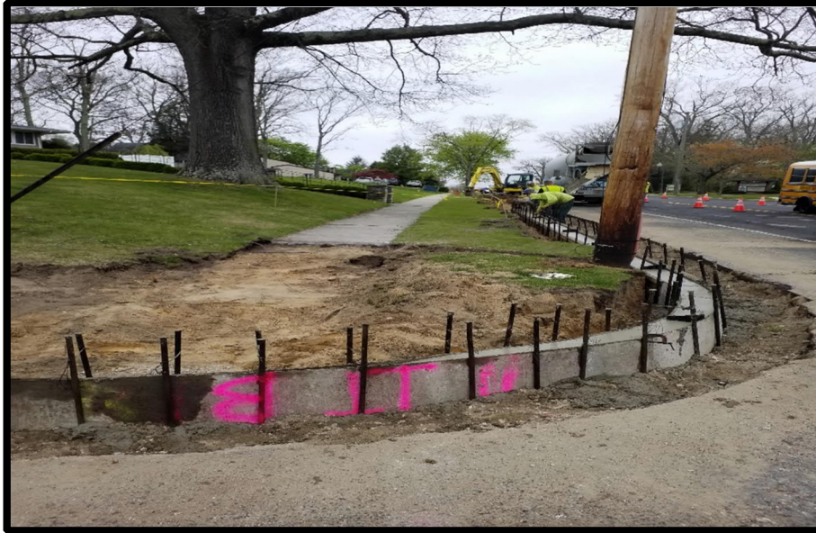
Photograph 4 – Curb Crew forming for vertical curb and handicap ramps at Second Street.
