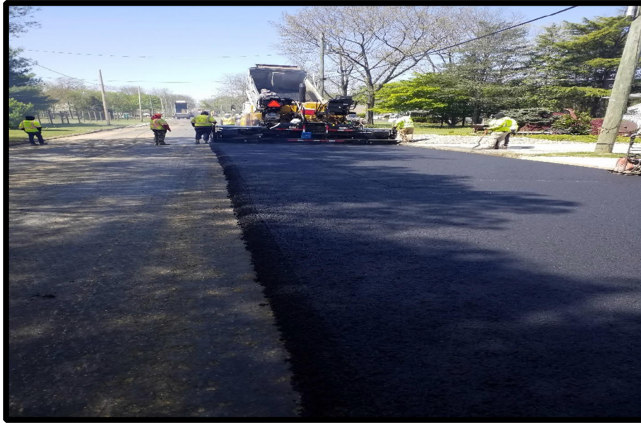
Photograph 6 – Base material installed from Fourth to Jackson.
