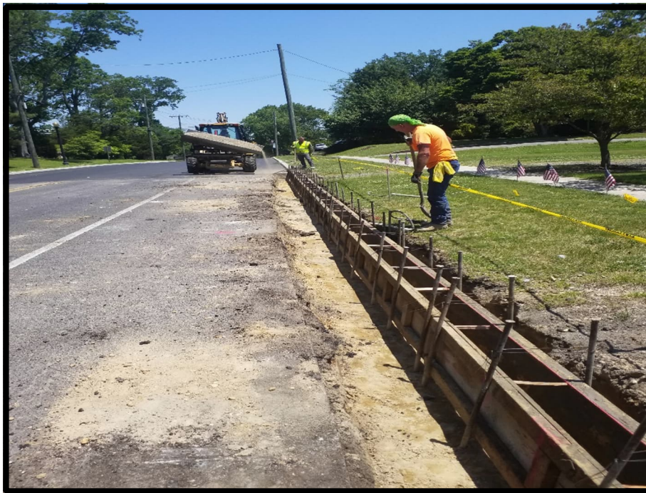
Photograph 1 – Curb Crew forming for vertical curb.
