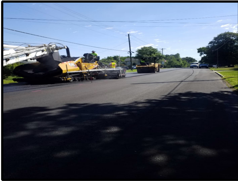
Photograph 2 – More Paving of Surface Course.
