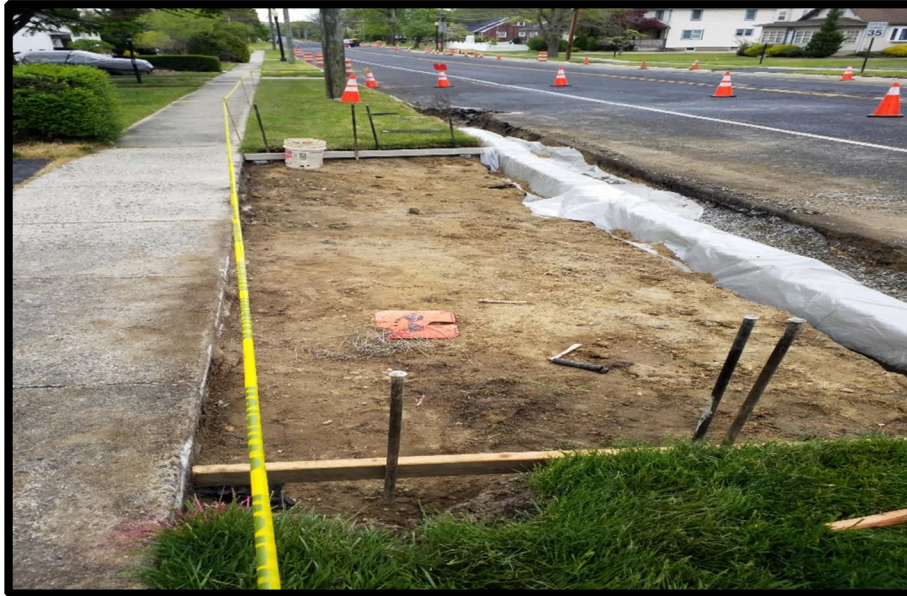
Photograph 6 – Preparing to pour concrete driveway apron.
