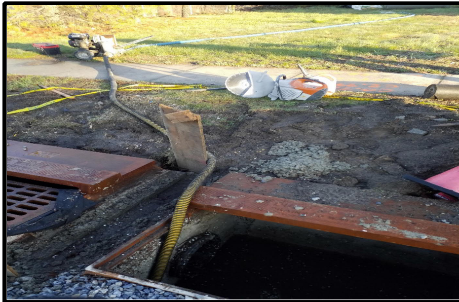
Photograph 7 – Inlets installed
