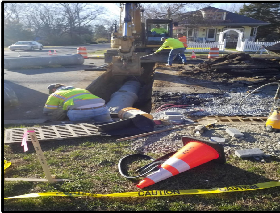
Photograph 2 – Installing 15” RCP Cross Drain at 3rd Street.
