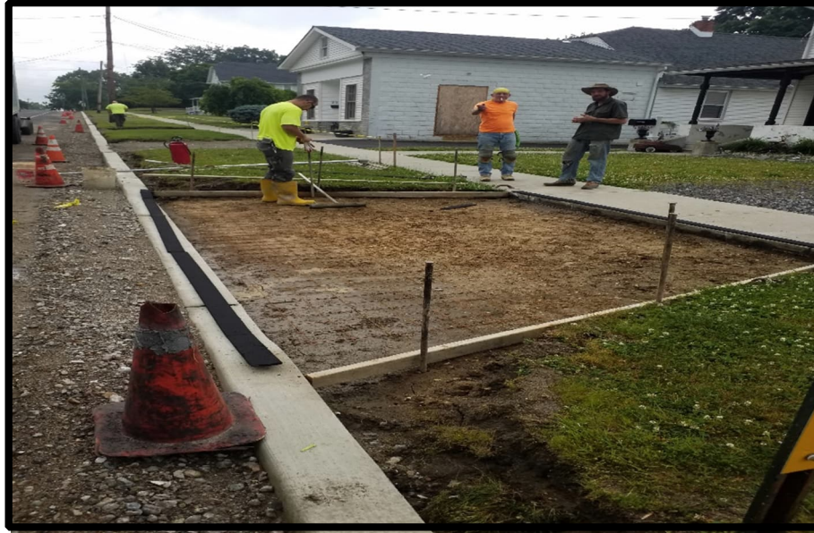
Photograph 4 – Forming for a concrete driveway apron near Church Street.
