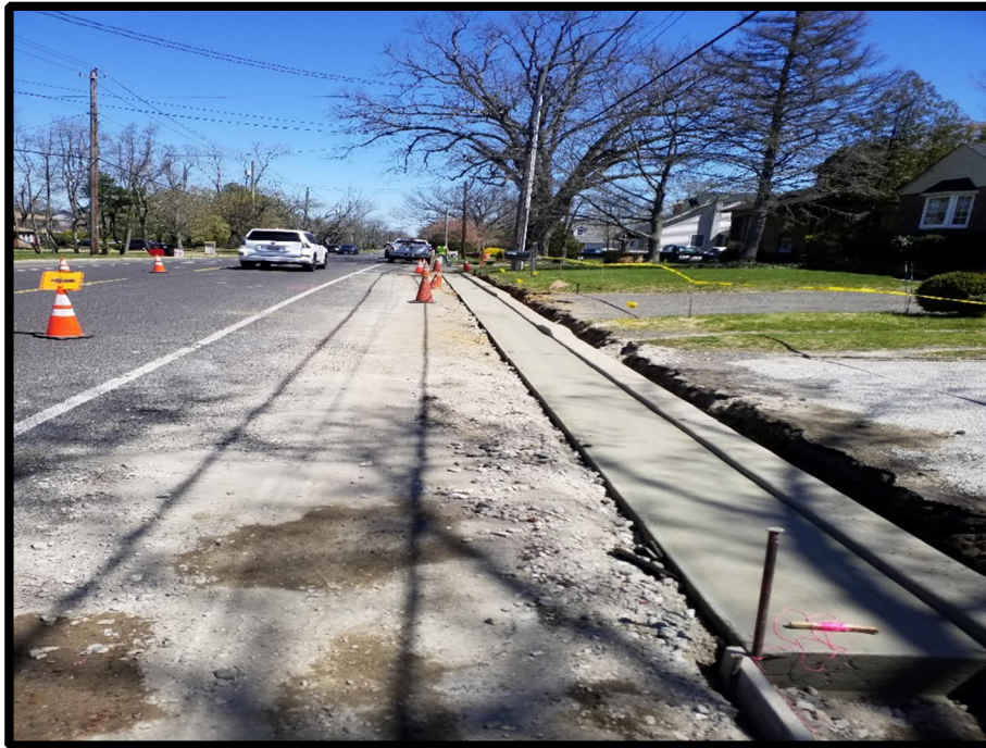
Photograph 2 – Curb Crew installing monolithic curb.
