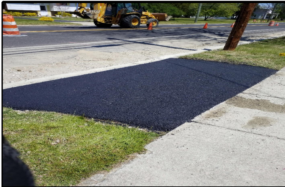
Photograph 7 – Asphalt Driveway aprons installed near Second Street.
