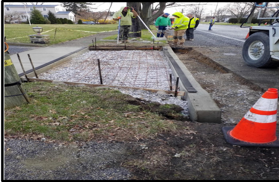
Photograph 4 – Getting ready to pour a new driveway apron.
