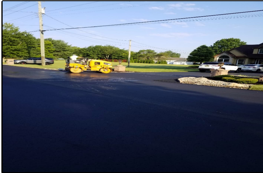
Photograph 6 – Final paving operation at Raritan.
