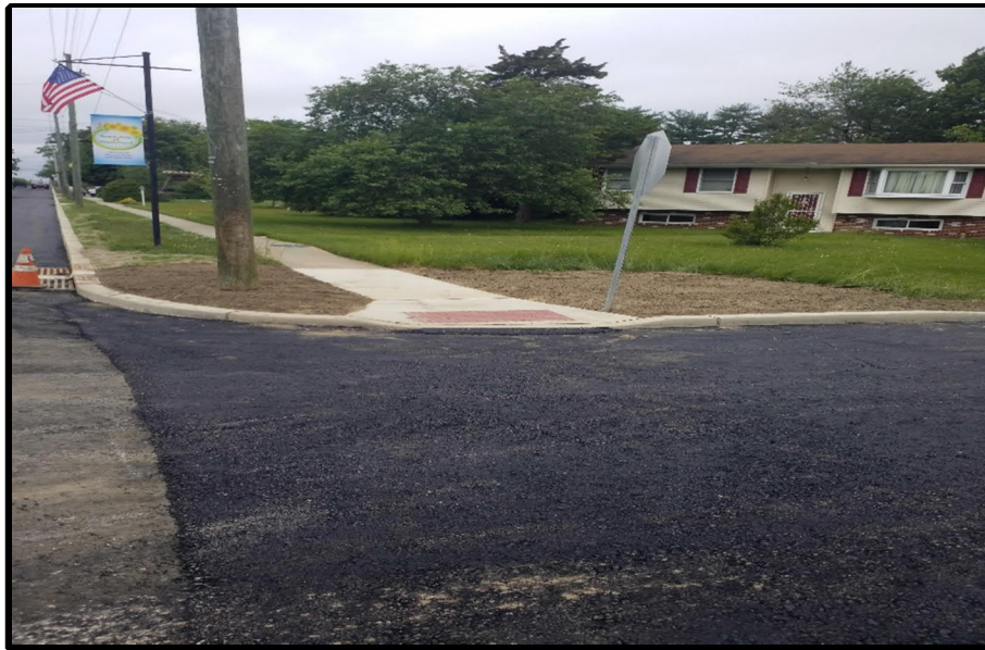
Photograph 6 – Paving base after milling to grade.
