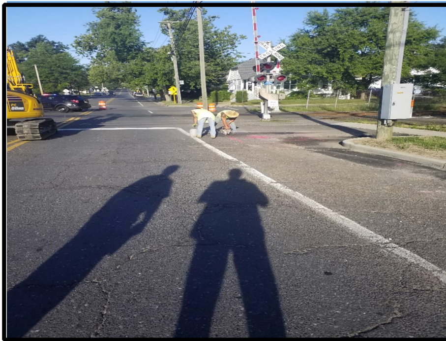
Photograph 1 – Crew cutting out for new inlet.
