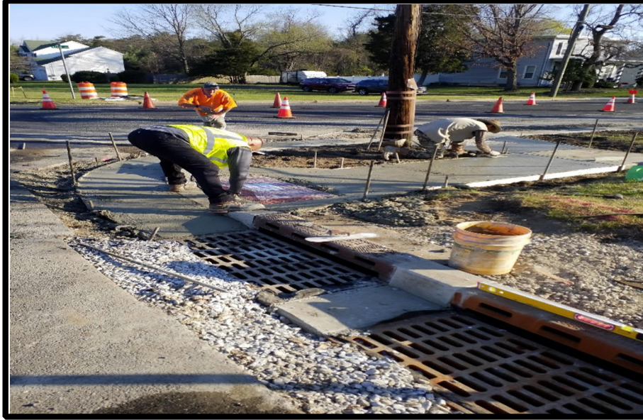
Photograph 4 – New Monolithic curb and handicap ramp installed at Atco & Third.
