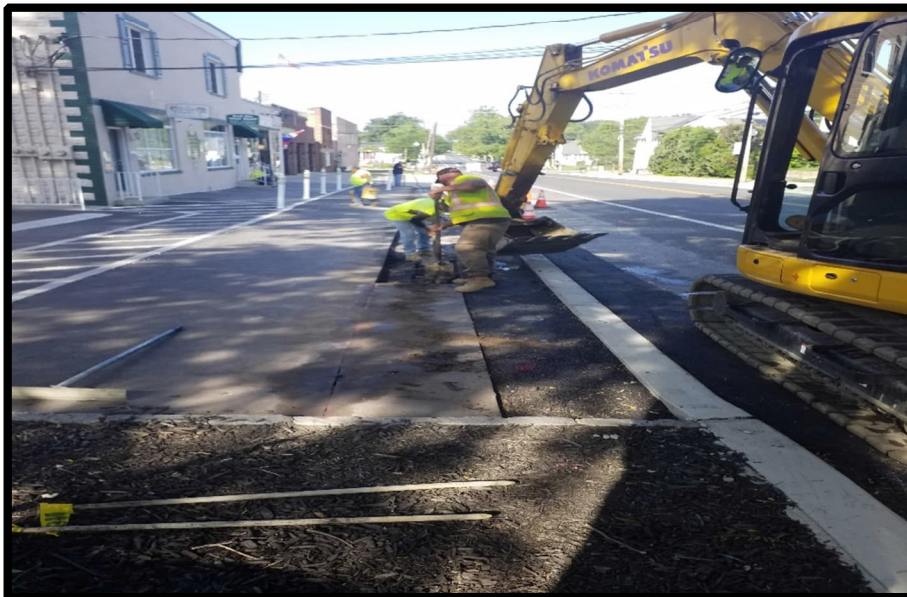
Photograph 4 – New inlet installed and connected .
