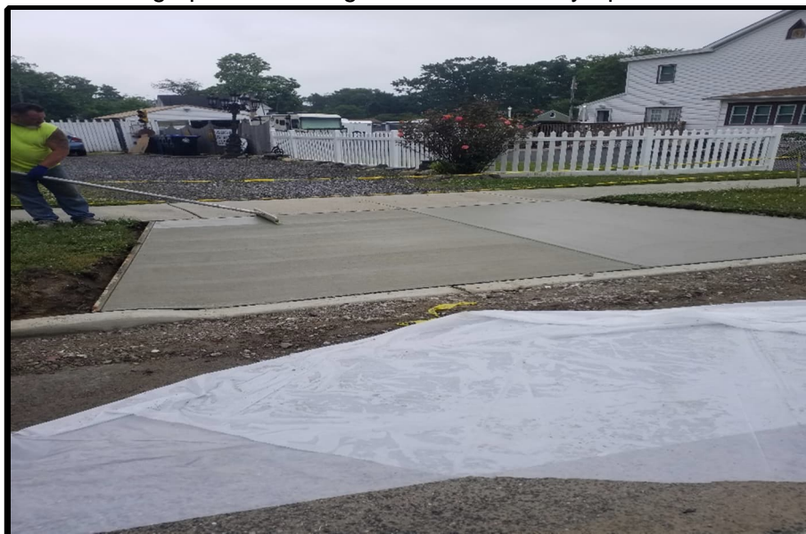
Photograph 6 – Pouring Concrete Driveway Apron.
