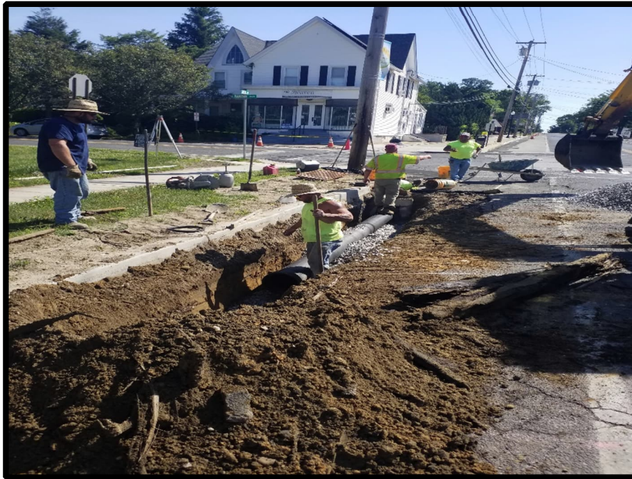
Photograph 2 – Crew installing Ductile Iron Pipe joining new inlets.
