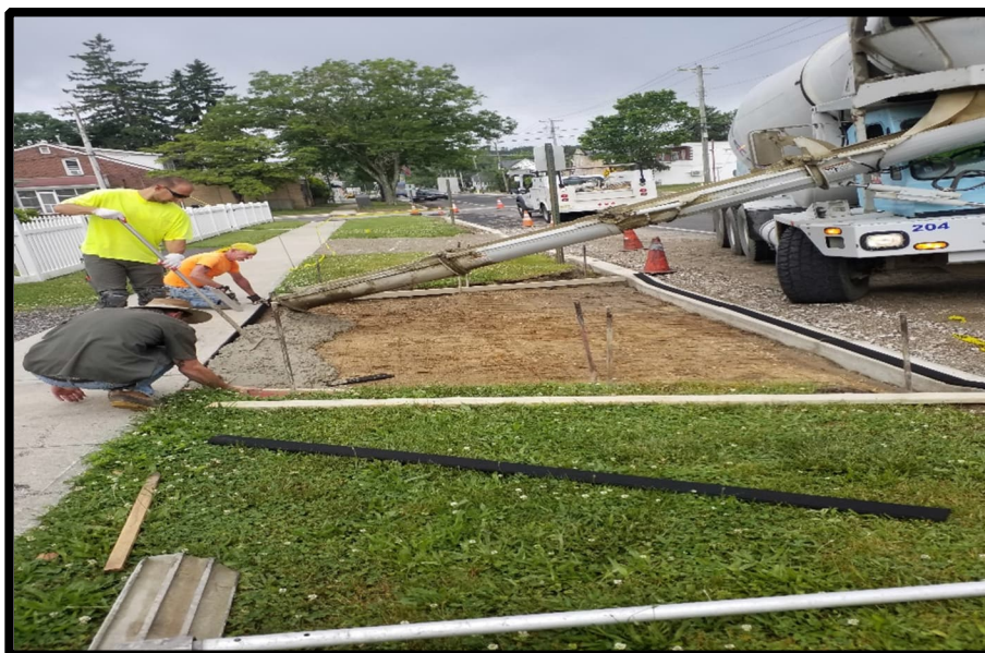
Photograph 6 – Pouring Concrete Driveway Apron.
