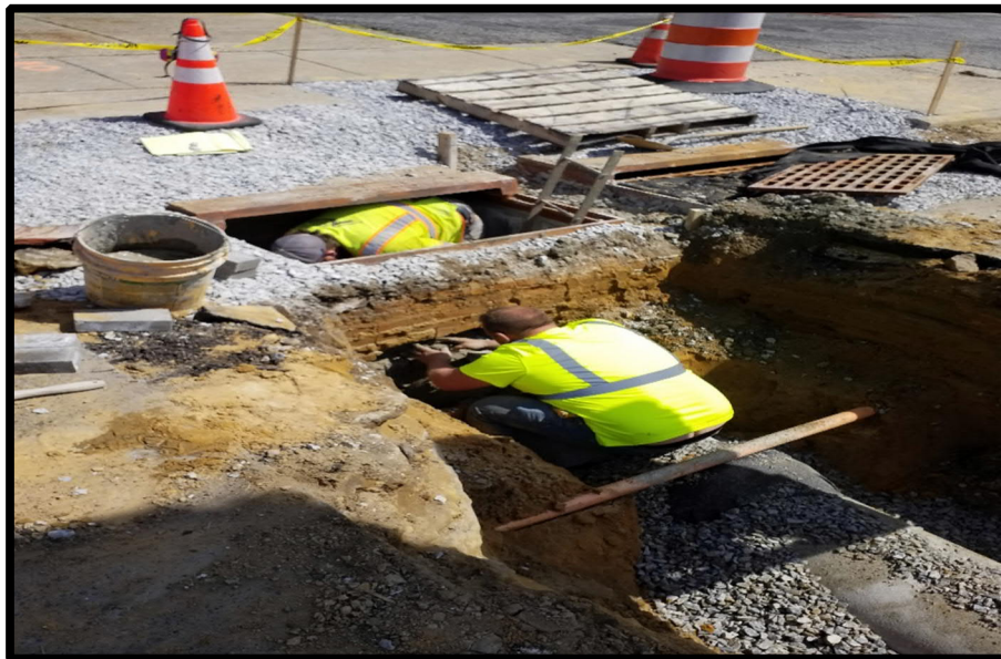
Photograph 3 – Pipe Crew connecting new pipe to "B" inlet
