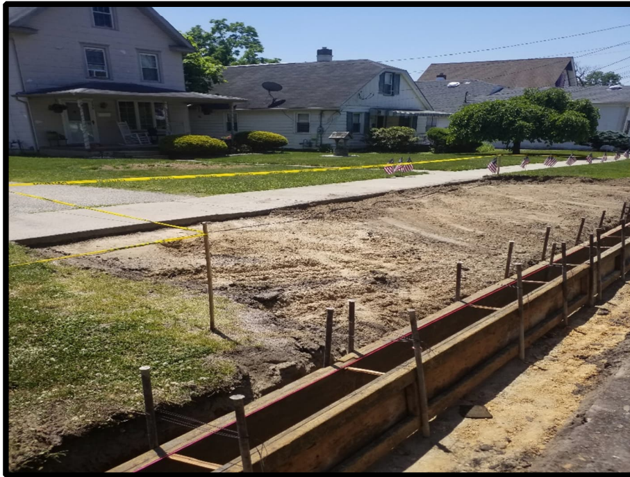
Photograph 2 – Curb Crew forming for vertical curb near Church Street.
