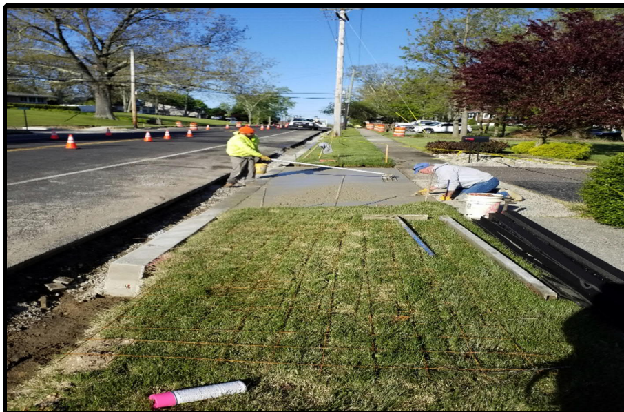
Photograph 7 – Finishing concrete apron near second.
