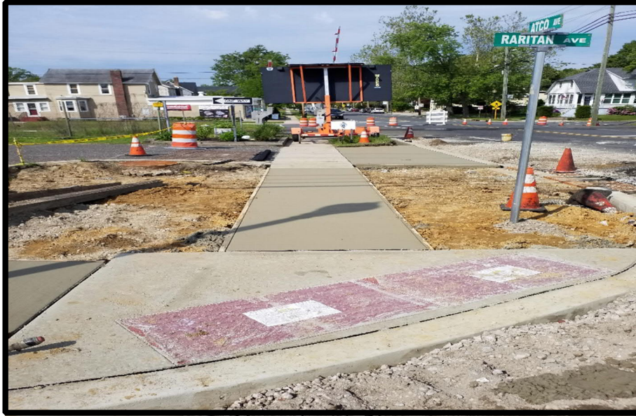
Photograph 4 – Handicap Ramp and sidewalk @ Raritan Avenue.
