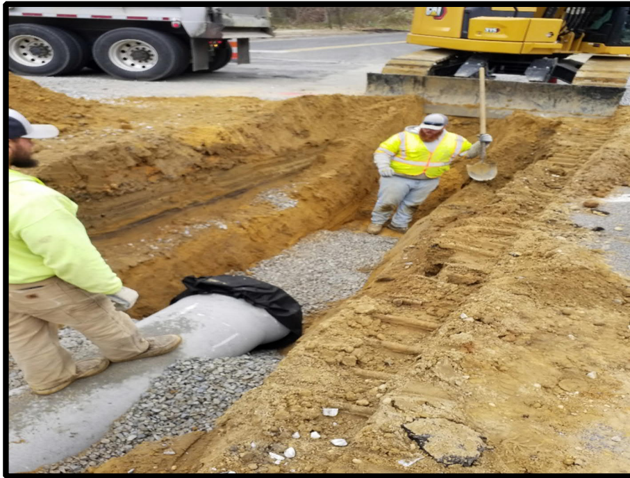
Photograph 2 – Pipe Crew installing drain pipe at Raritan ave.
