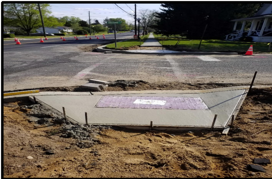
Photograph 4 – Curb Crew forming for vertical curb and handicap ramps at Second Street.
