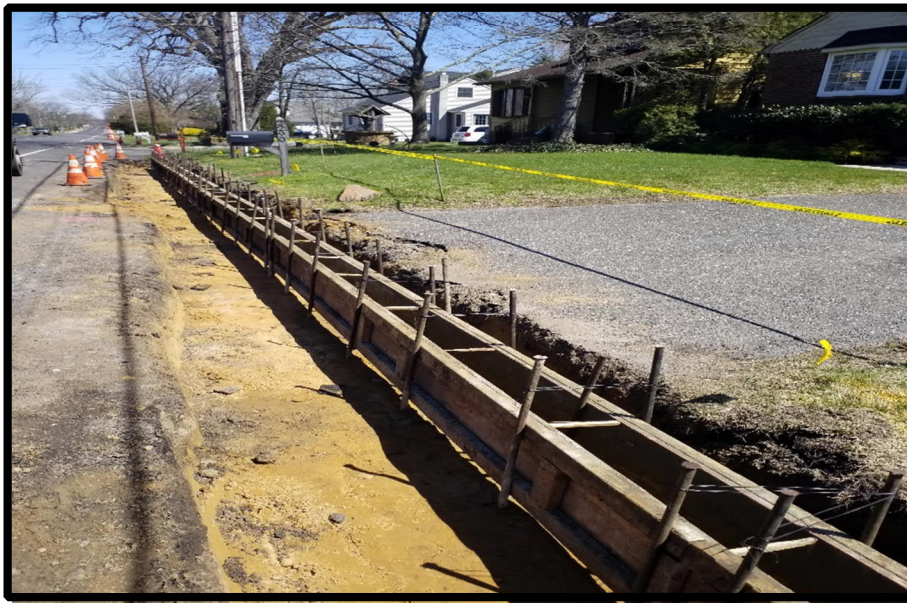
Photograph 5 – Forming for new curb.
