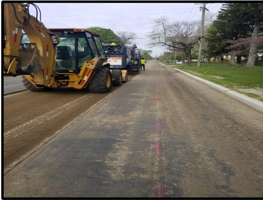
Photograph 2 – Road Crew milling to grade.
