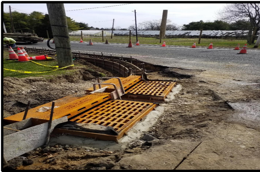
Photograph 4 – Installing New “B” Inlet and Drainage pipe under existing utilities.
