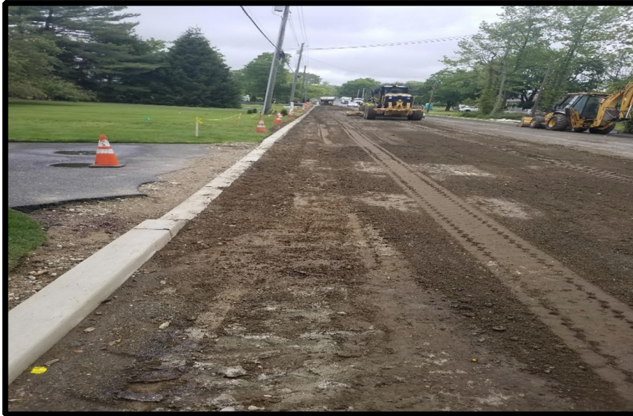
Photograph 6 – Full Depth reclamation Crew operation.
