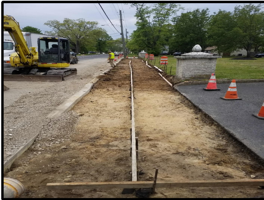
Photograph 1 – Curb Crew forming for sidewalk.
