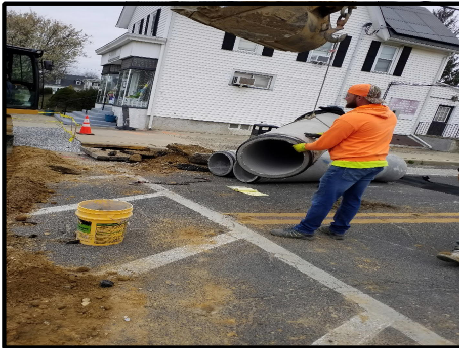
Photograph 1 – Pipe crew installing drainage pipe at Atco & Raritan aves.
