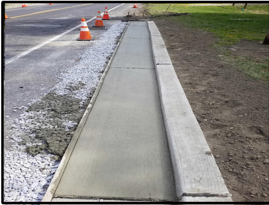
Photograph 1 – Contractor poured Concrete Gutter.
