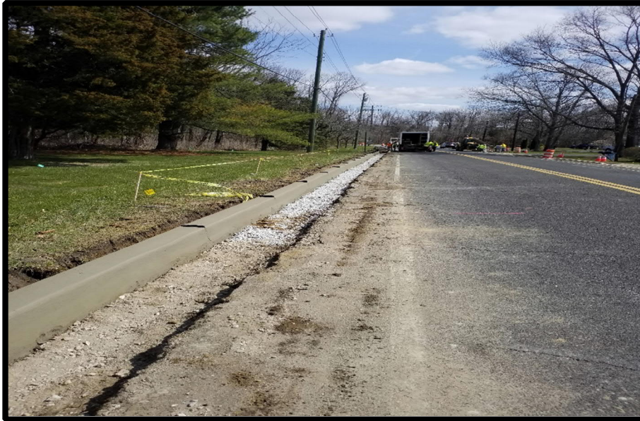
Photograph 6 – Progressing with Vertical Curb.
