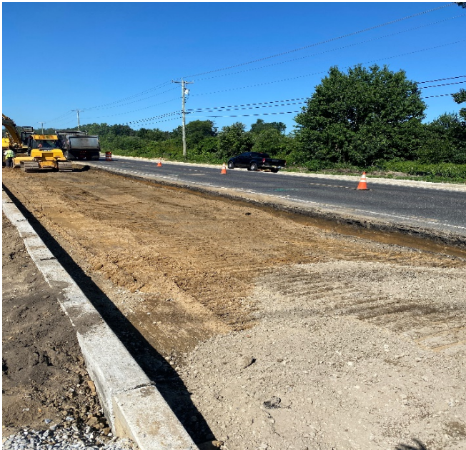
Figure 1: DGA Roadway Boxout (8" Thick)
