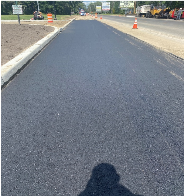
Figure 1: HMA25M64 Base Installation
