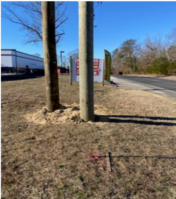
Figure 1: ACE Relocating Utility Pole
