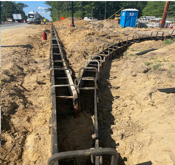
Figure 2: 9"X18" Concrete Vertical Curb Forms
