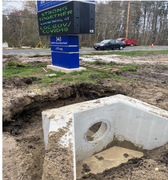
Figure 2: Headwall installation at CCTS
