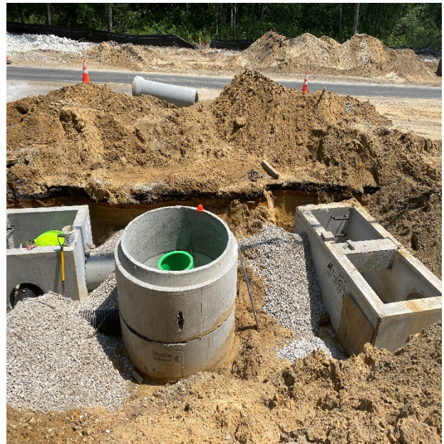
Figure 1: Riprap placement at dropbox (Sta. 10+20, LT) Figure 2: Placement of Dual Vortex Separator and Inlets
