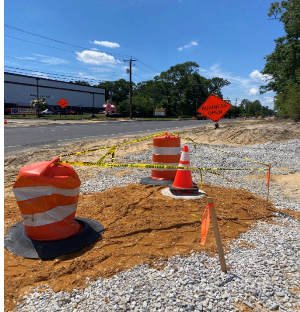
Figure 2: Light Post Foundation Installation
