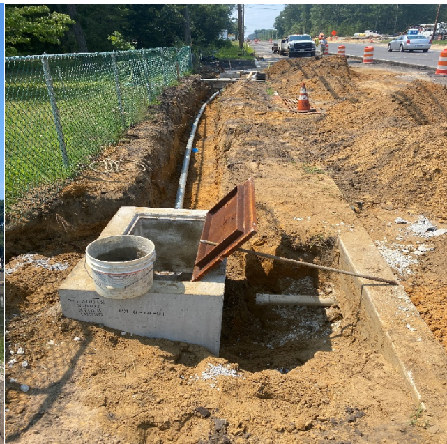
Figure 2: Junction Box/2" RMC Installation
