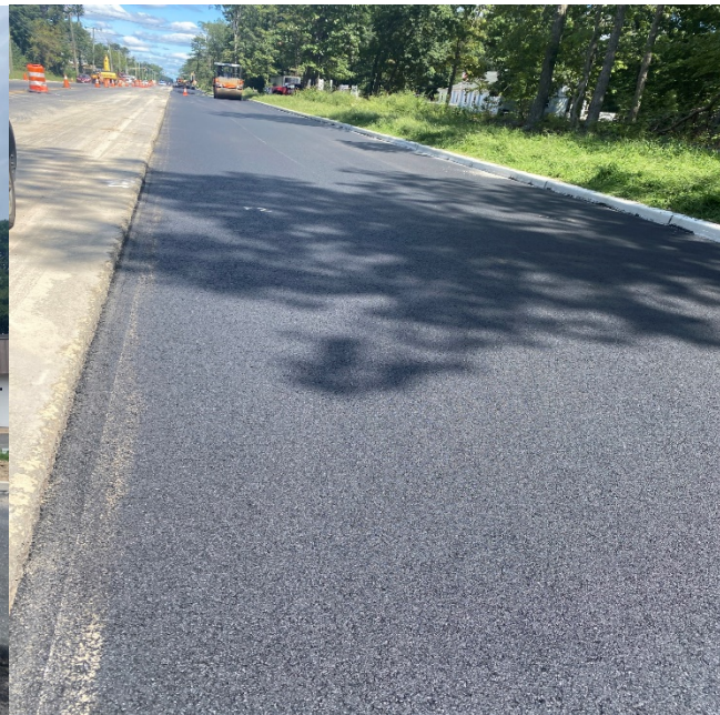
Figure 2: HMA Base Paving
