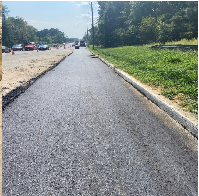
Figure 1: 12" DIP Water Main Repair (Thrust Blocks Added) Figure 2: 4" HMA Base Placement for Widening
