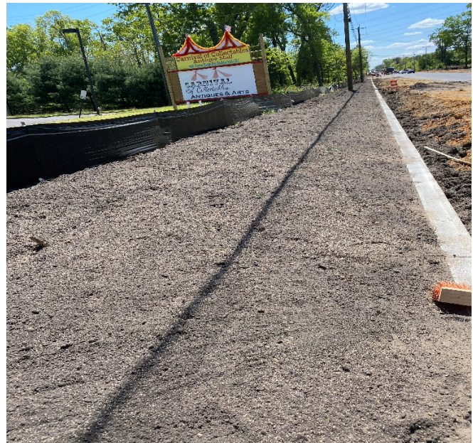
Figure 2: Topsoil/Seed placement behind new curb
