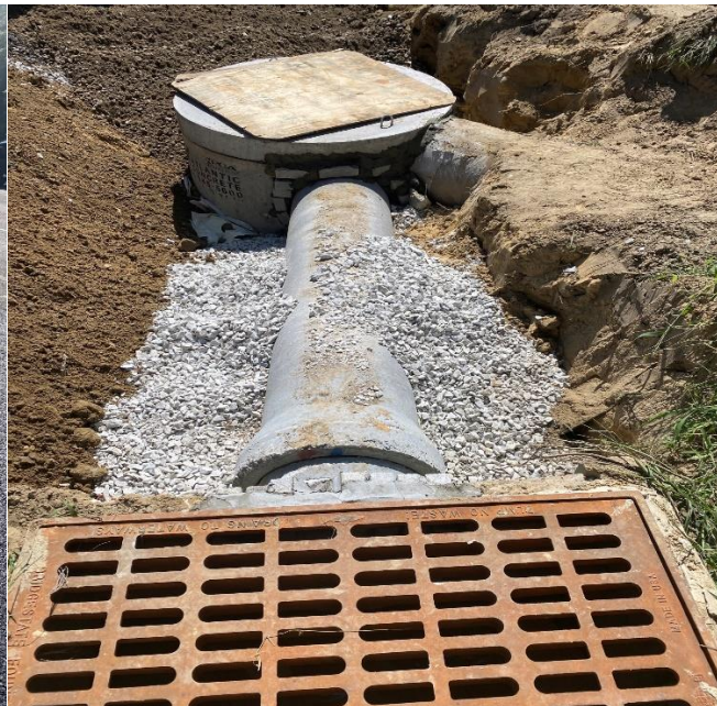
Figure 2: Manhole and Reinforced Concrete Pipe Placement
