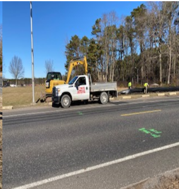
Figure 2: P&A Construction Installing Silt Fence
