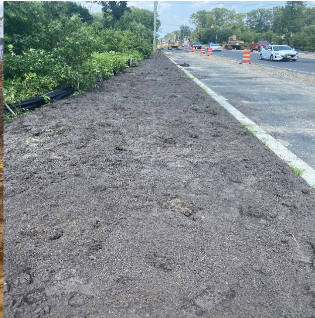
Figure 2: Topsoil/Seed Placement on Berlin Cross Keys Rd
