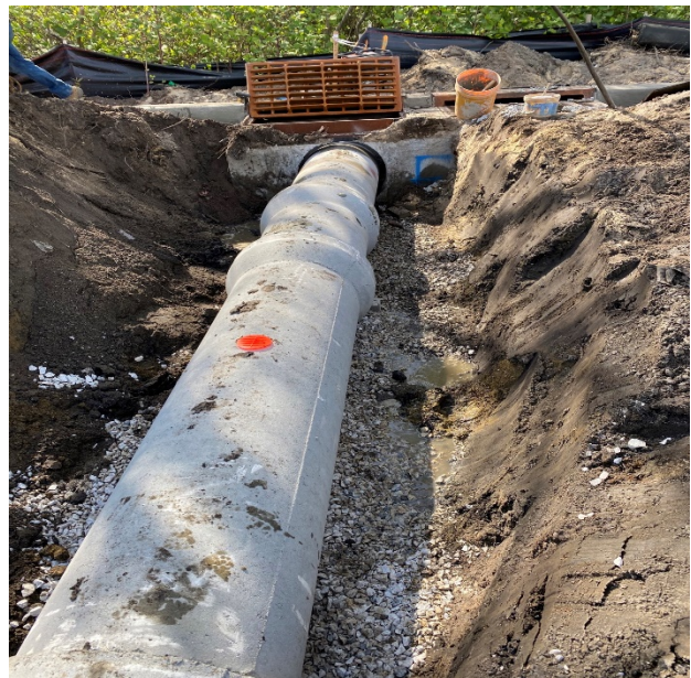
Figure 2: Pipe crossing installation
