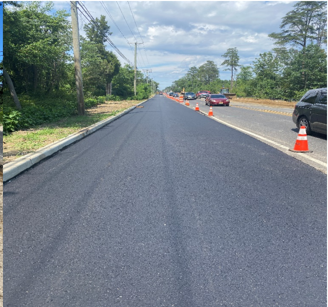
Figure 2: HMA 25M64 Base Paving
