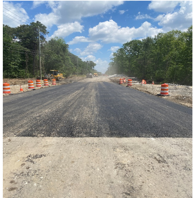
Figure 1: Dropbox installation for 20-18" Pipe Crossing Figure 2: HMA Paving over 20-18" DIP Crossing
