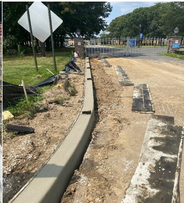
Figure 2: 9"X18" Concrete Vertical Curb Radius
