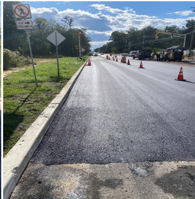
Figure 2: HMA Intermediate Course Placement
