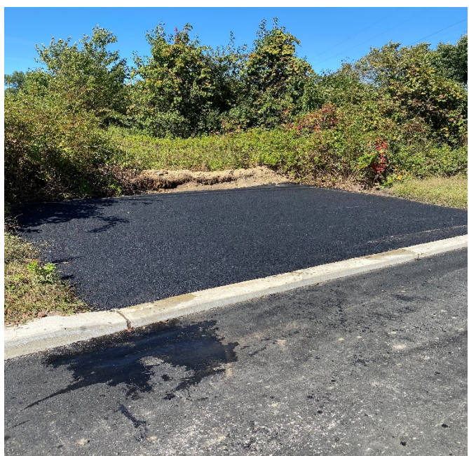
Figure 2: HMA Driveway Apron
