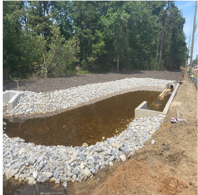
Figure 2: Topsoil placement behind Riprap/Dropbox
