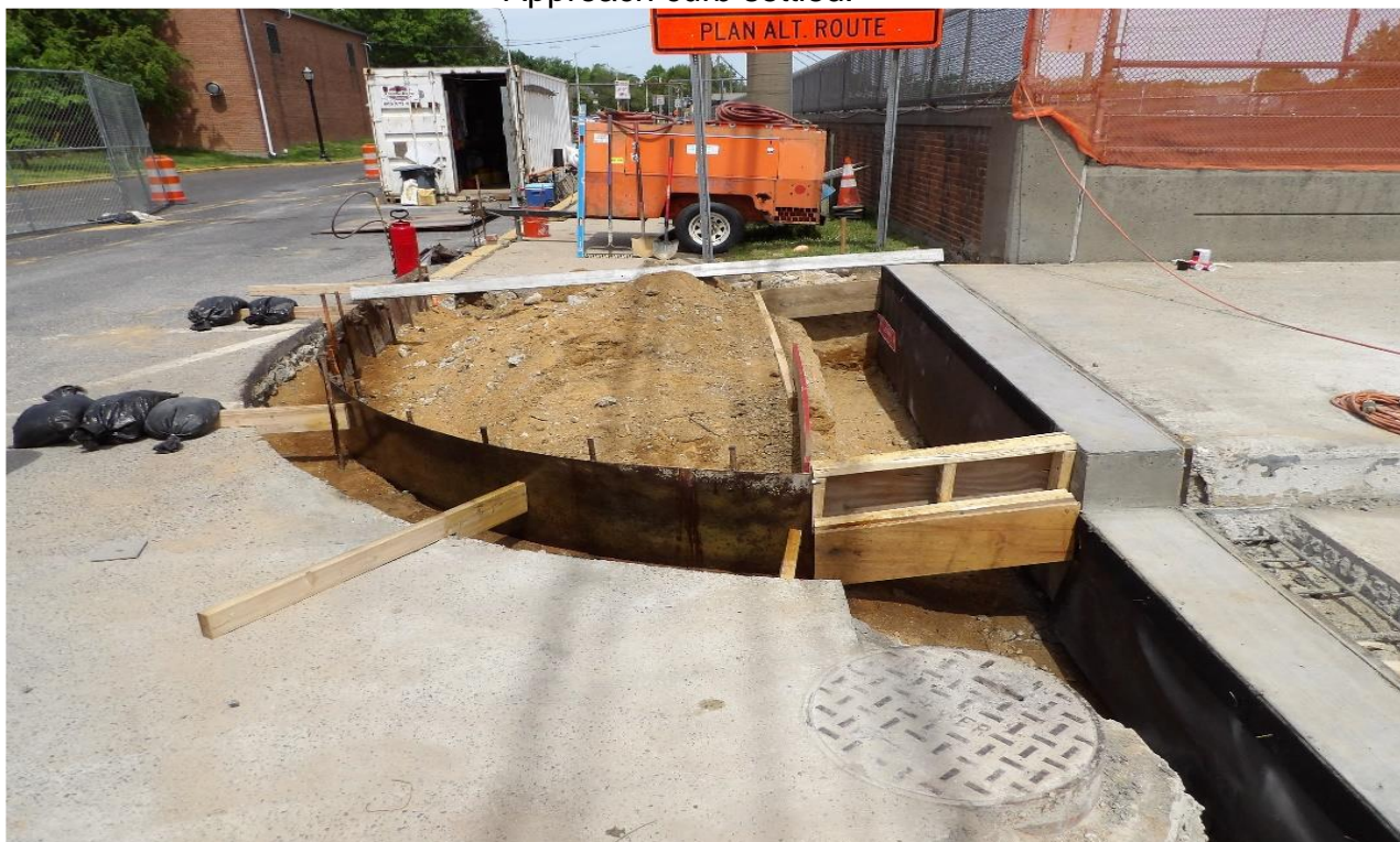
AFTER: Handicap Ramp and Curb during construction
