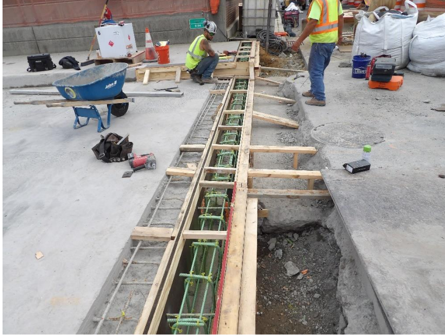
Figure 8 – Workers completed the west header formwork
