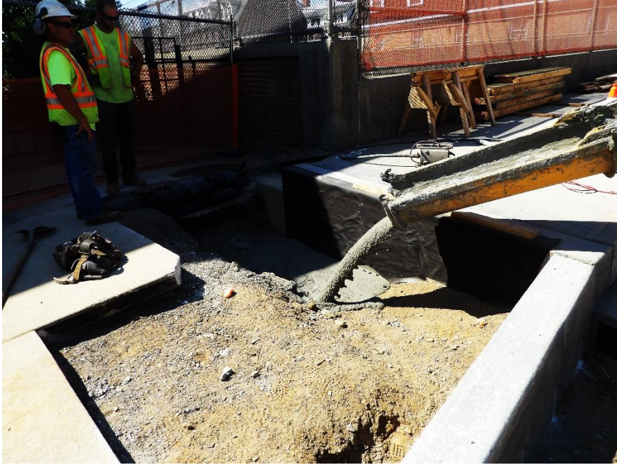
Figure 8 – Excavations behind the abutments were filled with flowable concrete fill
