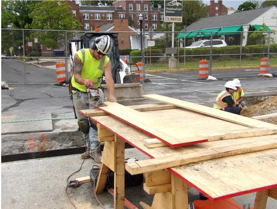
Figure 8 – Worker fabricating header formwork
