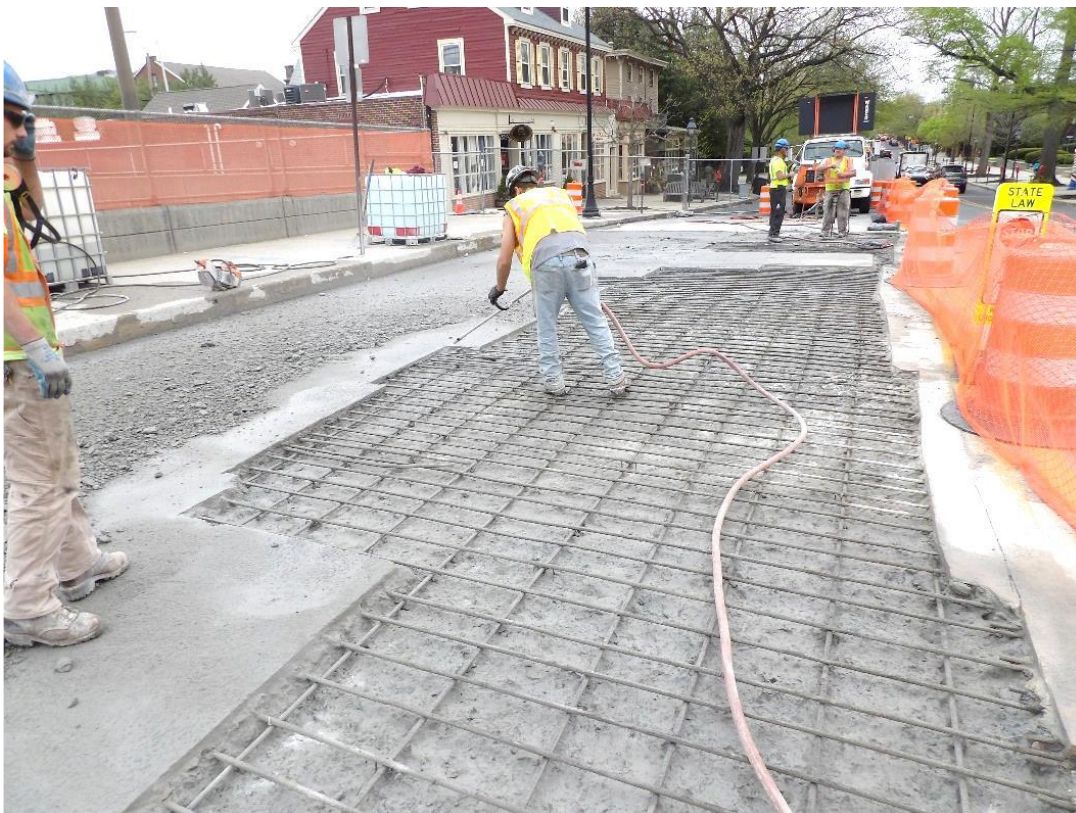
AFTER: Deck Concrete Base Repair during Construction
