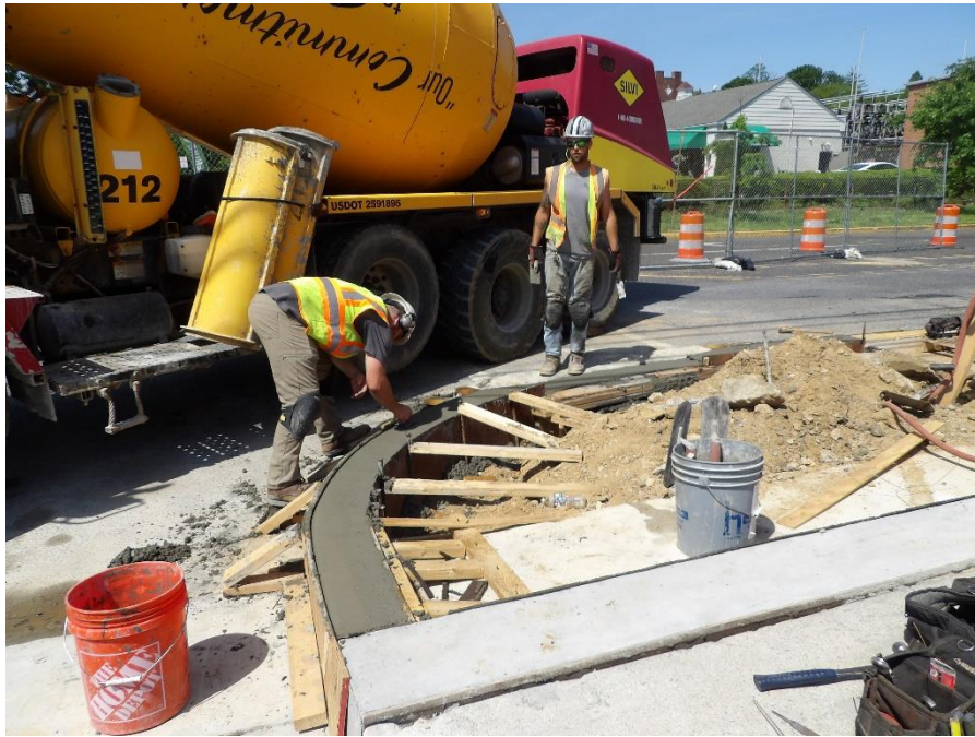
Figure 2 – Workers poured the approach curb concrete, Stage 1
