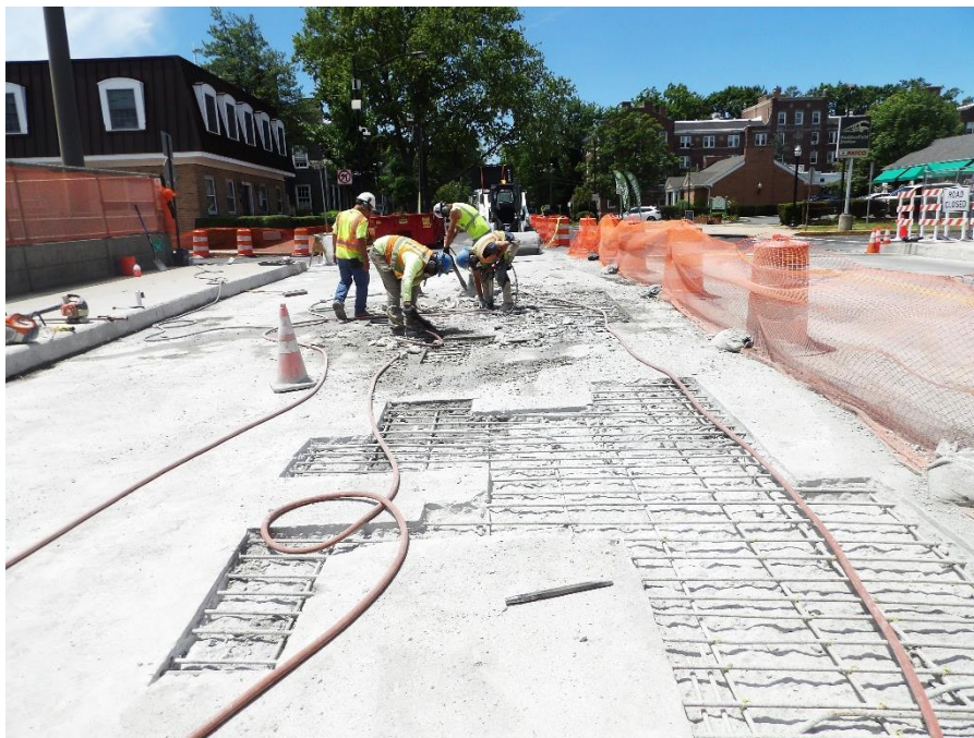
Figure 7 – Workers made progress with deteriorated concrete removal in the inner lane
