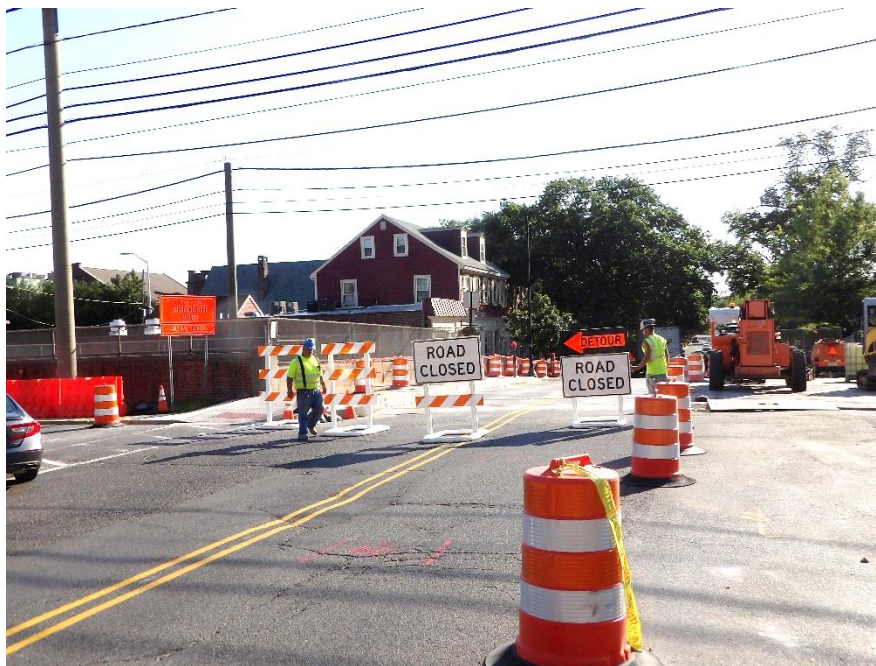
Figure 1 – Workers closed the Kings Highway bridge and set up the detour
