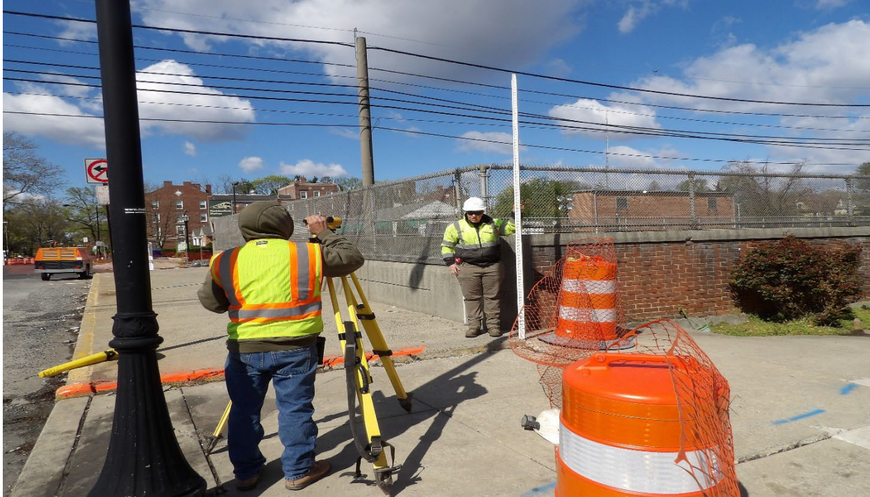
Figure 8: Survey of Existing Deck for Stage 1 construction.
