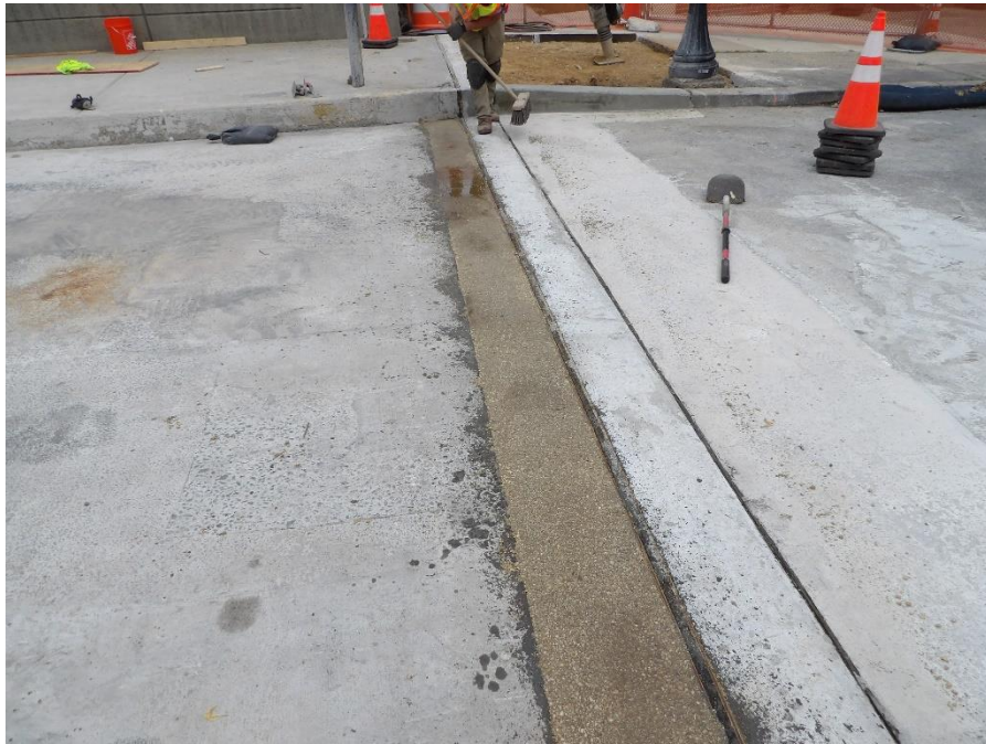
Figure 8 – Both deck end joint PPC pours were completed
