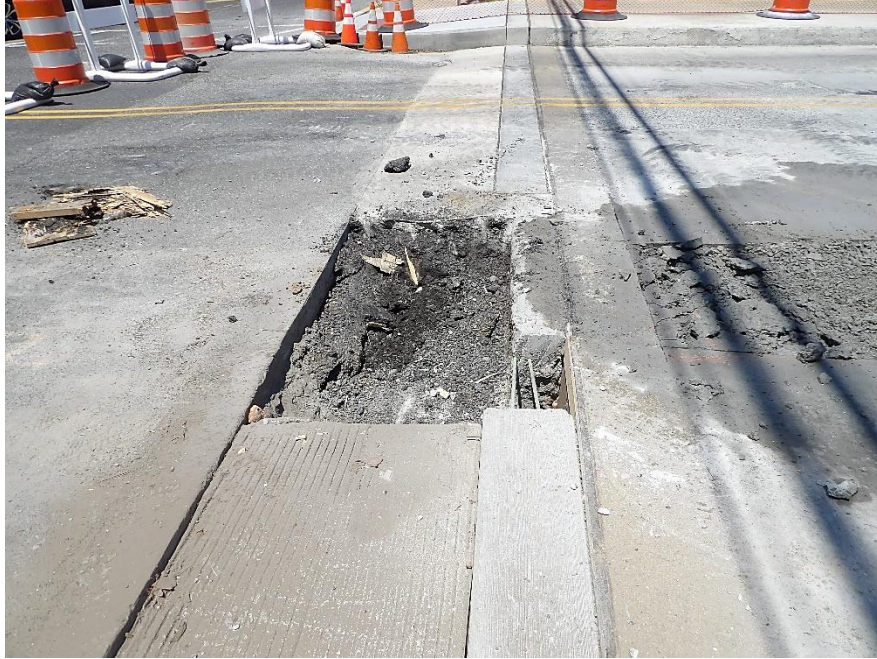
Figure 4 – The existing headers were excavated for removal
