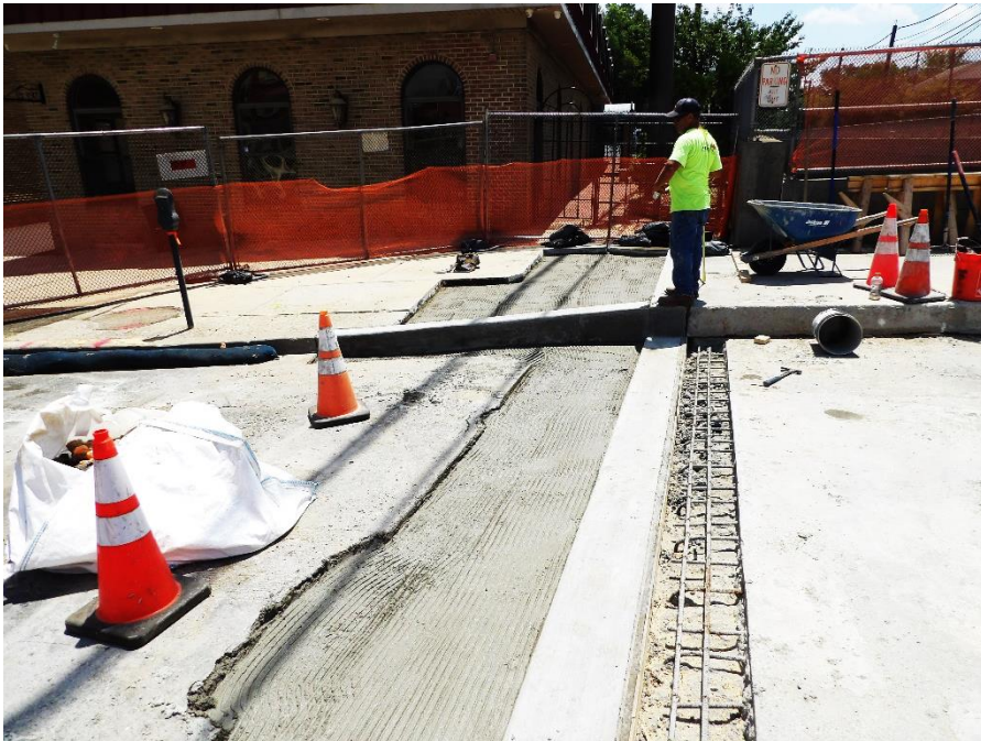
Figure 9 – Flow fill backfilling was completed, work will resume Tuesday, July 5th
