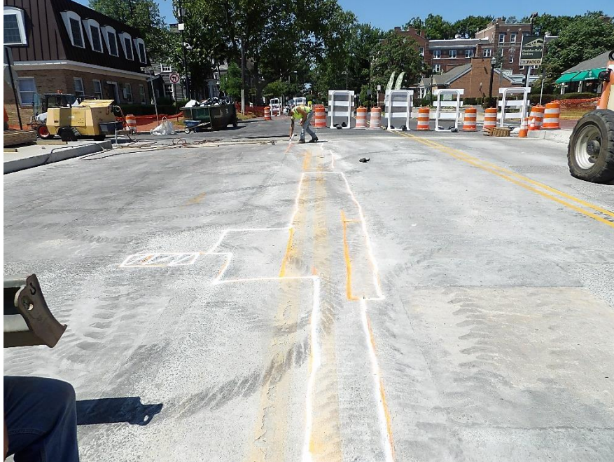
Figure 2 – Stage 3 deck was marked out for deteriorated concrete removal
