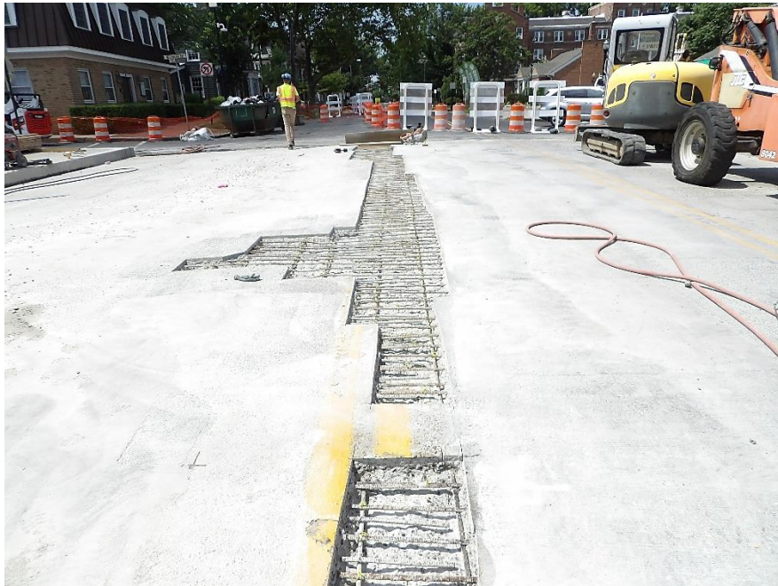
Figure 7 – Workers completed the deteriorated concrete removal from the top of deck
