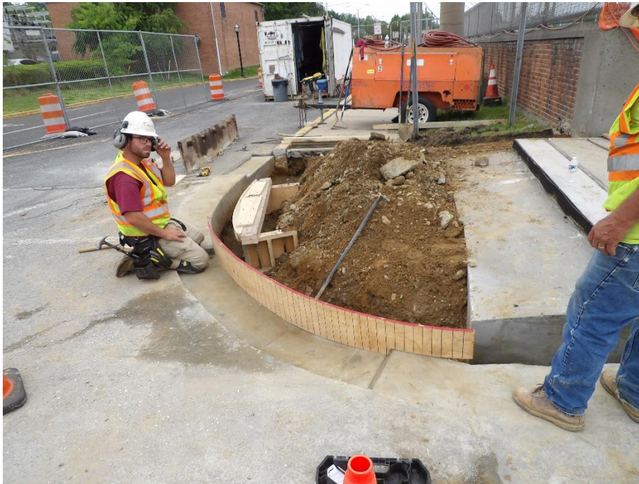
Figure 10 – Workers began forming curbs and sidewalks
