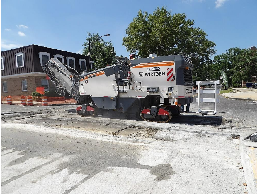
Figure 4 – The deck and approach roadways were milled for repaving
