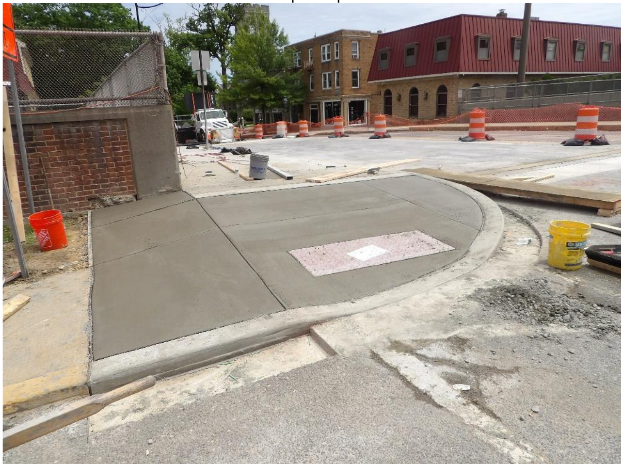
AFTER: Handicap Ramp improved
