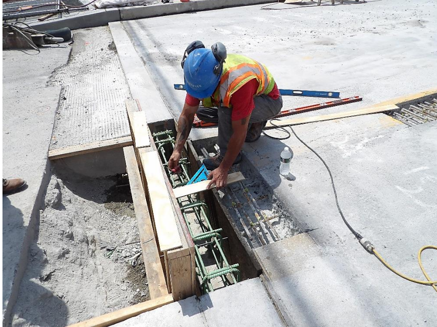
Figure 6 – New header rebar and formwork was installed
