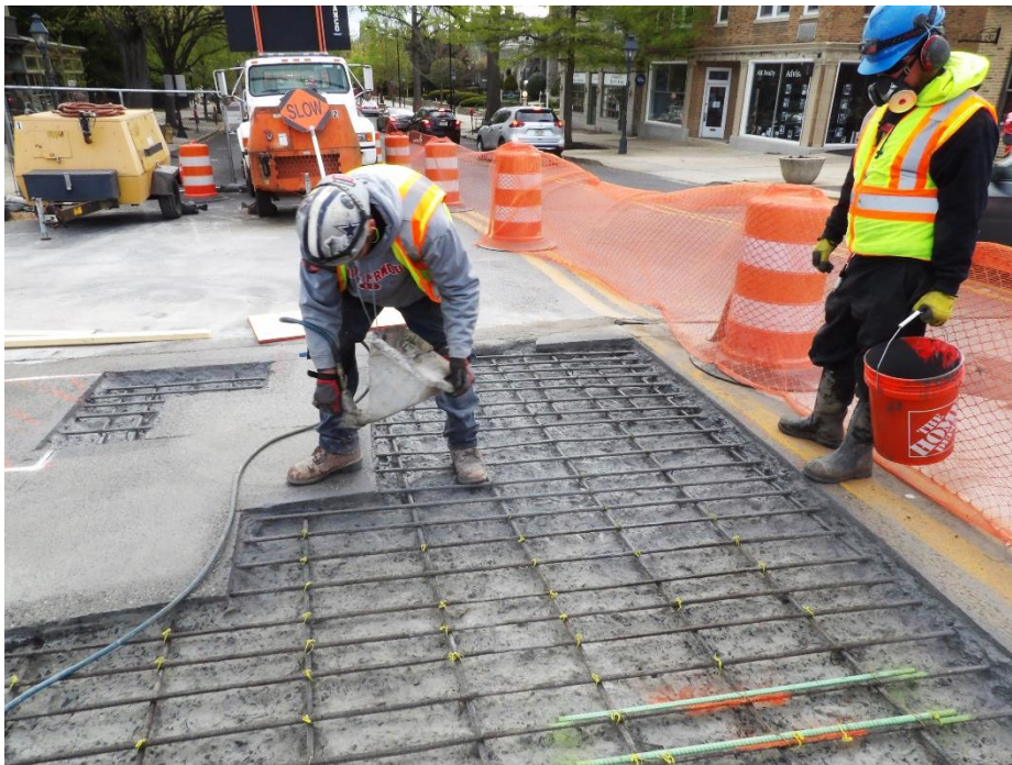
Figure 7 – Epoxy concrete bonding agent applied to concrete and reinforcing
