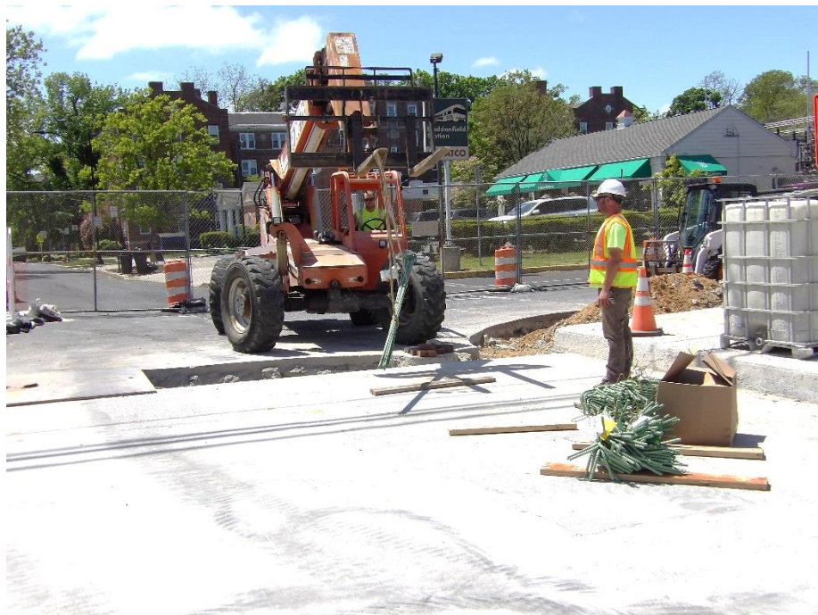
Figure 7 – New header reinforcing arrived and unloaded
