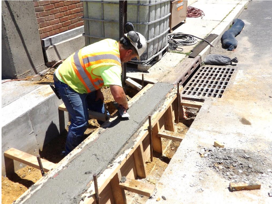
Figure 6 – New approach curb concrete was poured and finished
