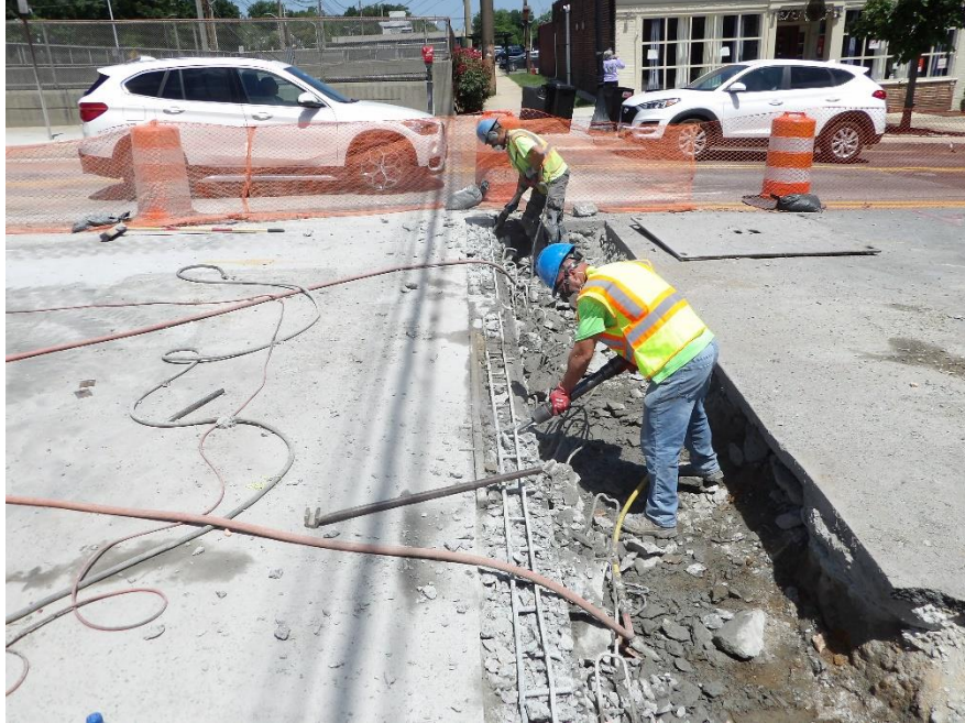
Figure 2 – Excavations were completed, and header demolition began
