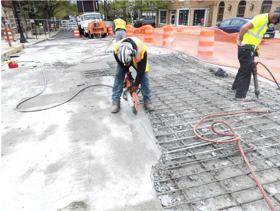
Figure 2 – Workers begin removal of deteriorated concrete areas
