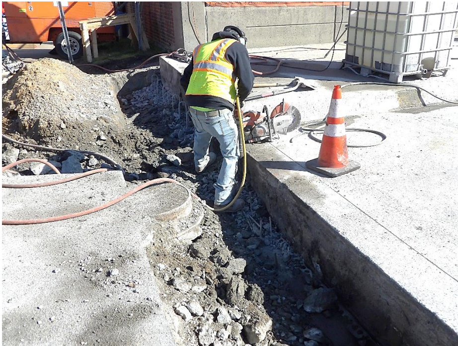
Figure 1 – Demolition of the existing west abutment header
