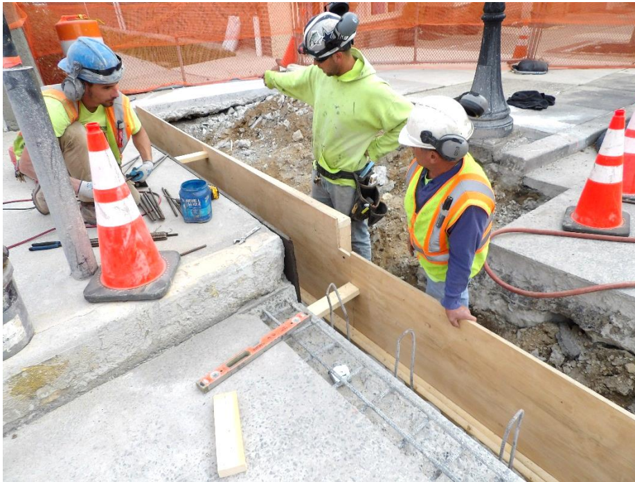
Figure 6 – New header formwork installation in progress
