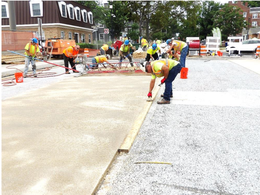
Figure 5 – PPC overlay progressed, and forms stripped
