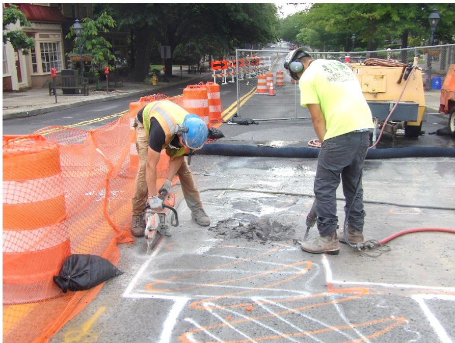
Figure 7 – Workers marked out deteriorated areas for removal in the inner lane
