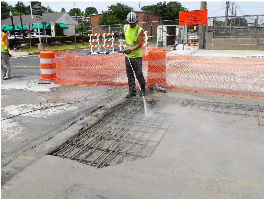
Figure 3 – Workers completed the removal for the second concrete pour and cleaned
