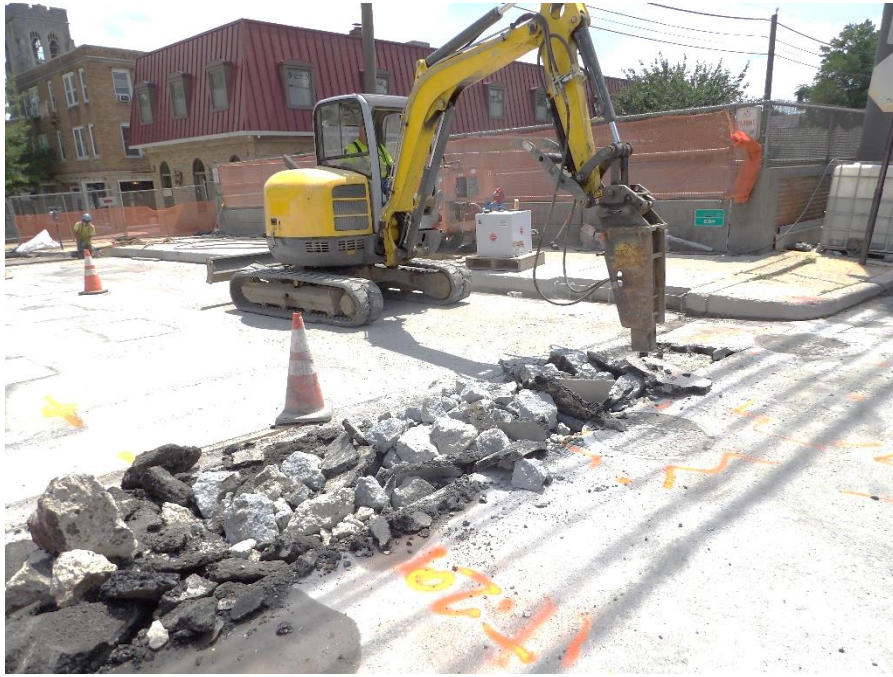
Figure 10 – Workers excavated behind the west abutment for header removal
