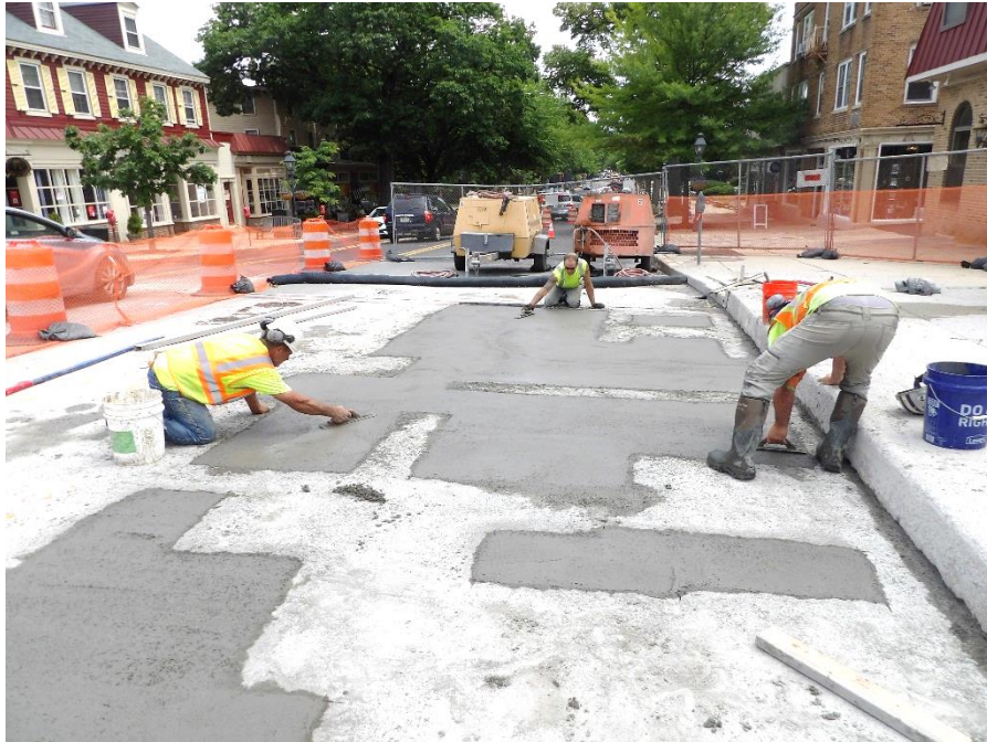
Figure 6 – Workers poured and finished the concrete patches
