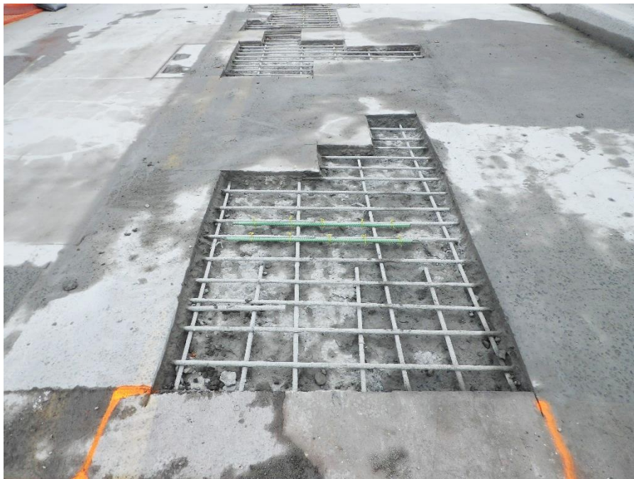
Figure 3 – Workers completed the removal for the first concrete pour
