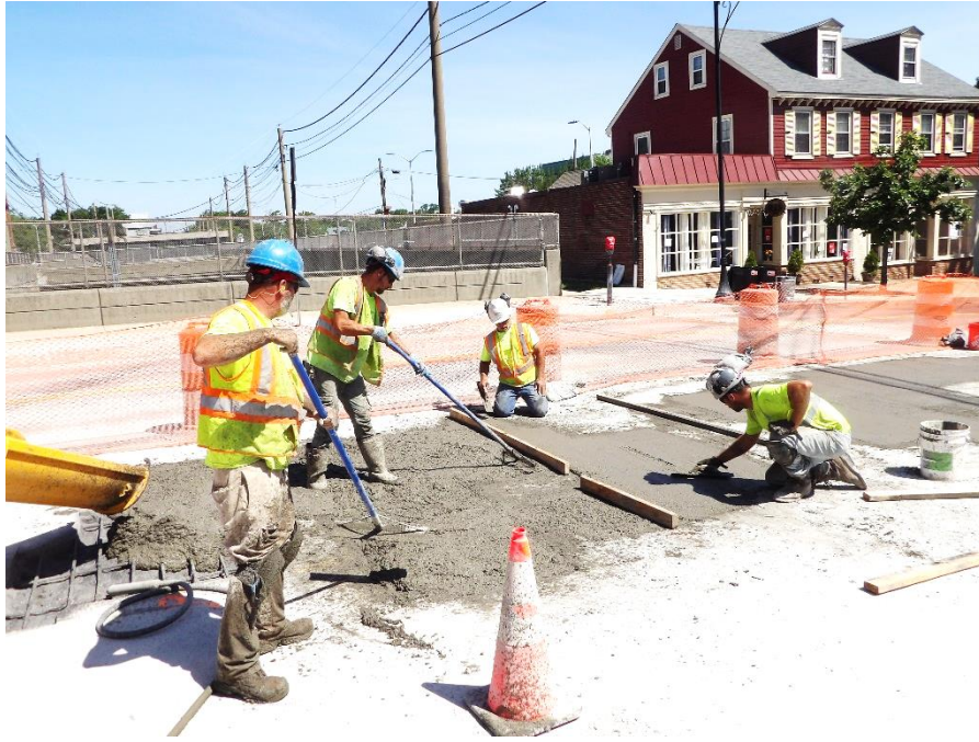
Figure 6 – Workers poured and finished the concrete patches
