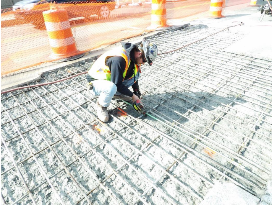
Figure 6 – Supplemental reinforcing tied in where required
