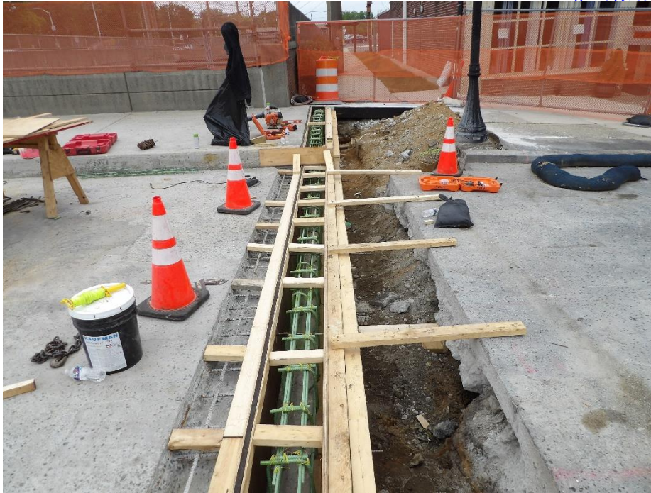
Figure 2 – Workers completed formwork installation for both new headers, Stage 1
