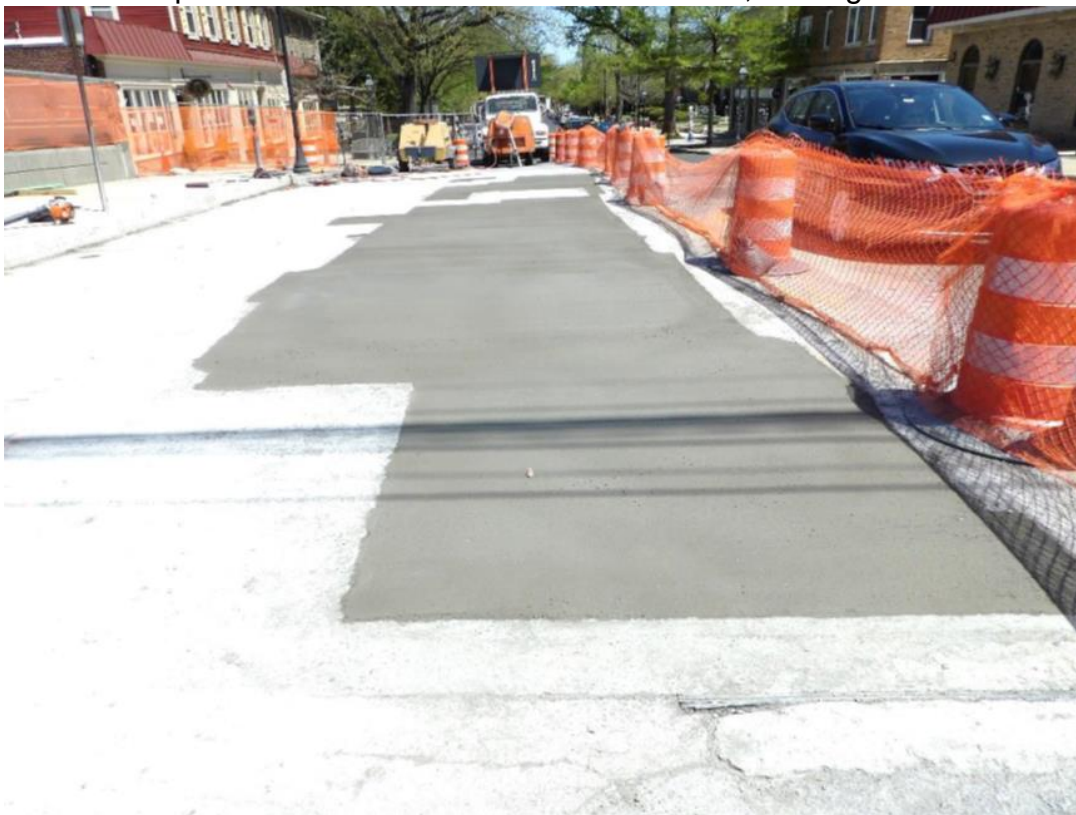
AFTER: Full depth Concrete repair done
