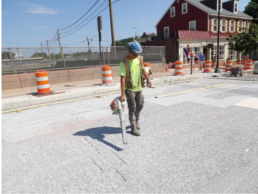
Figure 8 – Workers cleaned the deck prior to form and rail installation
