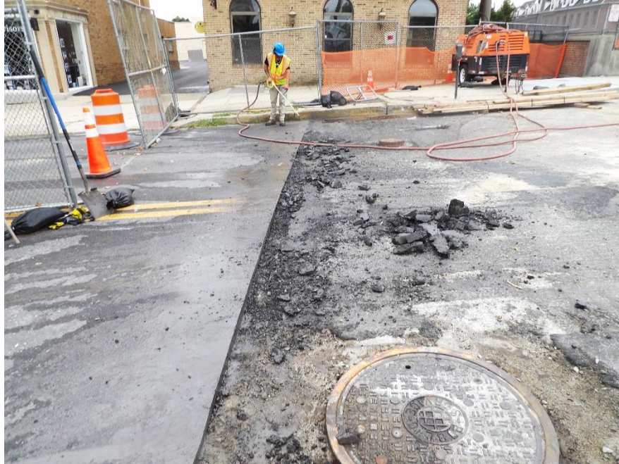
Figure 8 – Workers began preparing the approach roadways for re-paving
