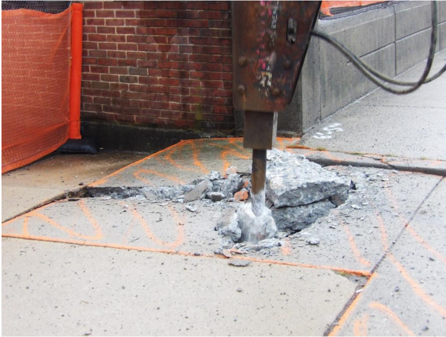
Figure 8 – Workers began removal of approach sidewalks and curbs
