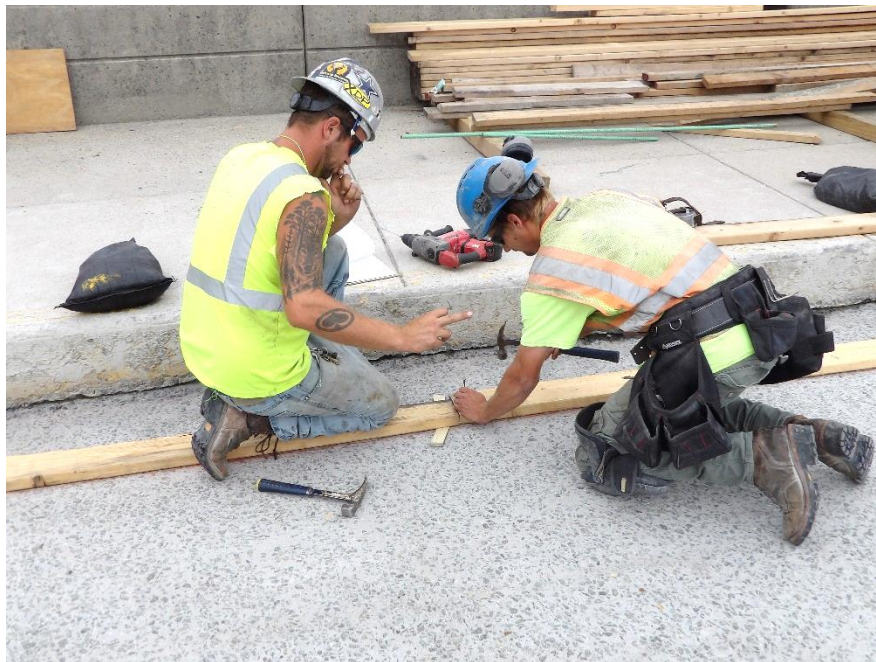
Figure 1 – Workers installed PPC deck forms
