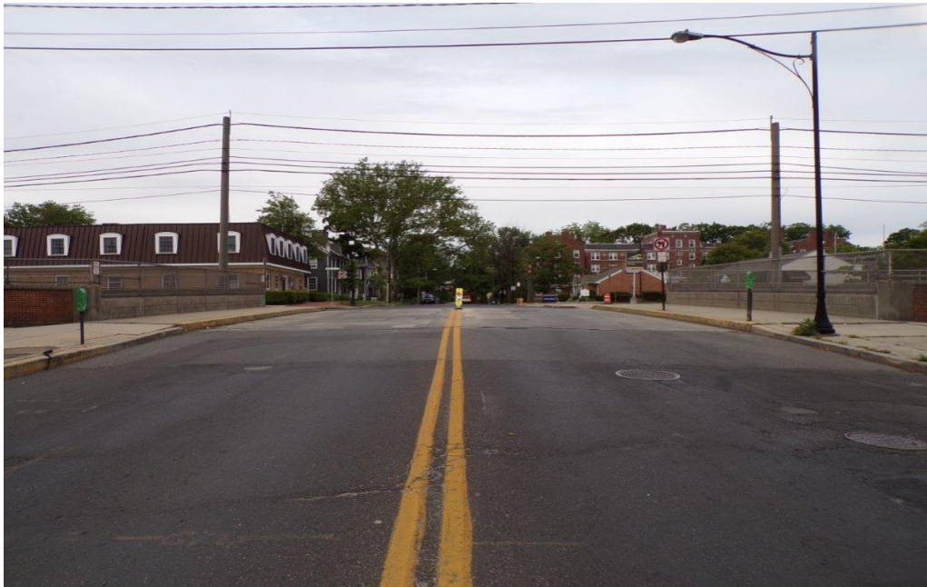
BEFORE– North Approach, looking south.
