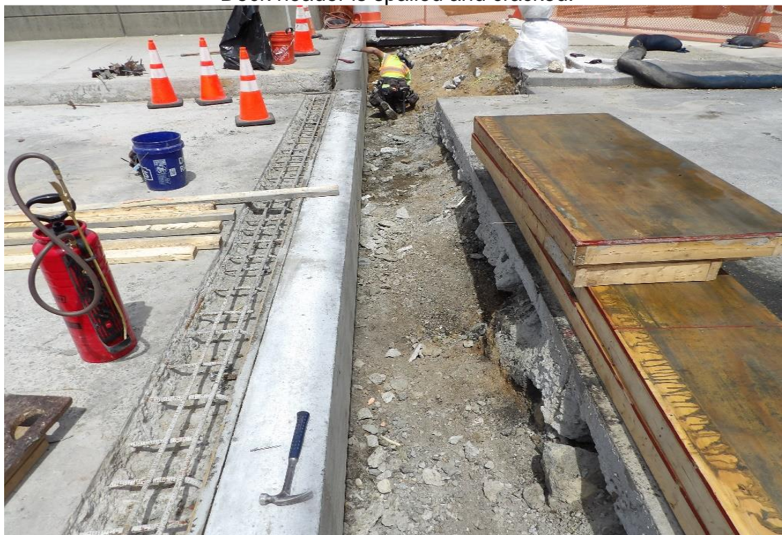
AFTER: Deck Header Repair during construction
