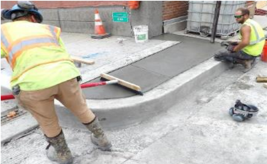
AFTER: Southeast corner after construction
