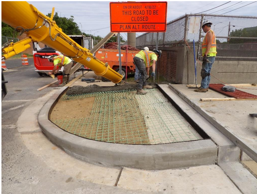
Figure 4 – Concrete for both north approach sidewalks was placed and finished
