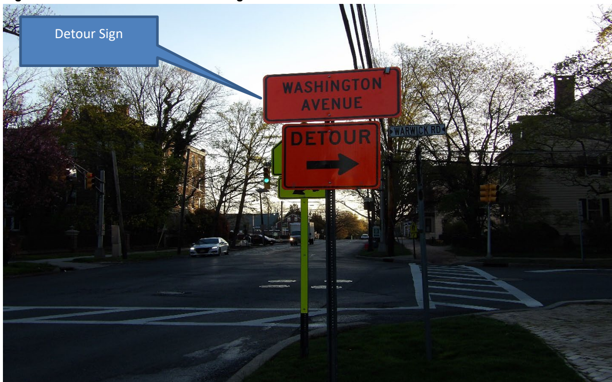
Figure 3 : Detour Signs for Stage 1 Construction
