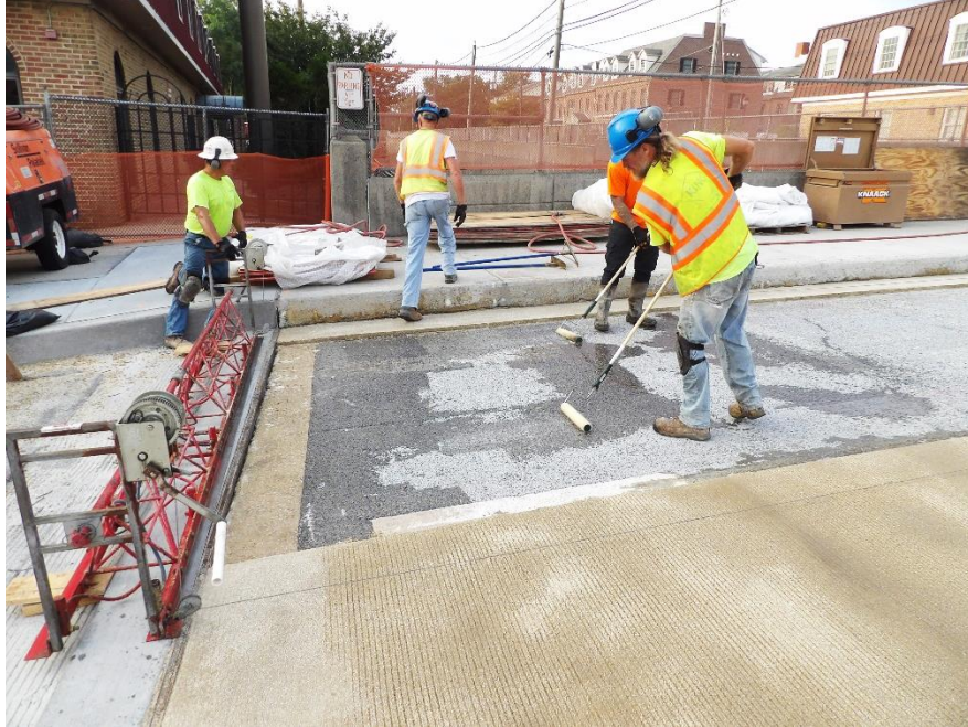
Figure 6 – Workers applied primer and continued to place PPC
