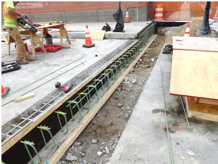
Figure 9 – Header reconstruction is in progress
