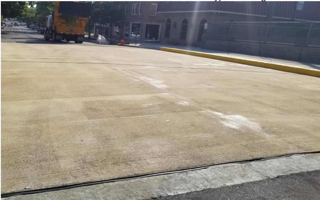
AFTER: General view of deck PPC Overlay
