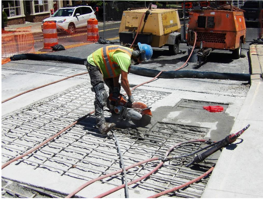
Figure 2 – Saw cutting and concrete removal progressed
