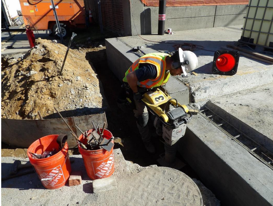
Figure 6 – Excavations behind the headers were compacted and prepared for backfill
