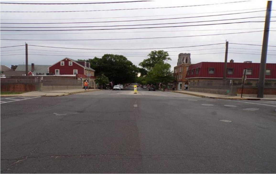
BEFORE: North Approach
