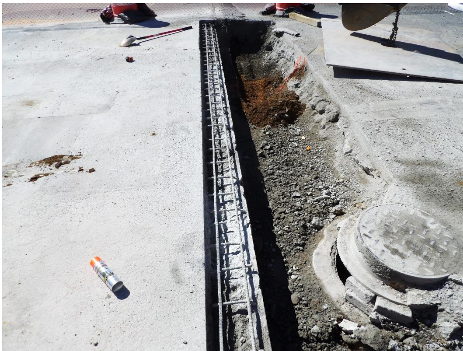
Figure 3 – Removal of existing headers and deck ends completed
