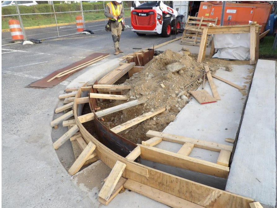
Figure 1 – Workers fabricated and installed new approach curb formwork
