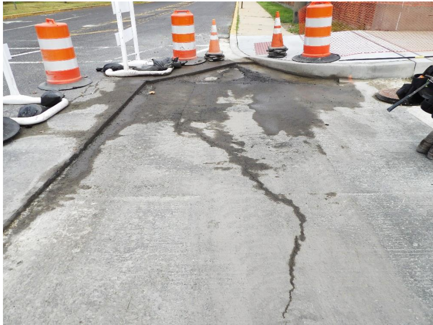
Figure 9 – Approach roadway pavement is prepared for paving
