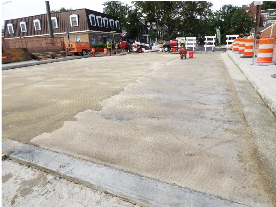
Figure 7 – Workers completed placing the overlay
