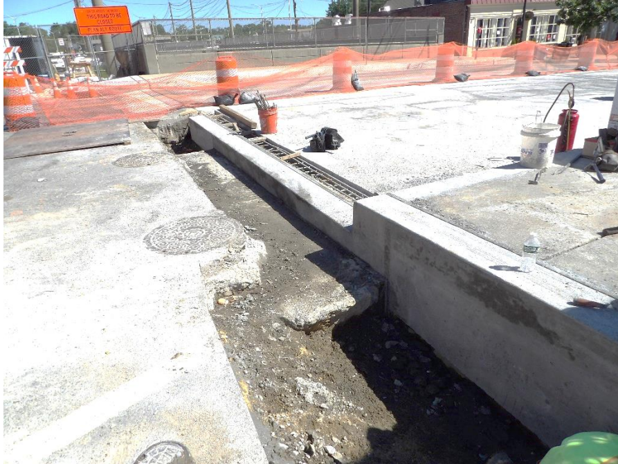
Figure 4 – Both abutment headers were completed in Stage 2
