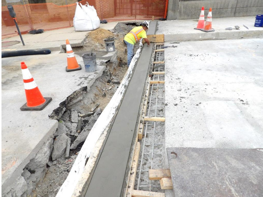
Figure 2 – New headers were poured and finished
