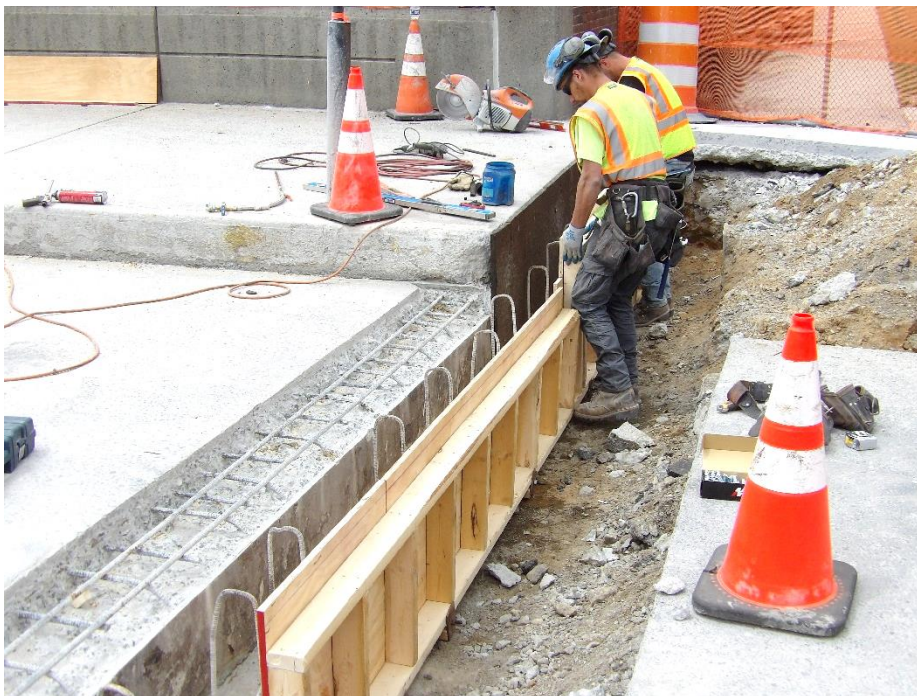
Figure 5 – Workers begin fabricating and installing header formwork
