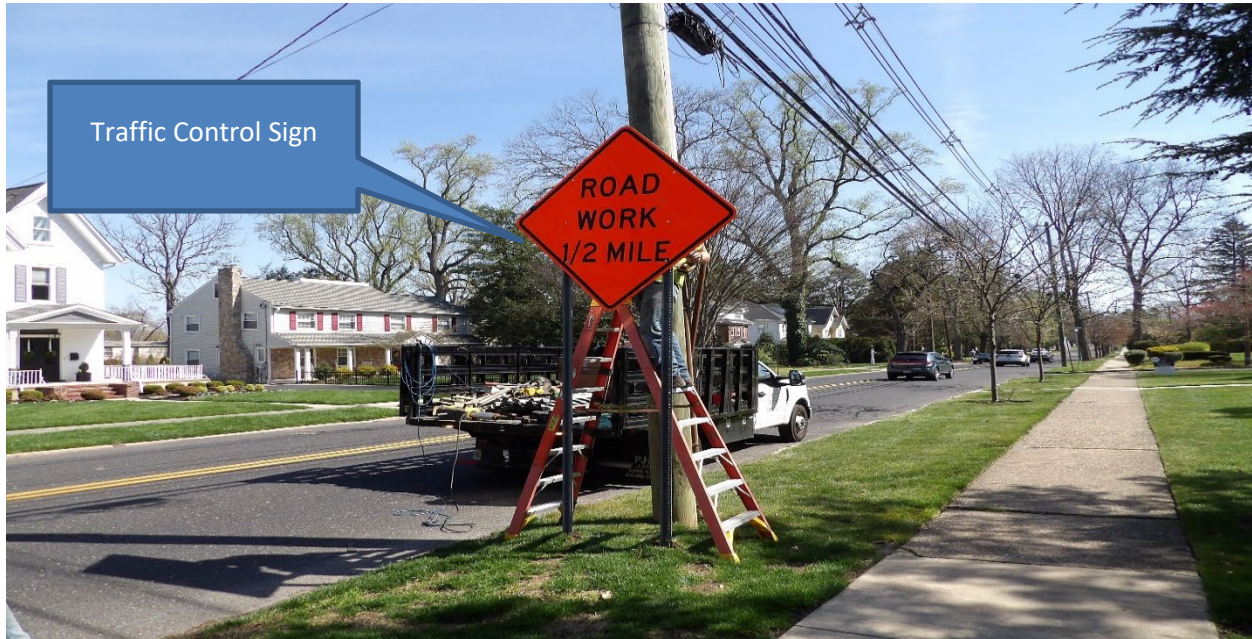
Figure 2: Traffic Control and Detour Signs were installed
