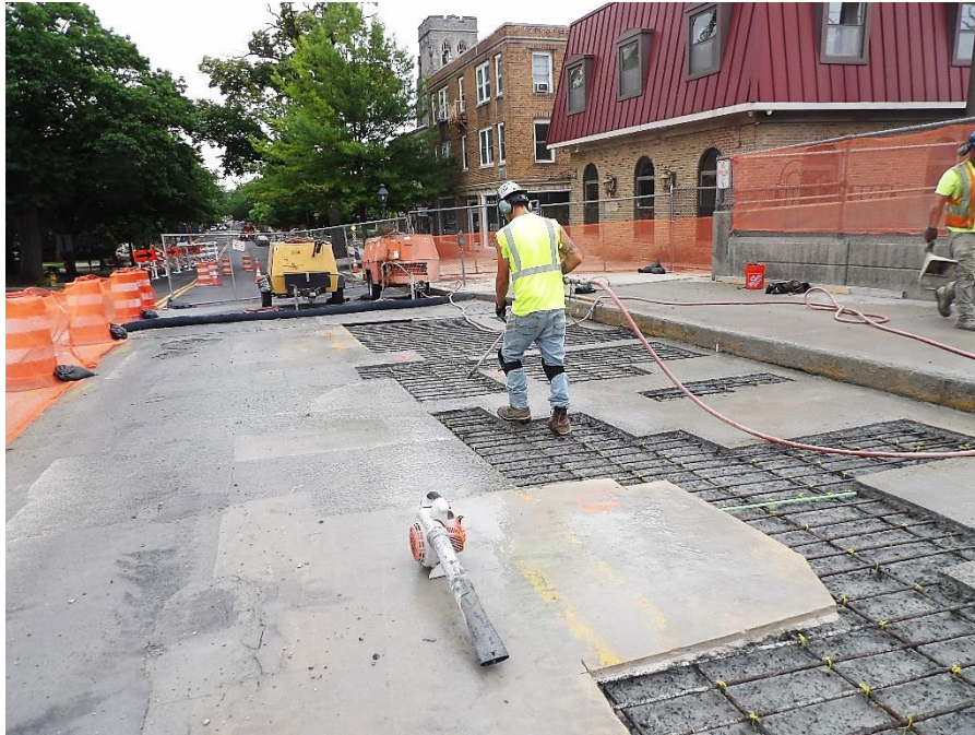
Figure 4 – Workers cleaned the areas to be patched
