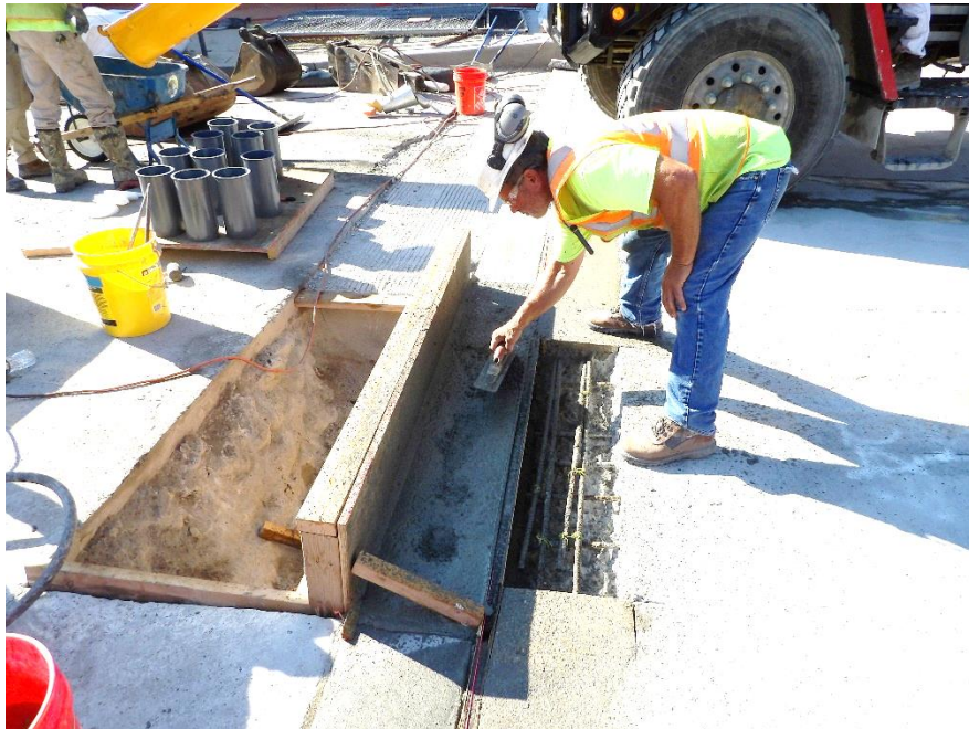
Figure 9 – Both abutment headers were poured and finished
