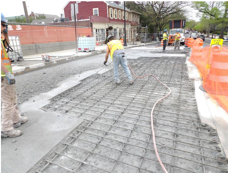
Figure 3 – Removal of deteriorated concrete progressed
