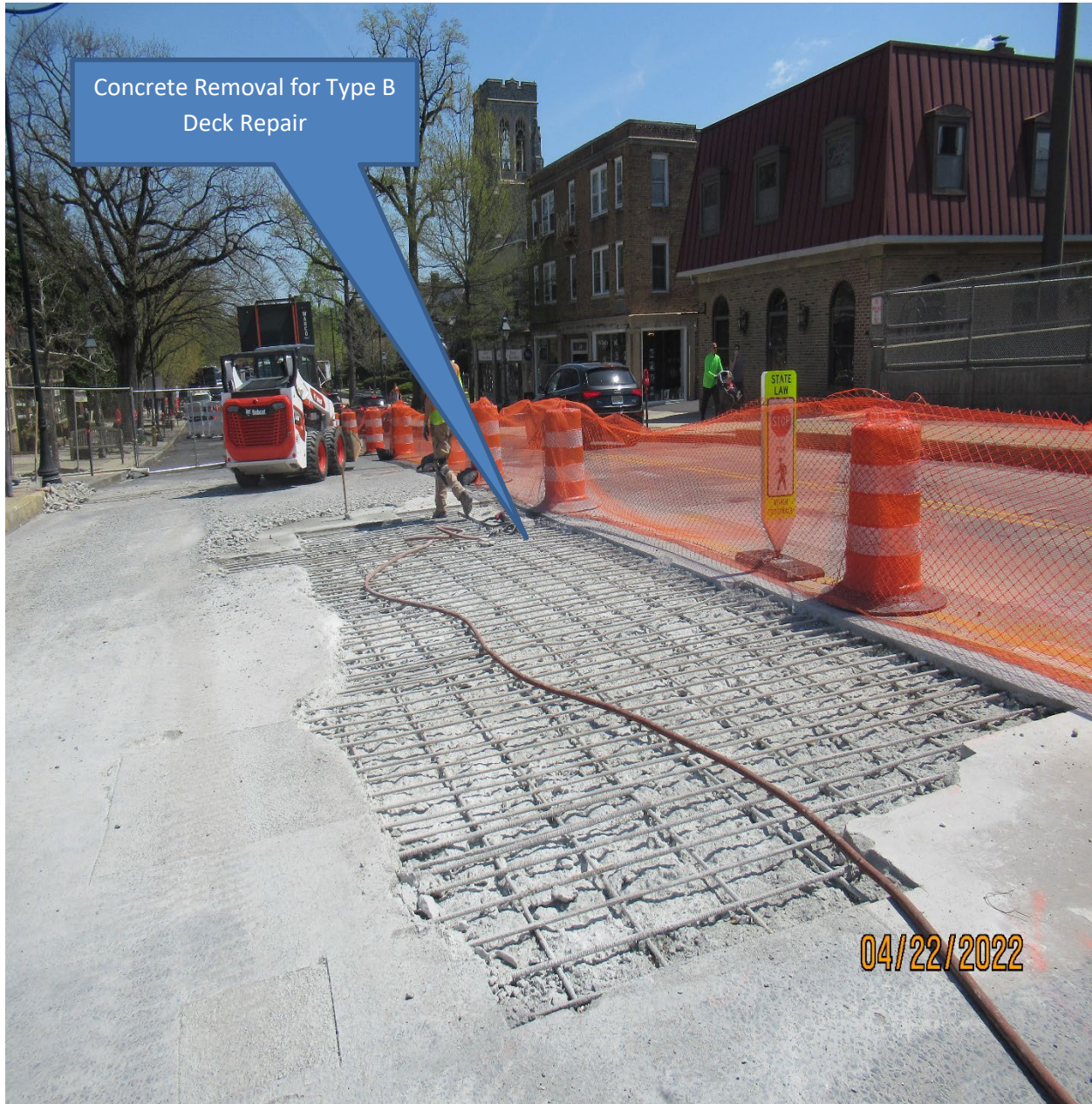
Figure 10: Stage 1 – Concrete removal is under progress for deck repair
