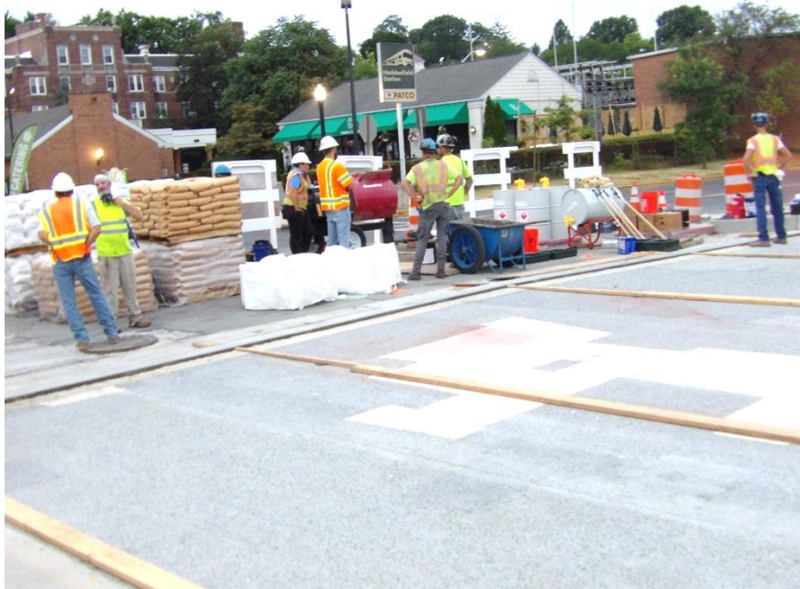
Figure 2 – PPC mixing station set up
