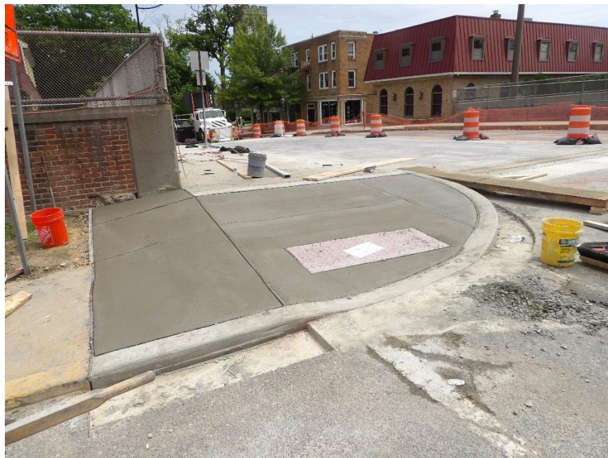
Figure 5 – New approach sidewalk with ADA ramp, northwest corner
