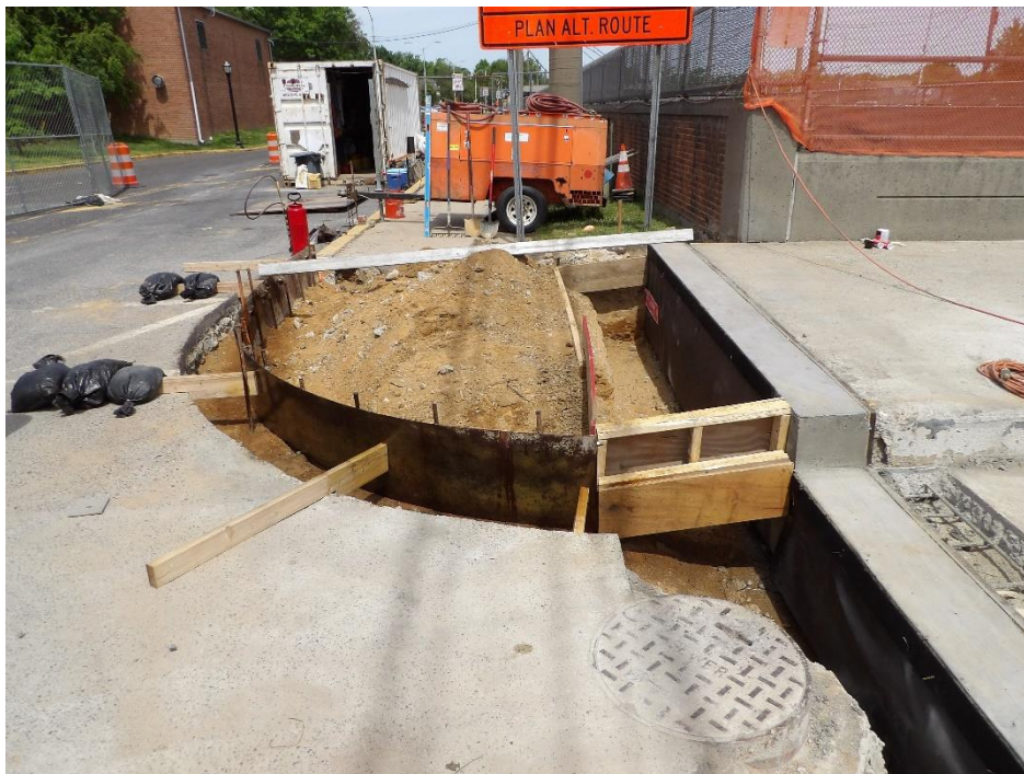
Figure 7 – Backfill bulkheads installed where required
