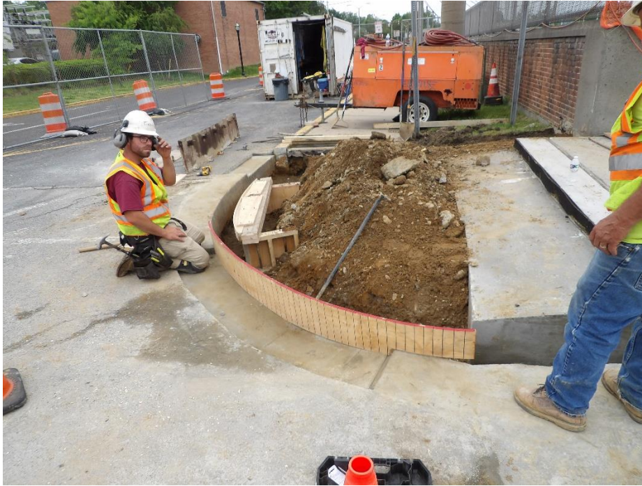
Figure 10 – Workers began forming curbs and sidewalks
