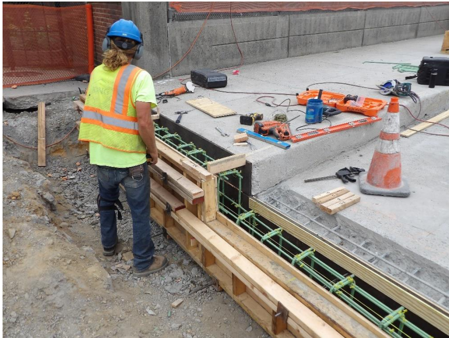
Figure 5 – Workers continued to install formwork for the new headers
