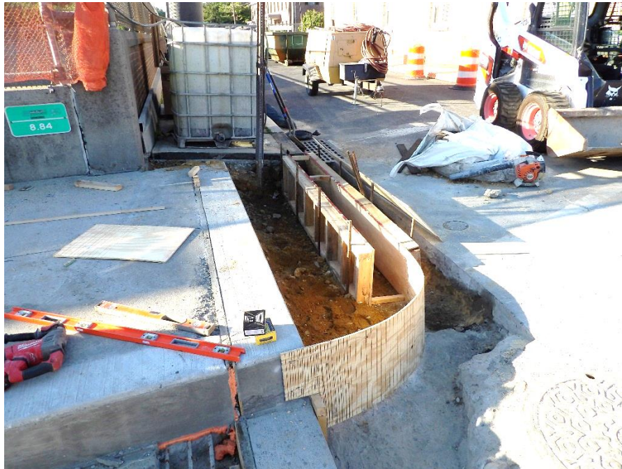
Figure 5 – Workers installed formwork for the new approach curbs
