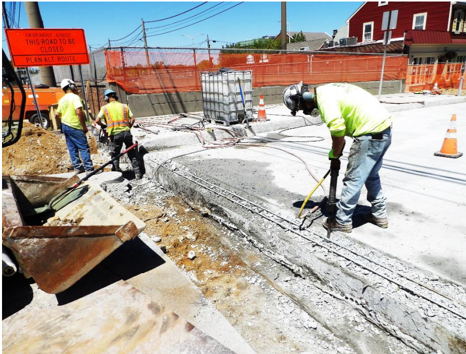
Figure 2 – Workers chipping the deck end for the PPC haunch/joint
