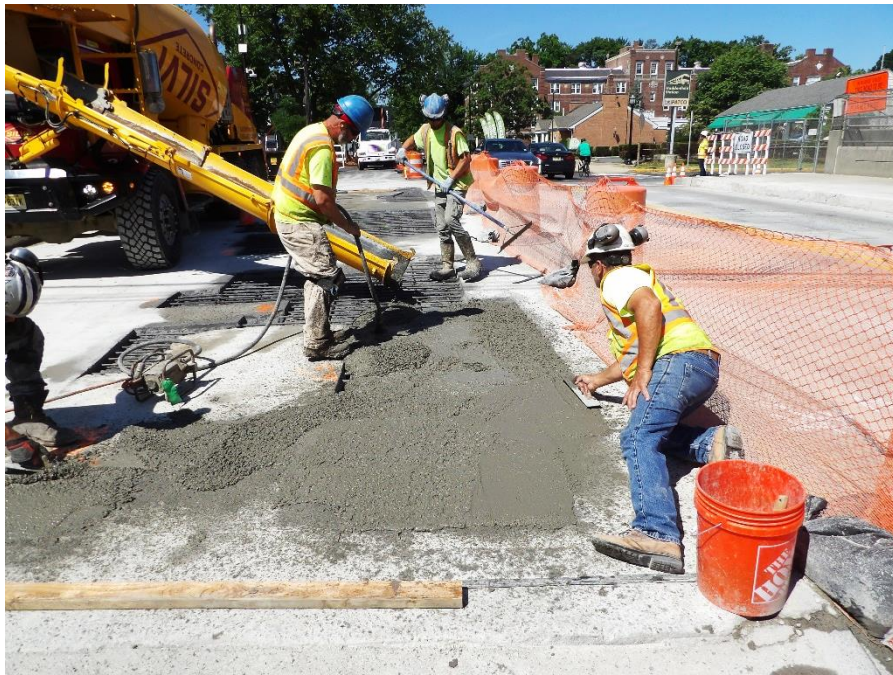
Figure 5 – Workers poured the patch concrete
