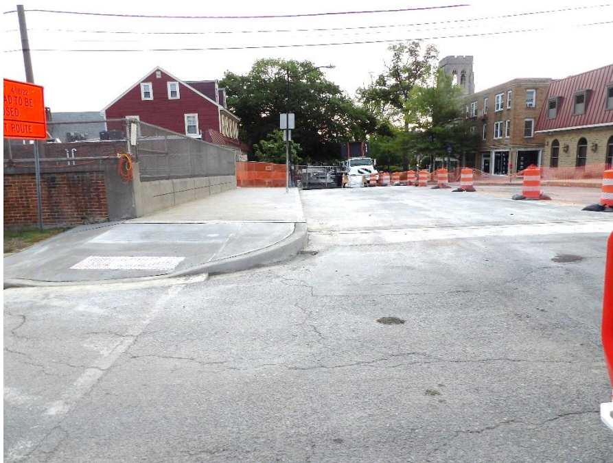
Figure 9 – Stage 1 reconstruction work has been completed
