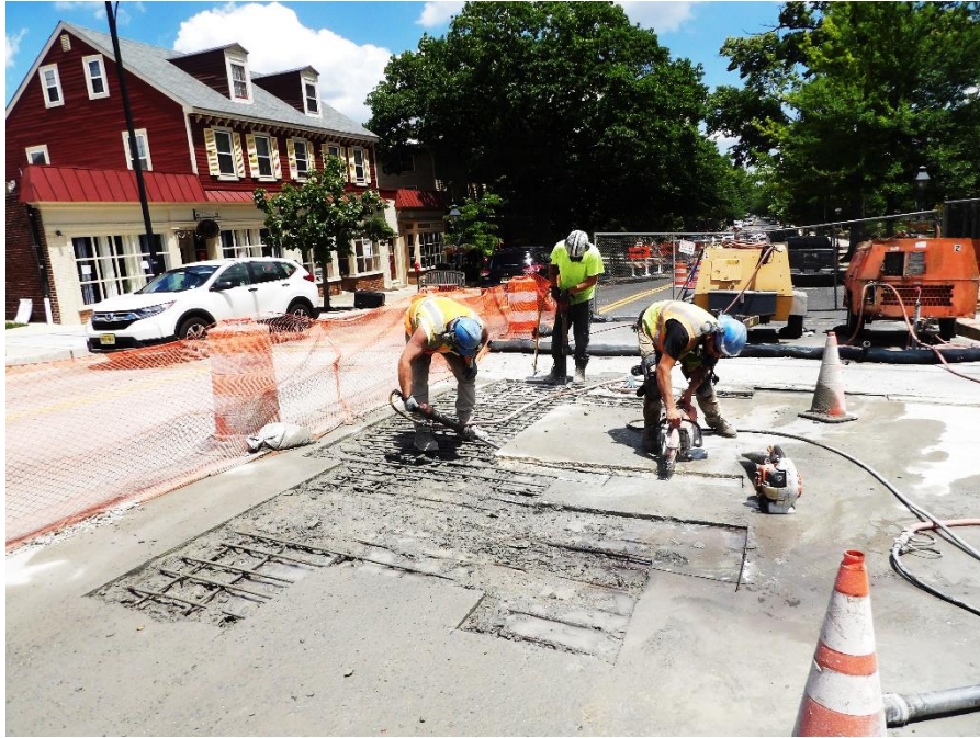
Figure 7 – Workers began removal of deteriorated deck concrete for the second pour
