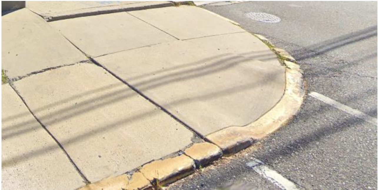
BEFORE: Handicap Ramp northeast corner
