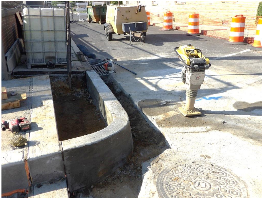
Figure 7 – New curb formwork was stripped
