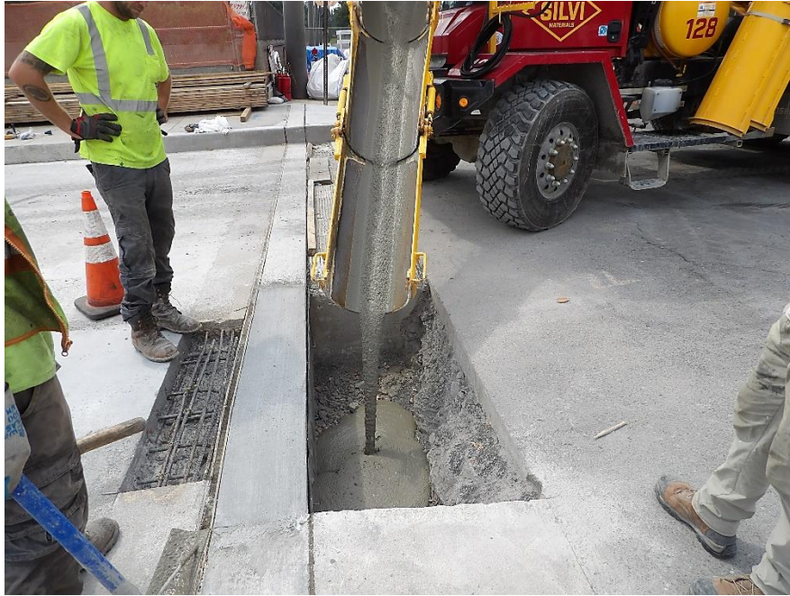
Figure 2 – Both abutments were backfilled with lightweight flowable fill
