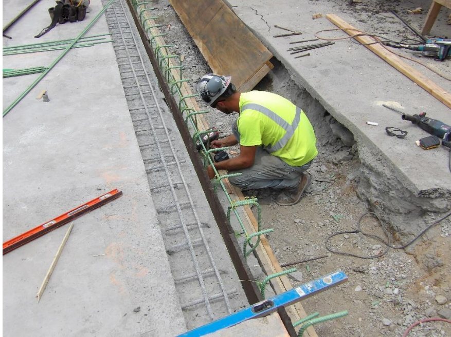
Figure 4 – New header reinforcing was installed and formwork install began
