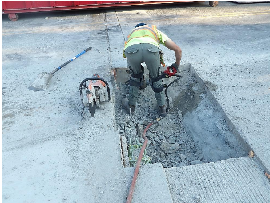
Figure 5 – Headers were chipped out and removed, Stage 3
