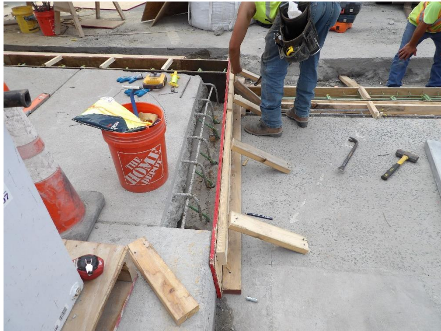
Figure 9 – Workers formed the curb repair at the southwest bridge corner
