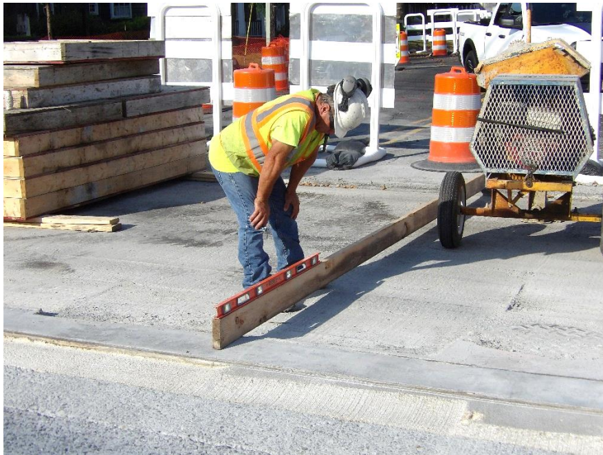
Figure 7 – Workers checking grades between the deck to approach transitions
