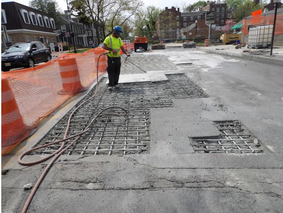
Figure 4 – Cleaning areas to be patched
