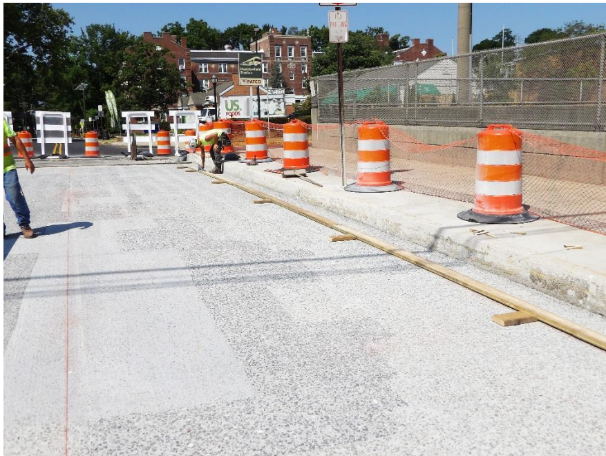
Figure 9 – Workers began lane and shoulder layout and began installing forms
