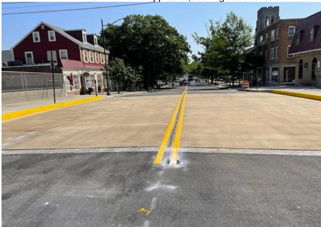
AFTER– North Approach, looking south
