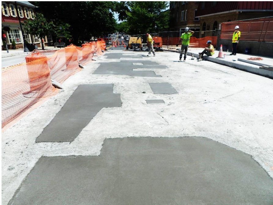
Figure 7 – Stage 2 patching was completed
