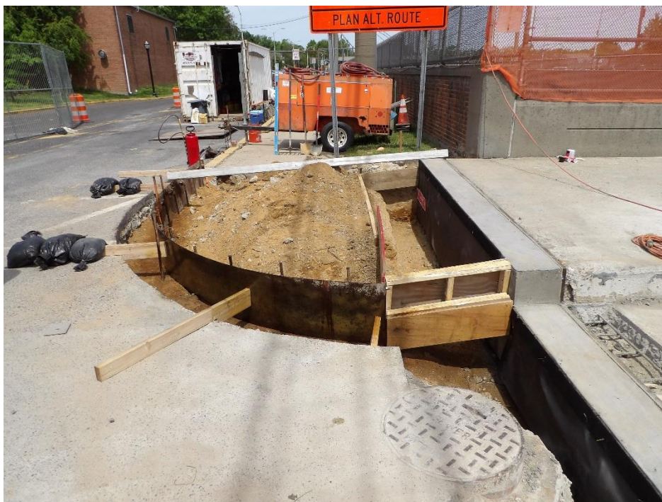
Figure 7 – Backfill bulkheads installed where required
