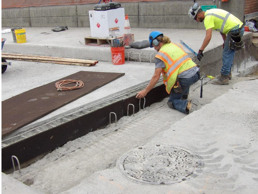
Figure 6 – Workers moved to the west header and began forming
