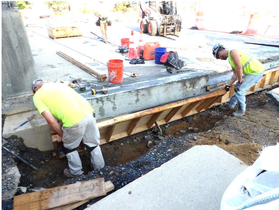
Figure 3 – Workers stripped the header forms
