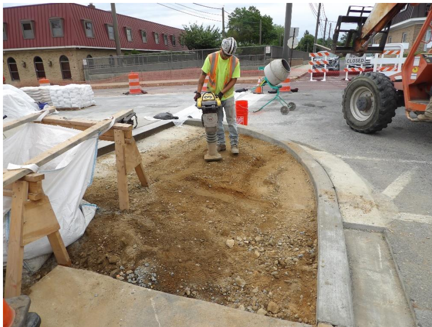
Figure 3 – Workers prepared the sub-base for sidewalk concrete pours
