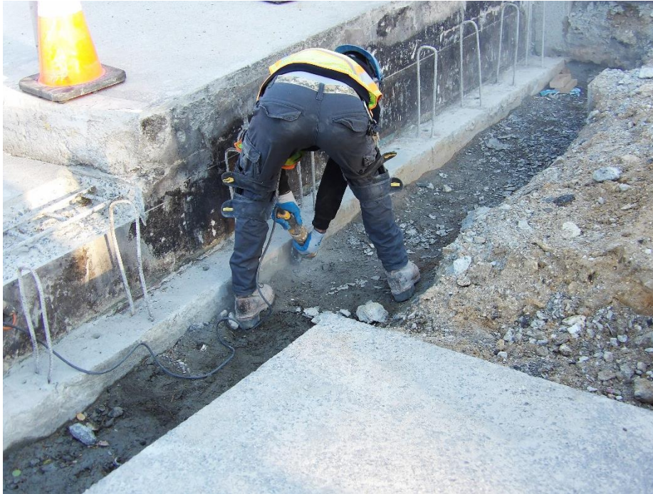
Figure 4 – Drilled holes in existing backwall for new header reinforcing
