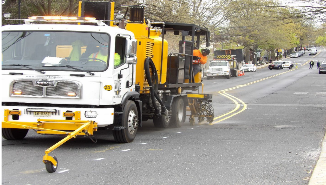
Figure 4: Stage 1 - Striping for Lane Shift .
