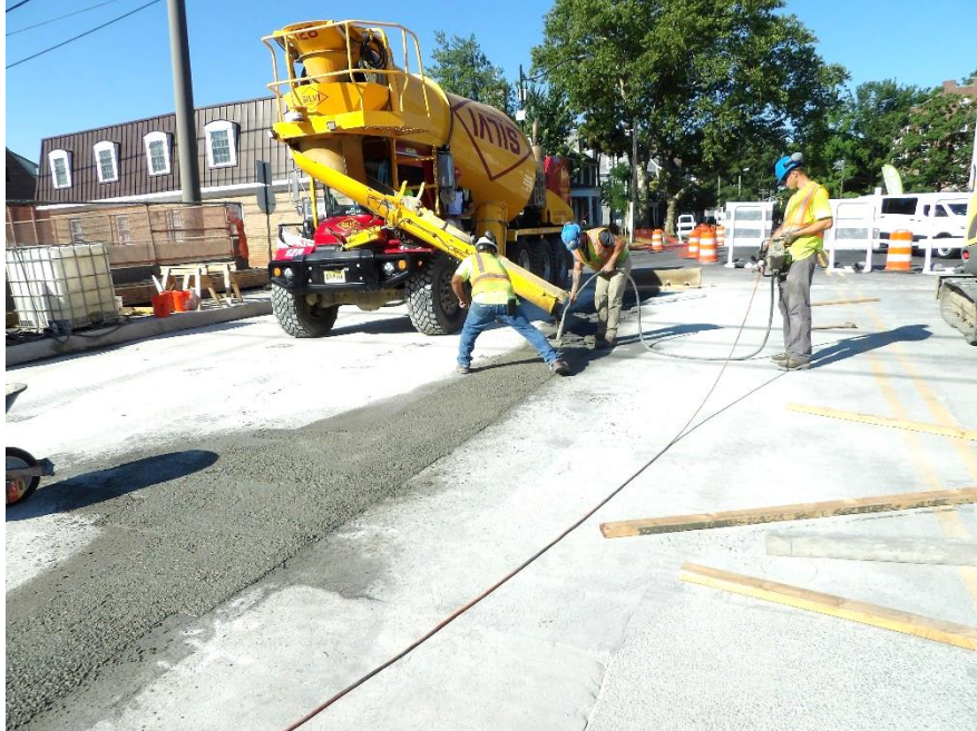
Figure 8 – Workers poured and finished the deck patches
