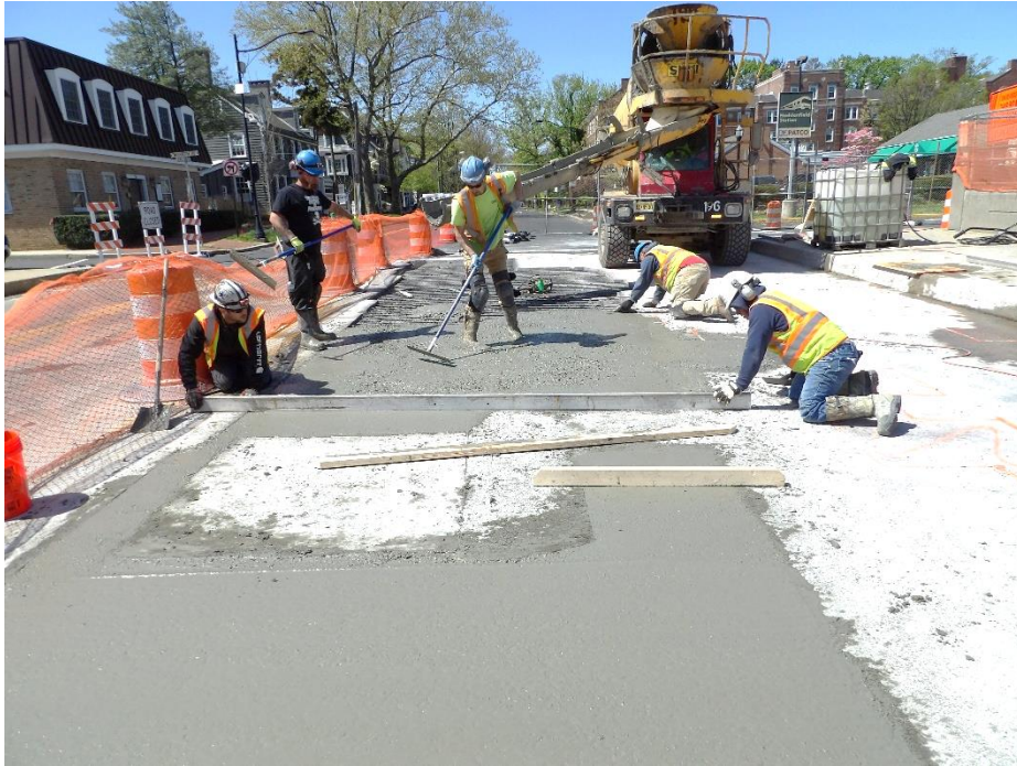
Figure 8 – Concrete was poured and finished
