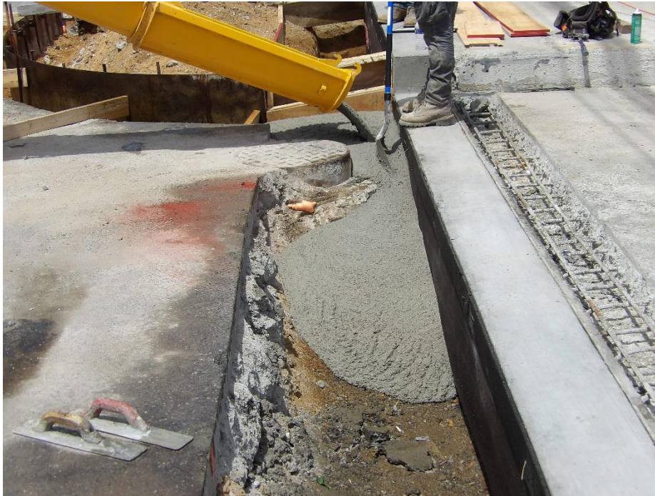
Figure 8 – Lightweight flowable backfill placed at each abutment
