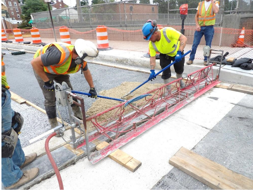
Figure 4 – Workers began placement and finishing of the PPC overlay
