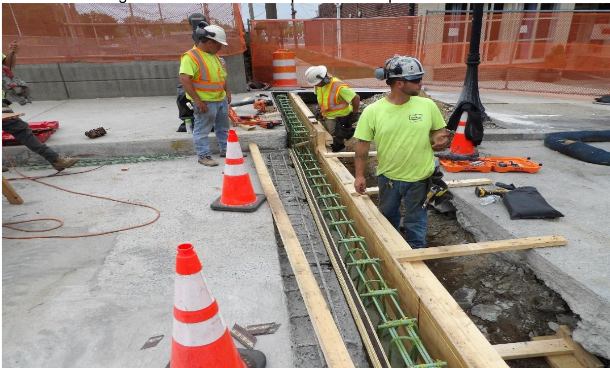
Deck Header Repair during construction
