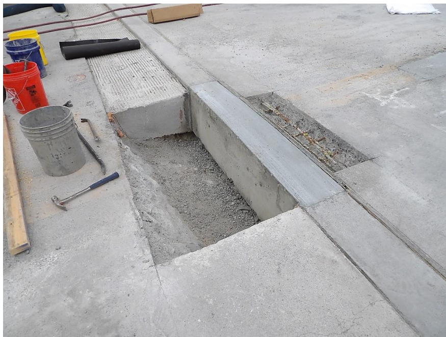
Figure 1 – Workers poured and stripped the Stage 3 headers
