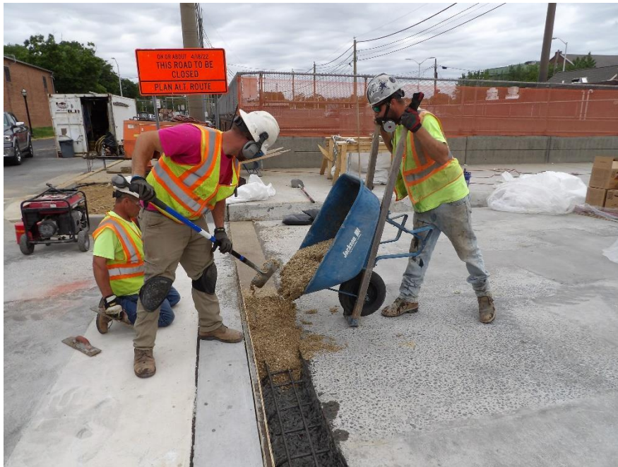
Figure 7 – Workers mixed and poured the deck joint PPC
