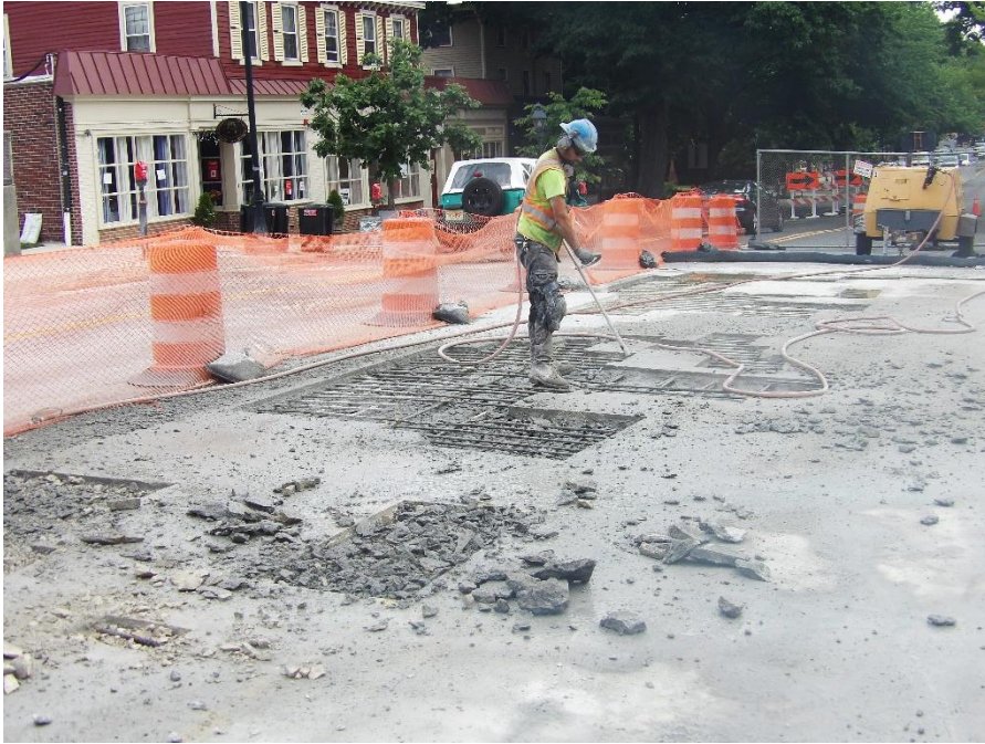
Figure 2 – Saw cutting and concrete removal progressed
