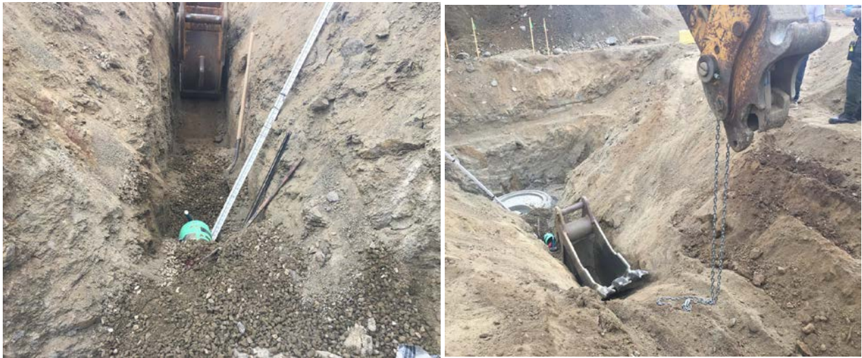
Exhibit 2 and 3. Alternate views of the trench.
