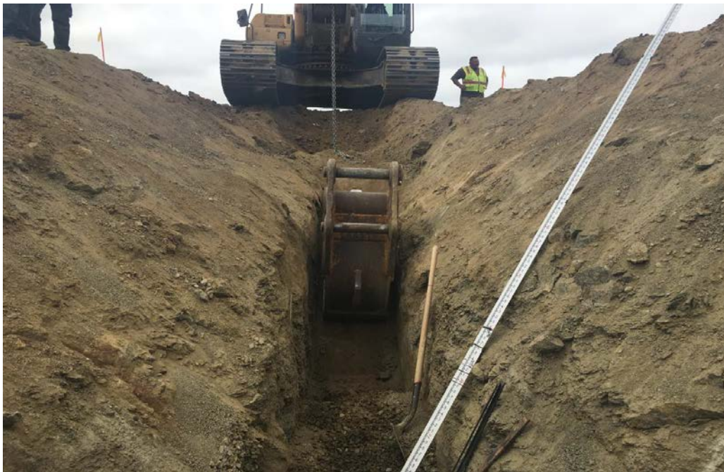
Exhibit 4. Slope and depth of the trench.
