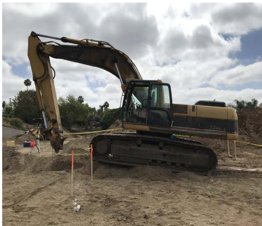
Exhibit 1. The excavator involved in this incident.
