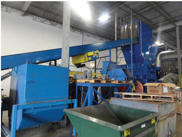
Figure 4. First tower and shredder. Photo by NIOSH.
