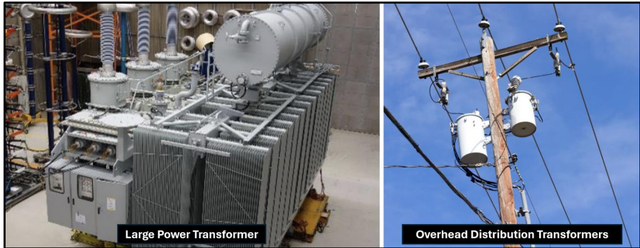
Figure 3: Large Power and Distribution Transformers 10
