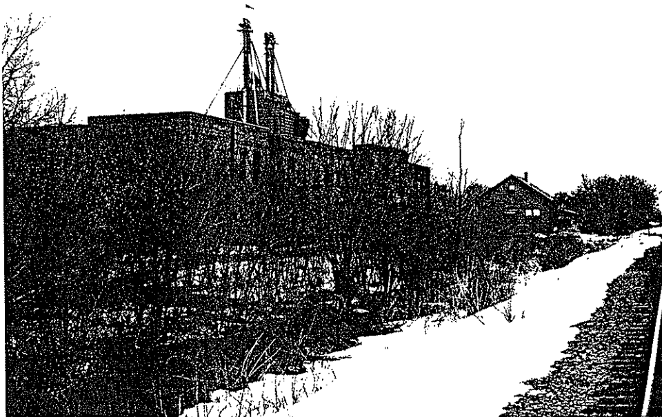
8 FEED MILL FROM WEST SIDE
