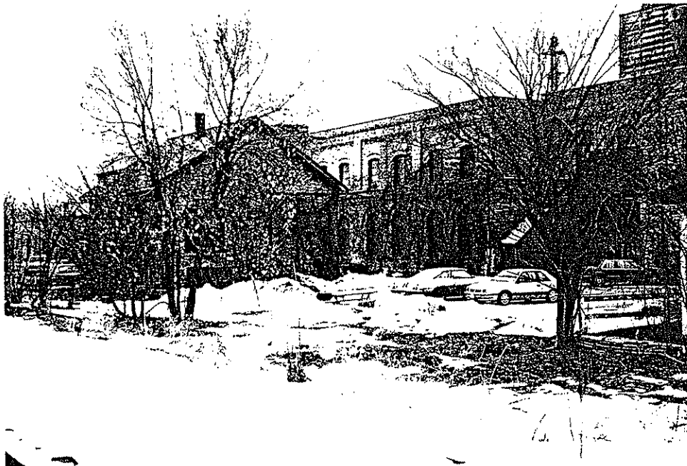
16 VIEW OF FEED MILL AND OFFICE FROM SOUTHEAST
