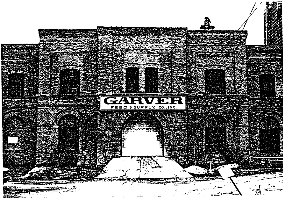
1 FRONT OF FEED MILL
