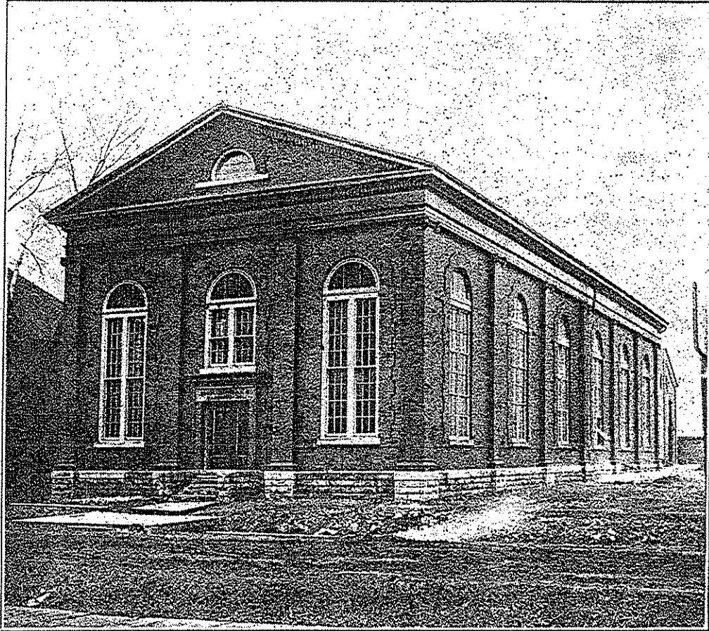
NEW POWER HOUSE, WHERE THEY "USE GAS FOR FUEL."
