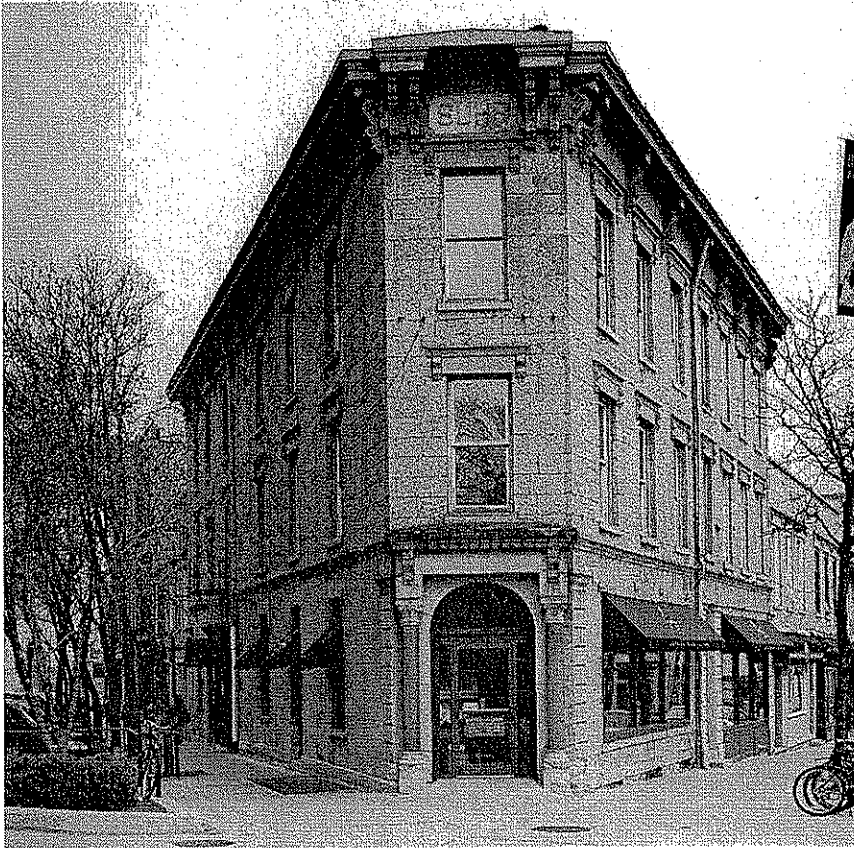
The Suhr Building 2001 (Zane Williams)
