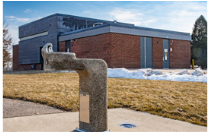
Madison Water Utility's Well 15, currently out of service
