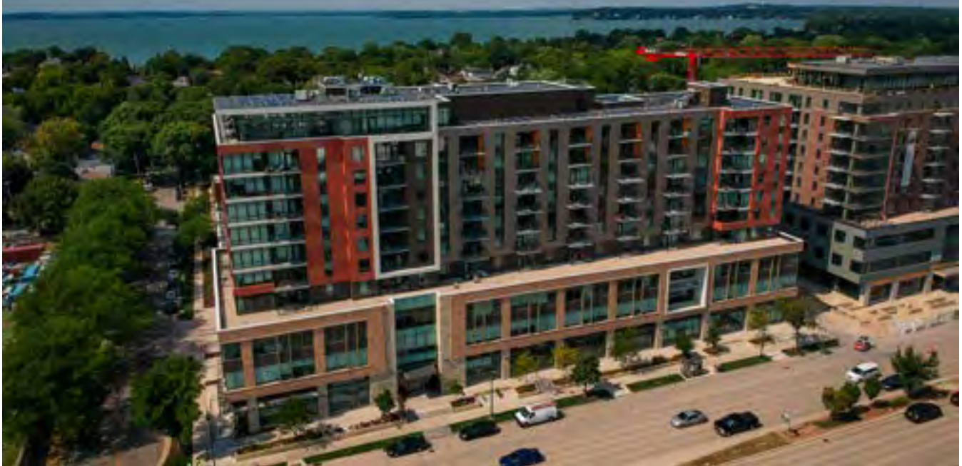
PHOTOS COURTESY OF STEVENS CONSTRUCTION
