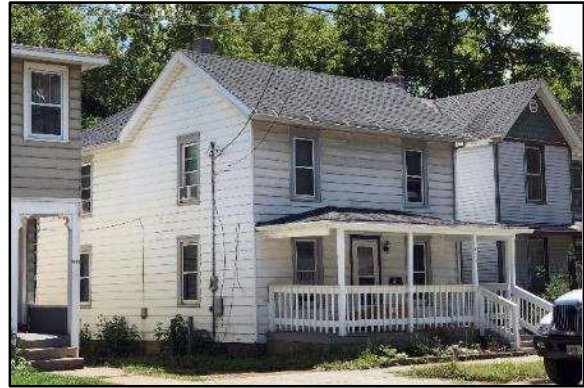
Benjamin and Amy Butts House 633 E. Johnson Street
