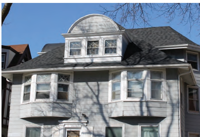
IMAGE 44: Bays, dormers, and other volumetric window articulation present on 248 Langdon Street is common throughout the district.
