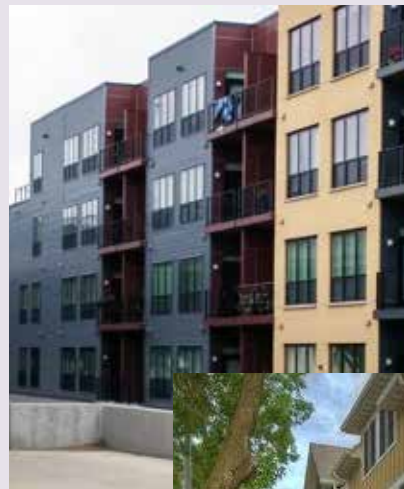
Stacked and Inset Balconies in Milwaukee
