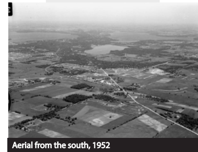
Aerial from the south, 1952
