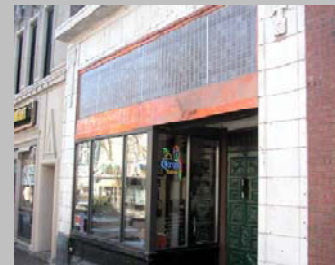
The facade of the Irish Pub after the exterior renovation, with the historically significant prism glass exposed.
