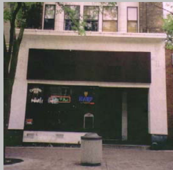
The facade of the Irish Pub prior to the exterior renovation
