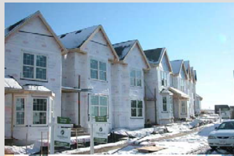
Townhouses in Grandview Commons during construction
