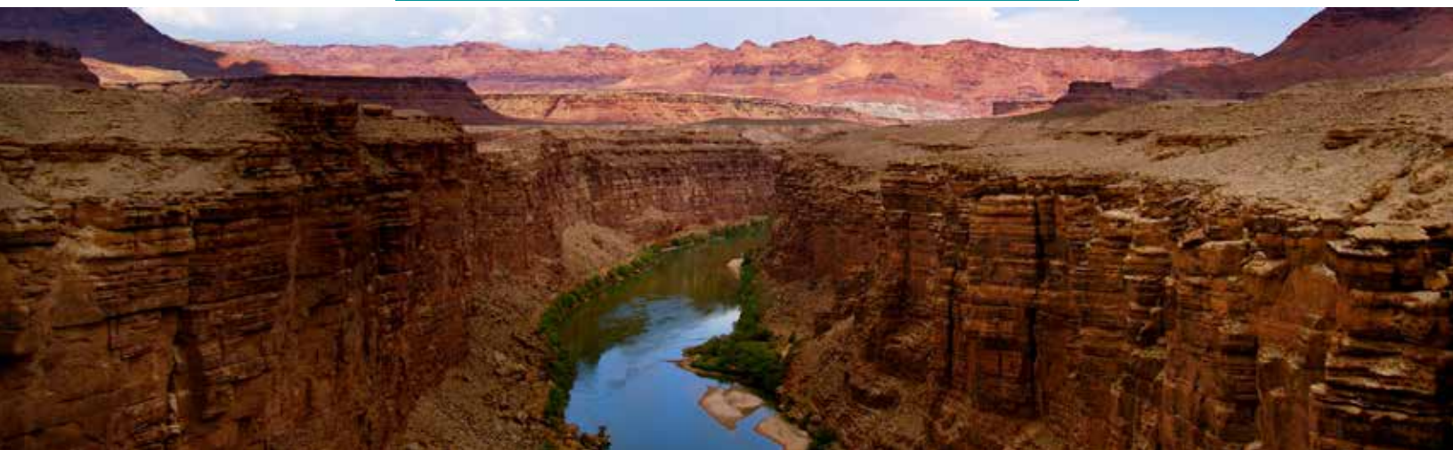
Marble Canyon on the Navajo Bridge. Photo: Creative Commons, Paul Falardeau.
