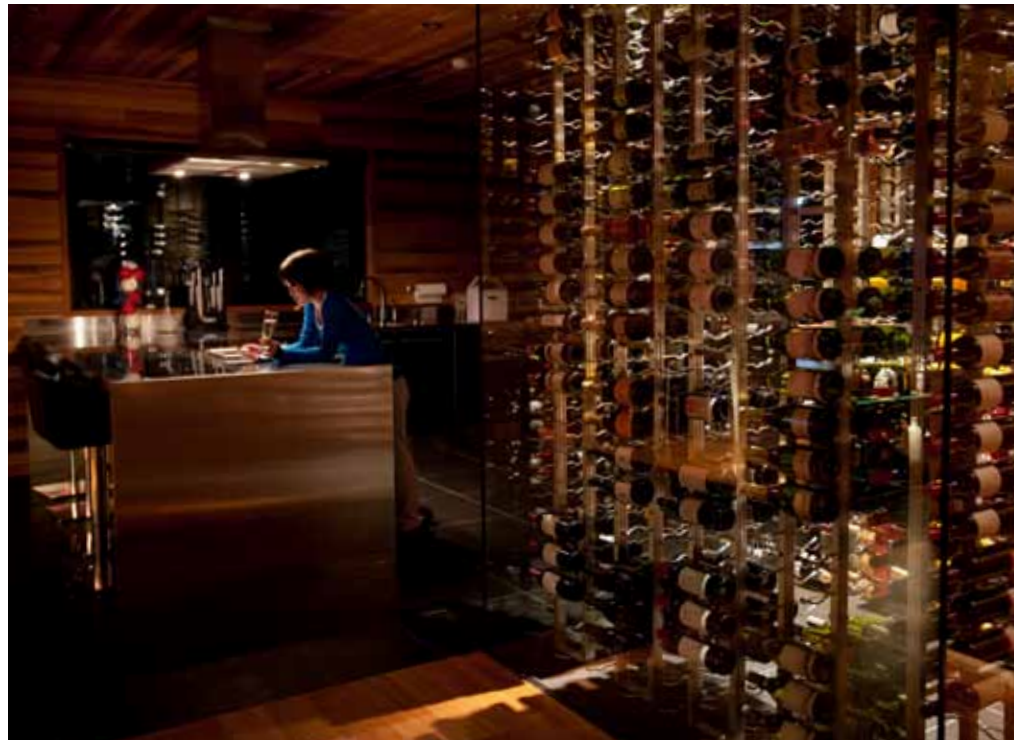
The expansive wine room, including multiple bottles of Dom Perignon, is climate controlled by the programmed shades, which open and close accordingly—and automatically—all year long.
