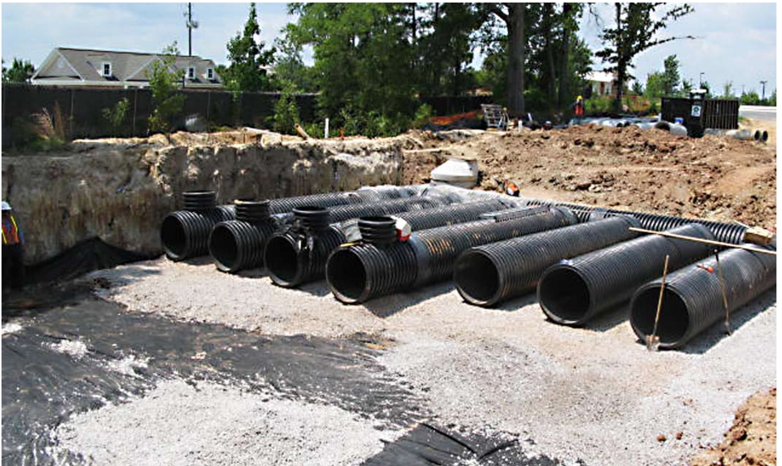
CPP factory fabricated fittings and manifolds allows for easy site assembly of CPP Stormwater Detention/Retention Systems
