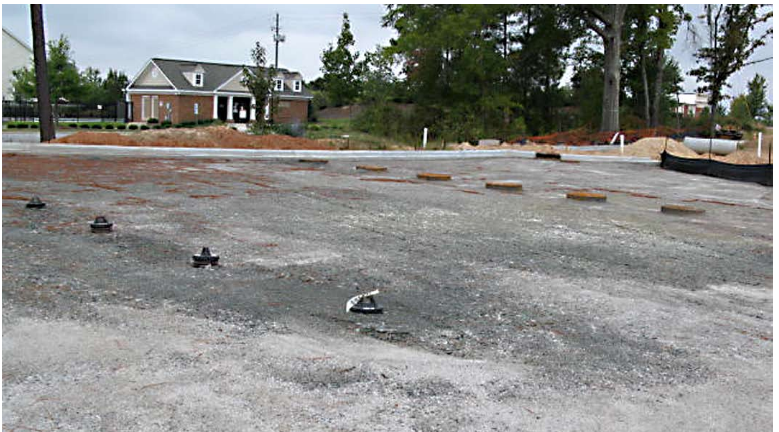
Compacted cover and ready for paving photos show Manhole Covers for inspection access and easy post construction maintenance
