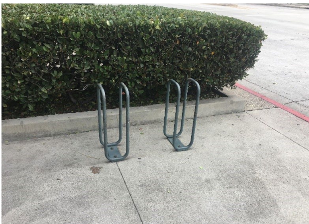
Some bike racks in Downtown Culver City do not provide two points of contact
