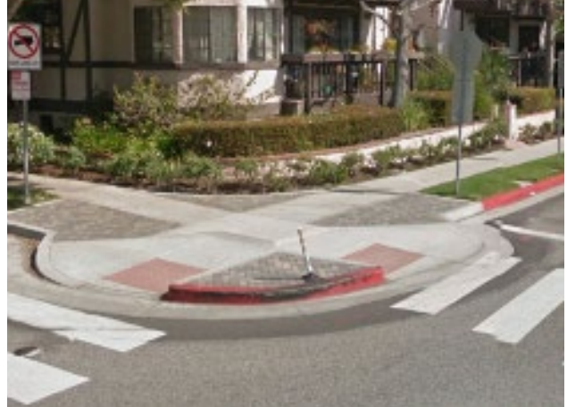
Recommended: Bulb-Out with bidirectional curb ramps for crossing in both directions at Duquesne Avenue and Lucerne Avenue. Source: Google Streetview
