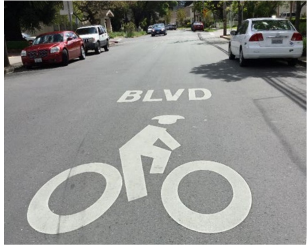
An example of an large pavement marking to reinforce that the street is a Bike Boulevard or Bicycle Boulevard.
