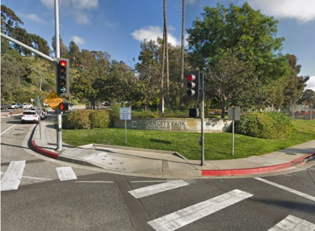
Not recommended: diagonal curb ramp configuration at Jefferson Boulevard and Duquesne Avenue. Source: Google Streetview
