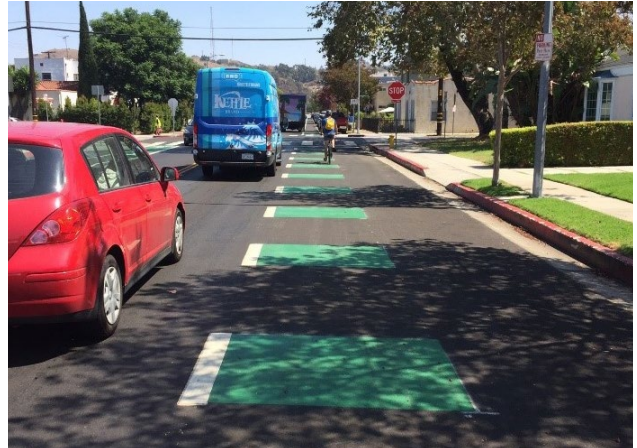
Green conflict striping in a Class II bike lane on Duquesne Avenue, Culver City
