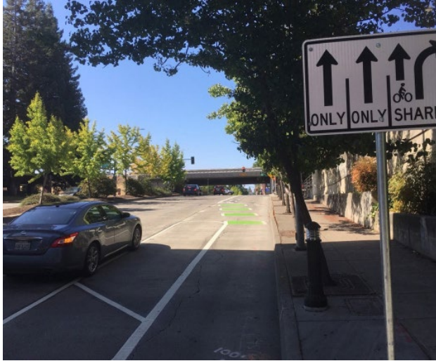
Buffered bike lanes transition into conflict markings.
