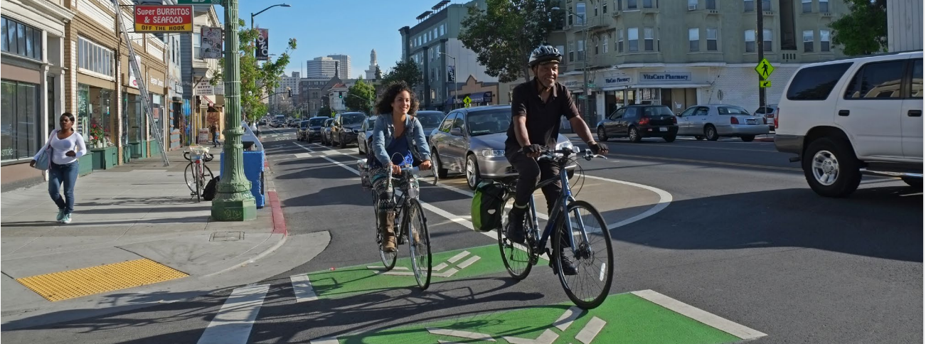
Parked cars serve as a barrier between bicyclists and the vehicle lane. Barriers could also include flexible posts, bollards, planters, or other design elements Source: Bike East Bay.
