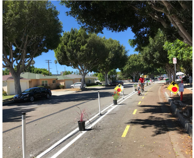
A family rides along a demonstration of a Class IV bikeway on Elenda Street
