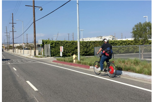
Standard Class II Bike Lane on Jefferson Boulevard
