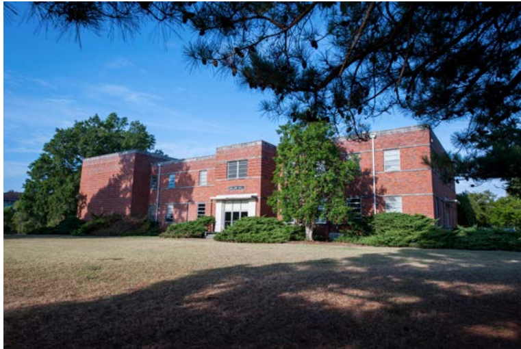
Ballew Hall renovations include a flexible teaching lab, development suite, conference room, recruiter suite, auditorium, and administrative spaces. (Photo by Russ Houston)
