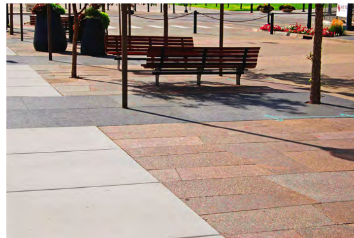
Sidewalk paving: composite of cast in place concrete strip next to the building with two colors of granite paving filling out the remaining sidewalk area. Primary granite is Carnelian in warm pink with Mesabi Black as accent rectangles around tree wells; tactile paving at corners is to be determined.
