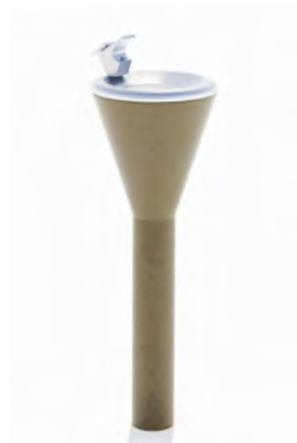
Drinking fountain: repair and renovate original; repaint in original grey color.
