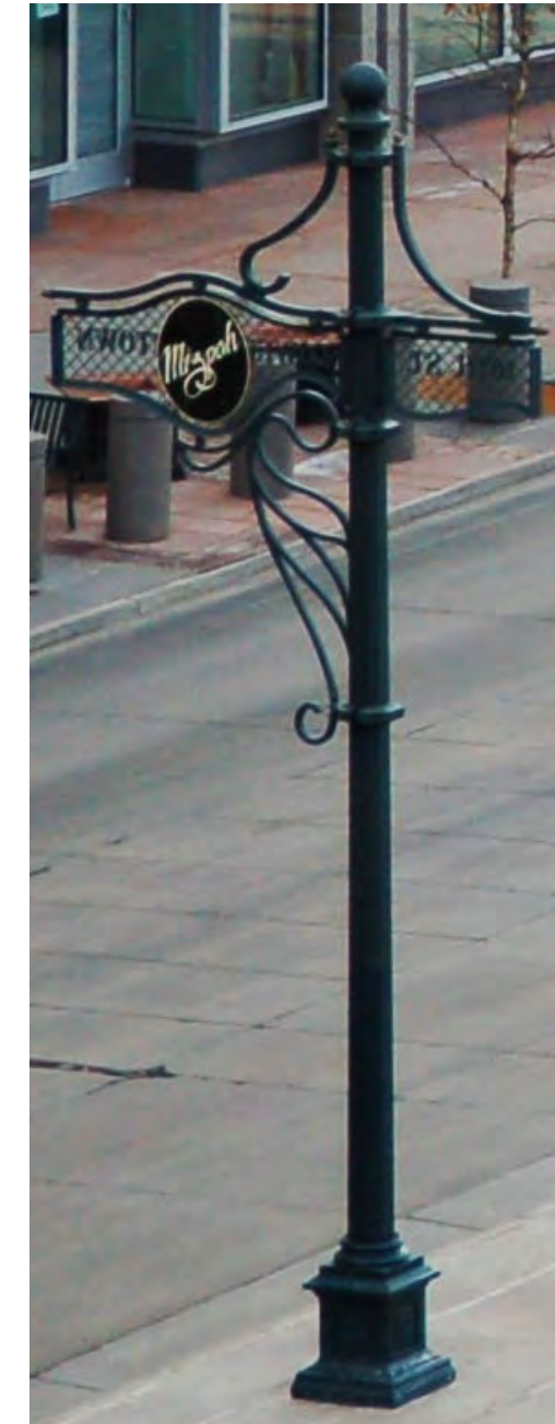
Lower downtown gateway marker: renovate; repaint in Federal Green color.
