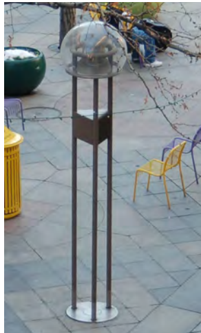
Pedestrian lights: a critical iconic component of the original design elements family; unique effect with median placement; high maintenance cost; position, height and current function don't achieve good lighting performance; several missing due to collisions.
