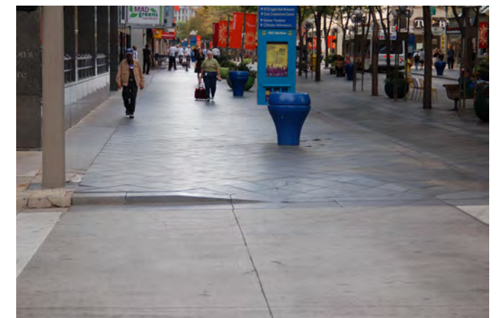
Mall curb ramps will be widened to the full walkway width
