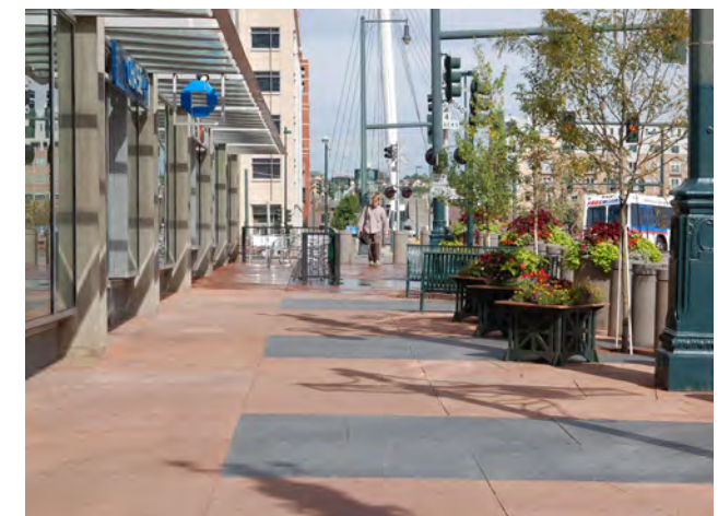
Sidewalk paving: replace original mortar-set sandstone paving with new aggregate-set, larger sandstone and granite paving to match blocks already renovated (Sugar Cube, 1600 Market, EPA blocks); Colorado Red Sandstone and Mesabi Black Granite; provide continuous tactile paving at all-flush corners; use 4" x 8" module pavers in Sierra White granite option or Hanover White Precast pavers in straight and custom-radiused pieces; mortar-set on existing or new subslab.
