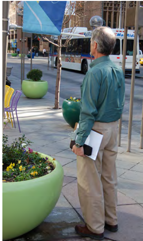
Lower banner pole stays need to be shortened to meet ADA clearance requirements at eye level; they protrude beyond the planter sides
