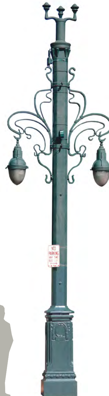
Street light/historic replica: renovate; consider re-lamping for enhanced lighting and energy performance; repaint in Federal Green color. Exception: remove existing fixtures at EPA block; re-use these at Market Street Station block. EPA block to be retrofitted with new DUS district lights.
