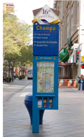
Way-finding signage: second generation, not part of original design elements; they provide a critical service for visitors and mark the shuttle stops; expensive to fabricate and maintain; some problem with water leaks, fogged glass and corroded electrical connections; appearance is questionable with original Mall furnishings.
