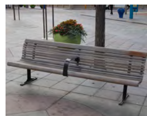
Bench: a replacement of the original benches; lack of center leg and frame has led to several being broken by vandalism.
