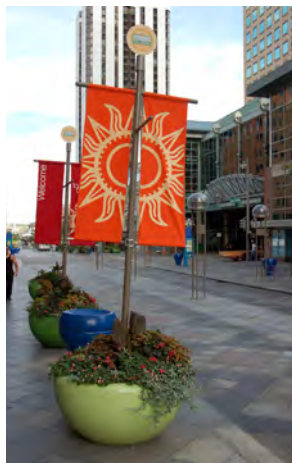
Planter/banner poles: custom-made; part of the original design elements family; relative light weight is an advantage for periodic moving for special events; fiberglass is repairable locally; original color – grey; banner pole bottom isn't secure so poles lean.
