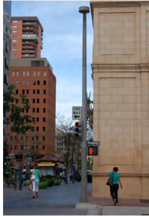
Corner street lights: part of the original custom design elements family; lighting and energy performance could be improved; countdown and audible pedestrian signals would be an improvement.
