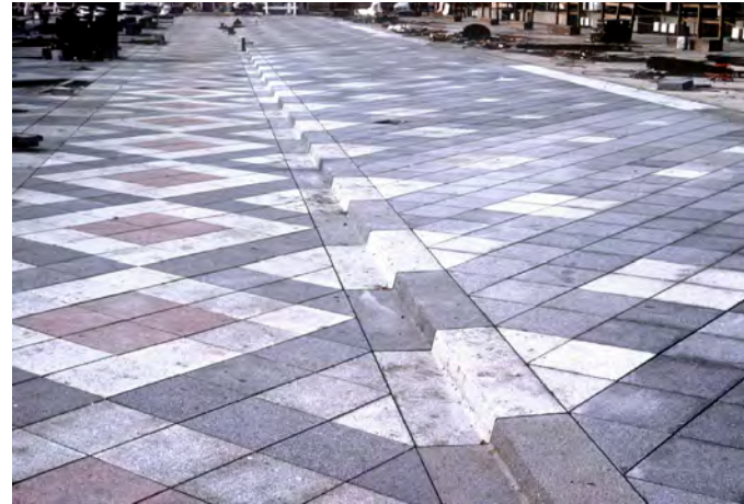
The original 3-color granite paving during installation
