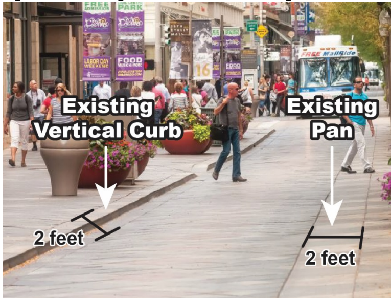
Figure 2-3. Existing Vertical Curb and Existing Pan on Median Block
