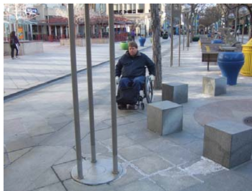
Less than 3' clear at median fountain 5
