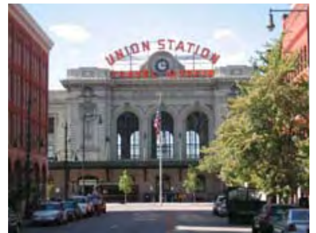
Denver Union Station and Civic Center Station will work in concert as hubs of regional and local transit.
