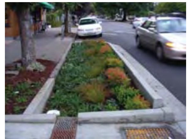
Portland, Oregon has made great strides in incorporating green street elements that naturally channel and filter stormwater into its streetscape designs.
