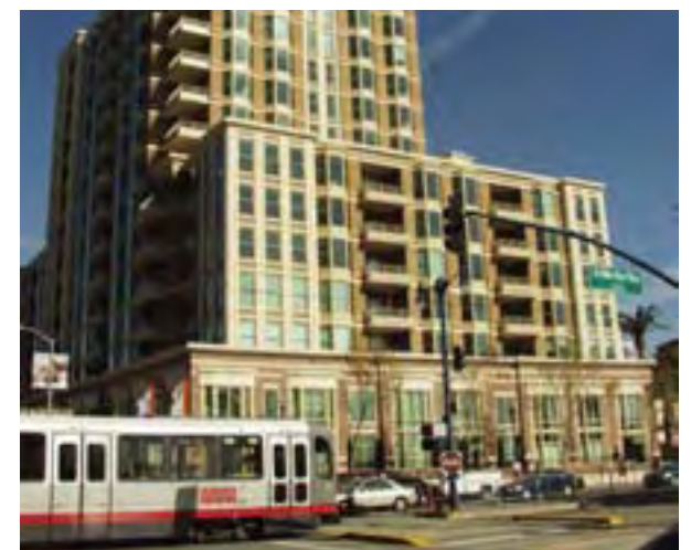
Strengthening transit will increase opportunities for transit-oriented development, such as this mixed-use housing project in San Francisco, CA.
