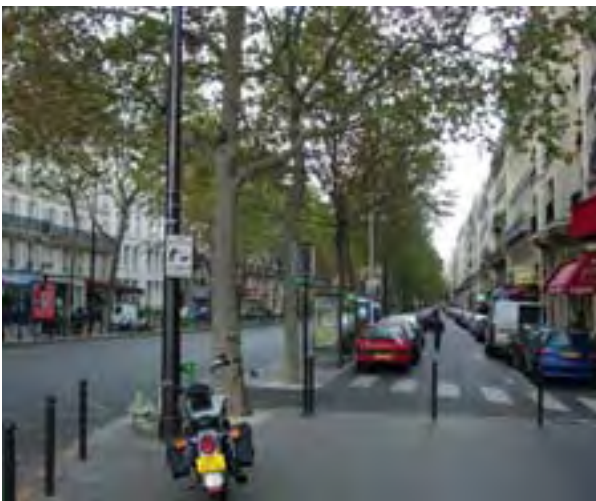
This boulevard in Paris, France allows through-traffic to travel down the center while local traffic travels down slower side access lanes.
