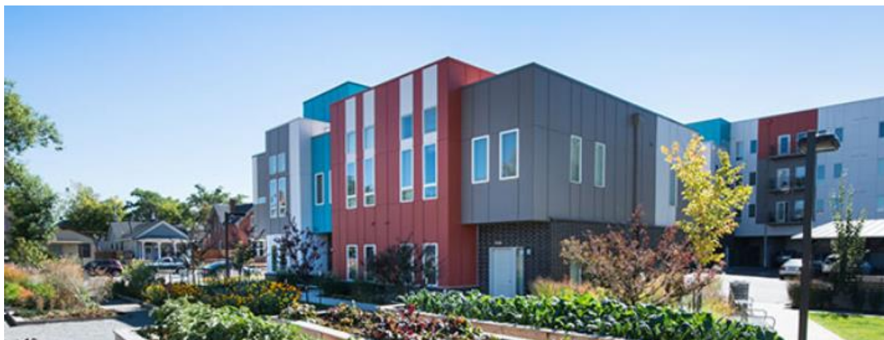
The Zephyr Building which is a part of the 700 mixed-income units and community space in the Mariposa Development
