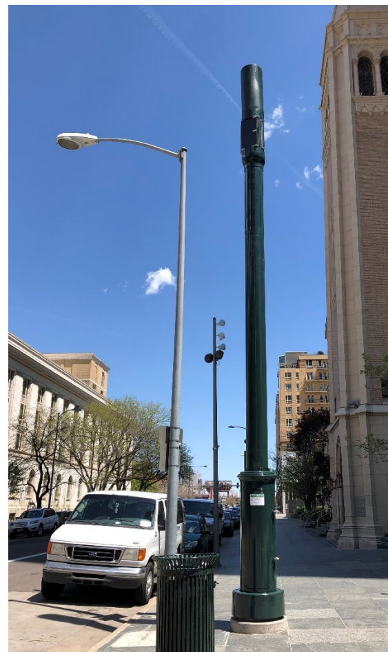
Figure 2-1: General Small Cell Pole
