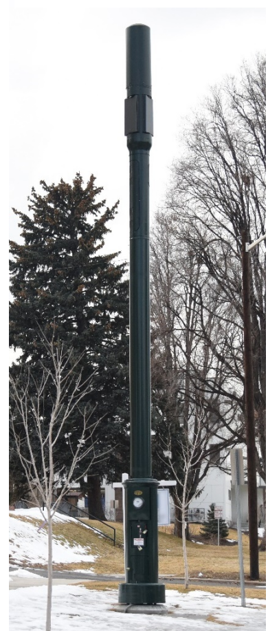
Figure 6-1: Type 4 Freestanding Small Cell Pole
