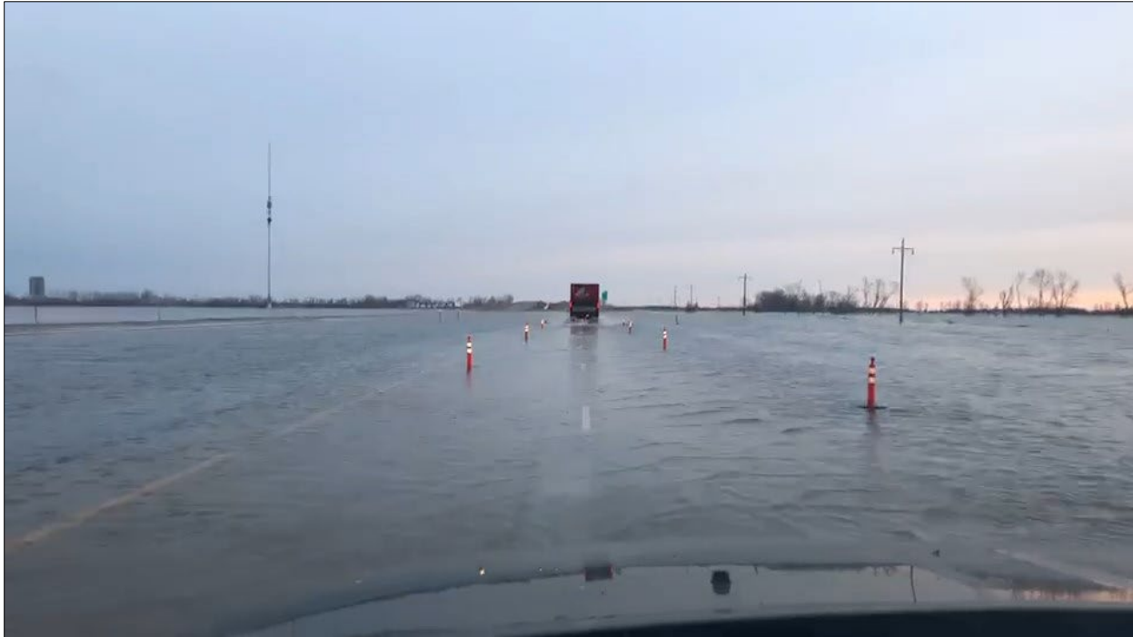
Figure 4.1-36: Interstate 29 near MP160, Inundated by Floodwaters.
