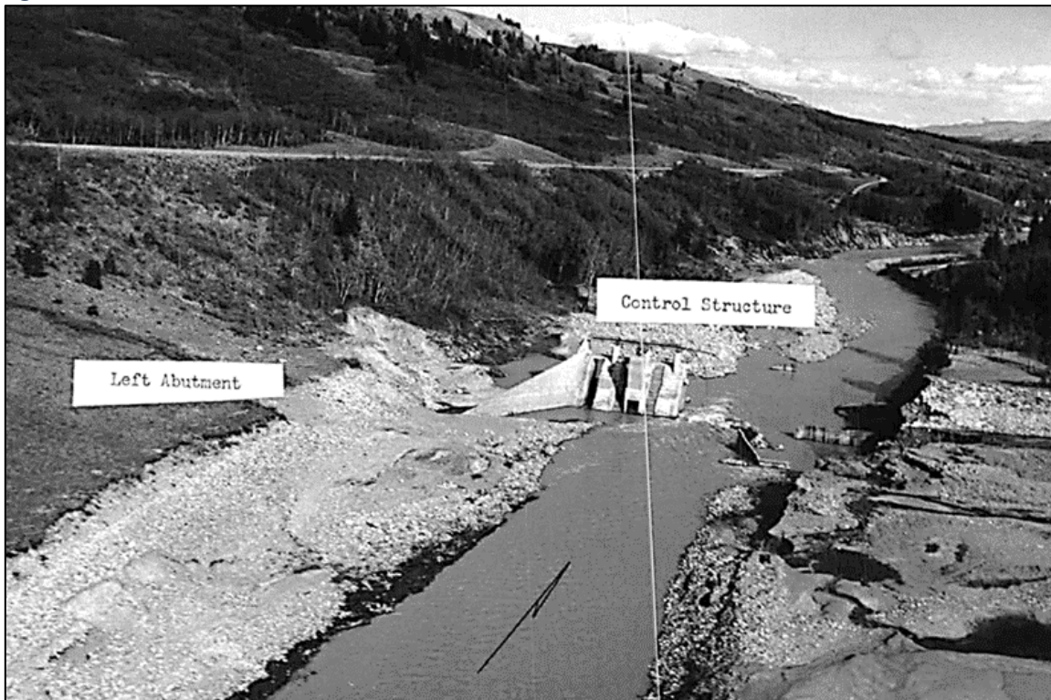
Figure 4.8-15: Two Medicine Dam after failure, Montana, 1964
