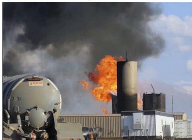
Figure 4.6-58: Saltwater Disposal Site Fire near Alexander
