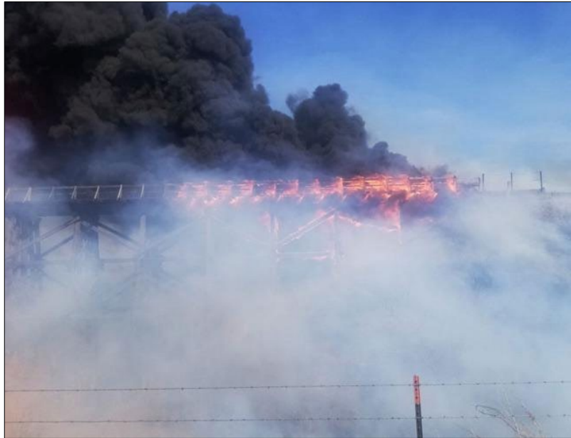
Figure 4.2-19: Destroyed Railroad Trestle Due to Wildfire
