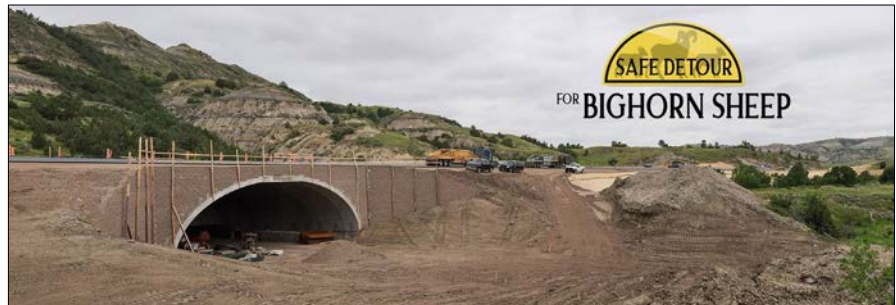
Figure 4.15-48: Wildlife Crossing on Highway 85 near Watford City
