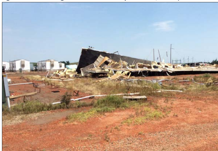
Figure 4.6-5: Damage from Watford City Tornado, 10 July 2018
