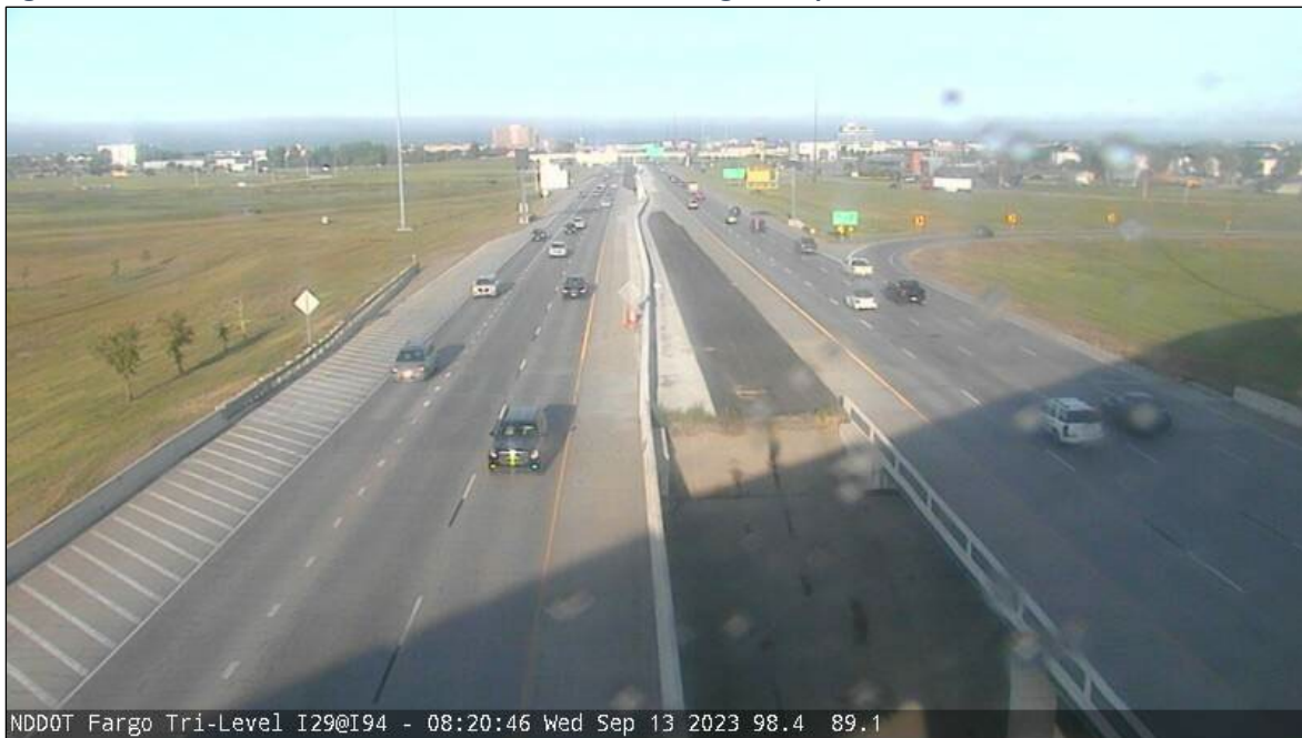
Figure 4.15-33: Traffic Camera Photo at I-29 and I-94 in Fargo in September 2023
