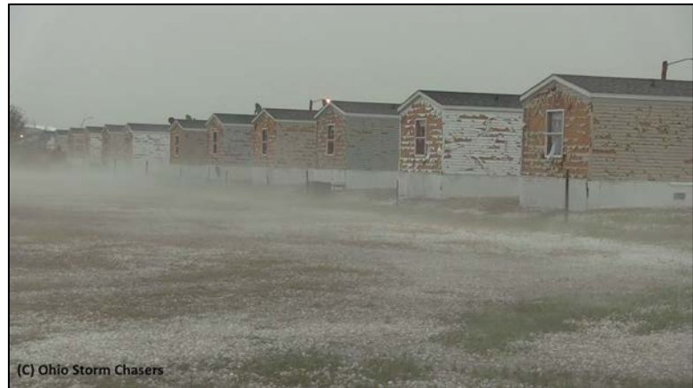
Figure 4.6-51: Hail damage in Killdeer, 10 July 2016.
