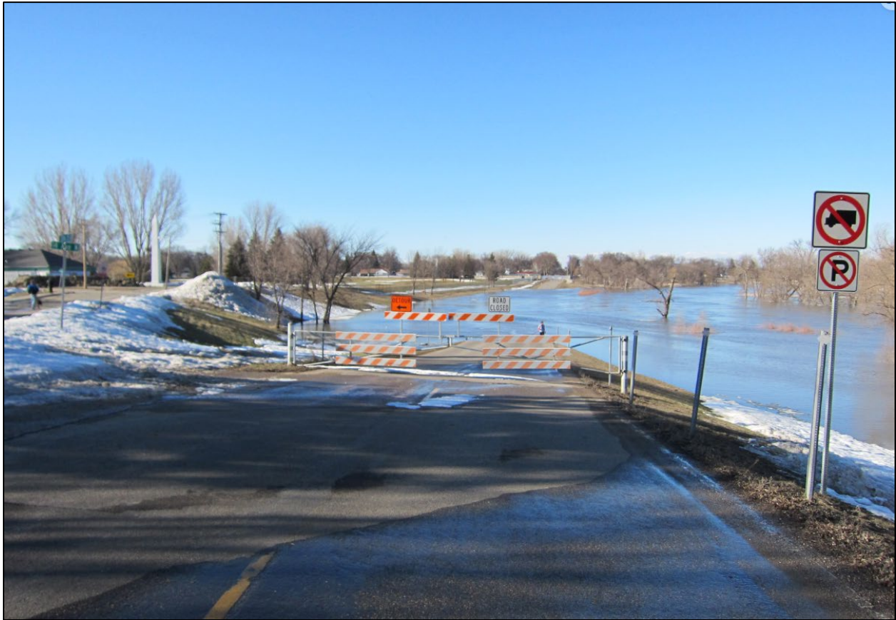
Figure 4.1-35: Elm Street in Fargo closed due to flooding.
