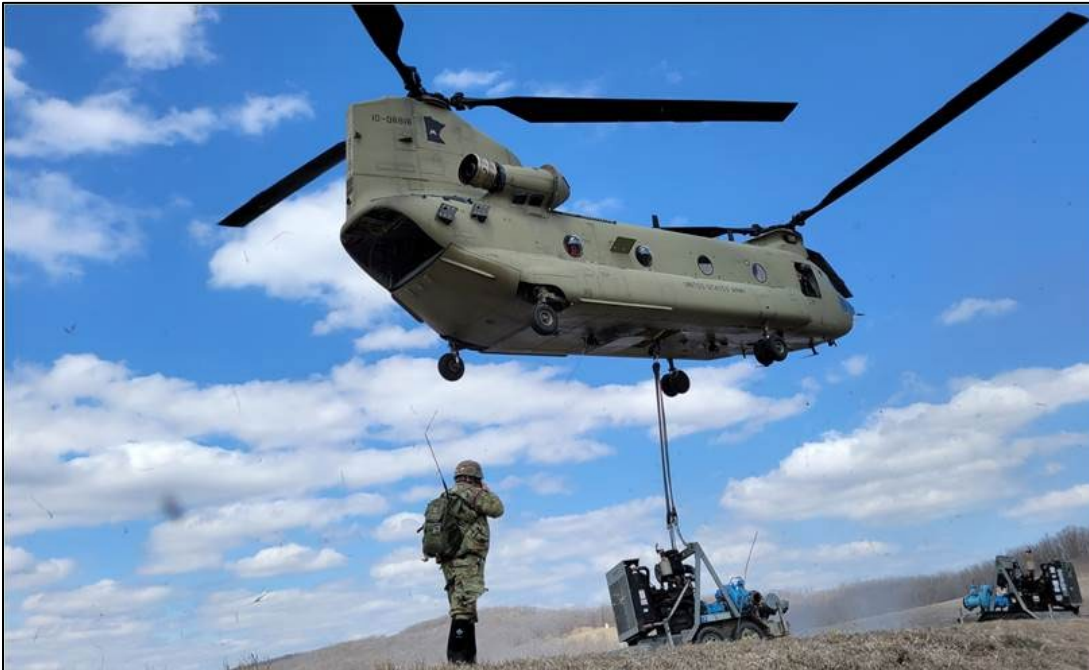
Figure 4.8-1: Chinook helicopter moving 5-ton pumps into place at Bourbanis Dam, 2022
