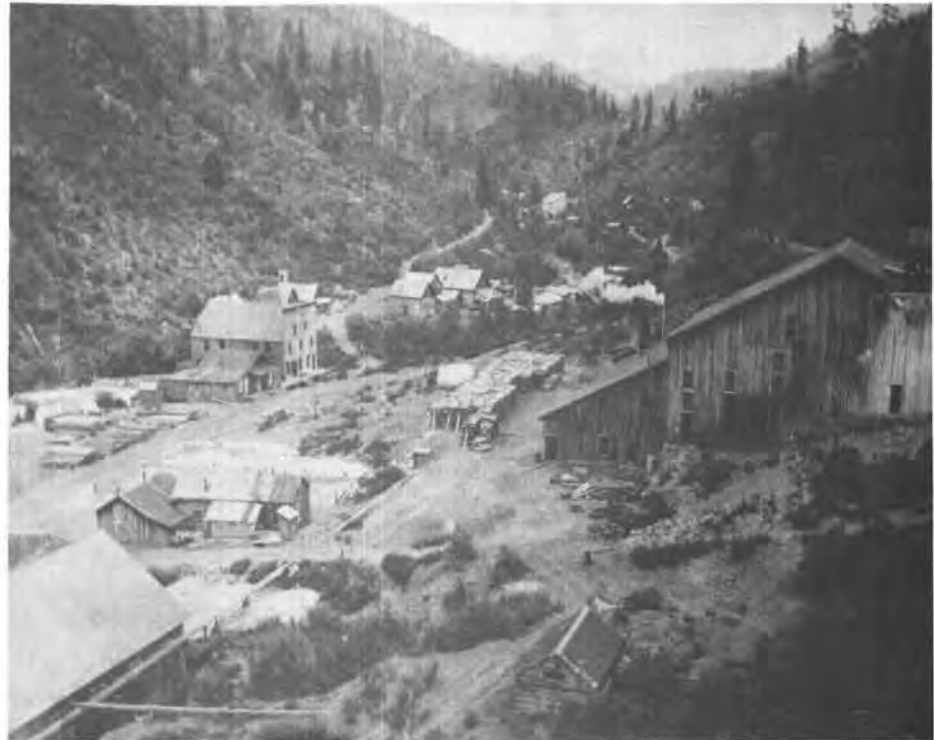
Blewett gold camp, Chelan County, in 1900. Gold mill on right treated most of the gold ore from mines in Culver Gulch. All that remains of the camp is the mill foundation as State Highway 97 passes directly through the old camp.
