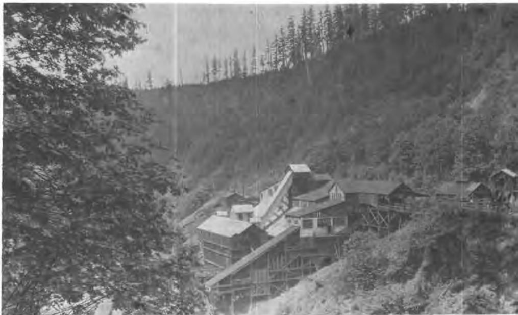
Pacific Coal Co. at Carbonado, Pierce County, in 1918. Tipple and washing plant shown in photo was near portal of mine.
