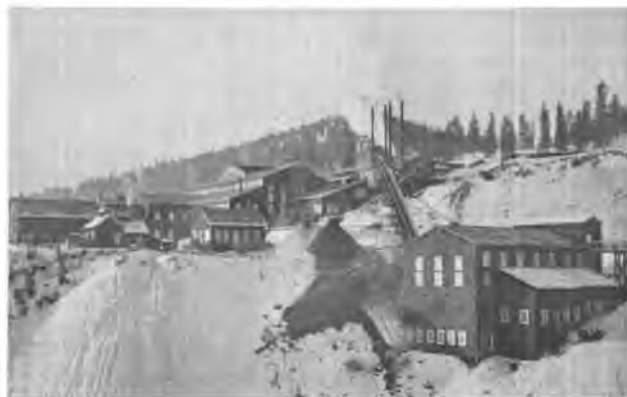
Republic mill at Republic, Ferry County, in 1900, was one of the largest gold mills in the state at the turn of the century. The 200-ton-per-day mill used roasting and cyaniding to recover gold and silver from siliceous ores of the Republic district.
