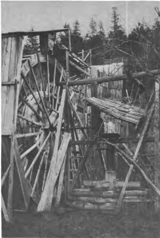
In several gold districts around 1890, arrastres were used to grind vein quartz to liberate the native gold, but because of their low capacity and poor gold recovery they were soon replaced by the more efficient stamp mill. Arrastre shown in photo was on Swauk Creek, Kittitas County, in 1924, and was powered by an overshot water wheel.
