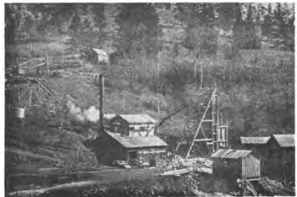
Last Chance gold mine, Republic district, Ferry County, in 1900, was typical of the many small gold mines in gold districts of northeastern Washington.
