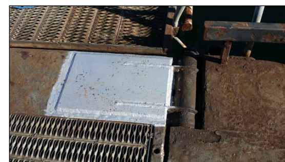
PHOTO 9 EXTERIOR WALKWAY HINGE CONNECTION
