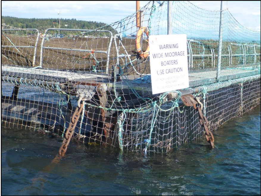
Photograph 8 : View of the Typical Steel Plate Condition.
