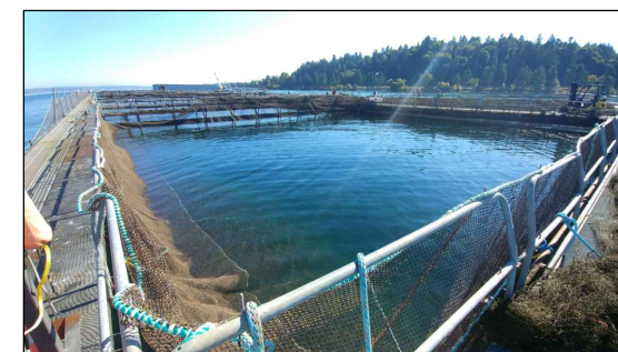
PHOTO 4 NET PEN DURING NET INSTALLATION
