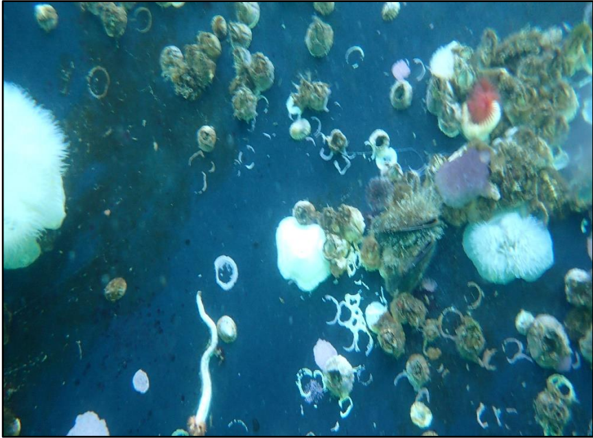
Photograph 3 : Underwater View of the Typical Marine Growth and Coating on the Pontoons.
