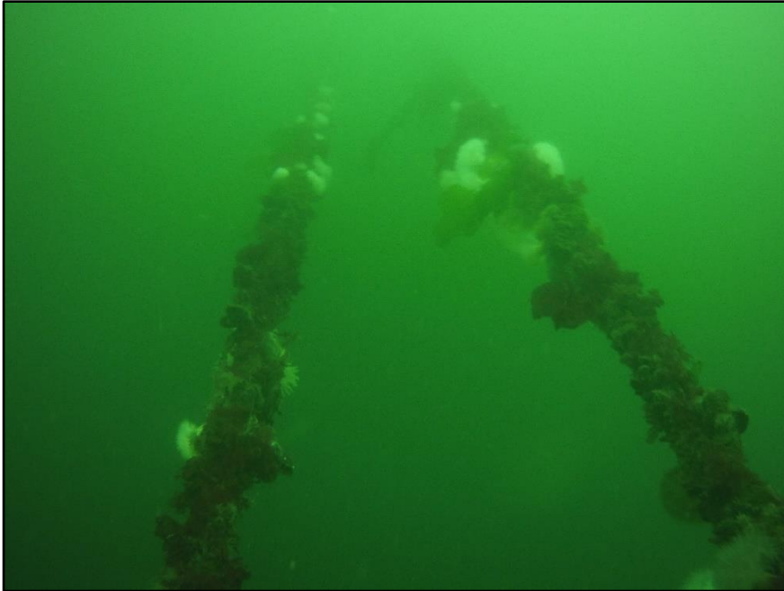
Photograph 13 : Underwater View of the Typical Rode Line Condition.
