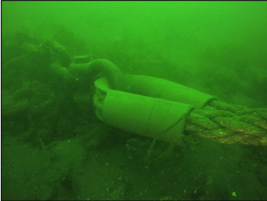
Photograph 17 : Underwater View of the Typical Rode Line and Thimble to Shackle Condition.
