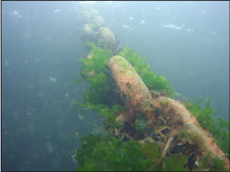
Photograph 10 : Underwater View of the Typical Marine Growth on the Anchor Chain.
