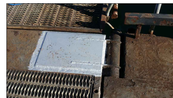
PHOTO 9 EXTERIOR WALKWAY HINGE CONNECTION
