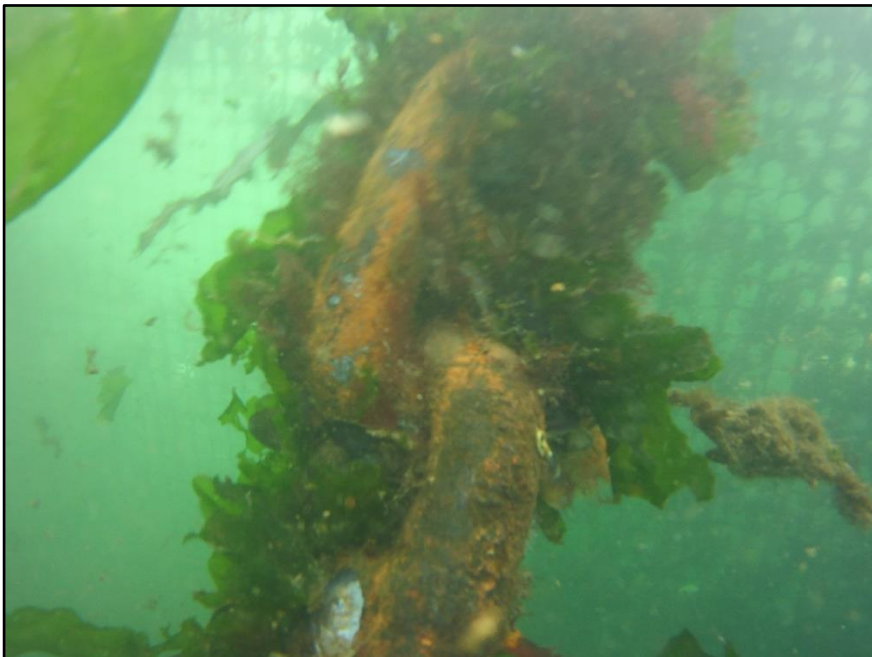
Photograph 12 : Underwater View of the Typical Surface Corrosion on the Anchor Chain.
