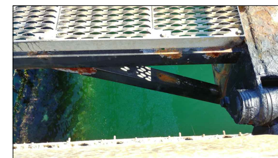
PHOTO 10 GRATING AND PREDATOR NET RAIL SUPPORTS
