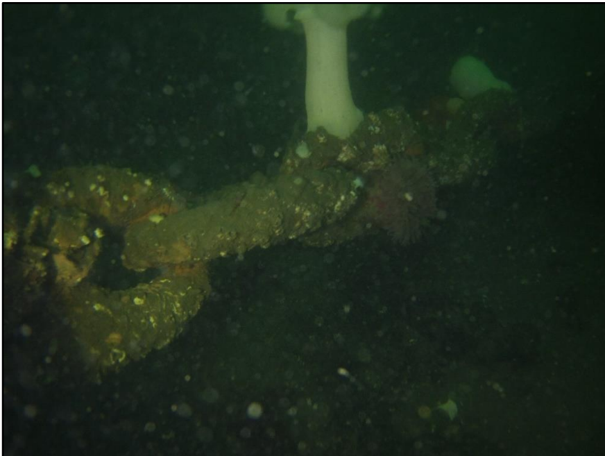
Photograph 14 : Underwater View of the Typical Condition of the Anchor Chain at the Channel Bottom.
