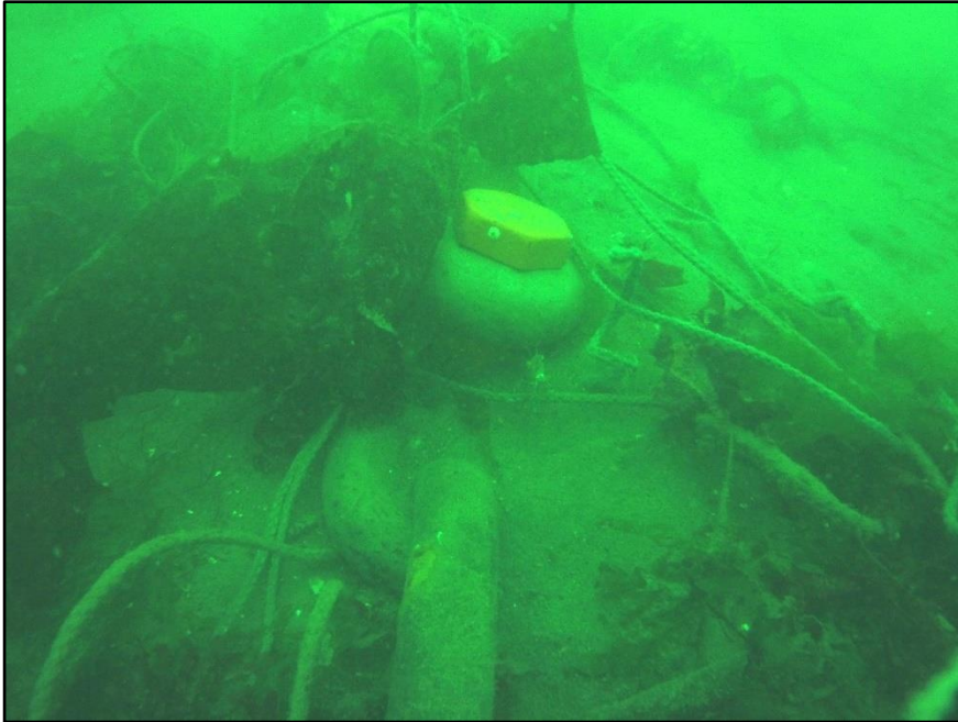
Photograph 19 : Underwater View of the Typical Buried Anchor Exposure.
