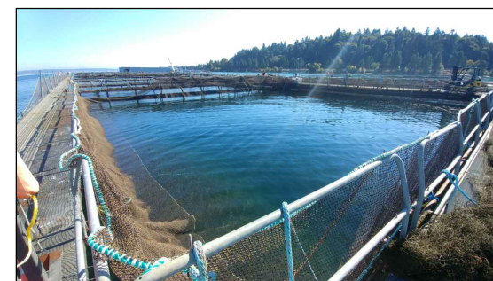
PHOTO 4 NET PEN DURING NET INSTALLATION
